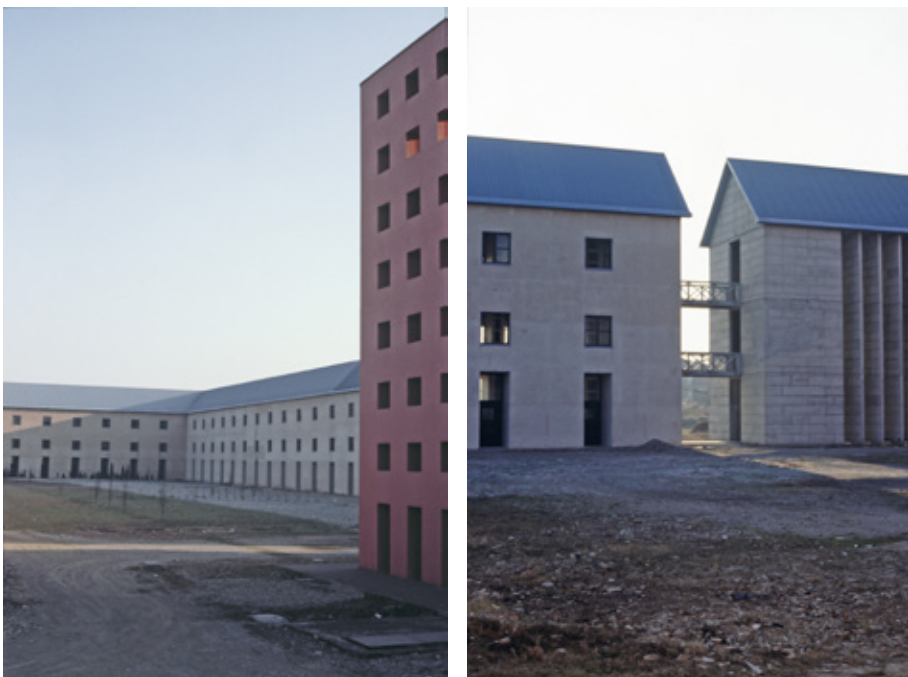
Figure 1 (left). Aldo Rossi, San Cataldo Cemetery, Modena, Italy, Ossuary and Perimetral building. Photo by the author.
