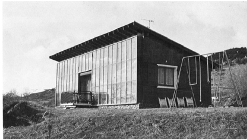
Figure 1. Experimental house equipped with a Trombe wall, Odeillo (France), 1967. Source: Detail.
