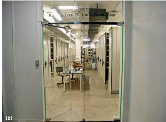
Installed environmental management system at the Goeldi Museum's new storage facility: an exterior brick shelter for supply air fans, seen from the west (a); in the storeroom (as seen from the entrance vestibule), two ceiling-mounted central supply air ducts and, underneath them, the compact shelving (b); and an exhaust duct and dehumidifier (c). Photos: Shin Maekawa. © J. Paul Getty Trust.
