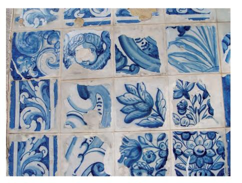
a permeable material, and when ambient humidity falls below the critical humidity value, the expansive recrystallization of the salt within the pores of a material or between materials, such as a coating and a substrate, can result in material rupture or delamination, blistering, and the flaking of finishes (fig. 2.6). In hot and humid climates, the typical ranges of ambient humidity generally span the critical humidity values for common salt compounds.
