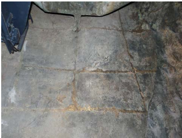
Figure 2.7. Statue of Bavaria. Detail of the interior: edges of the core's sections visible in the area under the armpit of the left arm Image: © Ursula Vedder
