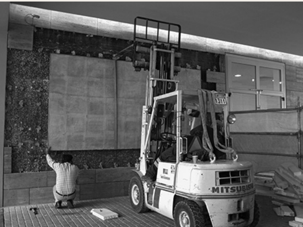
Figure 4 Mounting of the panel. Copyright © Lithou Sintirissis Inc.
