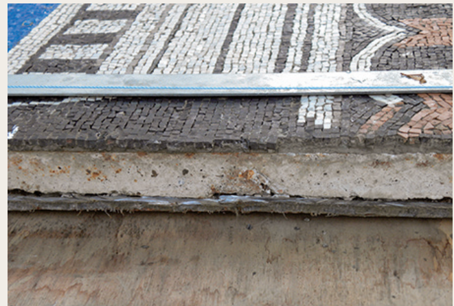
Figure 1 Cross section of the panel. Copyright © Lithou Sintirissis Inc.
