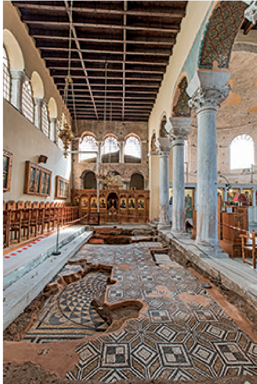
Figure 6 The three layers of flooring from the Roman bath (second to fourth centuries) under the north aisle. Photo: Courtesy Ephorate of Byzantine Antiquities of Thessaloniki
