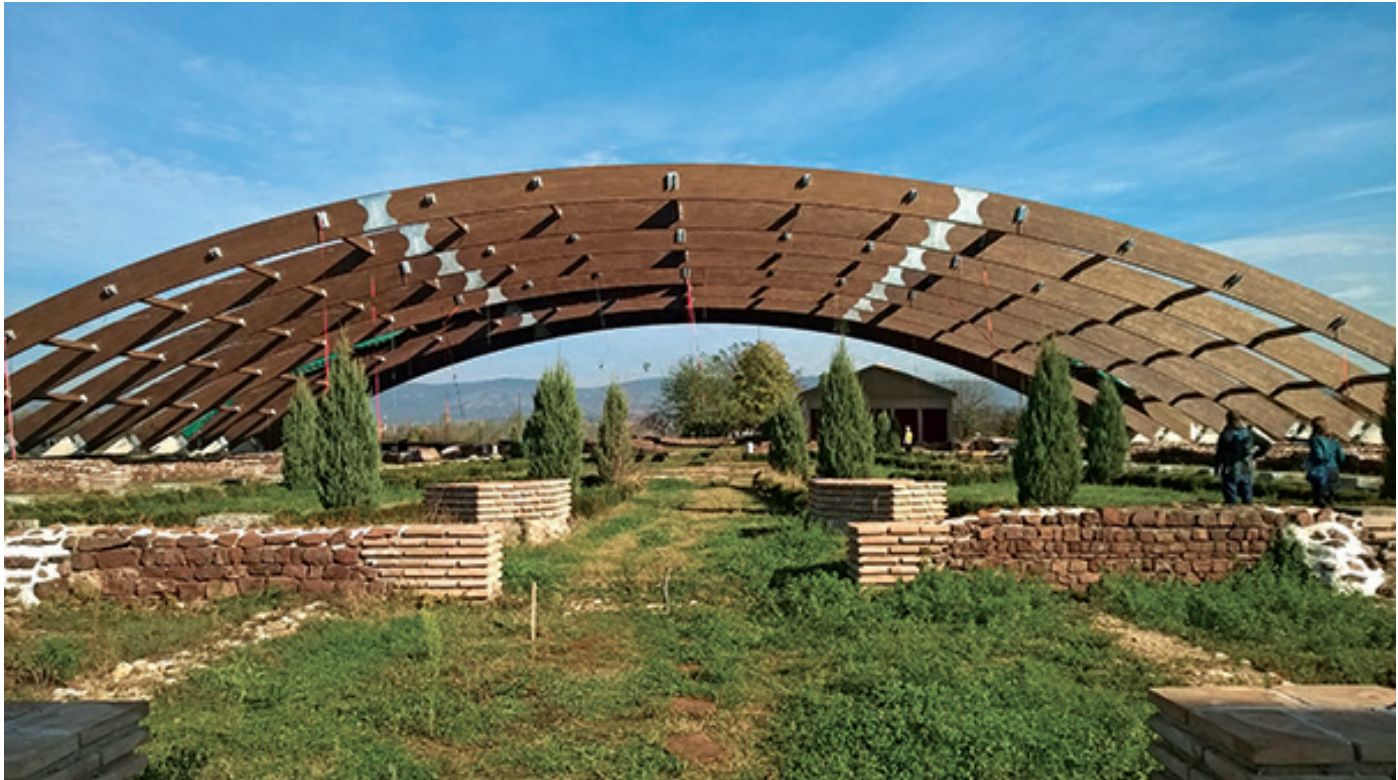
Figure 8 The shelter at the end of 2014; work in progress.
