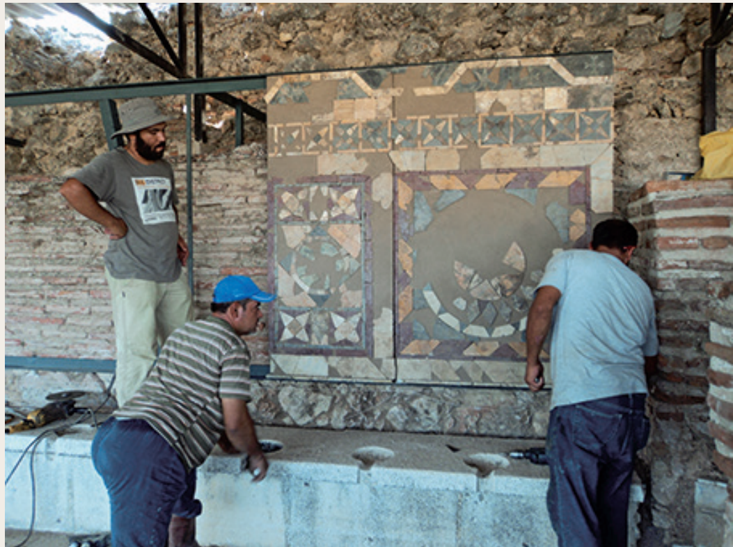
Figure 4 Mounting the opus sectile panels in place, 2012. Photo: Orhan Bingöl
