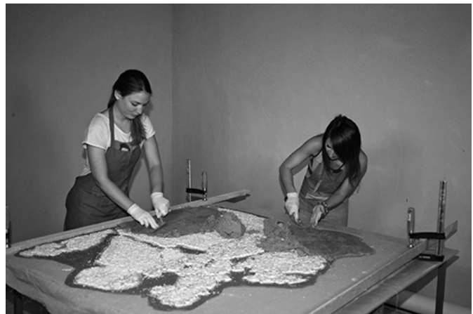
Figure 6 Application of the first layer of lightweight mortar with mineral additives. Photo: Documentation RC ZVDKS
