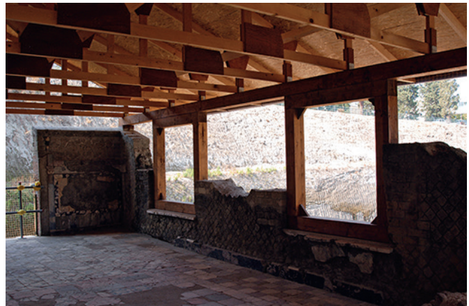
Figure 5 Temporary shelter over the triclinium of the House of Telephus at Herculaneum. Photo: Gionata Rizzi
