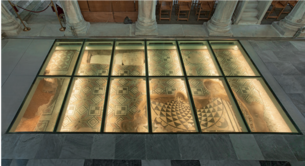
Figure 7 Walk-on glass installed over the exposed flooring of the Roman bath. Photo: Courtesy Ephorate of Byzantine Antiquities of Thessaloniki
