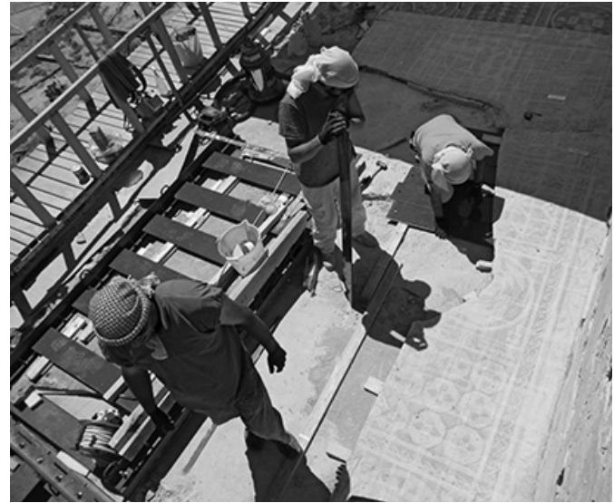
Figure 4 Dismantling phase of the panels: insertion of galvanized iron strips to facilitate the dismantling, lifting, and transport of the mosaic. Photo: ISCR Archive
