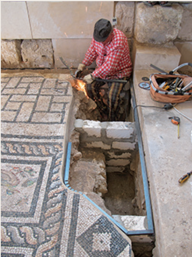
Figure 3 Placement of metal grills over the trenches around mosaic edges. Photo: E. Parandowska
