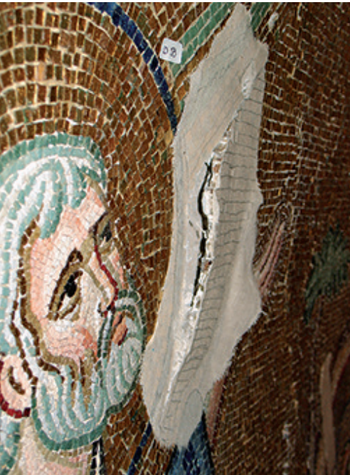
Figure 2 Bulge in the mosaic surface after the earthquake. Photo: © Hellenic Ministry of Culture and Sports
