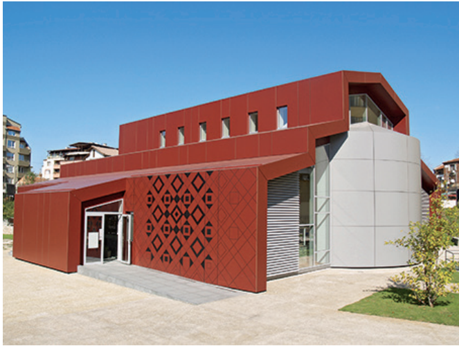
Figure 7 The protective building of the site seen from the exterior.
