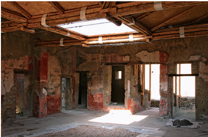
Figure 4 Temporary shelter over the atrium of the House of the Gemma at Herculaneum. Photo: Gionata Rizzi
