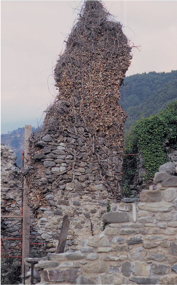
Figure 8.2 After the plant has been killed. The removal or rotting of the roots can still cause serious damage to the masonry and may lead to its collapse.
