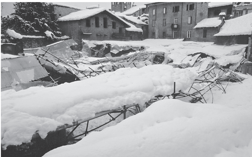
Figure 6.2 A poorly conceived and implemented shelter of corrugated roofing and scaffolding. A medium-intensity snowfall (25 cm in a 24-hour period, the same as that featured in fig. 6.3) caused its total collapse. The same materials and “modular” construction were used for both shelters (slope of the roof, distance between vertical supports). If this proved sufficient to protect the vertical structure featured in figure 6.3, the failure of the same for the greater horizontal area of the first shelter indicates that the roof needed a much steeper slope or that the spacing between vertical support elements needed to be much reduced.
