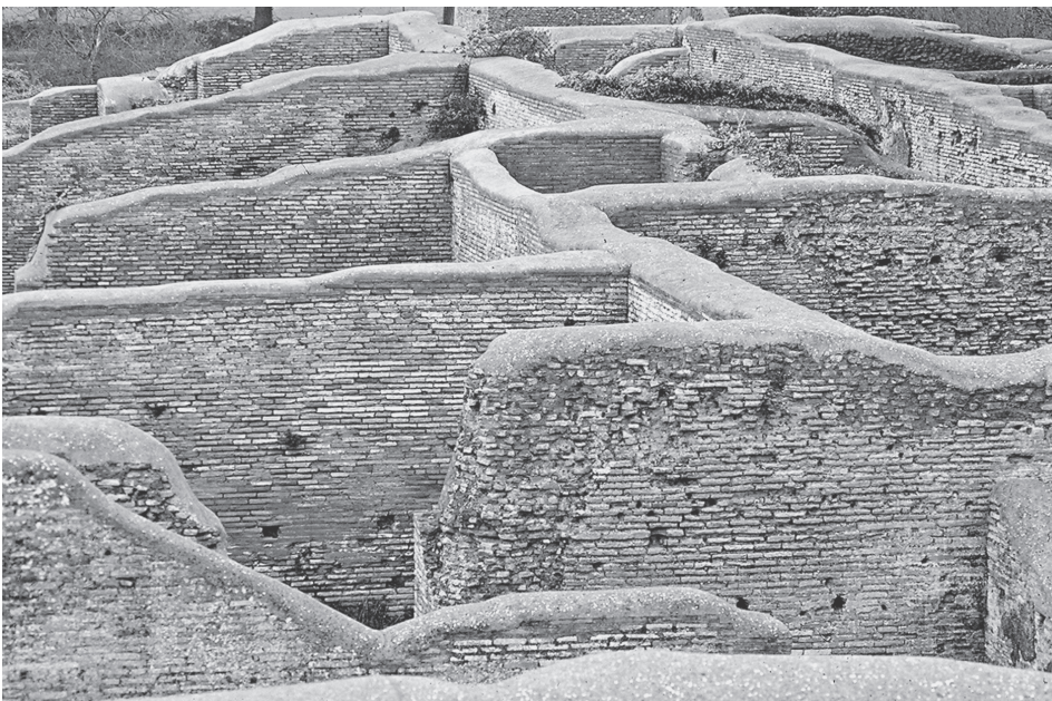
Figure 16.6 Ostia Antica. Typical mortar capping from the 1950s. Protection is ensured at the expense of the visual impact and legibility of the ruins.
