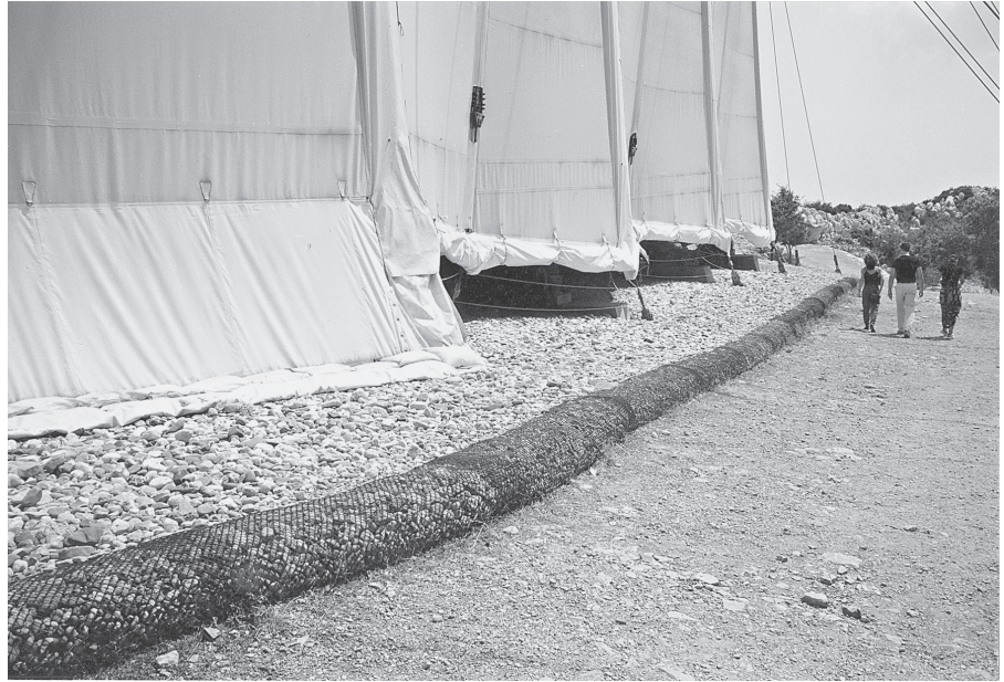
Figure 16.2 Vassos, Arcadia, Greece. Detail of the gravel drainage and its system of containment. Note that the lower part of the protective shelter can be raised to allow for the circulation of air during the hottest periods of the day.
