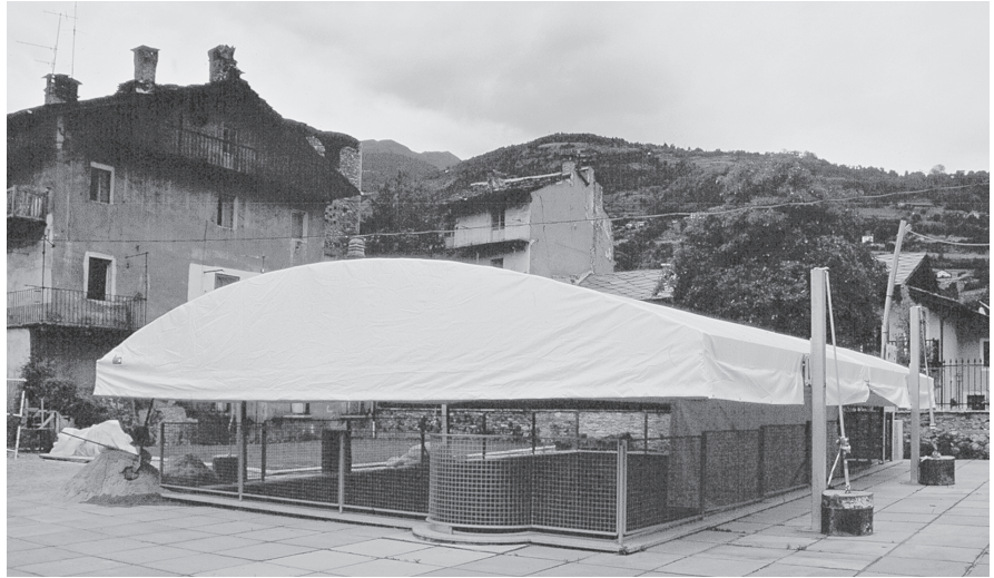
Figure 6.6 A mobile shelter for the temporary protection of areas under excavation in the urban center of Aosta.
