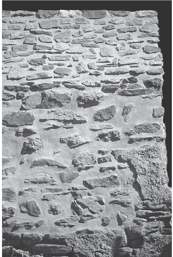
Figure 16.7 Castle of Cly (Valle d’Aosta). Detail of a battlement merlon. The upper portion was re-created with rubble stones that were smaller in size than the original stones. At the lower level, gaps between the original stones were repointed.
