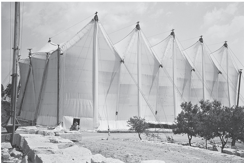
Figure 16.1 Vassos, Arcadia, Greece. Protective shelter for a Hellenistic temple situated in difficult climatic conditions (temperature fluctuations of up to 60°C between summer and winter). The remote and inaccessible nature of the site and the frequency of rain were the factors justifying this type of intervention, prioritizing conservation over some aesthetic elements, such as the relationship between the temple and the landscape.
