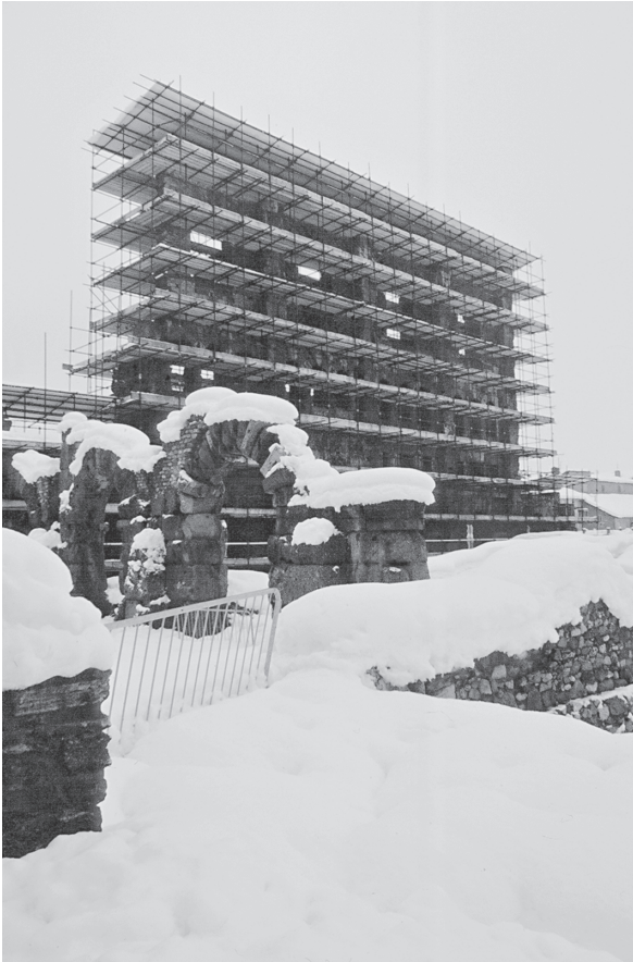
Figure 6.3 A protective shelter properly constructed. The slope of the roof is appropriate for the horizontal area covered, allowing for the progressive discharge of precipitation, even in the event of snow.
