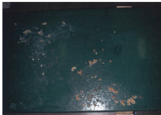
FIGURE 7B Detail of figure 7A showing corrosion.
