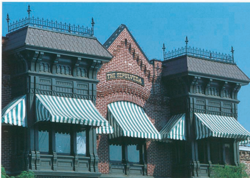
The facade of the Sepúlveda House, before and after restoration.
