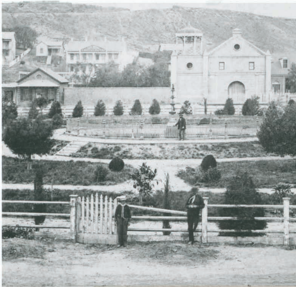
The Plaza, Los Angeles, ca. 1880. The view is from the second floor of the Lugo House. To the left of the Plaza Church is the adobe of Andrés Pico; Fort Moore Hill, an early Los Angeles landmark, rises in the background. Carleton Watkins, albumen stereograph.
