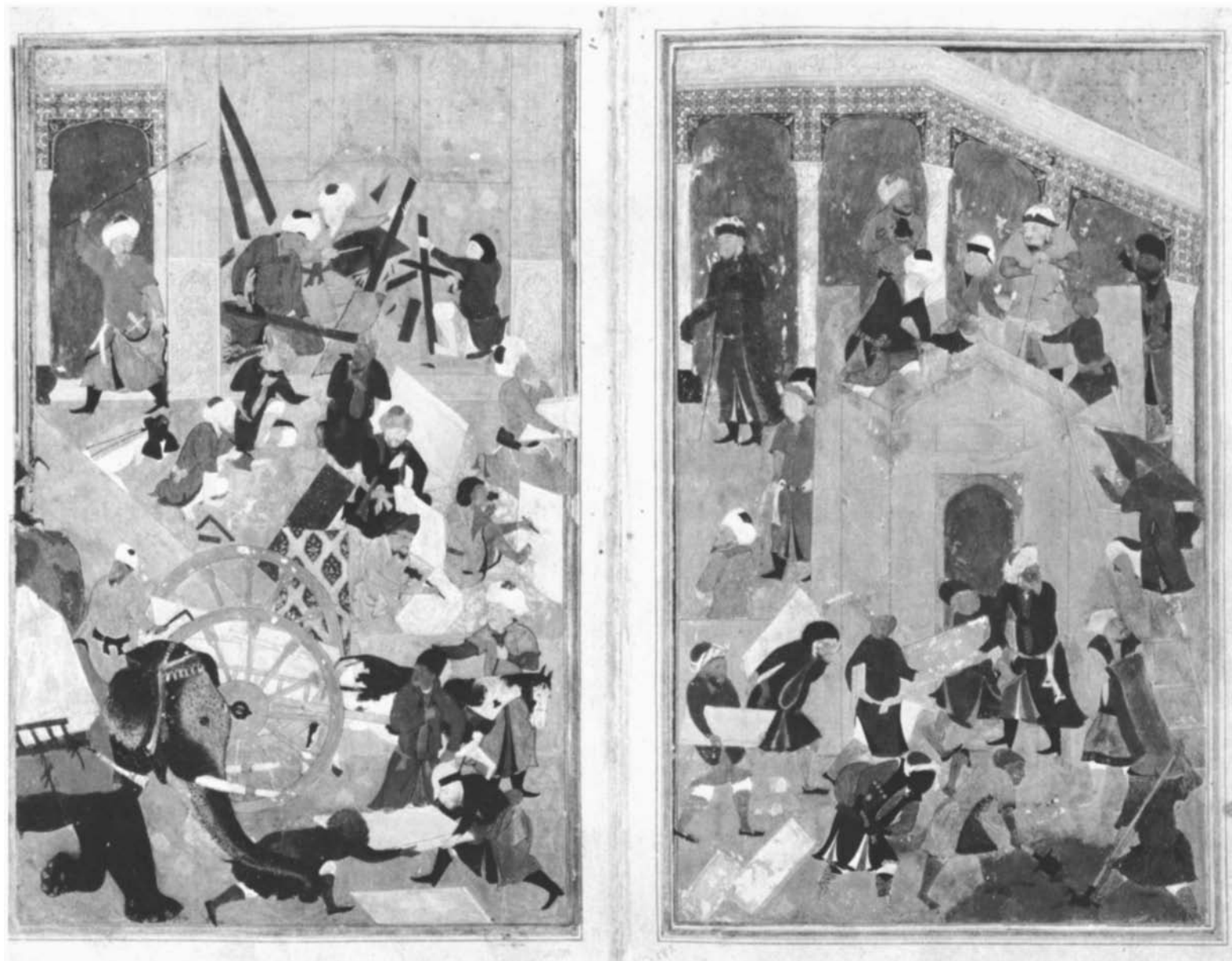
77. Construction of the Masjid-i Jami' of Timur in Samarqand, double-page miniature painting. From Sharaf al-Din 'Ali Yazdi, Zafarnāma (Book of victories), ca. 1467. Baltimore, The Johns Hopkins University, John Work Garrett Library, fols. 359v, 360r.
