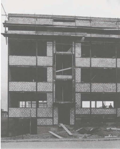
**Fig. 42. The IRON SKELETON as HOUSING FORM. 1927. Apartment block of the Stuttgart Werkbundsiedlung by Mies van der Rohe. 1927**
