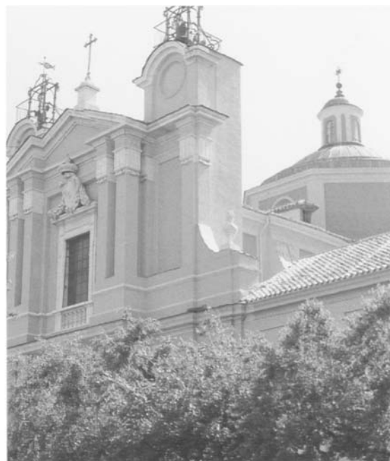
FIGURE H Facade of the Church of San Pascual Baylon, Aranjuez, Spain. Photo: Madrid, Patrimonio Nacional.
