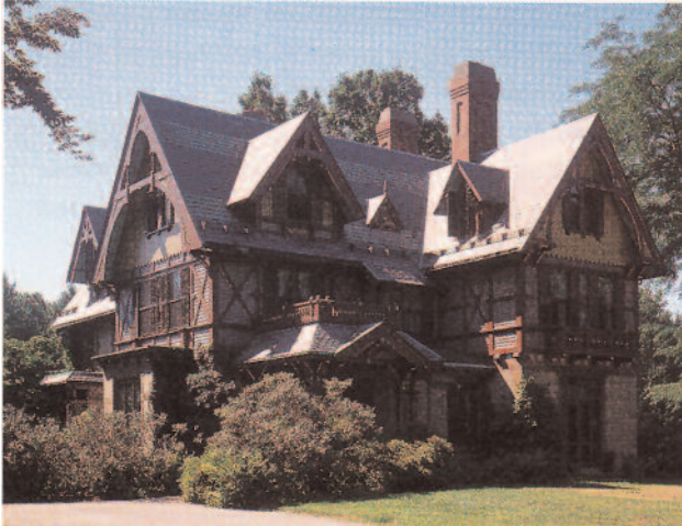
Figure 3 Hunnewell cottage, 1995. Original paint scheme re-created.
