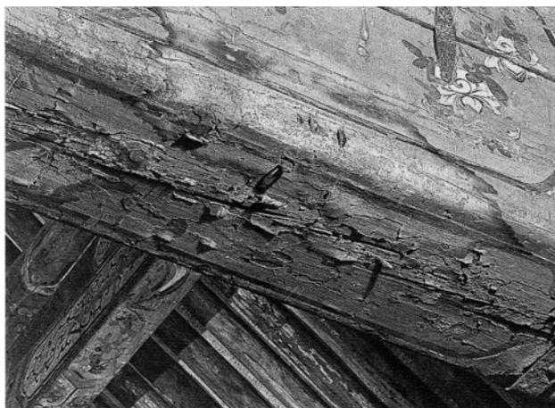
The test areas were evaluated at intervals of one month and two years by assessing adhesion of the paint to the wood and visible alterations to the surface quality of the paint. Change in saturation of color or the matte quality of the paint was undesirable. It was found that many of the adhesives stained the wood and saturated the color, especially the layer of blue-dyed calcite and lead white.
