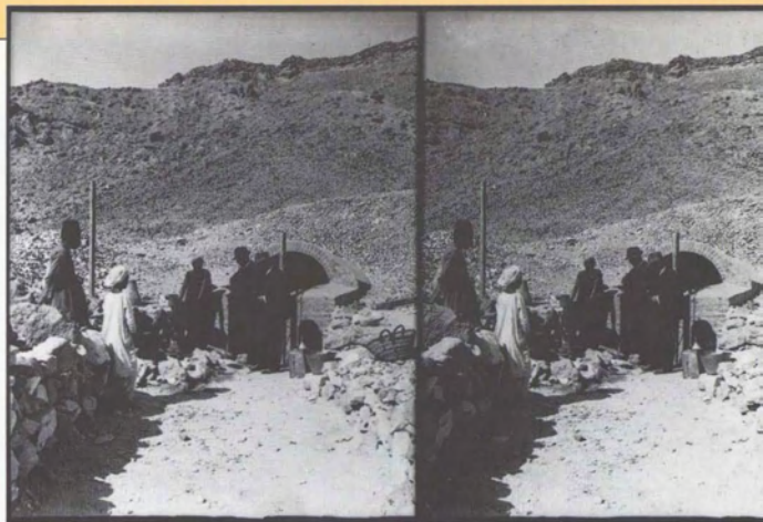
Stereo view of Ernesto Schiaparelli (far right) at the entrance to the tomb of Nefertari after construction of the brick portal.
