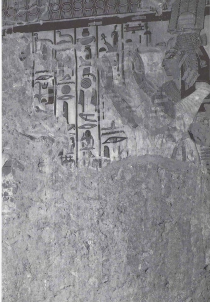
Chamber K, east side of the south wall, showing the deterioration that occurred between 1904 (opposite) and 1989.
