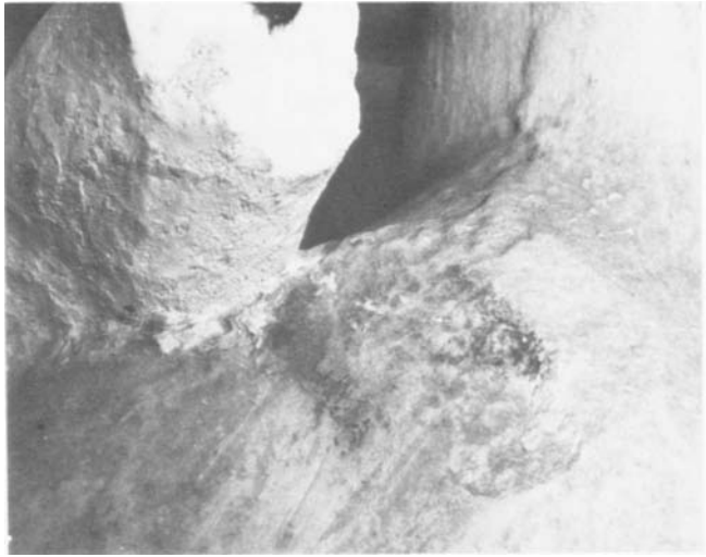
35 Left shoulder before conservation, showing damaged and trimmed surface, grain of marble exposed by weathering, and deteriorated eighteenth century club end
