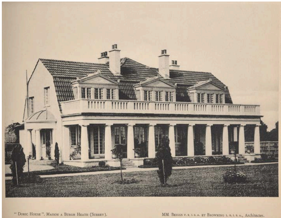
FIG. 13. — “Doric House,” Furze Hill, Surrey, constructed in 1912, from Charles Massin, Villas Normandes & Anglaises (Paris: s.n., 1913), pl. 2.
