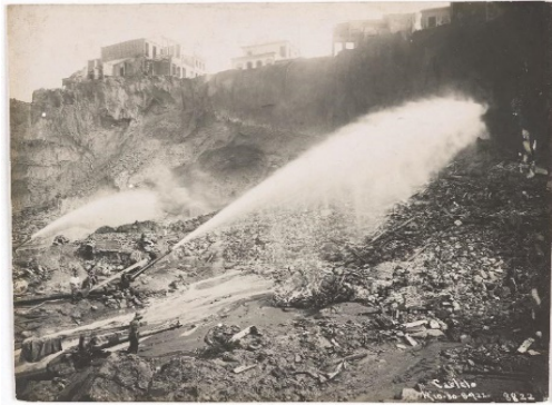
Castelo hill demolition with water jets, view taken from Santa Casa de Misericórdia. Photograph taken by Augusto Malta in 1922. Courtesy Instituto Moreira Salles
