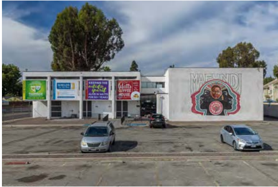
1. Mafundi Building, built 1969, Watts, architects Robert Kennard and Arthur Silvers. Photo: Stephen Schafer, © 2020 schafphoto.com. Founded in the wake of the 1965 Watts rebellion as an arts education center devoted to community empowerment, the Mafundi Institute (also known as the Watts Happening Cultural Center) was housed in this building from 1969 to 1975.
