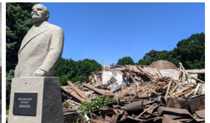
[pic.2] Demolition of Penza planetarium in 2021. Photographer sergeykaldyrkaev. From Wikipedia archive.
