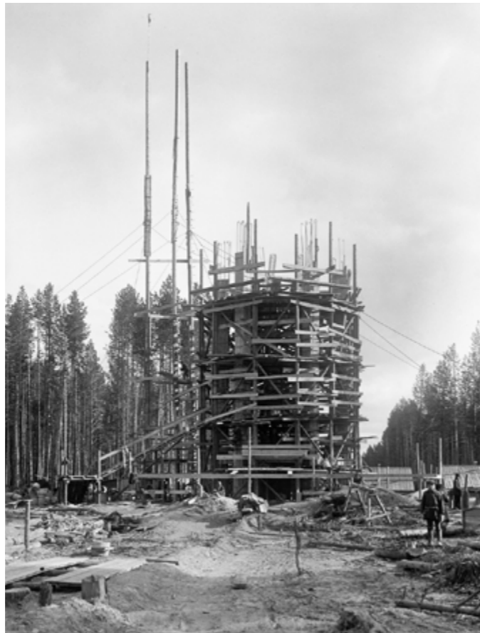
[pic.37] Construction of the load-bearing frame started. Autumn 1930. Photographer N. Tatarchenko.
