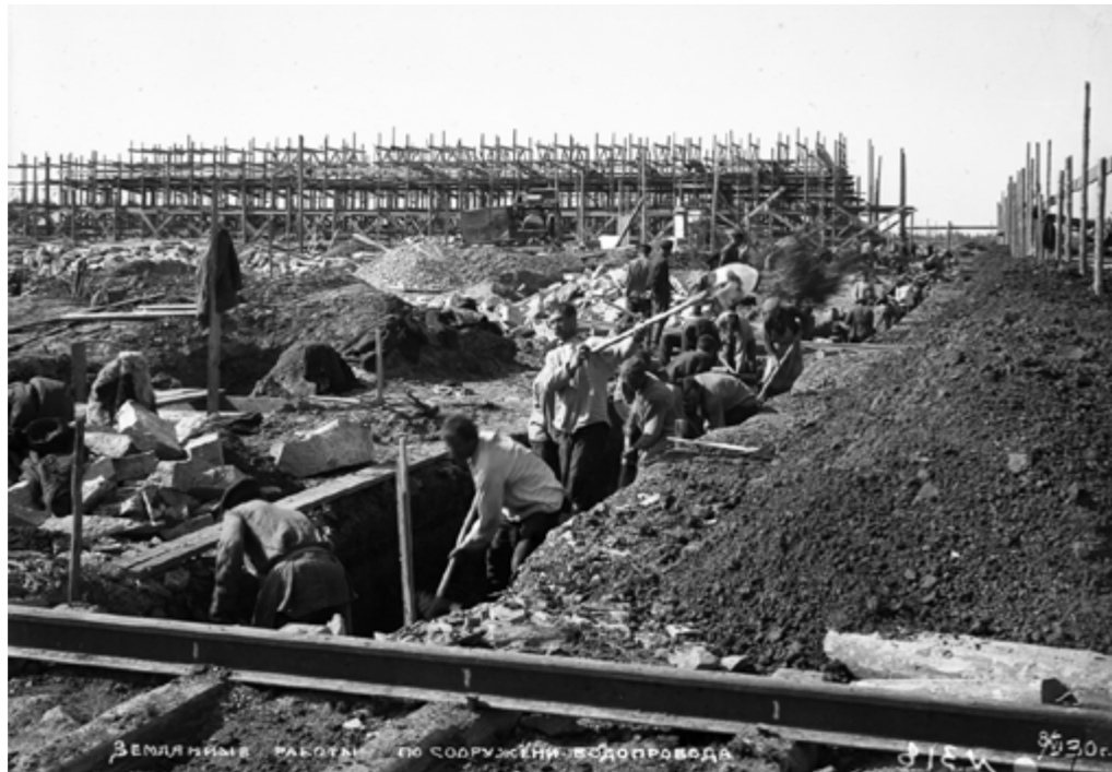
[pic.11] Construction of a water pipeline. June 8, 1930. Photo from the UZTM History Museum photo archive.
