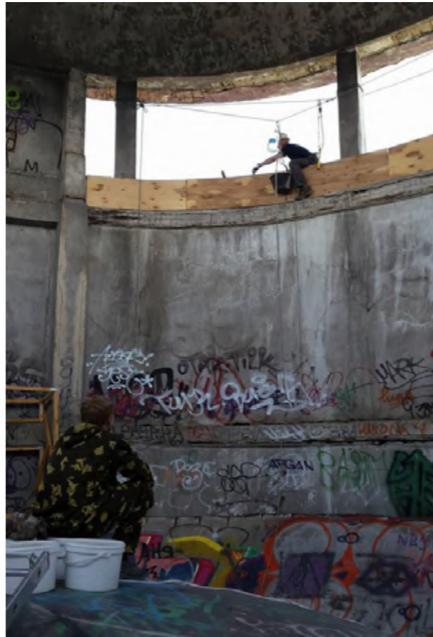
[pic.8] Emergency work in the tank. Photo taken for author's supervision. From the archives of the arch-group Podelniki.
