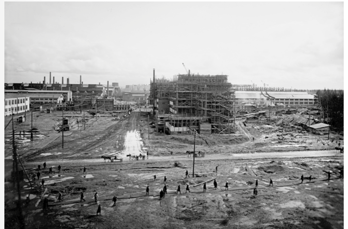
[pic.12] Panoramic view of the construction of the plant and buildings on Pervoi Pyatiletki Square. Photo from the photo archive of the UZTM History Museum.
