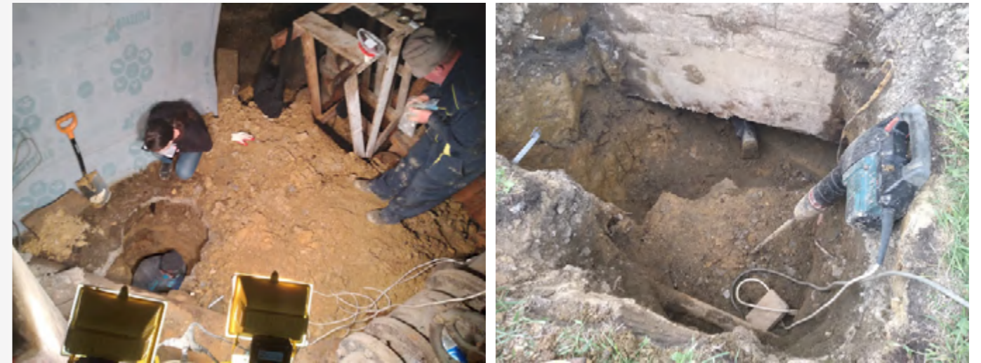
[pic.24–25] May 14th, 2021. Excavation under the foundation slab of the basement and under the foundation outside.
