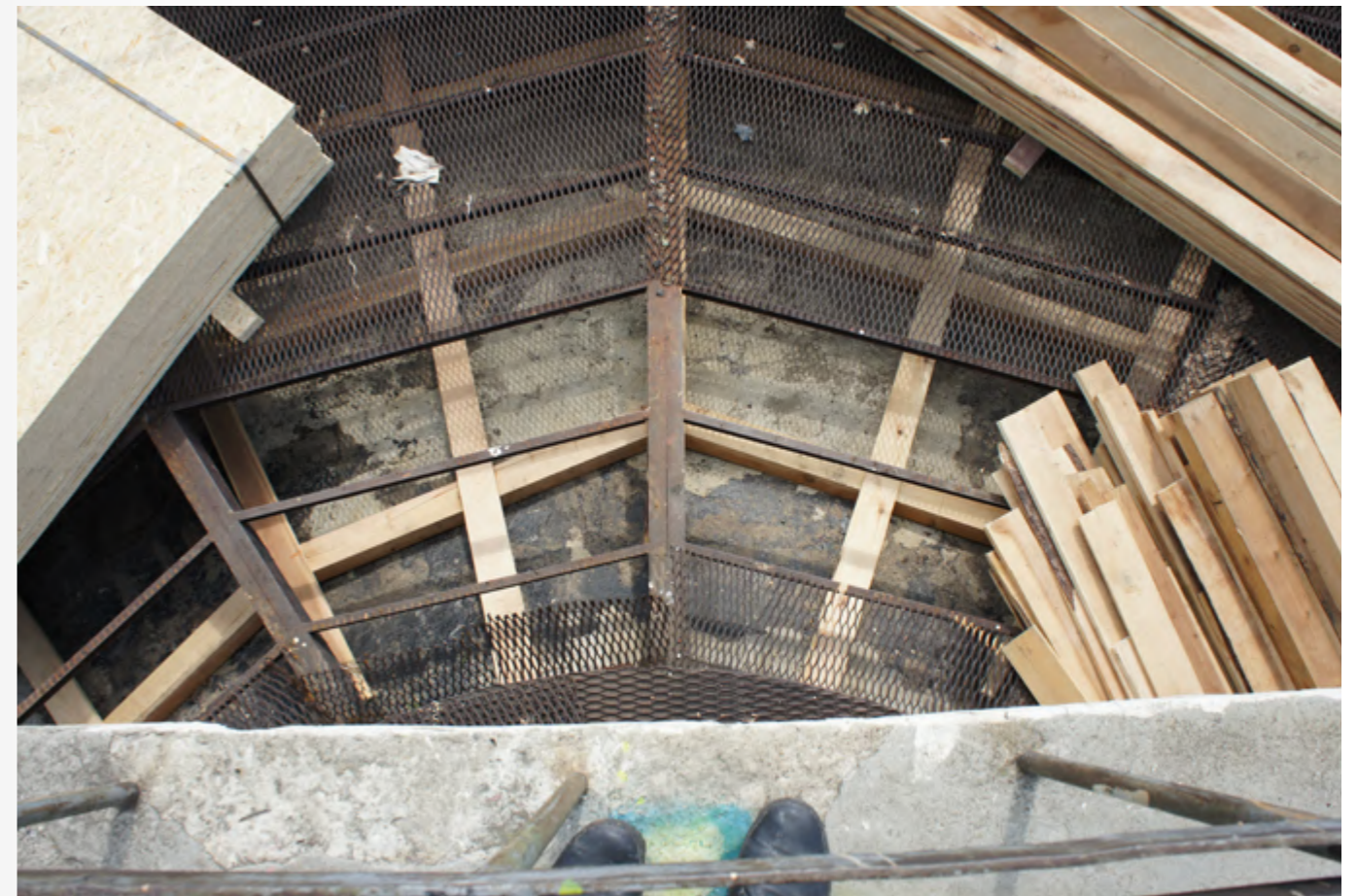
[pic.10] Photo of the additional OSB structure for waterproofing the dome above the tank. Photo taken for author's supervision. From the archives of the arch-group Podelniki.
