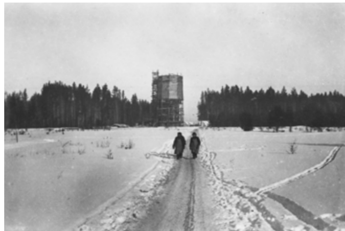
[pic.38] Construction of the tower in the winter of 1930–31. Photographer N. Tatarchenko.
