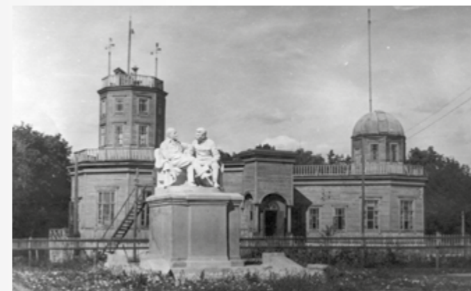
[pic.1] Planetarium in Penza. Built in 1928. Photographer V. Shelyapin. From Wikipedia archive.
