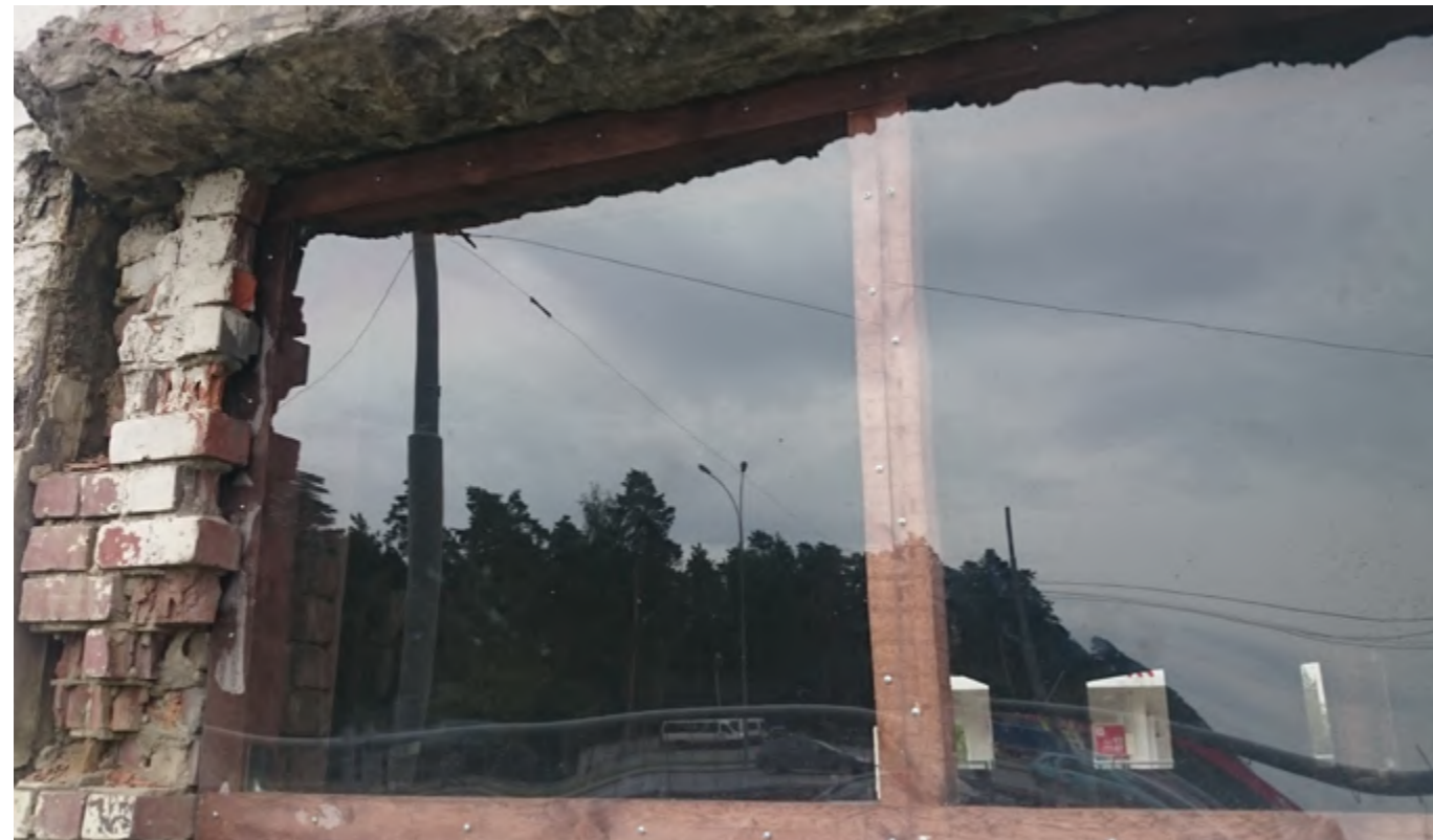
[pic.9] Sealing window openings with temporary structures - wooden frames and cast polycarbonate. Photo taken for author's supervision. From the archive of the arch-group Podelniki.
