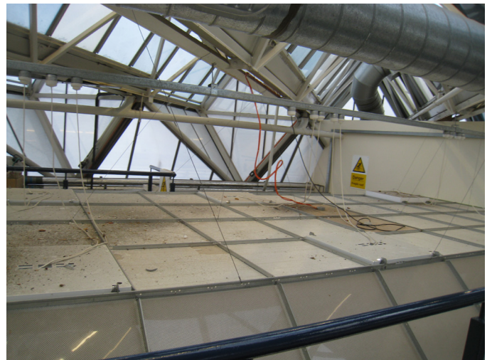
108. False ceiling in S-Block: unusable space obscuring views of the roof
