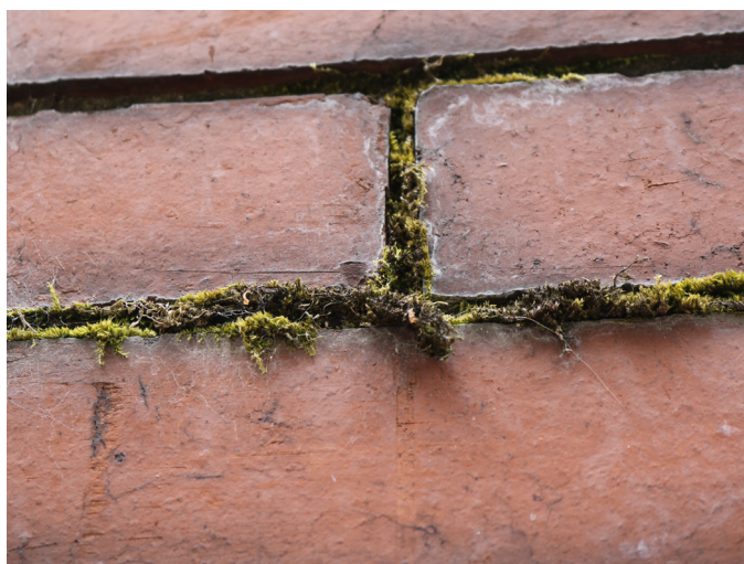
100. Moss growing in recessed brickwork joints
