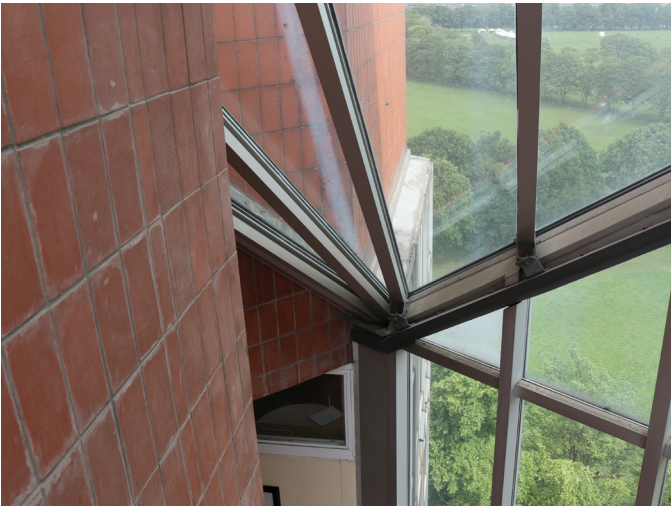
95. Stained tiles, coarse glazing details, dirty glazing
