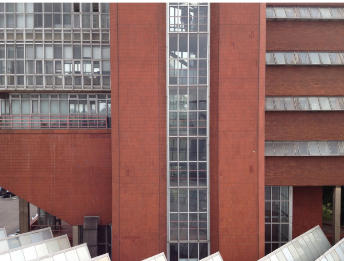
42. Tiled and brick cladding to the tower ensemble
