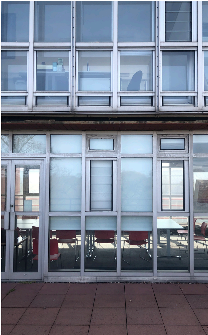
98. Heavy framing elements in 1980s tower glazing
