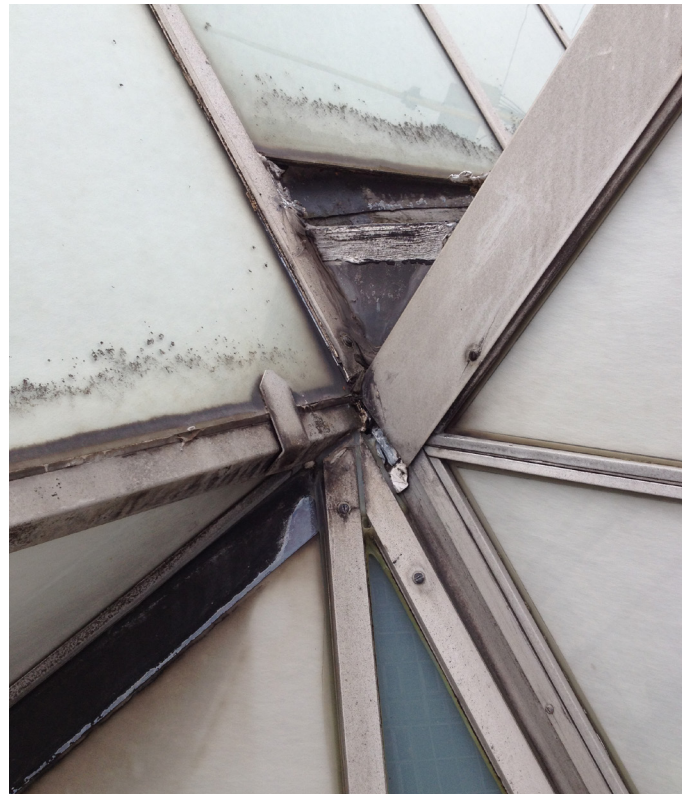
48. Gutter end node in 2012, with 1980s restraint clip
