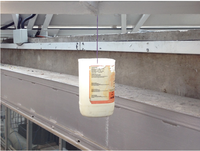
70. 'Bucket' in workshop to catch water dripping through roof, 2013
