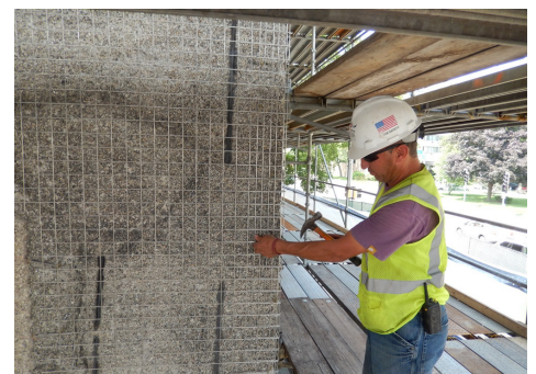
Figure 11. Installation of mesh reinforcement to control shrinkage. (Harboe Architects)
