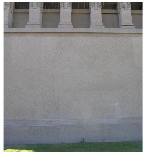
Figure 4. Halos around repaired shotcrete were resolved with modification in the facade cleaning treatment. (Harboe Architects)
