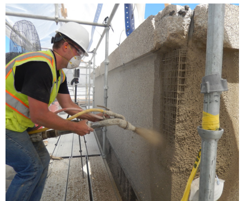
Figure 7. The shotcrete patch was cut-out and re-patched with a mix design that worked for both colors of existing shotcrete. (Harboe Architects)
