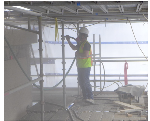
Figure 8. The shotcrete aggregate was exposed utilizing abrasive blasting. (Harboe Architects)
