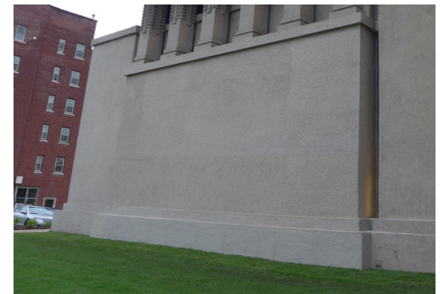
Figure 10. Rejected shotcrete patches at the north elevation were cut-out and are re-patched with a revised mix to provide a closer match. (Harboe Architects)
