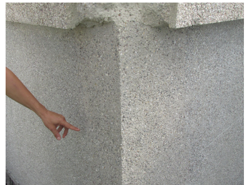
Figure 6. Shotcrete at corner with two different colors of 1974 shotcrete. Our new patch matched the material on the right but not the left. The mix on the right was accepted for local shotcrete repairs. (Harboe Architects)
