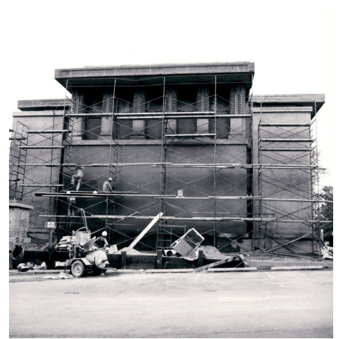
Figure 2. 1974 photo of shotcrete application. (UTP LLC)
