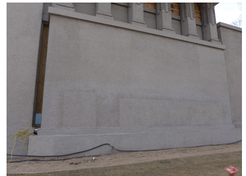
Figure 9. Rejected shotcrete patches at the north elevation. (Harboe Architects)
