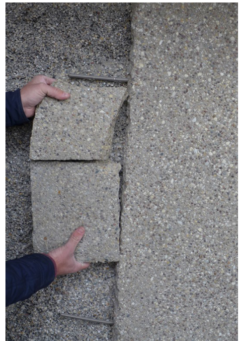
Figure 5. Selecting custom shotcrete mixes for repairs. (Harboe Architects)
