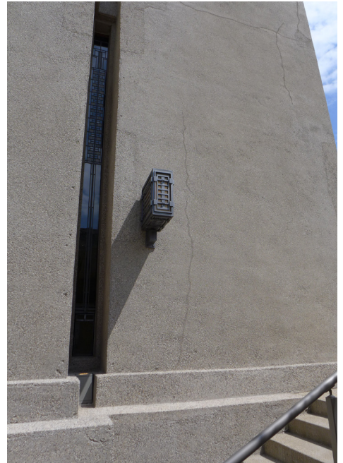
Figure 12. Rejected crack repair. (Harboe Architects)
