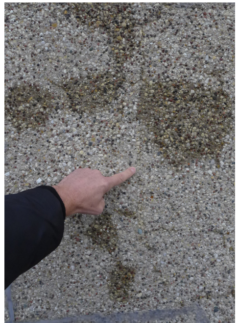
Figure 13 The rejected crack repairs were cut-out and the cracks were re-patched to more closely match the approved mock-up sample. (Harboe Architects)
