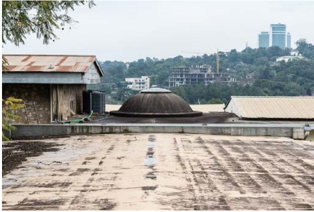
Figure 85 –The flat roof over the Education Wing
