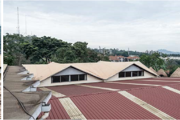
Figure 86 –The metal roof over the Car Gallery looking to the Science and Industry Gallery
