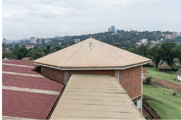
Figure 91 –the sloped metal roof connecting the Natural History
