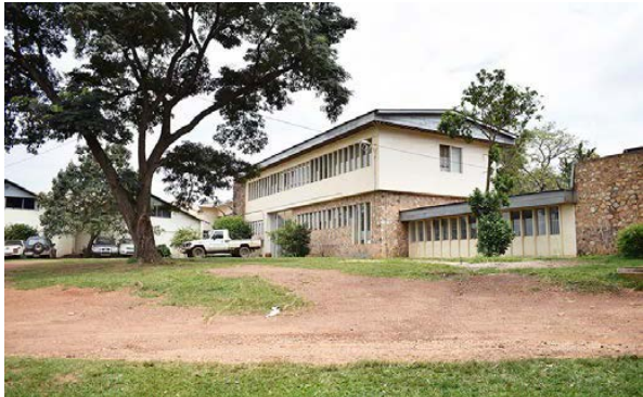
Figure 64 – Soil erosion at the front of the museum by the stores
