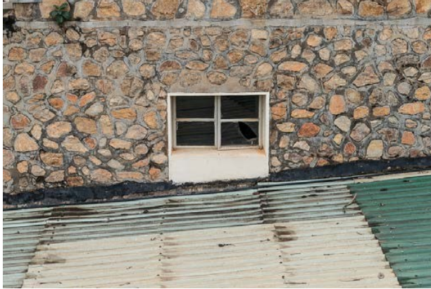
Figure 92 –given the numerous extensions, roofing is a major challenge
