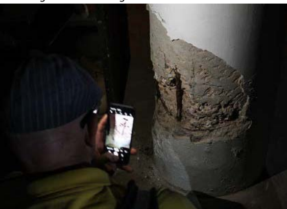
Figure 71 – Destructive concrete tests in the basement
