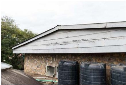
Figure 121 – Plastic water tanks on roof
