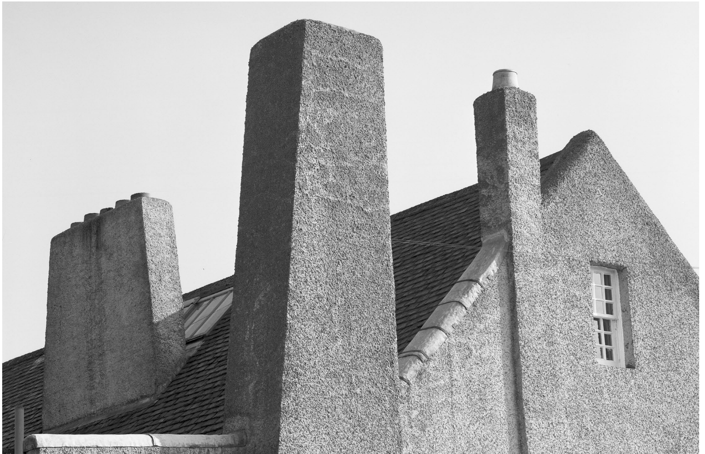
62 RCAHMS 1973 showing Wallhead repair work carried out by Margaret Brodie
