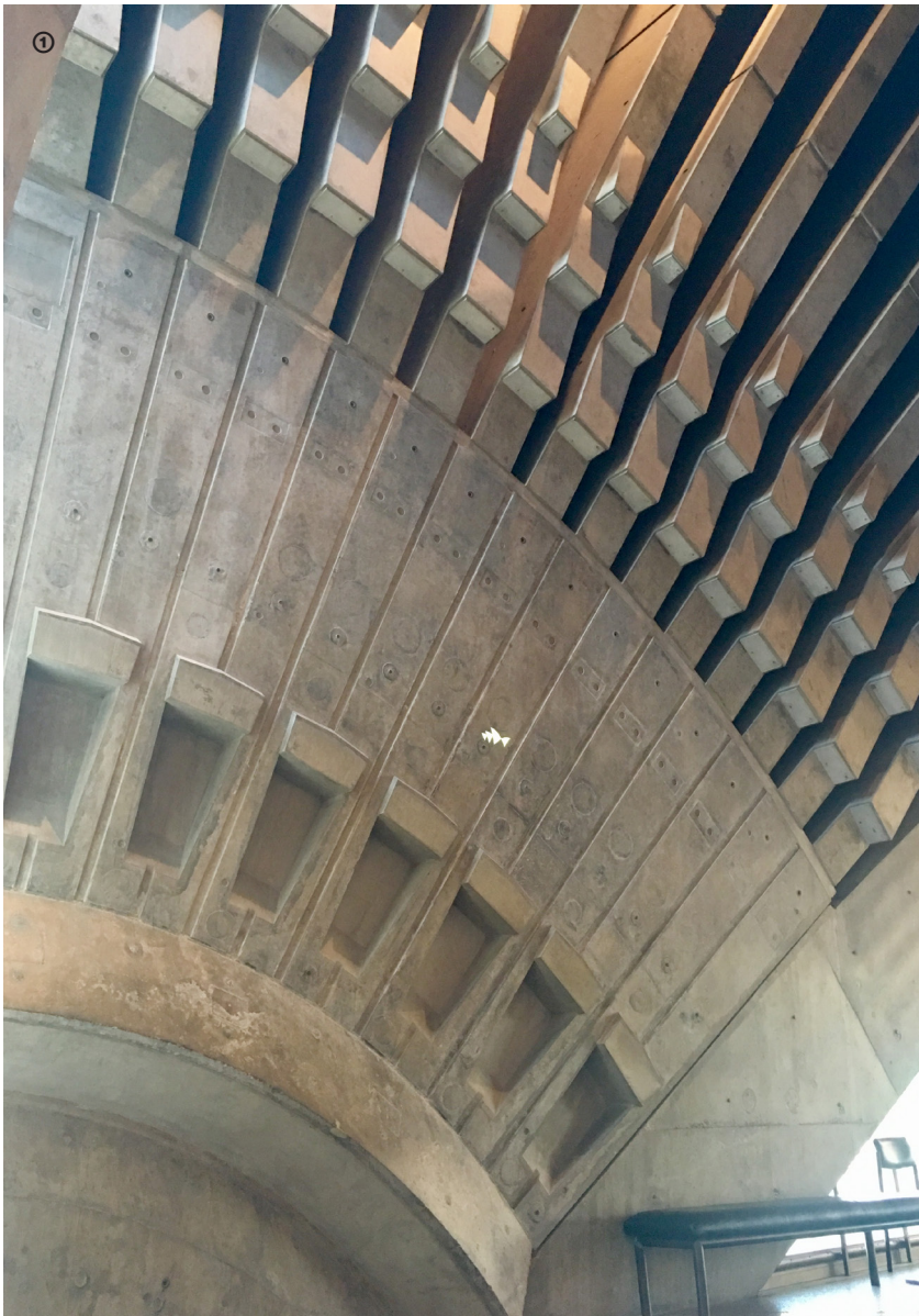
① In-situ concrete pedestal
