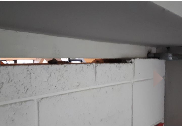
Air Gap between Wall & Beam
