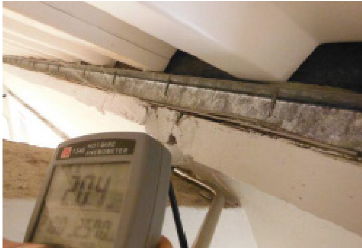
8. Leakage to Hall (F4) Large gap identified at top of blockwork wall in F4.
