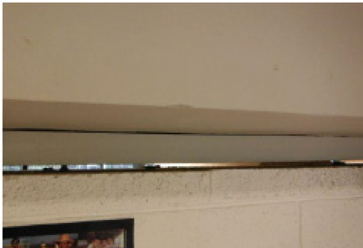
8. Leakage to Hall (F4) Large gap identified at top of blockwork wall in F4.
