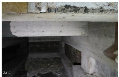
Figure 23 a/d - Views of the basement of the additions, seen from the east curved wing: a) and b) structural elements ( $\bigcirc$ Liberatore 2020); c) detail of the junction between a beam of the addition and one of the curved wing ( $\bigcirc$  Martella 2020); d) junction detail between a beam of the addition and the wall of the wing ( $\bigcirc$  Liberatore 2020)
