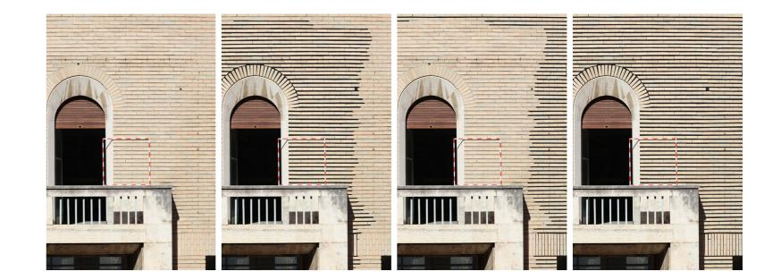
Figure 15/16 - Identification of the area of Litoceramic cladding characterized by mortar of different colours; graphic representation (© Santarelli, Giorgi, Ciacchella, Pandolfi 2020)
