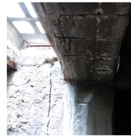
Figure 4 a/d - East curved wing, basement level: a) bars oxidation, spalling of concrete, cracks in the masonry wall (© Martella 2020); b) bars oxidation, spalling of concrete, cracks in the masonry wall (© Martella 2020); c) oxidation of stirrups and longitudinal bars and consequent spalling (© Liberatore 2020); d) oxidation of stirrups due to reduced concrete cover especially at the lower side corners (© Martella 2020).
