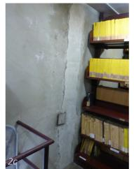
Figure 2 a/d - Front building, book deposit at the third level of the library: a) smeared cracks on the surfaces close to the skylight (© Martella 2020); b) smeared cracks, vertical and horizontal cracks on the beam intrados (© Liberatore 2020); c) inhomogeneity due to interventions on installations (© Liberatore 2020); d) damage due to the interaction with the steel slab (© Liberatore 2020)
