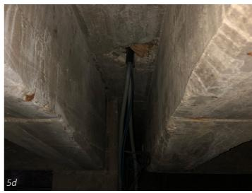
Figure 5 a/f - East curved wing, basement level: a) pipes hanging on longitudinal reinforcements (© Liberatore 2020); b) stirrup oxidation, pipes hanging on longitudinal reinforcements (© Liberatore 2020); c) stirrup oxidation, pipes hanging on longitudinal reinforcements (© Martella 2020); d) hole in the reinforced concrete slab for the passage for cables (© Martella 2020); e-f) hole in a reinforced concrete beam for the passage for pipes (© Sorrentino 2020).
