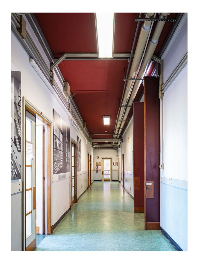
Figure 11 - Front building, first floor, bundling of cables, ducts, and wiring in the office corridor (© Sardo 2021)
