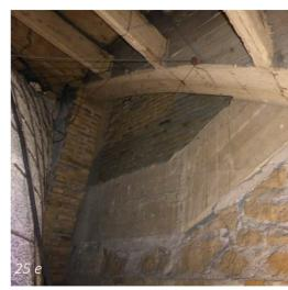
Figure 25 a/f - Different types of masonry built as infill of the reinforced concrete structure: a) room WE\_Bs\_01 (© Martella 2020); b) WE\_Bs\_01 (© Sorrentino 2020); c) room T\_Bs\_01 (© Martella 2020); d) room T\_Tr\_09 (© Martella 2020); e) room T\_Fr\_9 (© Liberatore 2020); f) room T\_Fr\_9 (© Liberatore 2020)
