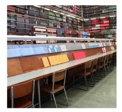
Figure 19 - The reading tables of the library with evidence of subsequent modifications due to the change of the lighting fixtures and of the embedded radiators with fan coils ( $\bigcirc$  Petraroia 2020)
