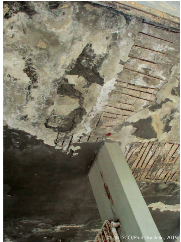
The soffit of the Secondary Entrance has exposed welded-wire mesh and water staining, indicative of the failure of the waterproofing membrane above.
