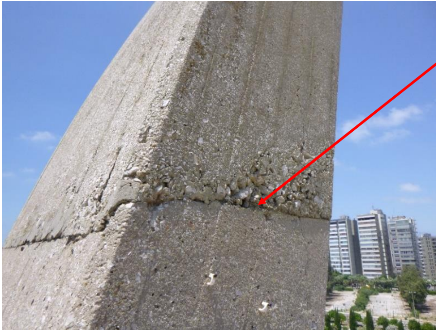
Figure 18. View of placement lift or construction joint in Arch
