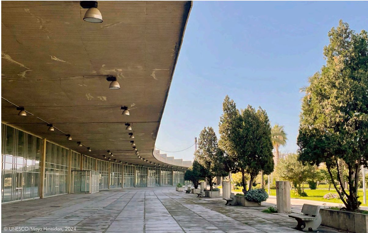
The rehabilitated southern part of the Grand Cover. Notice the added suspended lighting fixtures in the outdoor cantilevered ceiling, as well as the concrete benches, trash bins, and planters in front of the Grand Cover.
