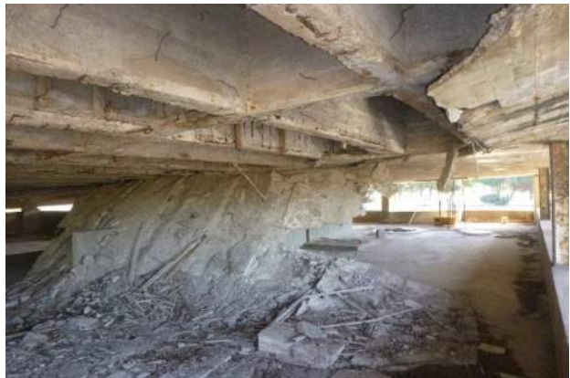
Figure 2. Collapsed soffit slab section that was cored for the studies.
