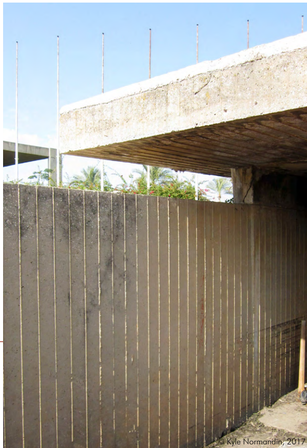
Board-formed exposed concrete wall at the Ticket Booth. This exposed concrete finish along with the brick cladding of the exterior are among the main attributes that define the character of this structure and need to be retained.
