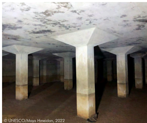
Status of the underground shelters. Most of the structures suffer from flooding and water stagnation.
