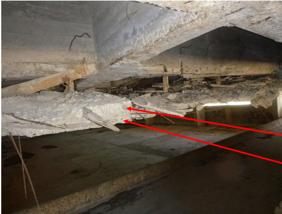
Figure 31. Overpour concrete, likely from placement of the beams, on the top of the soffit slab
