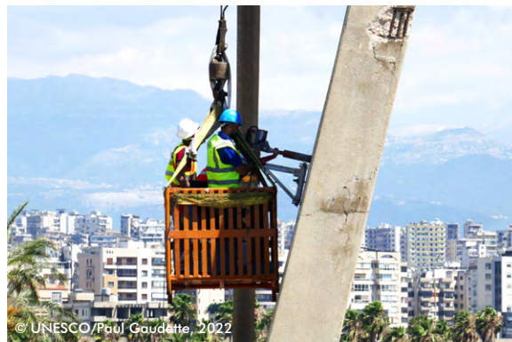
Concrete coring at the Arch.
