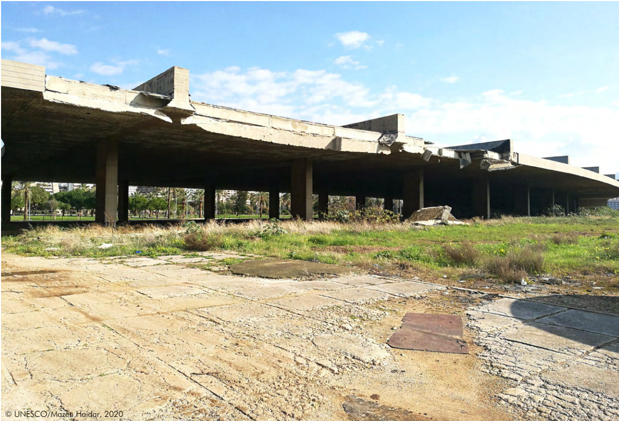
The Grand Cover in 2020, showing the failure of the anchorage for the prefabricated fascia.
