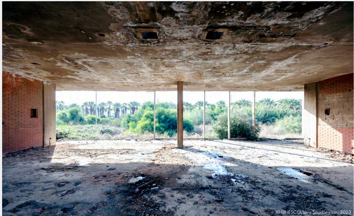
Interior of the Administration Building, looking west. Note the spontaneous vegetation that has overgrown in the site's western boundary and the detached brick cladding to the right of the image on the wall.
