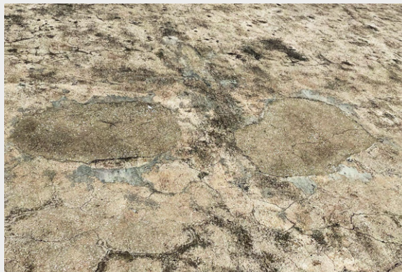
Left Previous repair and concrete patching.
