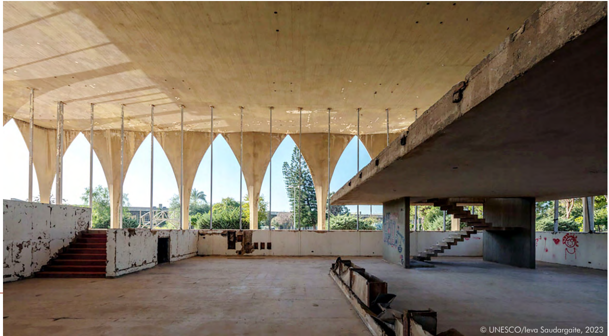
Interior of the Lebanon Pavilion stripped from its linoleum tiles and white marble.
