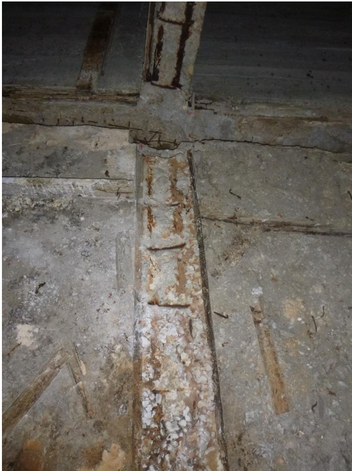
Figure 26. Soffit slab debonded and pulling away from beams
