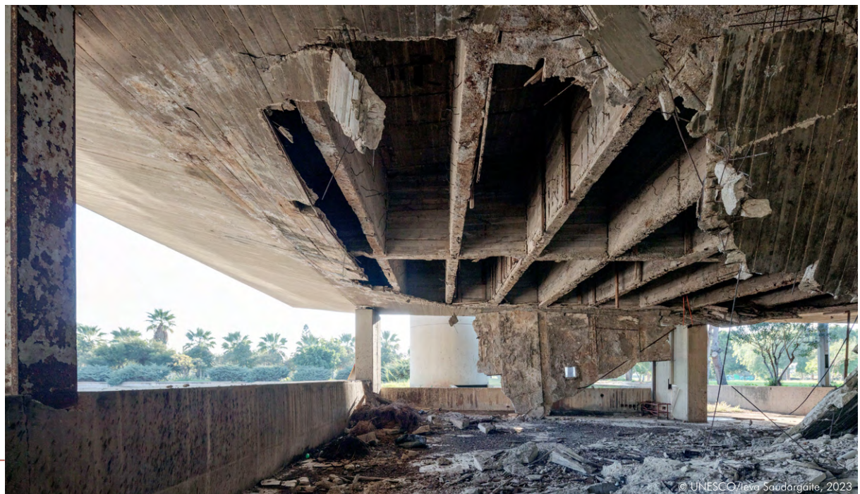
The collapsed soffit of the Open-Air Theatre.
