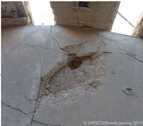
Evidence of the Civil War throughout the site needs to be carefully evaluated and potentially preserved and interpreted. In the Water Tower, there is damage to the slab from an unexploded ordnance.
