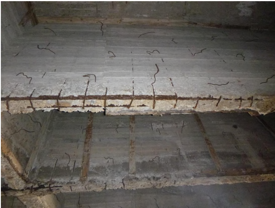
Figure 30. Spalled bottom of concrete beam and corrosion of reinforcing in beams
