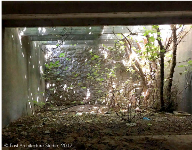
Status of one of the non-rehabilitated guest rooms (left) along with its loggia (right) at the Guest House. Finishes are damaged and the small gardens at the edge of each guest room are totally overgrown.
