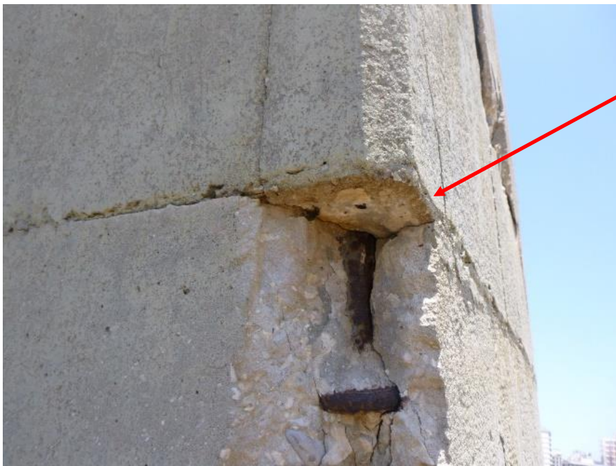
Figure 20. Spalled concrete with corroded reinforcing steel at corner of Arch near construction joint
