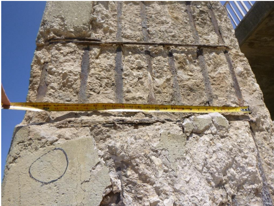
Figure 22. Corrosion of reinforcing bars resulting in section loss, at inspection opening near base of the Arch
