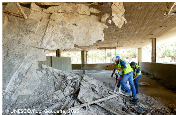
Concrete coring at the collapsed ceiling of the OAT.
