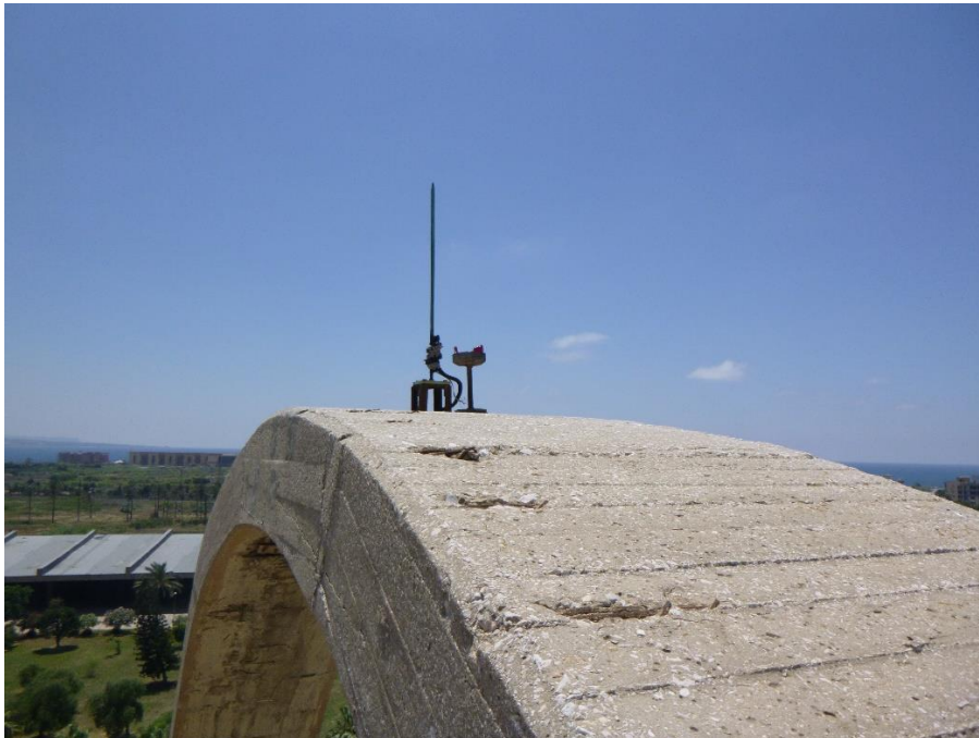
Figure 24. Paste erosion at the top of the Arch
