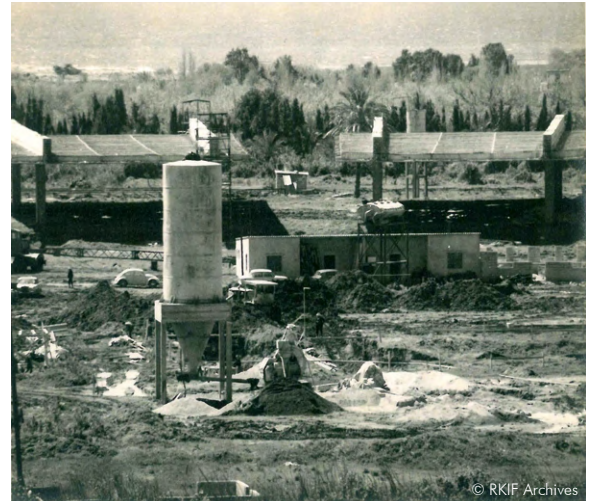
Onsite concrete batching, 1956-1966. Source: Ferdinand Dagher Collection, Courtesy of Fadlallah Dagher.
