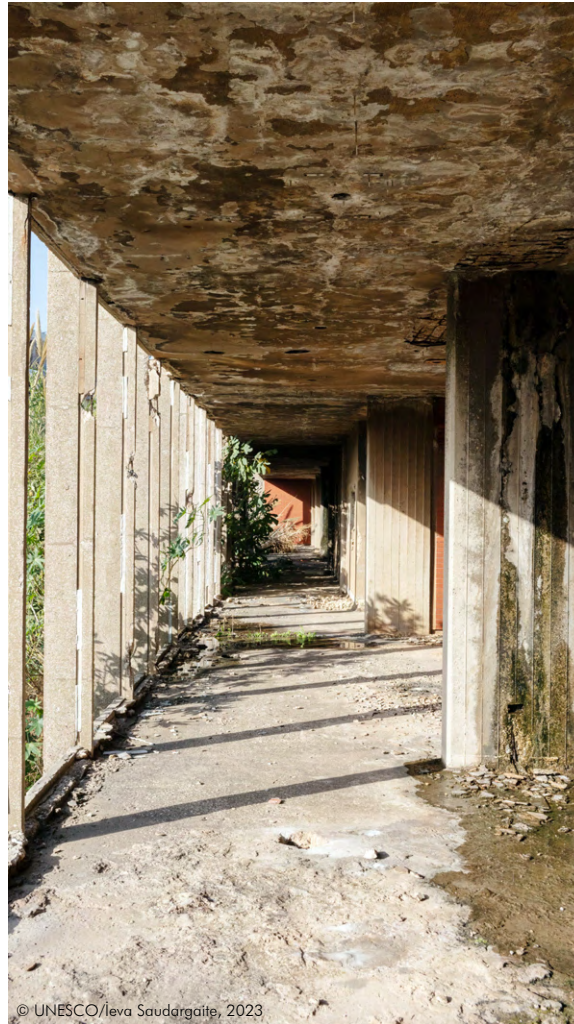
Interior of the Administration Building exposed to the elements. Staining on the underside of the slab is indicative of moisture passing through the concrete. Spalling is also visible at the bottom of the concrete column which is standing in a puddle of water. Water intrusion causes rebar corrosion, which results in concrete spalls.
