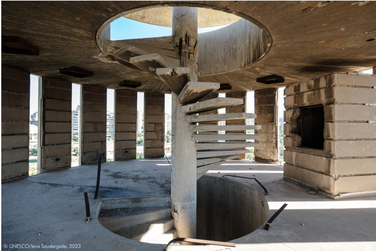
Interior of the restaurant at the 3 rd level of the Water Tower, showing the stairs leading up to the panoramic platform. Note the deterioration of the central column supporting the Water Tower's roof.
