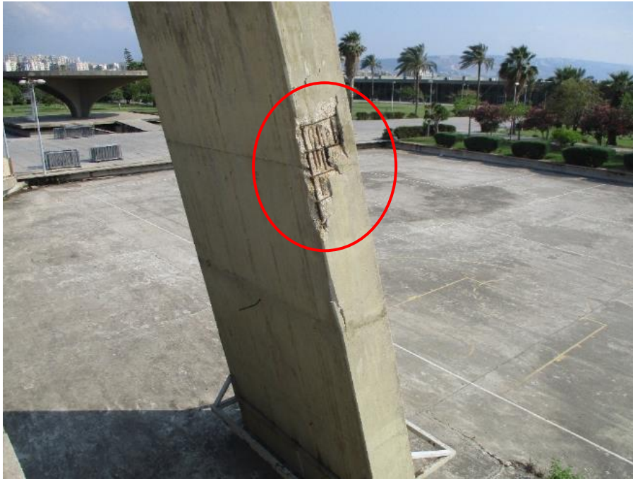
Figure 19. Spalled concrete near a construction joint
