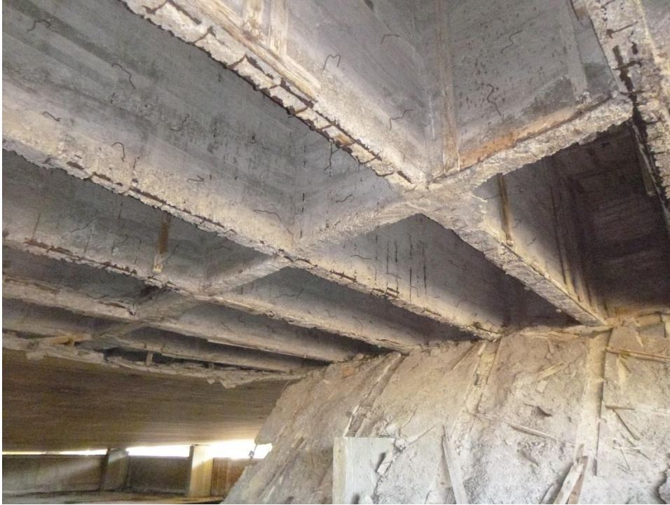
Figure 27. Soffit slab partially collapsed and pulling away from beams
