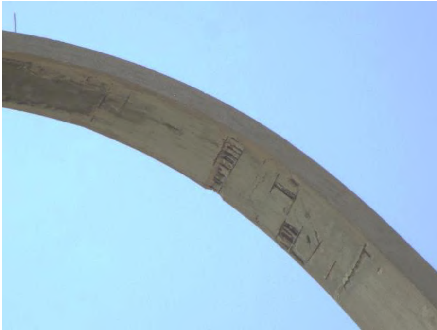
Figure 21. Spalled and delaminated concrete near rebar splice location in Arch
