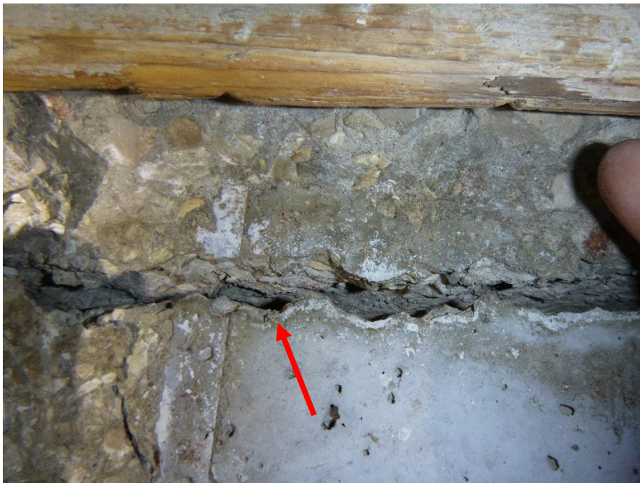
Figure 32. Separation at cold joint between the soffit slab and beam near shored area of slab
