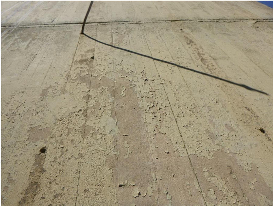
Figure 23. Peeling, blistering, and thin or missing areas of coating
