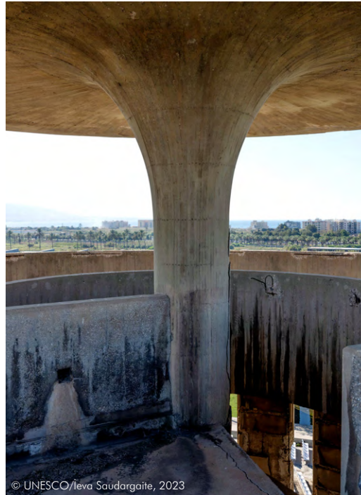
The central column supporting the Water Tower roof which offers a panoramic view of the whole site and its surroundings.
