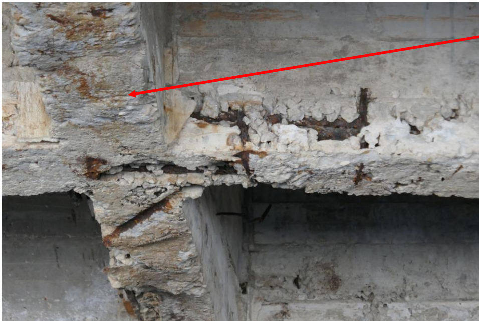
Figure 28. Honeycombing and corrosion of reinforcing in beams. Note the beam side of the cold joint between the soffit slab and beams, and stirrups at the bottom of beams.
