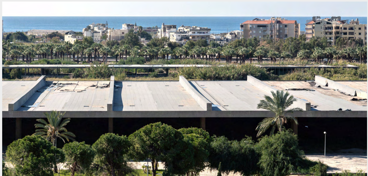
The Grand Cover's waterproofing membrane is in poor condition and has outlived its service life. Waterproofing membranes degrade in UV and require periodic replacement every 20-25 years.
