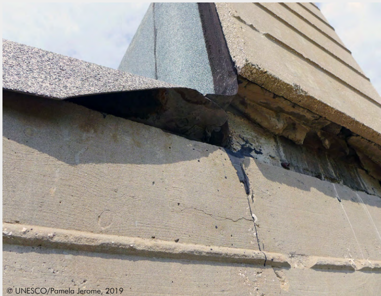
The precast-concrete panel cover at the vertical face of a main beam at the roof of the Grand Cover. Note signs of installed roof plies that are loose at perimeter edges.
