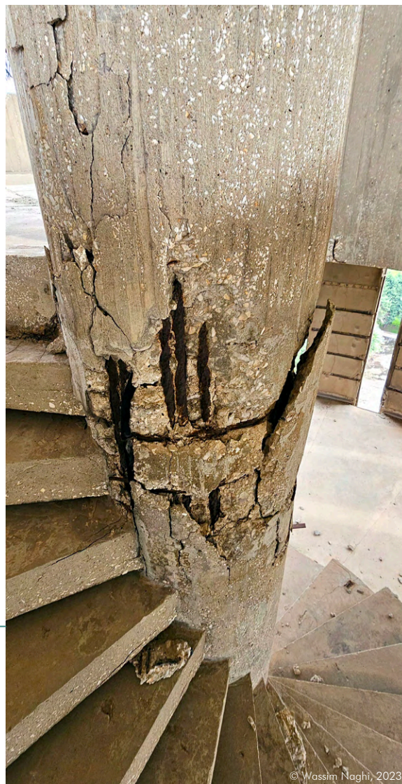
The condition of the central column of the Water Tower holding the rooftop in December 2023. Severe corrosion of the steel rebars has caused delamination of the concrete (spalling) compromising the structural integrity of the column.
