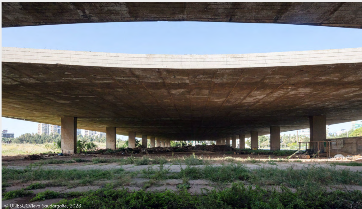
Status of the northern half of the Grand Cover. Evidence of staining on the soffit is indicative of water passing through the slab due to lack of maintenance of the waterproofing membrane; this results in rebar corrosion and concrete spalling.
