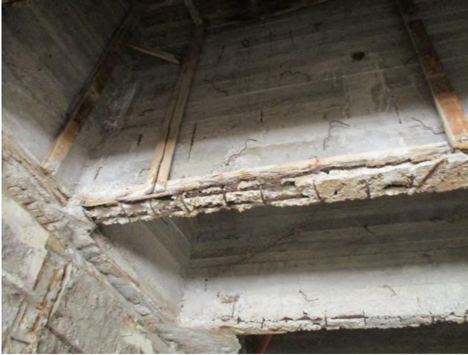
Figure 29. Spalled bottom of concrete beam and corrosion of reinforcing in beams. Note original formwork that remained in place.
