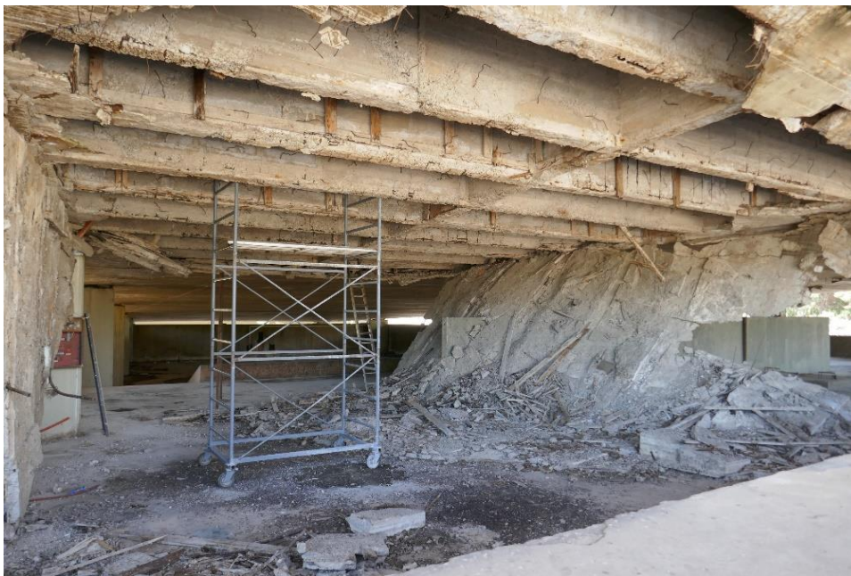
Figure 25. Collapsed area of OAT below upper-level with fallen soffit
