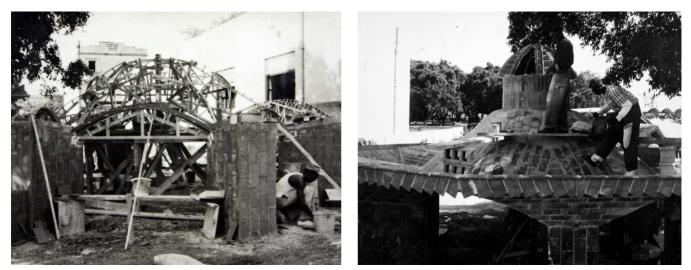
Figure 1 - The school initiated by Gumersindo to teach to local manpower the catalan vaulting building technique. The caption written by José Mosquera next to this set of pictures is: *«Banco de pruebas. Escuela para aprender la tecnica constructiva».* Pictures date back to a period comprehended between October 1961 and February 1962 (ISA archive).
