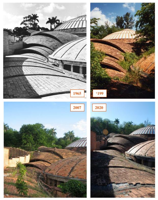
Figure 101 - The *paseo arquitectonico* of the School of Ballet during different on-site inspections: 1965 - Photo by P. Gasparini; 90's and 2007 - photos stored in ISA archive.
