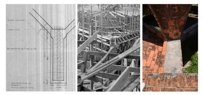
Figure 55 - On the left, the original design of the concrete block located at the top of the pillars (ISA archive). In the middle, a picture from the construction site showing some iron bars jutting from the pillar (ISA archive). On the right, a recent picture of the top of the pillars. Notice that, once again, the external layer of bricks acted as a formwork for the concrete.
