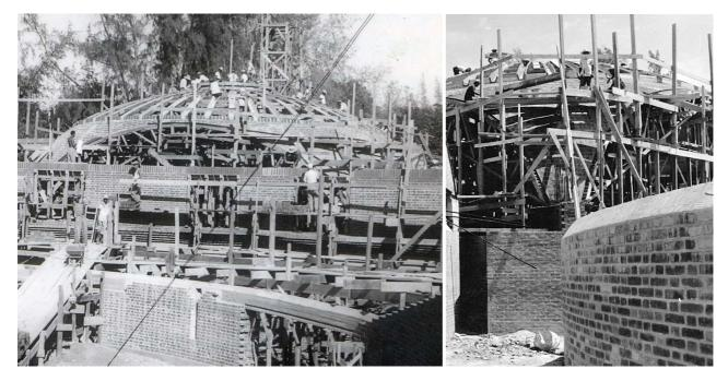
Figure 26 - Dance pavilion: layering of the clay-tile formworks for the construction of the pendentives (ISA archive).
