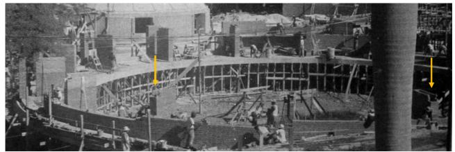
Figure 45 – Picture from the construction site showing the empty brick formworks at the top of the pillars on the mezzanine level (ISA archive).
