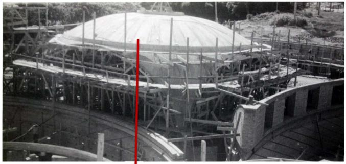
Figure 32 - Dance pavilion: view of the dome after the second concrete casting (ISA archive).
