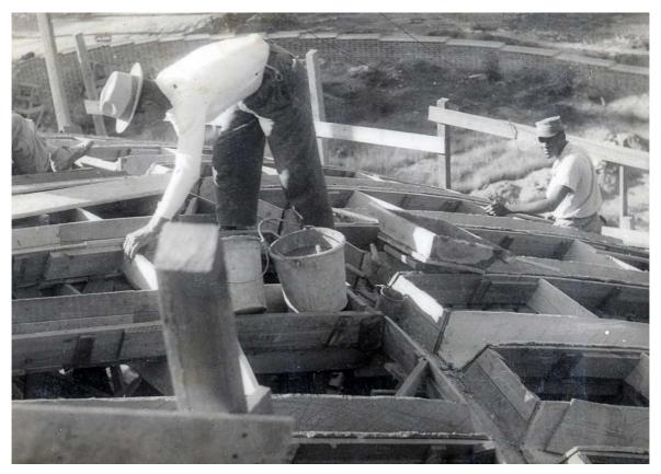
Figure 25 - Choreography Theater: Lining of the wooden formworks with clay tiles (ISA archive).
