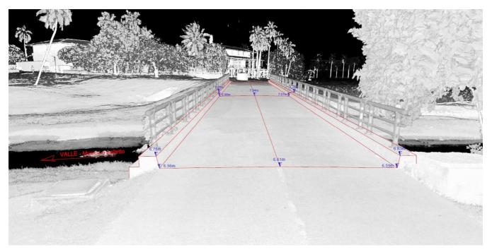
Figure 23 - Absolute elevations of some elements of the bridge near the Rectorate building.
