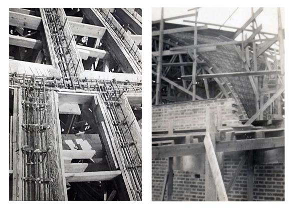
Figure 28 - Dance pavilion: positioning of the rebars. Left: view of the grid-shell. Right: view of one pendentive (both images are taken from the ISA archive).
