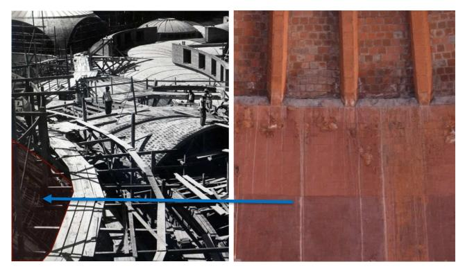
Figure 27 - Choreography Theater: clay tile formwork of the annular sector of the dome (the photo on the left is taken from the ISA archive).
