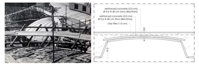
Figure 46 - On the left, construction site picture (ISA archive) showing the reinforced grid above the "false Catalan vault", whose stratigraphy is represented on the right.
