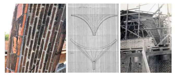
Figure 53 - On the left, the side of the pendentive simulating the catalan vaulting technique. In the middle, original drawing by Garatti illustrating the intended arrangement of the rebar (ISA archive). On the right, a picture of the construction site showing the positioning of the concrete reinforcement (ISA archive).
