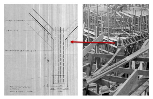
Figure 29 - On the left, the original design of the concrete block located at the top of the pillars. In the middle, a picture from the construction site showing some iron bars jutting from the pillar (images taken from the ISA archive).
