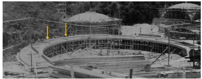
Figure 41 - The Choreography Theater during construction of the mezzanine level. The configuration of the pillars' base does not seem to indicate the presence of a reinforced core into the masonry pillars (ISA archive).
