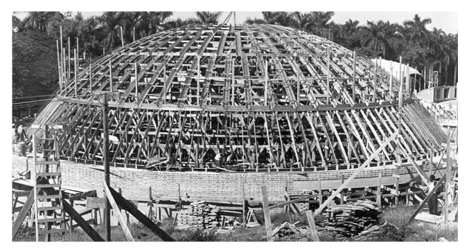
Figure 30 - Choreography Theater: formworks and rebar arrangement (ISA archive).
