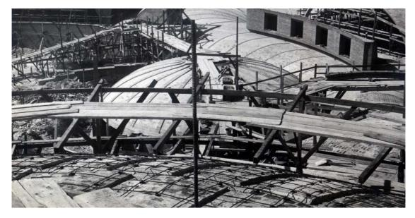
Figure 31 - Choreography Theater - view of the "catalan vaulting" filling the voids between the ribs (ISA archive).
