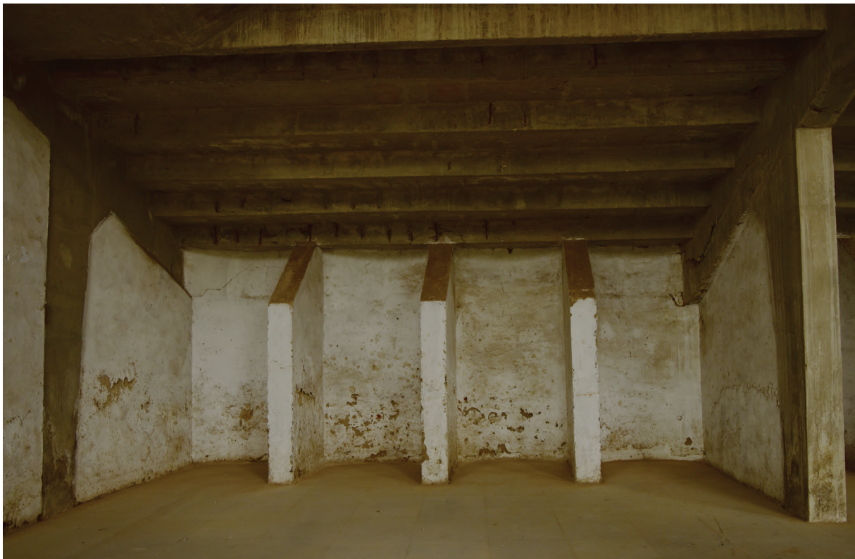
Fig. 50: View of the retaining walls and buttresses at the concourse level under the North, East and West stands
