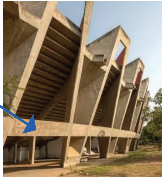
Fig. 78: Tie beam marked with a blue arrow
