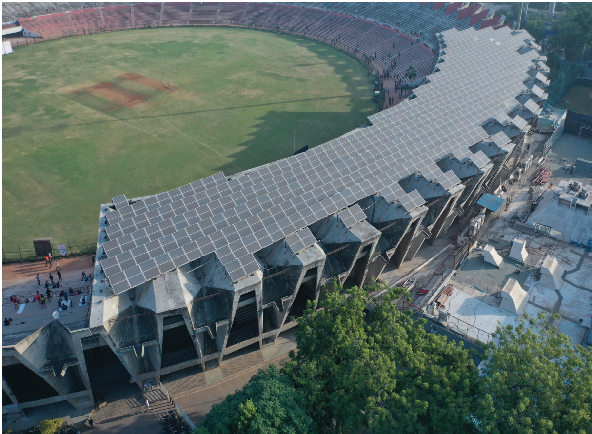
Fig. 86: Solar panels installed on the cantilevered canopy of the South Pavilion
