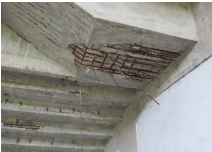
Fig. 101: Corrosion-induced spalling of concrete in the staircase
