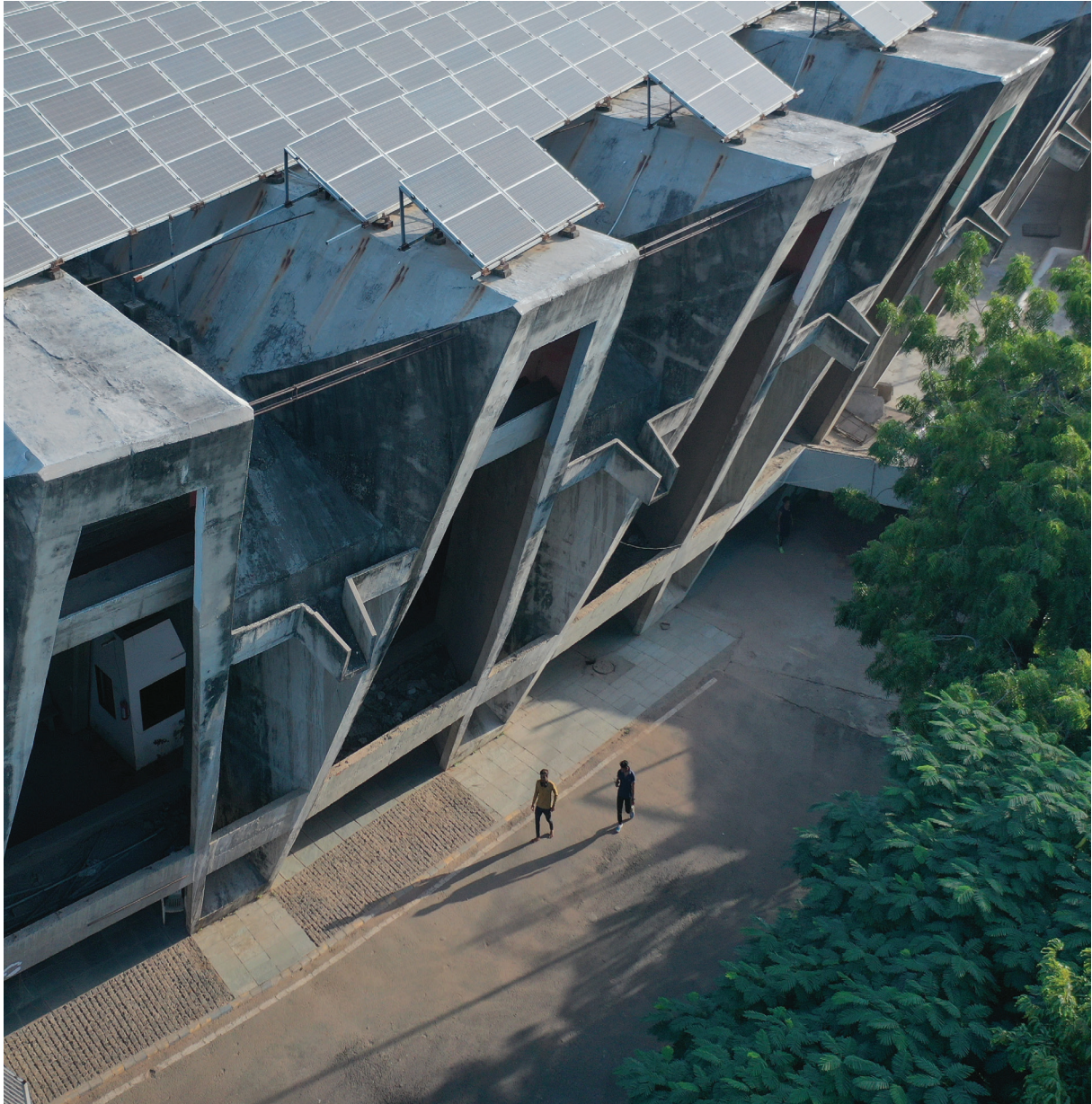
Fig. 12: Bird's-eye view of the cantilevered roof and A-Frames constructed using folded plates in SVP Stadium
