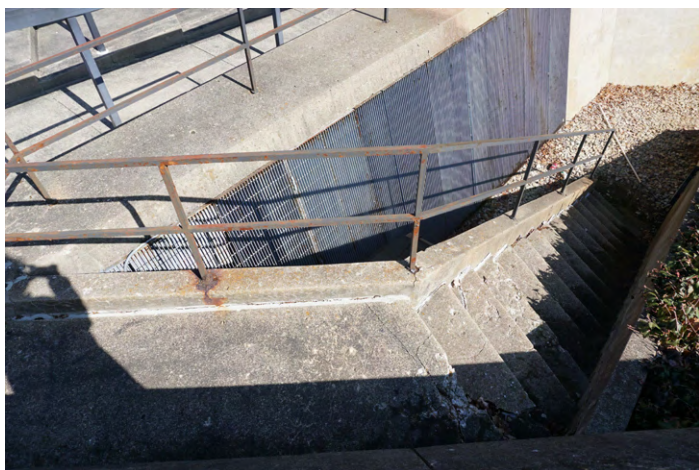
Corrosion at exterior rails - image by P&P
