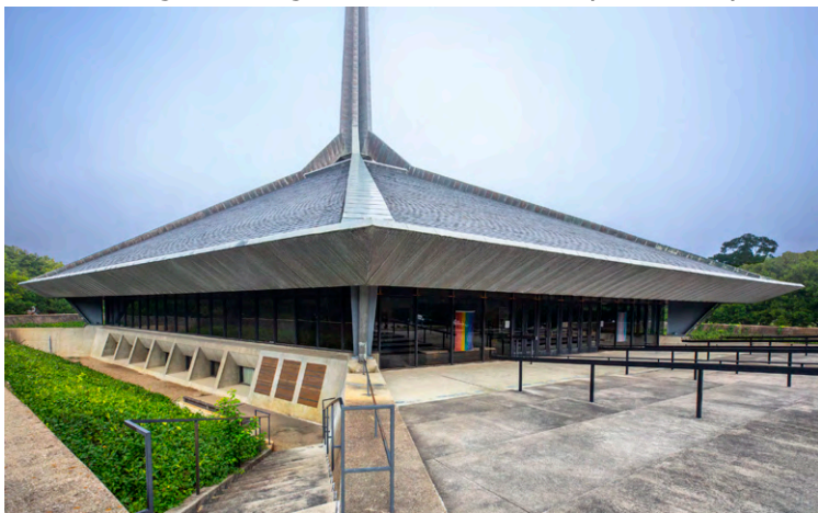
View showing roofing materials, entry level curtain wall, lower level concrete wall, and shallow entry steps - image by Hadley Fruits, 2018
