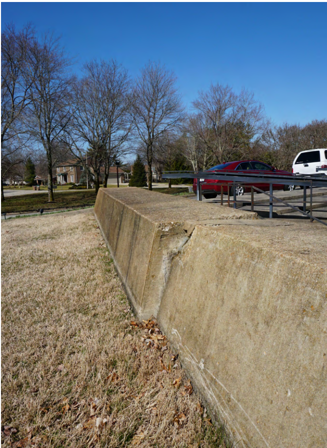
Shifting moat "retaining walls" - image by P&P
