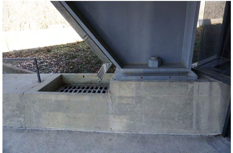
Cracks at concrete; metal corrosion at support - image by P&P
