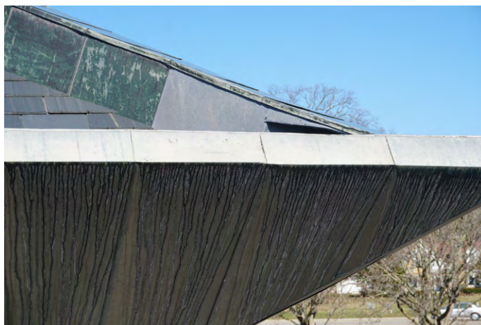
Streaking at metal roof fascia - image by P&P
