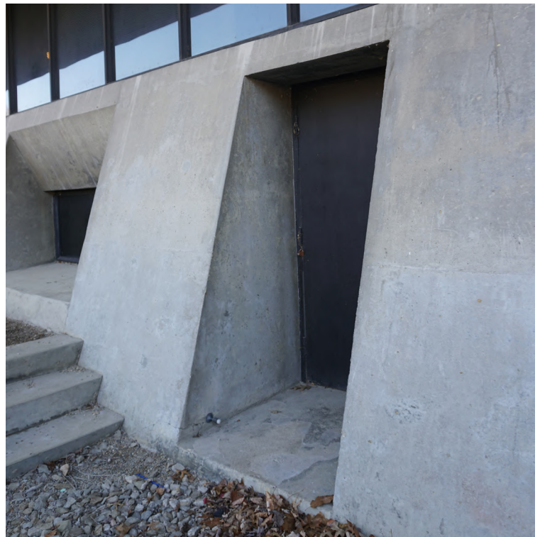
Spalling at exterior envelope - image by P&P
