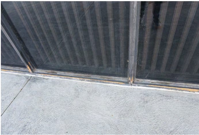
Weathered wood curtain walls - image by P&P
