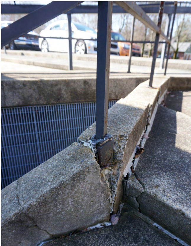
Deterioration at stairs- image by P&P
