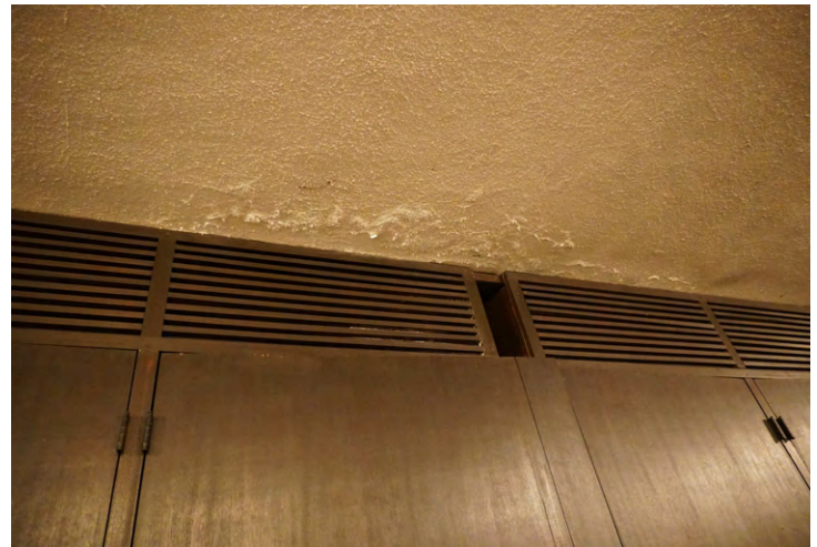
Water damage at youth activity room ceiling - image by P&P
