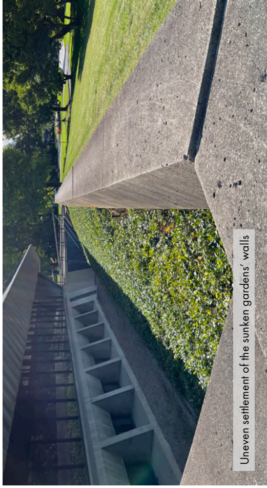
Uneven settlement of the sunken gardens' walls
