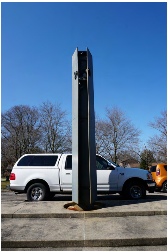
Corrosion at vent stack - image by P&P
