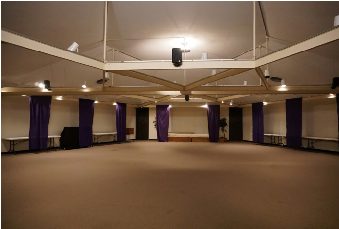
Interior of auditorium showing plenum-forming ceiling, and Unistrut lighting system - image by P&P
