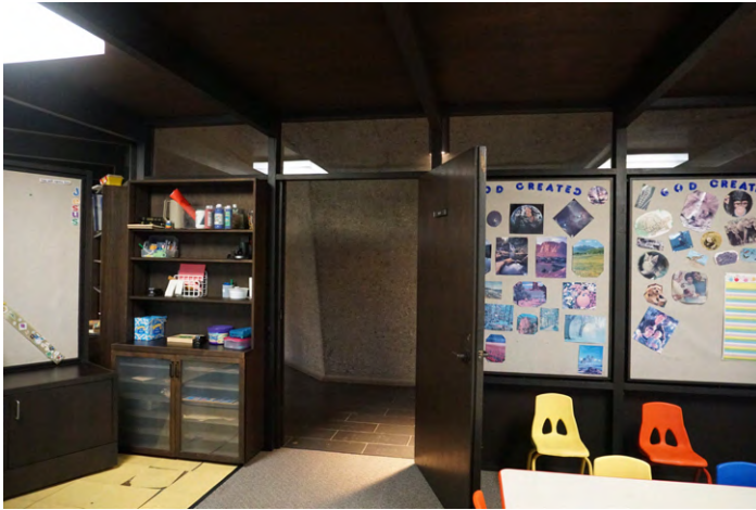
Image shows interior of office/classroom partitions and transoms, original built-in furniture, ceiling joists & studs following curtain-wall module, and lifting vinyl floor tiles – image by P&P
