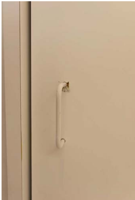
Figure 45 Minor Micarta damage at cabinet door handle in laundry.
