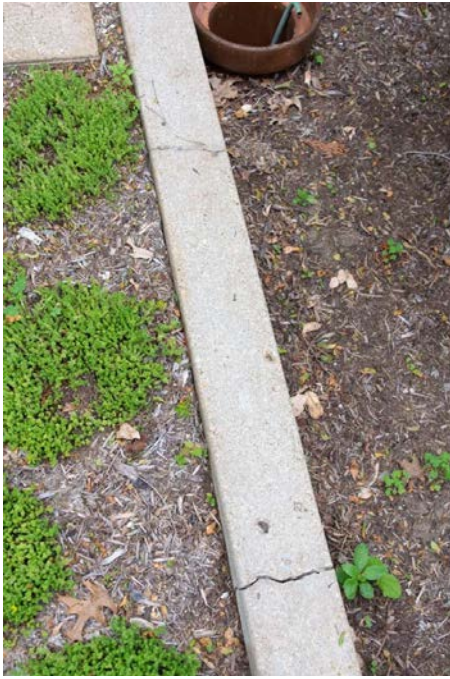
Figure 81 Cracks in concrete curb.
