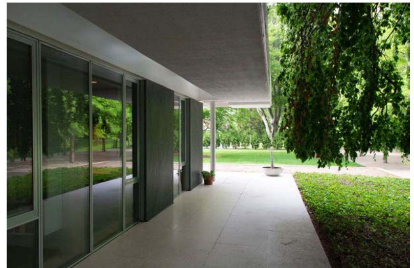
Figure 1 West soffit of house, looking south. Note the wide textured plaster soffit; the light to the left is coming through the laylights.
