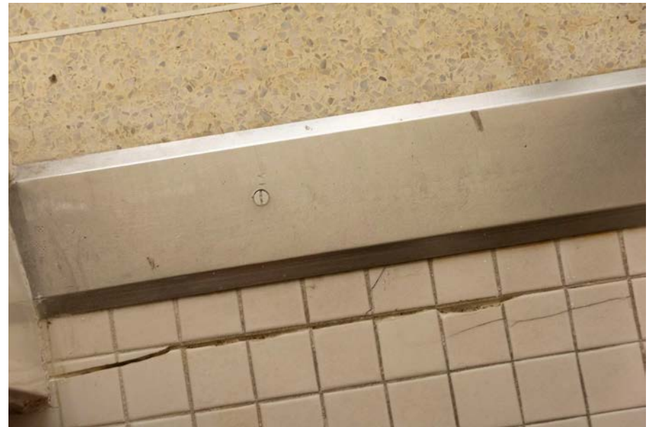
Figure 60 Cracked floor tile.
