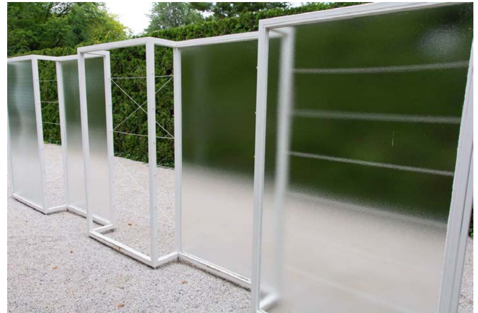
Figure 65 Missing glazing at central panel, north espalier. Note the wires for tying the branches of trees.
