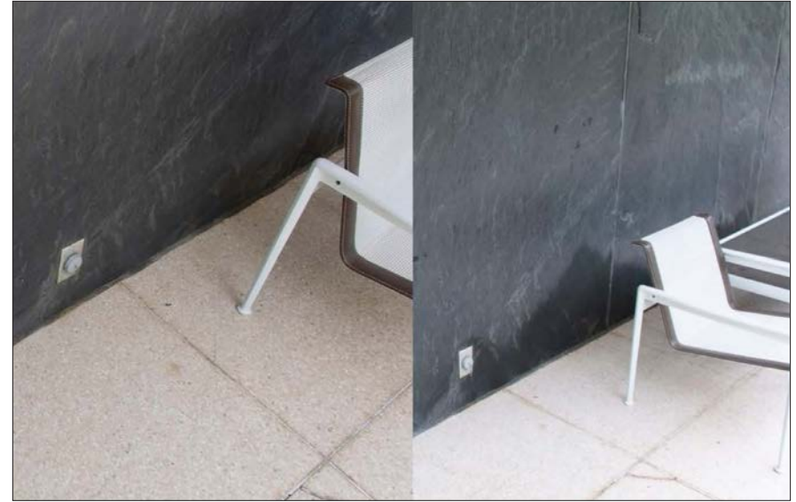
Fig. 6.6.16 Slate at southwest corner of house on dry day (left) and during a rain event (right). Date: June 2021. Photo credit: Building Conservation Associates
