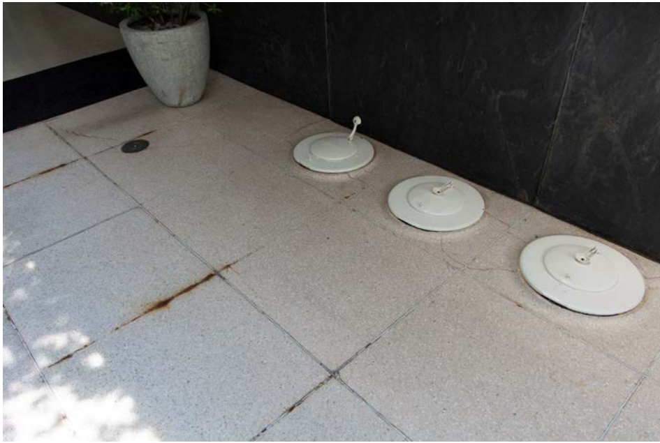
Figure 25 Most significant instances of corroding dividers due to plastic cover failure and water infiltration, northeast of house.
