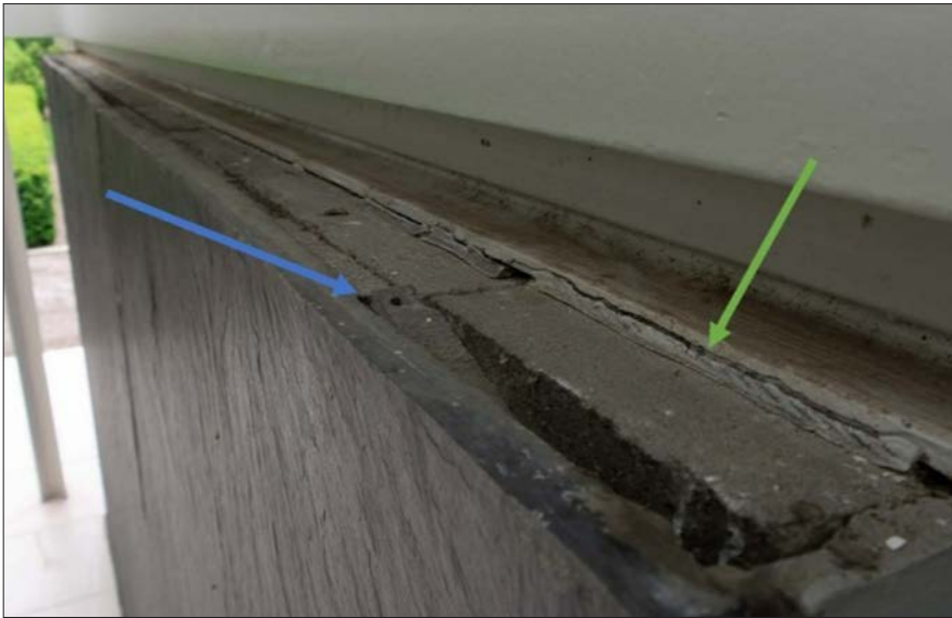
Fig. 6.6.10 Tops of slate slabs showing deteriorated mortar at top joint with CMU backup (blue arrow), typical. Note also deteriorated sealant at joint with metal angle (green arrow), typical. Date: June 2021. Photo credit: Building Conservation Associates
