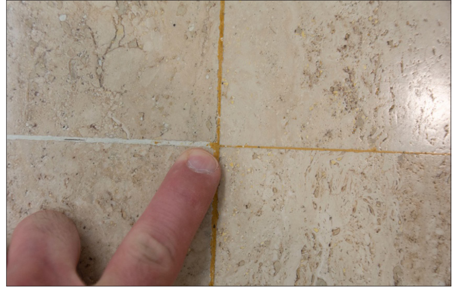
Fig. 6.4.16 Yellowed later repair grout, typical. Date: June 2021. Photo credit: Building Conservation Associates
