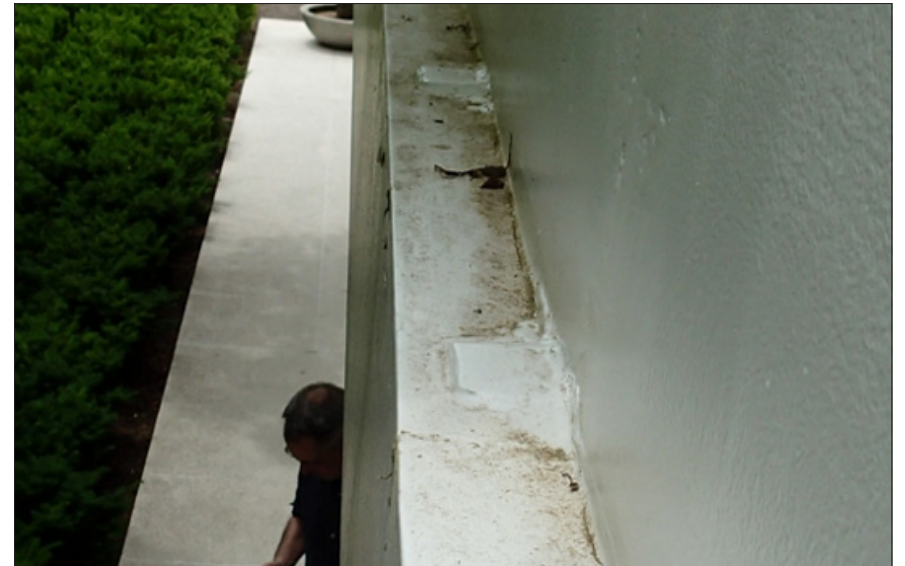
Fig. 6.3.6 Evidence of water ponding and past corrosion at the parapet/fascia joint. Date: June 2021. Photo credit: Michael C. Henry
