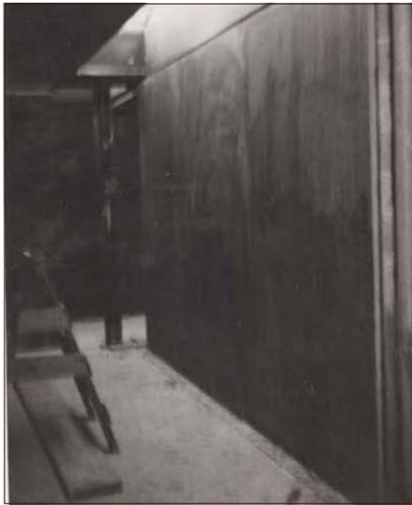
Fig. 6.6.3A "Slate on east side of Guest Wing. The verticle [sic] streaks are a result of washing. They will be removed when slate is oiled." Date: August 24, 1956. Photo credit: MHG_la_B001_f003_016-022, Miller House and Garden Collection (M003), Newfields Archives
