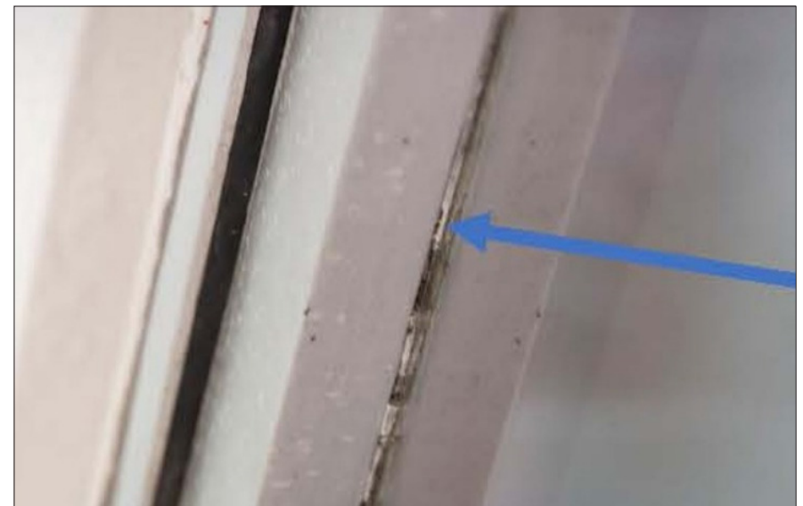
Fig. 6.7.2 Small white deposits of surface corrosion at aluminum window frame, typical. Note also the deteriorated sealant at arrow. Date: June 2021. Photo credit: Building Conservation Associates
