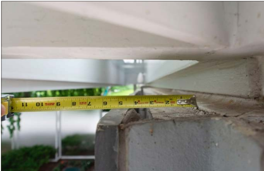
Fig. 6.6.11 Gap between concrete backup and slate slab in excess of 1". However, note that the joint between the steel angle in the foreground and the slate slab is close to the 3/8" specified in the drawings. Date: June 2021. Photo credit: Building Conservation Associates
