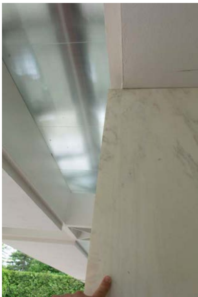
Figure 18 Subtle vertical streaks near laylight at edge of marble slab, north of house.
