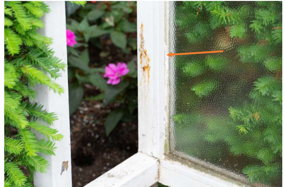
Figure 64 Paint failure and corrosion at espalier, typical. Note also the failing sealant at glazing (arrow).
