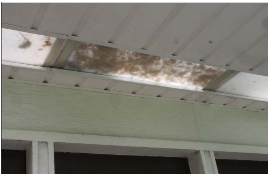
Fig. 6.17.3 Greenhouse/Office: View of soffit over window, showing debris above plexiglass panels. Note also cracks and checking in plywood "intel." Date: June 2021. Photo credit: Scattergood Design
