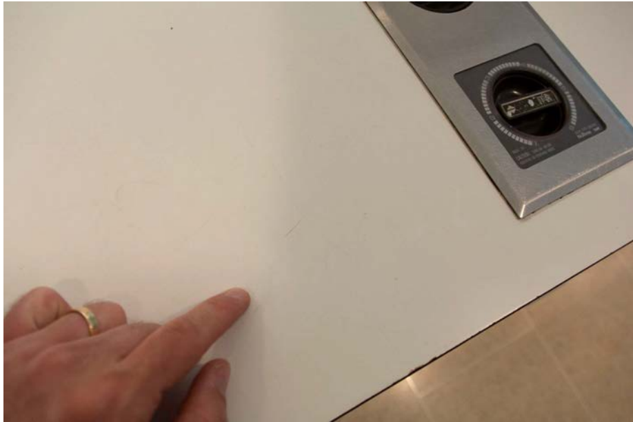
Figure 44 Numerous small scratches in Micarta kitchen countertop.
