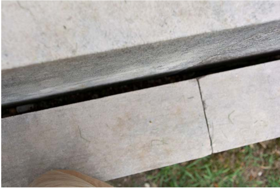
Figure 75 Photo looking down into large gap between curb and paving units, typical at west of platform.
