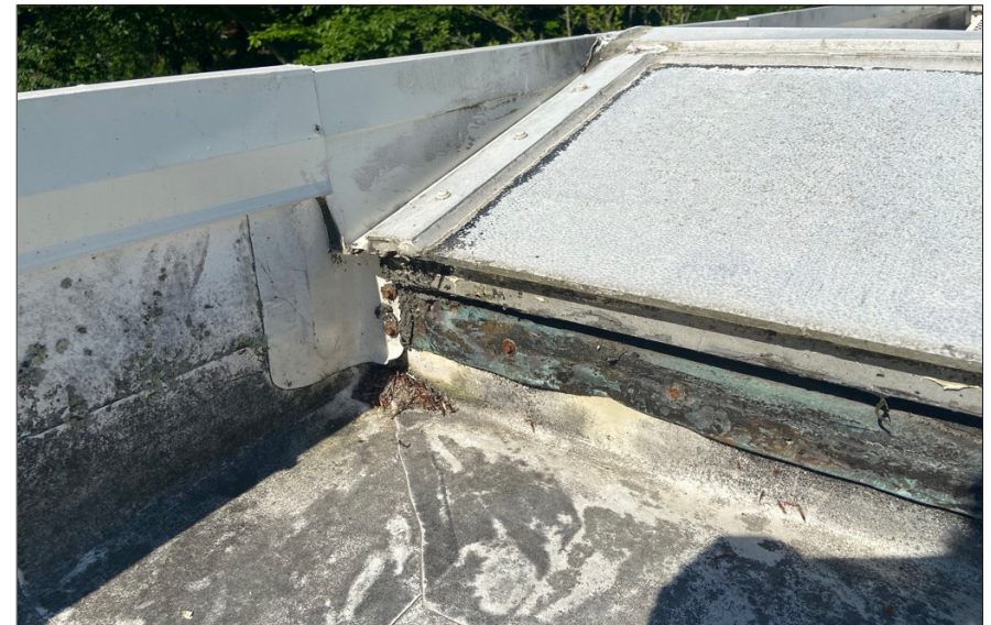
Fig. 6.4.8 Copper counter flashing perforated by steel fasteners (right). Non-original cap flashing on parapet (left). Date: June 8, 2020. Photo credit: Newfields.
