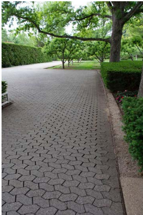
Figure 69 Larger region of settlement at far east of driveway, between front and rear halves. Note curvature of edge and gaps between units.
