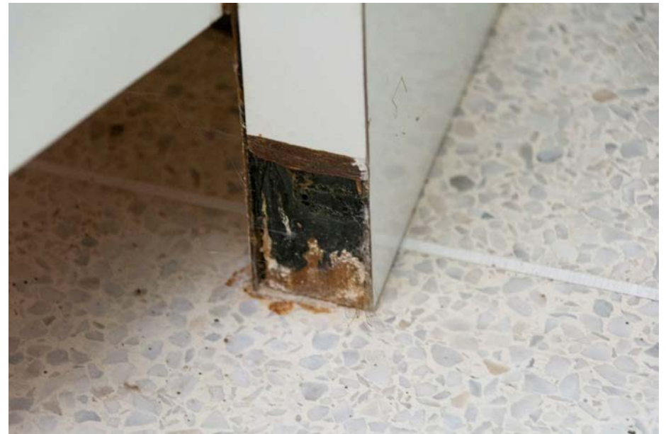
Figure 47 Largest loss of Micarta noted, at divider in master bathroom.
