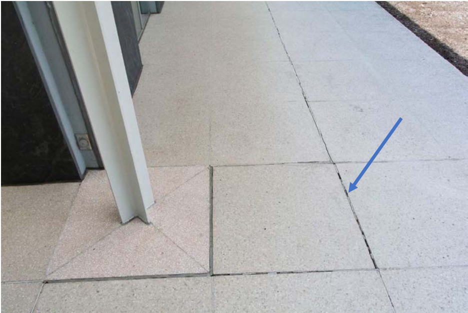
Figure 26 Widened joint at arrow has been with sealant that has failed, typical.
