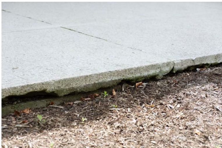
Figure 23 Terrazzo and eroded setting bed overhanging concrete slab at north of house, typical.
