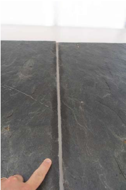
Figure 14 Apparent staining adjacent to sealant joint in slate, typical.
