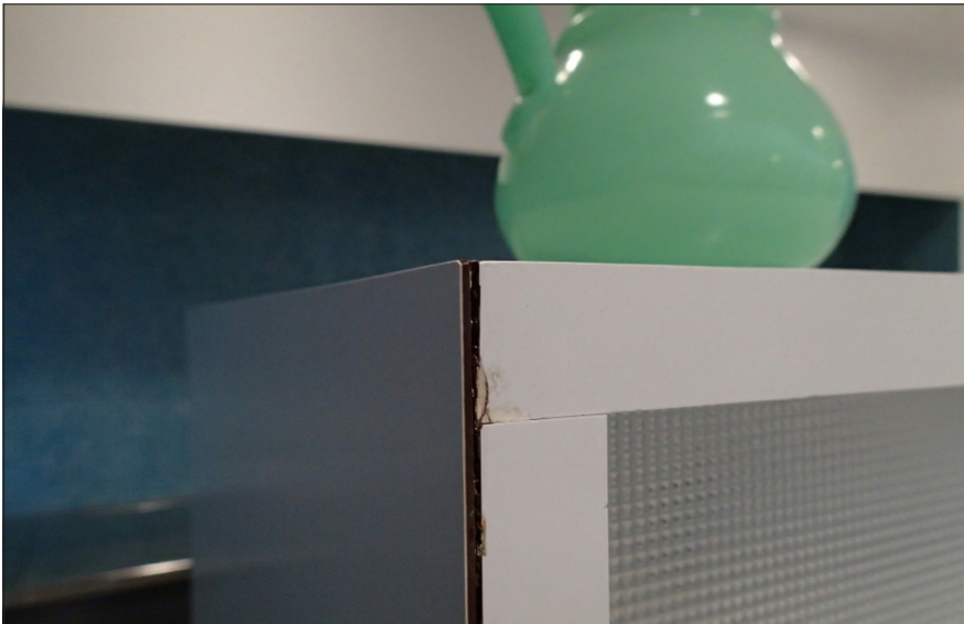
Fig. 6.6.23 Chipped micarta laminate at kitchen storage unit. Date: June 2021. Photo credit: Scattergood Design
