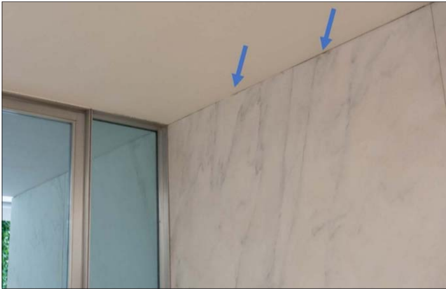
Fig. 6.6.18 Small chips at top of slab (arrows) presumably from picture hangers such as those visible at right of photo. Date: June 2021. Photo credit: Building Conservation Associates
