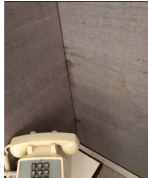
Fig. 6.6.21 Water damage on silk wallcovering in recessed area of Master Bedroom. Date: June 2021. Photo credit: Scattergood Design
