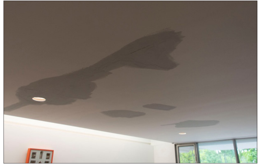
Fig. 6.4.15 Largest area of plaster damage due to roof leaks, in Children's Playroom/ Mrs. Miller's Office. Date: June 2021. Photo credit: Building Conservation Associates
