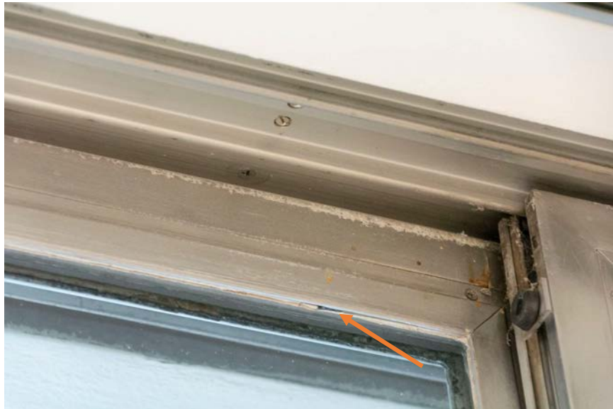
Figure 48 Isolated location of heavy corrosion deposits at sliding doors west of house. The reason for their concentration at this location is unknown. Note also deteriorated sealant (arrow).
