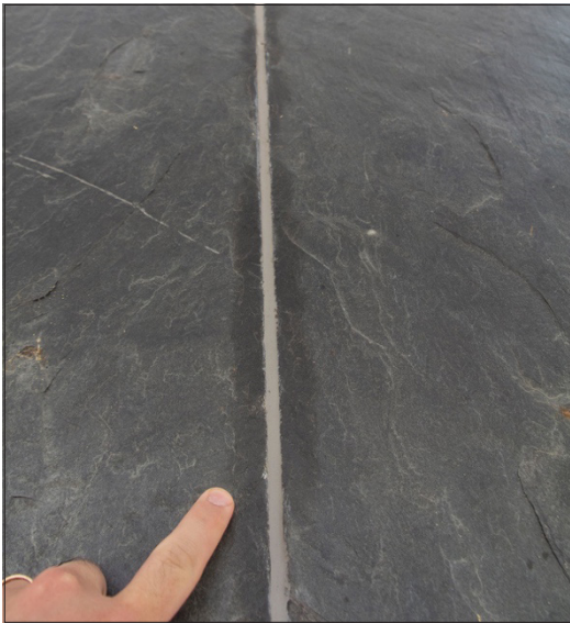
Fig. 6.6.15 Apparent staining adjacent to sealant joint in slate, typical. Date: June 2021. Photo credit: Building Conservation Associates
