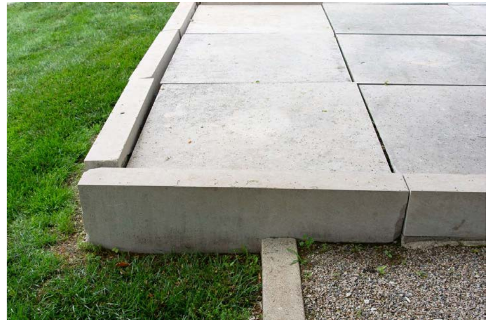
Figure 74 Displaced units, typical.
