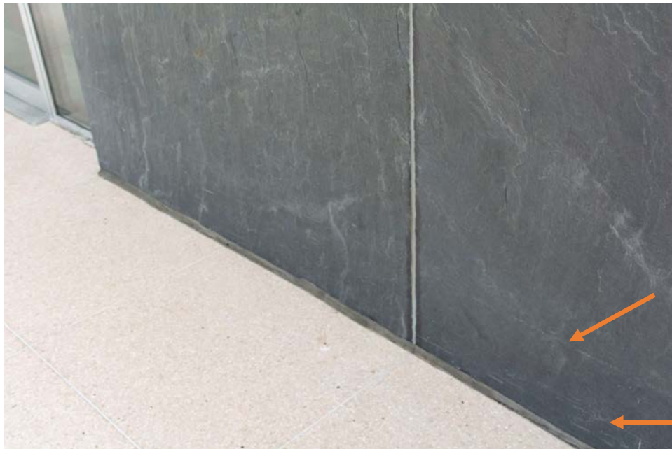
Figure 16 Horizontal scratches (arrows) near base of slate slabs, typical.
