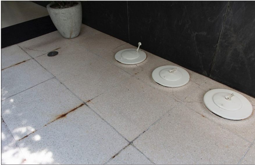
Fig. 6.2.6 Most significant instances of corroding dividers due to plastic cover failure and water infiltration, northeast of house. Date: June 2021. Photo credit: Building Conservation Associates
