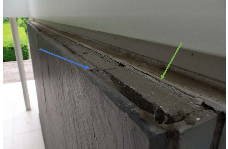
Figure 6 Tops of slate slabs showing deteriorated mortar at top joint with CMU backup (blue arrow), typical. Note also deteriorated sealant at joint with metal angle (orange arrow), typical.
