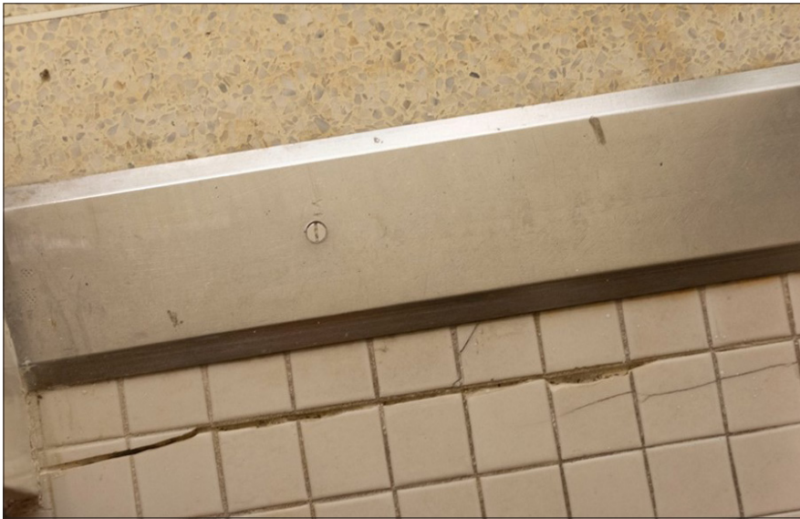
Fig. 6.4.17 Cracked floor tile in bathroom. Date: June 2021. Photo credit: Building Conservation Associates
