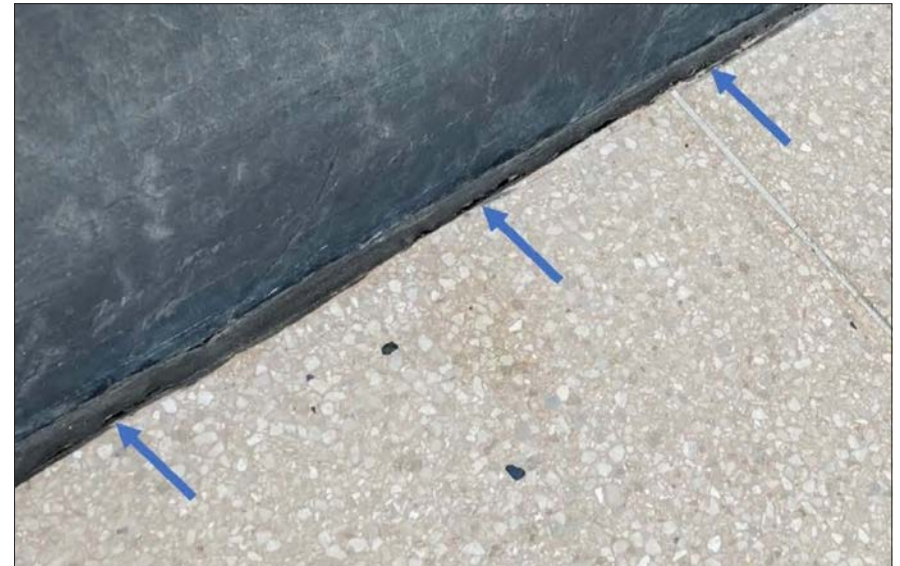
Fig. 6.6.13 Gaps in sealant show what appears to be the edge of the terrazzo (arrows), which stops short of the slate. Note also that the divider strip cover clearly stops short of the slate. Date: June 2021. Photo credit: Building Conservation Associates
