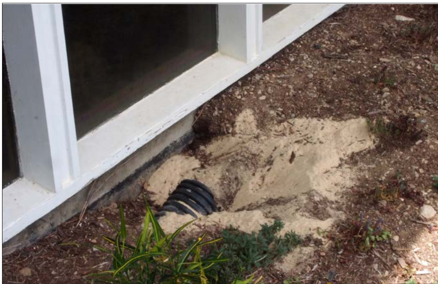
Fig. 6.17.4 Greenhouse/Office: View of planter below south window wall showing build-up of earth and scouring around drain due to excessive runoff. Date: June 2021. Photo credit: Scattergood Design
