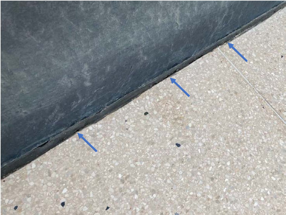
Figure 10 Gaps in sealant show what appears to be the edge of the terrazzo (arrows), which stops short of the slate. Note also that the divider strip cover clearly stops short of the slate.
