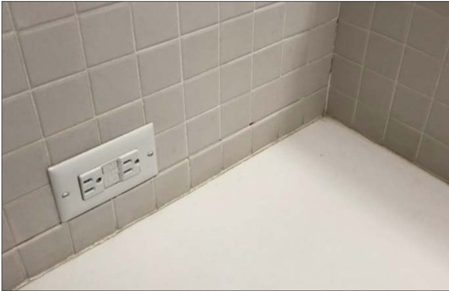
Fig. 6.6.22 Typical ceramic tile on bathroom walls. Note cracked grout in corner joint and at counter. Date: June 2021. Photo credit: Scattergood Design
