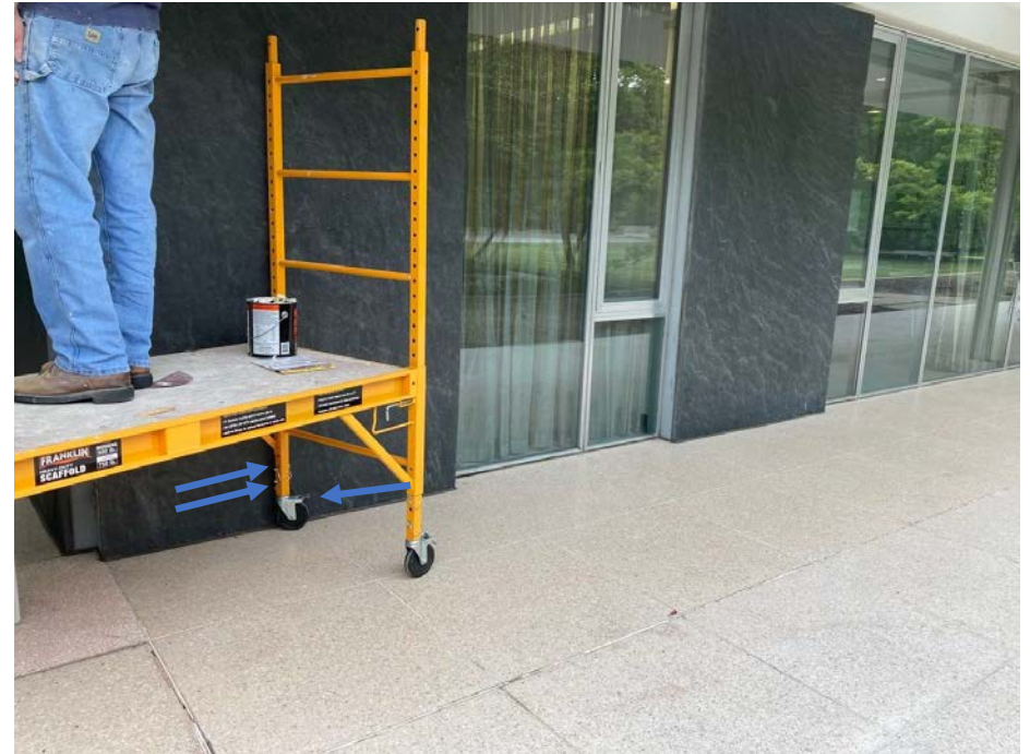
Figure 17 Potential points of contact between Baker scaffold and slate (arrows).
