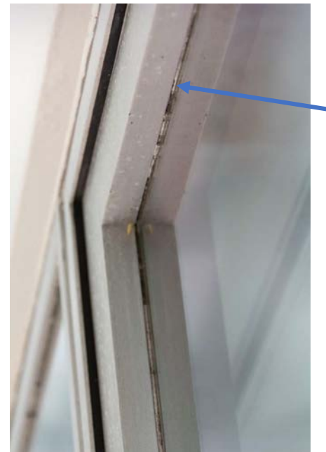
Figure 29 Small white deposits of surface corrosion at aluminum window frame, typical. Note also the deteriorated sealant at arrow.
