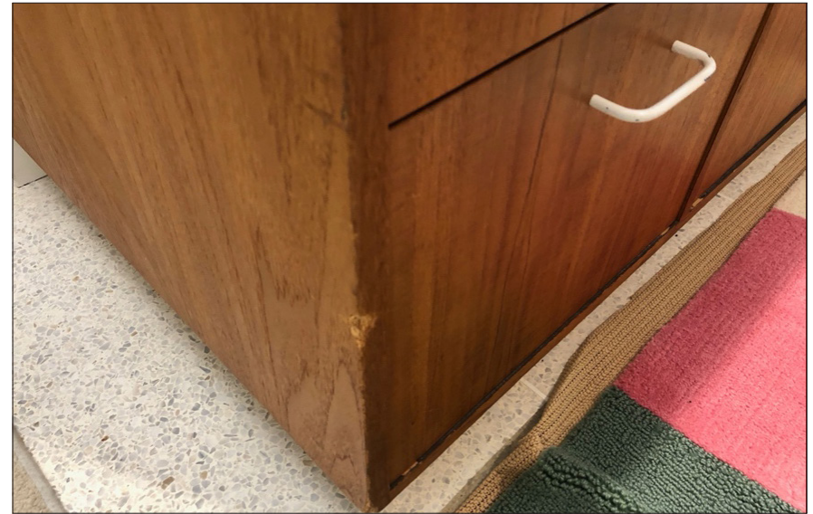
Fig. 6.8.11 Gouged wood on lower corner of storage unit, likely caused by vacuum attachments or power cords. Date: June 2021. Photo credit: Scattergood Design
