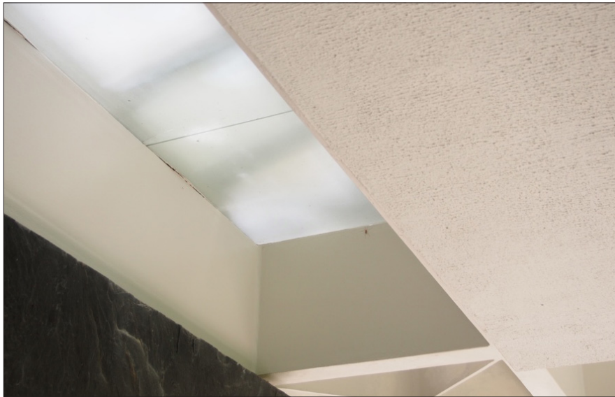
Fig. 6.4.14 More roughly-stippled plaster finish may be a later repair. Date: June, 2021. Photo credit: Scattergood Design
