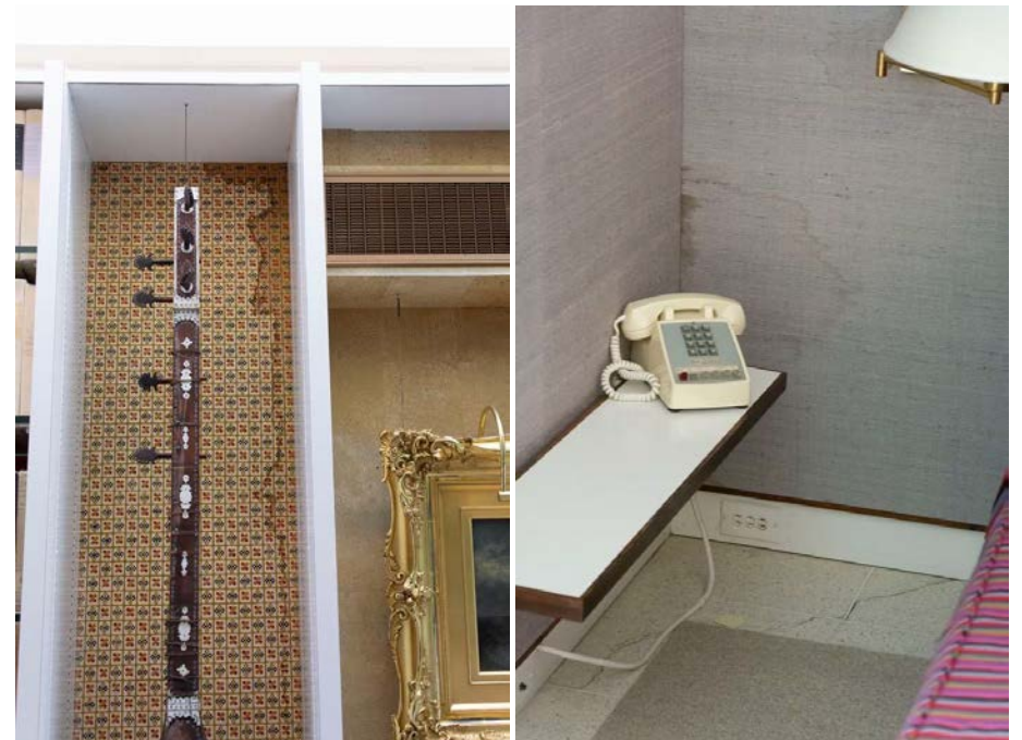
Figure 41 Water staining at storage wall and in master bedroom.
