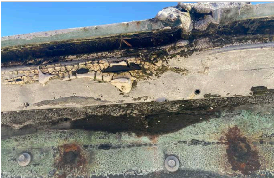
Fig. 6.4.10 Accumulation of sealants at intersection of roof and skylight. Date June 8, 2020. Photo credit: Newfields.
