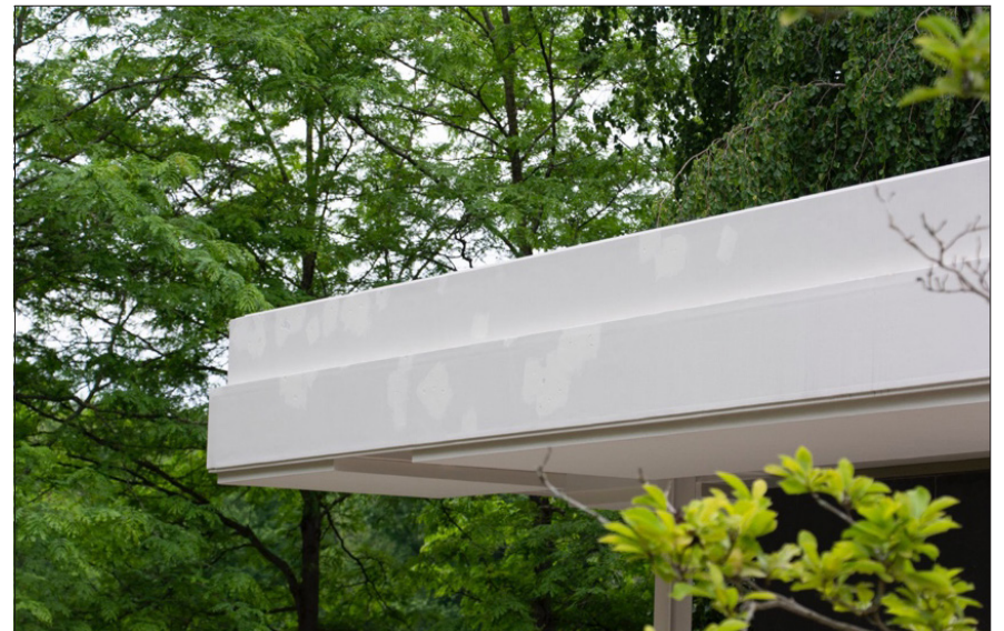
Fig. 6.4.12 Evidence of many touch-up campaigns at fascia of steel eaves, southwest corner of house. Date June 8, 2020. Photo credit: Newfields.
