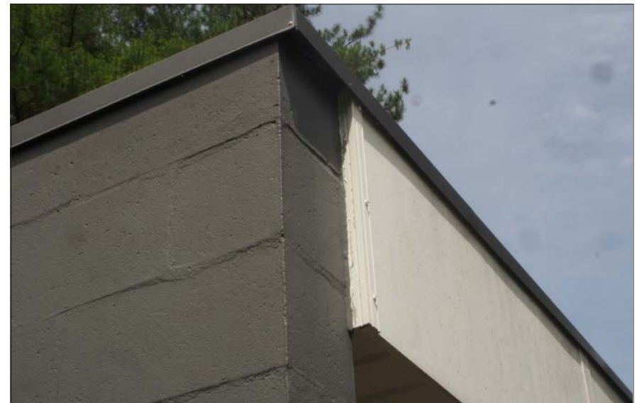
Fig. 6.17.2 Greenhouse/Office: Detail of fascia over south window, showing exposed plywood edge. Date: June 2021. Photo credit: Scattergood Design
