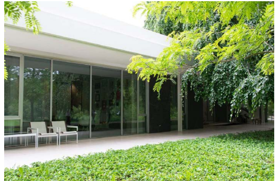
Figure 28 Fixed and operable windows in aluminum glazing assemblies at the west of the house.
