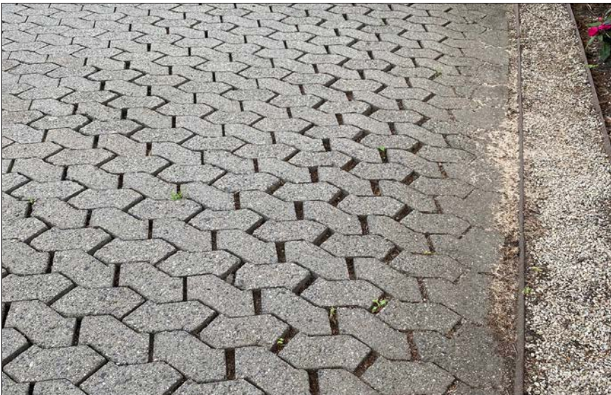
Fig. 710.2 Service Drive, south end (note damage to paving and depression at metal planter edge.) Date: 2021. Photo credit: PennPraxis/RM.
