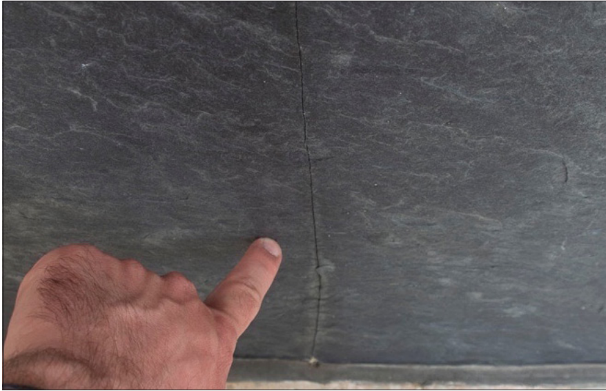
Fig. 6.6.14 Widest of the hairline cracks in the slate. Other cracks appear more associated with natural veining. Date: June 2021. Photo credit: Building Conservation Associates
