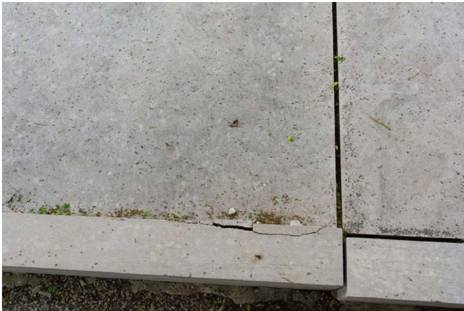
Figure 76 Crack in stone curb.
