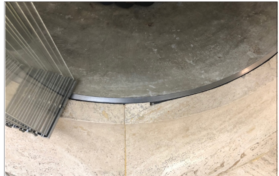
Fig. 6.11.2 Cracking and loss at edge of fireplace hearth. Date: June 2021. Photo credit: Scattergood Design
