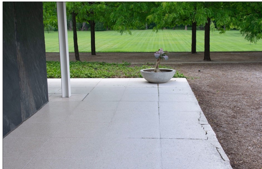
Fig. 6.2.5 Broken terrazzo at edge, typical, likely due to the unsupported condition shown in Fig. 6.2.4. Date: June 2021. Photo credit: Building Conservation Associates
