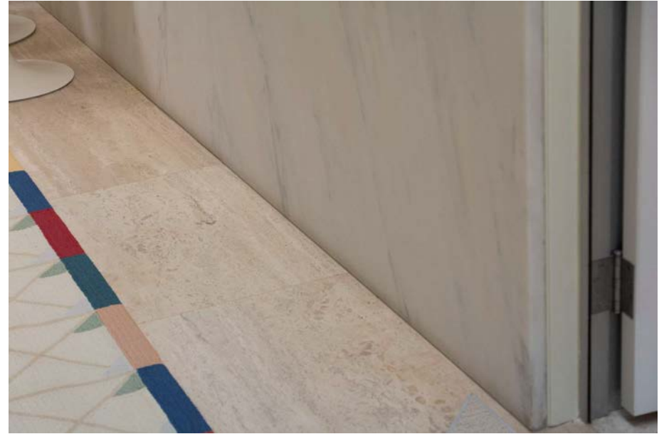
Figure 35 Discoloration at bottom inch of marble, likely due to floor polishing.
