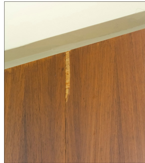
Fig. 6.8.12 Largest area of lost veneer, possibly caused by contact with adjacent steel when opened. Date: June 2021. Photo credit: Building Conservation Associates
