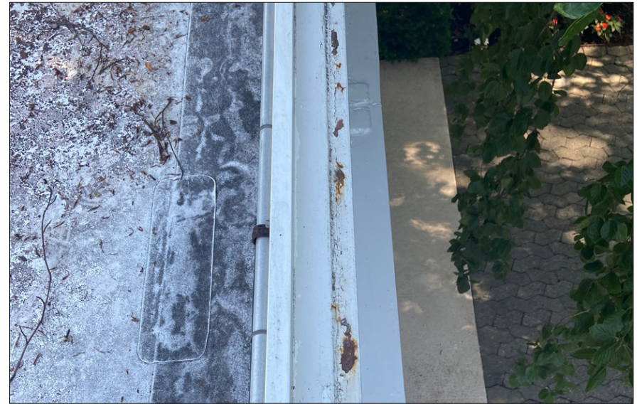
Fig. 6.4.11 Cap flashing on parapet. Note corrosion on top flange of steel channel beam. Date: June 8, 2020. Photo credit: Newfields.
