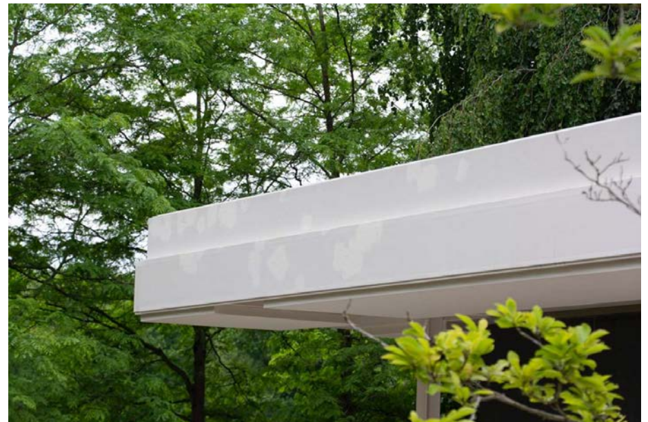
Figure 3 Evidence of many touch-up campaigns at fascia of steel eaves, southwest corner of house.
