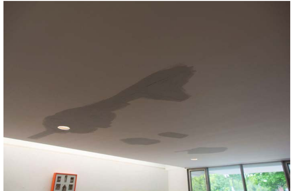
Figure 33 Largest region of plaster damage due to roof leaks in children's bedroom suite.
