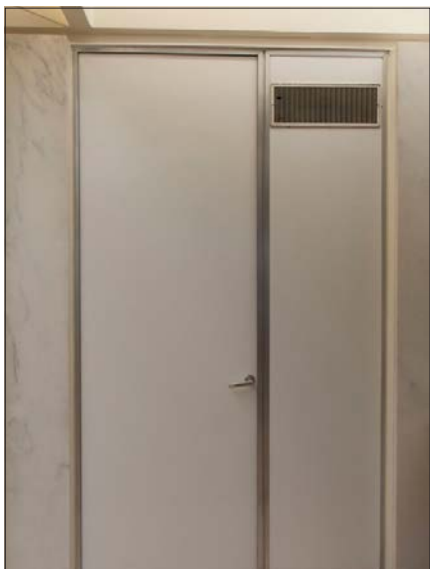
Fig. 6.6.8 Typical Micarta door and wall panel assembly with stick aluminum framing. The wall panels typically formed enclosures for wiring, light switches and/or ductwork, as in this photo. Date: June 2021. Photo credit: Building Conservation Associates
