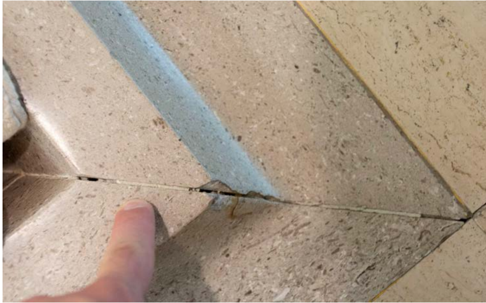
Figure 55 Suspected original white grout at perimeter of conversation pit. Note the losses.
