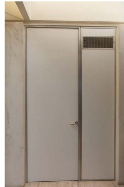
Figure 43 Typical Micarta door and wall panel assembly. The wall panels typically house light switches or ductwork, as in the above photo.
