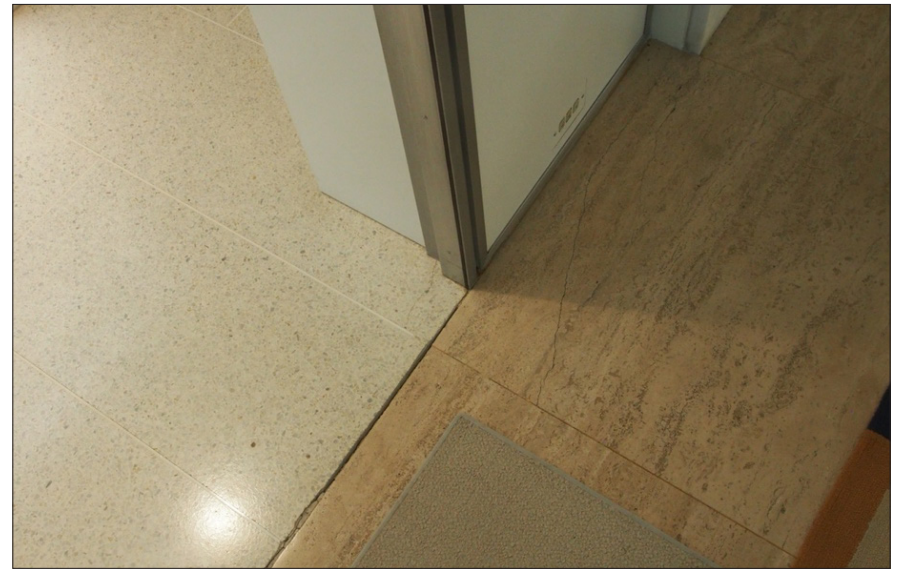
Fig. 6.2.8 Open joint between travertine and terrazzo at doorway between Dining Room and Kitchen. Date: June 2021. Photo credit: Scattergood Design
