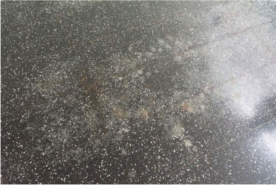
Figure 27 Staining at black terrazzo and dividers in carport.
