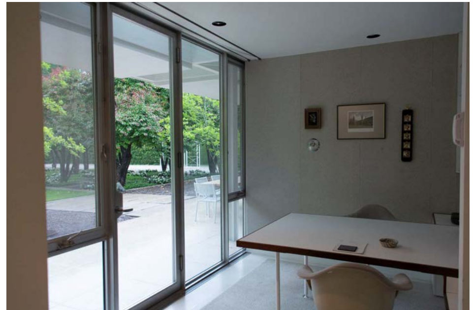
Figure 20 Exterior terrazzo viewed from the interior at the northwest corner of the house, where the terrazzo flooring is almost continuous.
