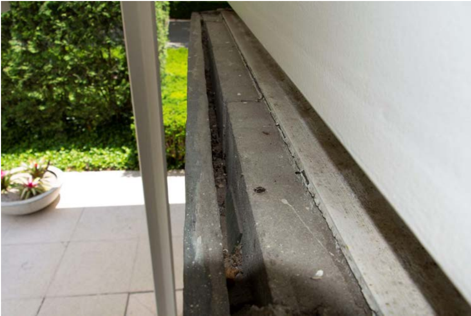
Figure 9 Top of slate slab with joint entirely open. Note the large amount of debris in the cavity.
