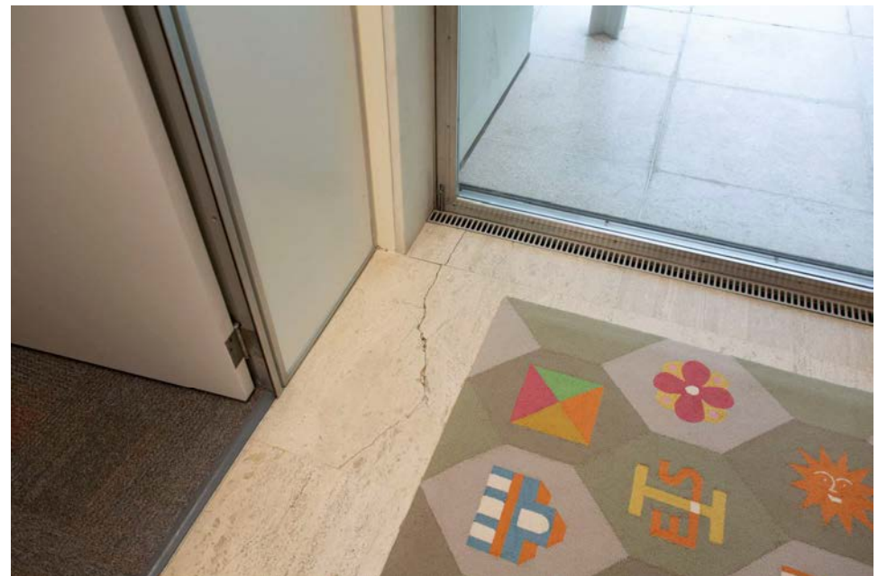
Figure 54 Cracked travertine in dining room.
