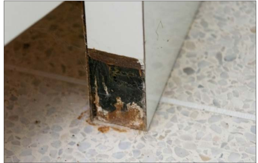
Fig. 6.6.24 Largest loss of Micarta noted, at divider in Master Bathroom. Date: June 2021. Photo Credit: Building Conservation Associates
