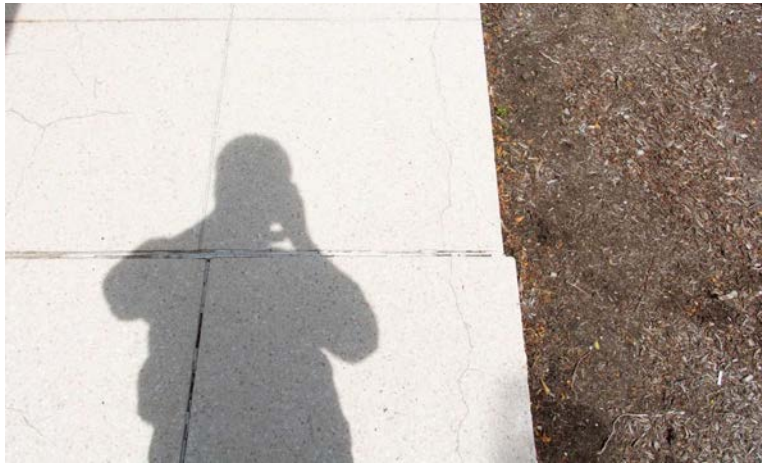
Figure 22 Extent of displacement at the southwest corner of the house as evidenced by the protruding units in the bottom of the photograph. Note also that every unit is cracked.
