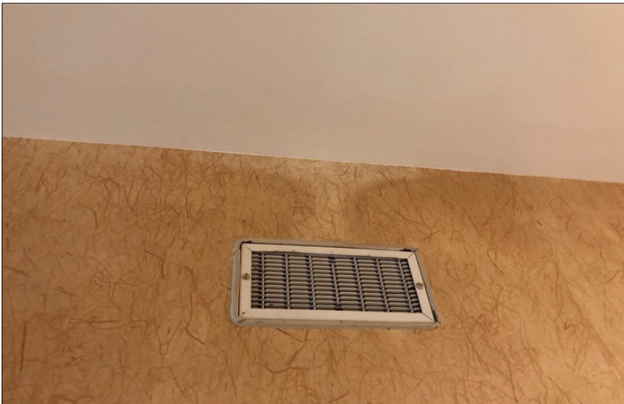
Fig. 6.6.19 Water damage or fading adjacent to return air grille in Powder Room. Date: June 2021. Photo credit: Scattergood Design
