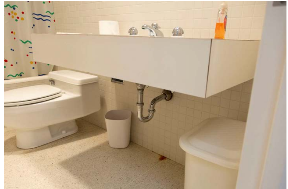
Figure 58 Iron staining at terrazzo in children's suite bathroom.
