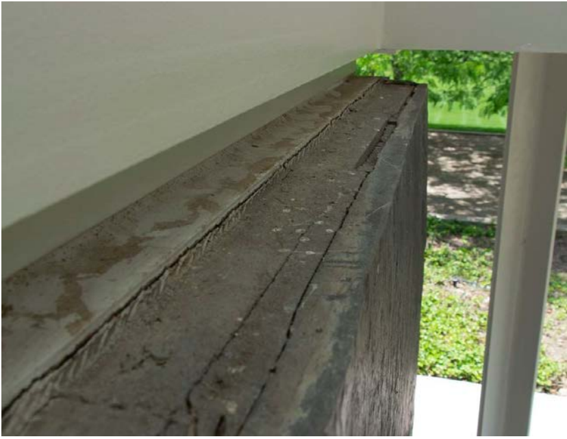
Figure 8 Top of slate slab with joint relatively intact. Note the difference in the joint width between the foreground and background of the photograph.
