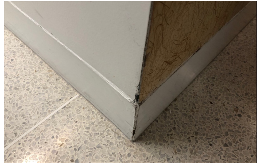
Fig. 6.6.20 Wear at metal base, plaster and wallpaper in corridor leading to Power Room, likely caused by housekeeping equipment. Date: June 2021. Photo credit: Scattergood Design
