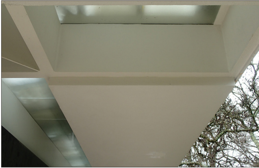
Fig. 6.4.5 Projecting soffit panel and exposed steel frame. Date: February 2019. Photo credit: Michael C. Henry
