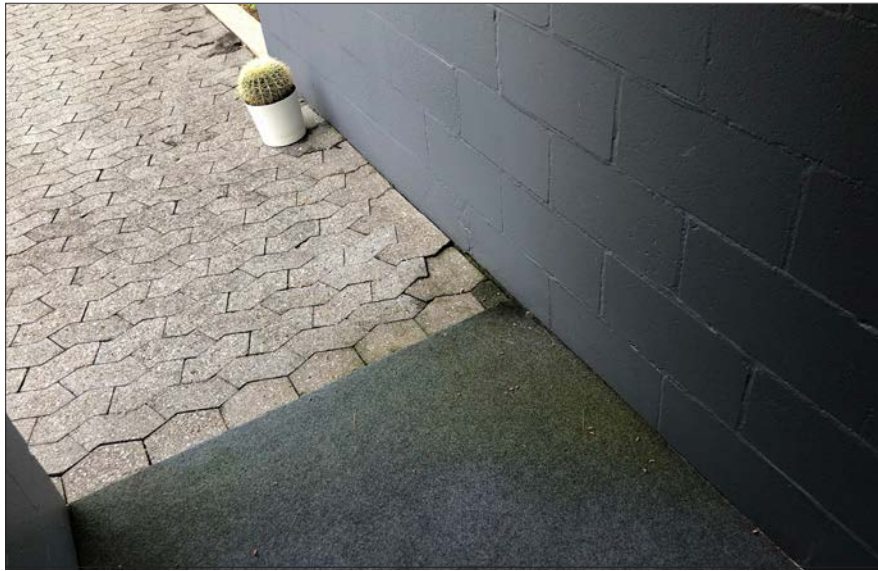
Fig. 6.17.7 Greenhouse/Office: misaligned and broken pavers adjacent to entrance. Date: June 2021. Photo credit: Scattergood Design
