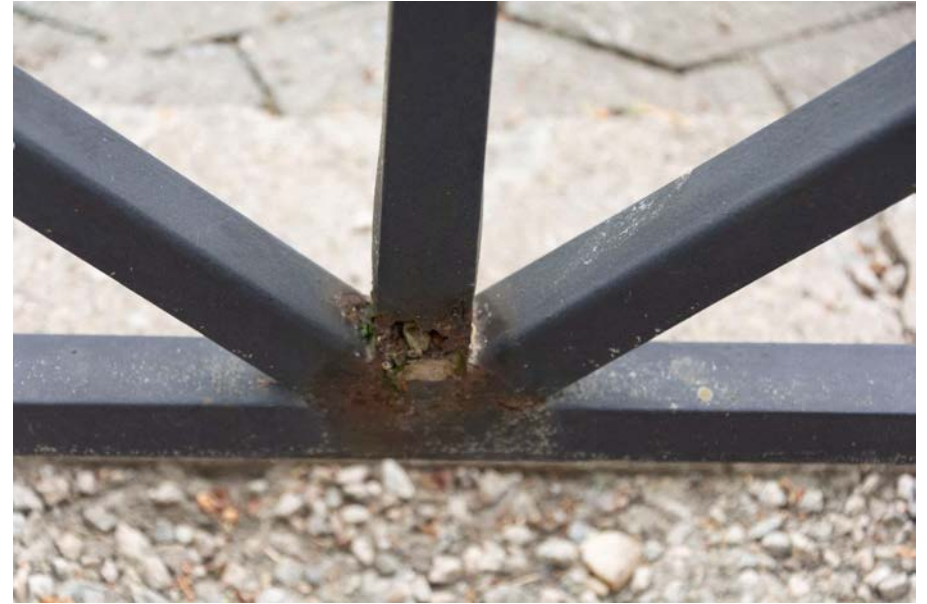
Figure 72 Corrosion to the point of loss at geometric gate, typical.
