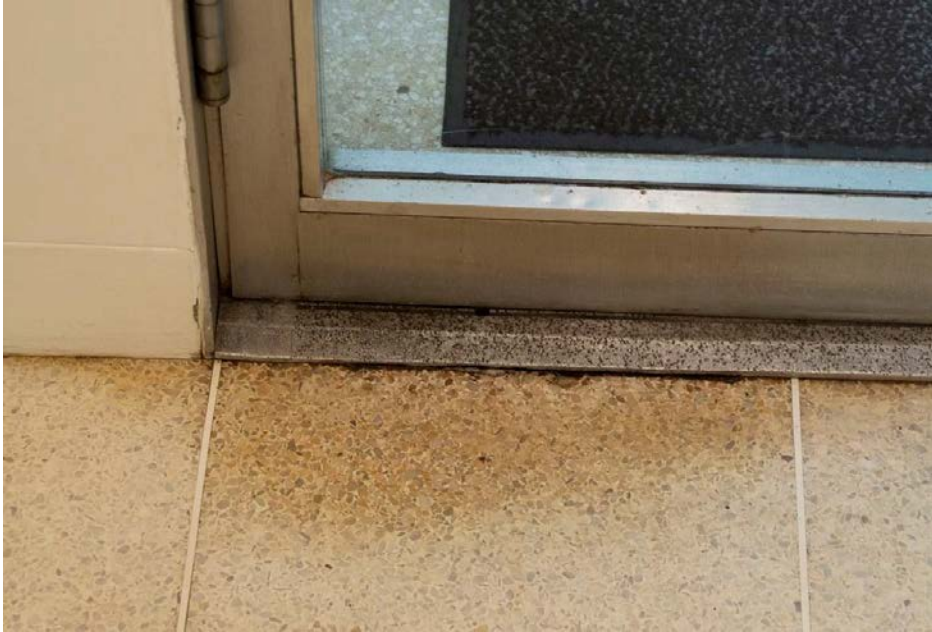
Figure 30 Pitted aluminum threshold, typical.
