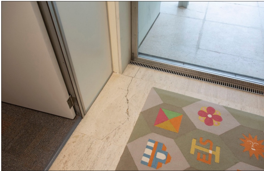
Fig. 6.2.10 Cracked travertine in Dining Room. Date: June 2021. Photo credit: Building Conservation Associates
