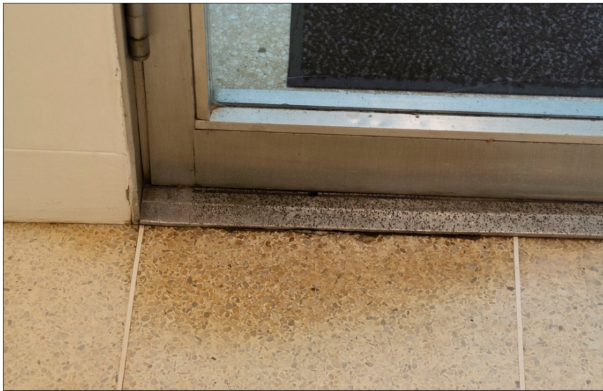
Fig. 6.7.3 Pitted aluminum threshold, typical. Date: June 2021. Photo credit: Building Conservation Associates
