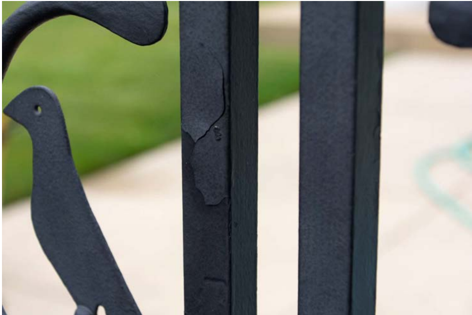
Figure 71 Early stages of paint failure at pool gate.
