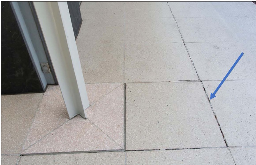
Fig. 6.2.7 Note mis-matched replacement terrazzo and widened joint at arrow, where sealant has failed, typical. Date: June 2021. Photo credit: Building Conservation Associates
