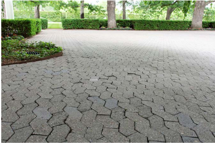
Figure 68 Isolated region of settlement near carport entrance.
