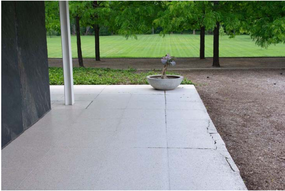
Figure 24 Broken terrazzo at edge, typical, likely due to the unsupported condition shown above.
