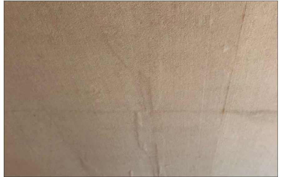
Fig. 6.17.10 Greenhouse/Office: stained ceiling tiles as a result of roof leaks. Date: June 2021. Photo credit: Scattergood Design
