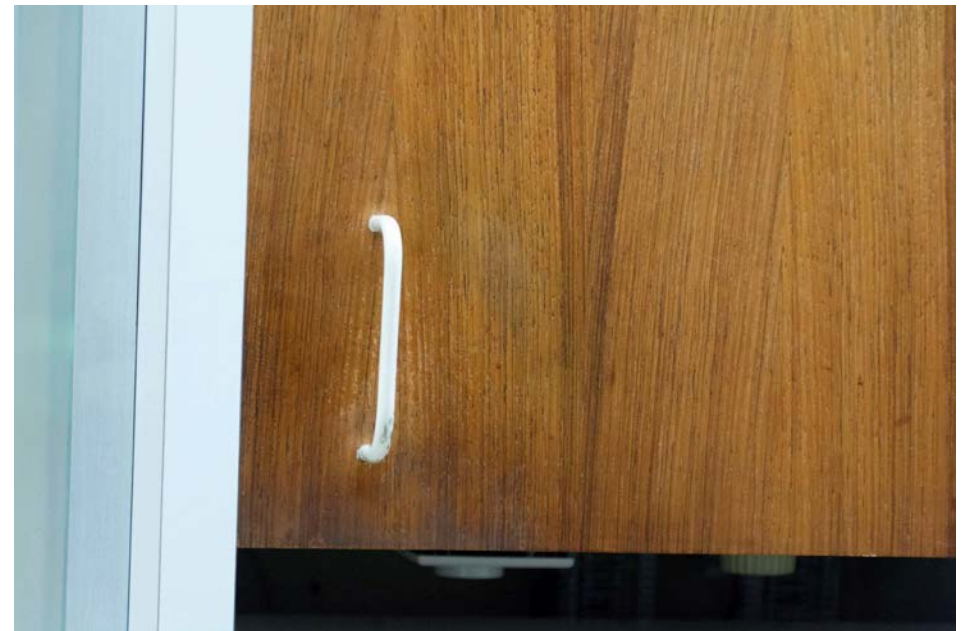
Figure 52 More subtle wear of veneer near cabinet handles, storage wall.
