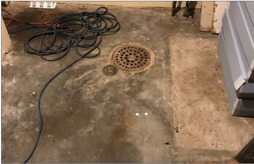
Fig. 6.17.11 Greenhouse/Office: evidence of drainage issues in mechanical area. Date: June 2021. Photo credit: Scattergood Design
