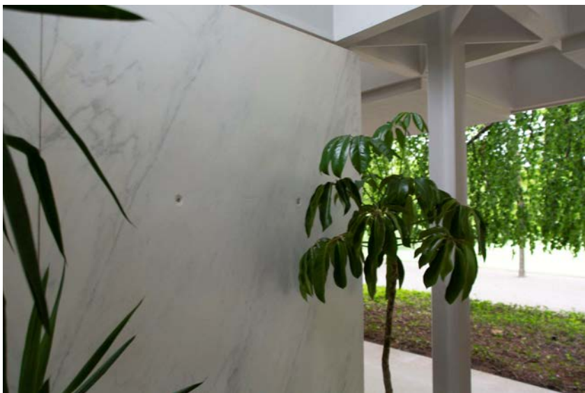
Figure 19 Two small losses at anchor points where art was formerly hung, west of house.
