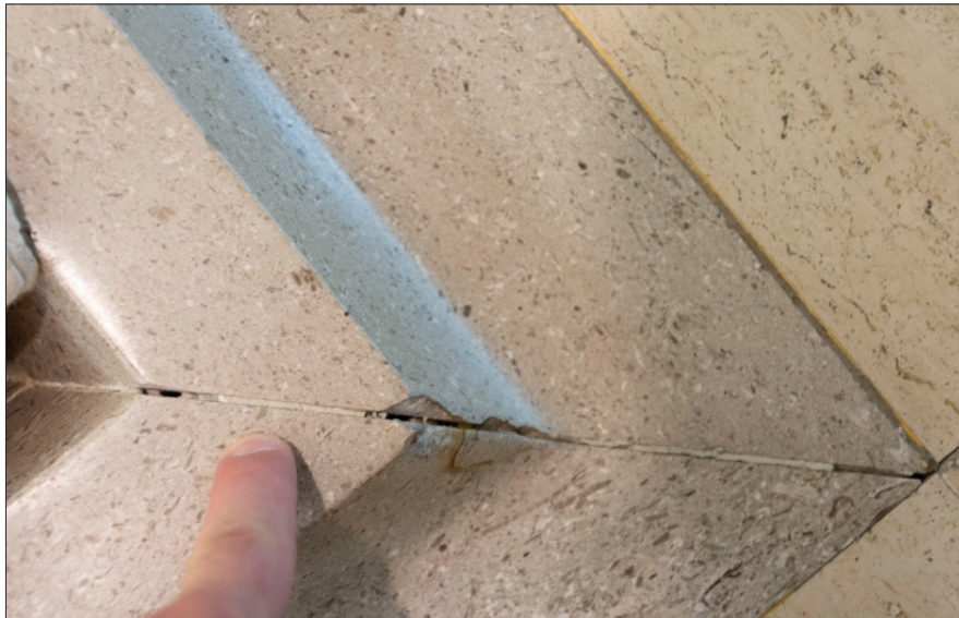
Fig. 6.2.11 Suspected original white grout at perimeter of conversation pit. Note the losses. Date: June 2021. Photo credit: Building Conservation Associates
