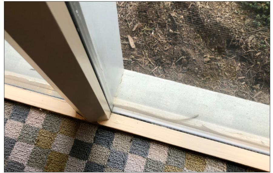
Fig. 6.17.9 Greenhouse/Office: view showing loose glazing putty/caulk at bottom of windows. Date: June 2021. Photo credit: Scattergood Design
