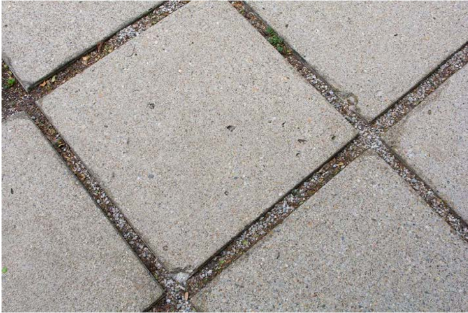
Figure 80 Small edge losses in concrete pavers.
