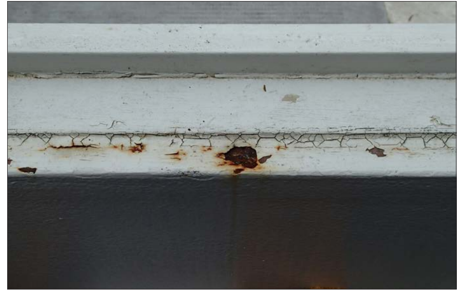
Fig. 6.3.5 Corrosion on the top of the parapet steel. Date: June 2021. Photo credit: Michael C. Henry
