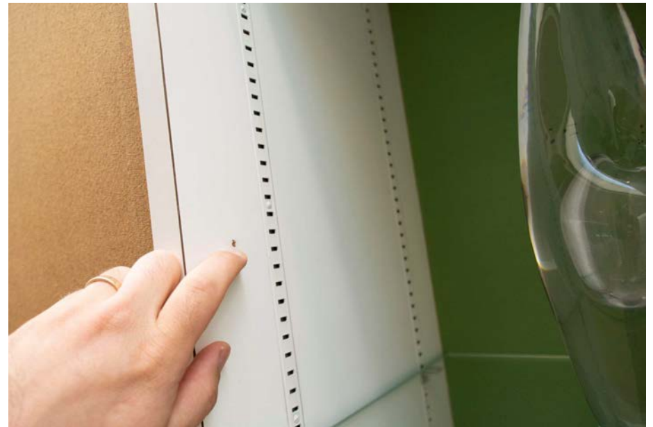
Figure 46 Small chips in storage wall Micarta.
