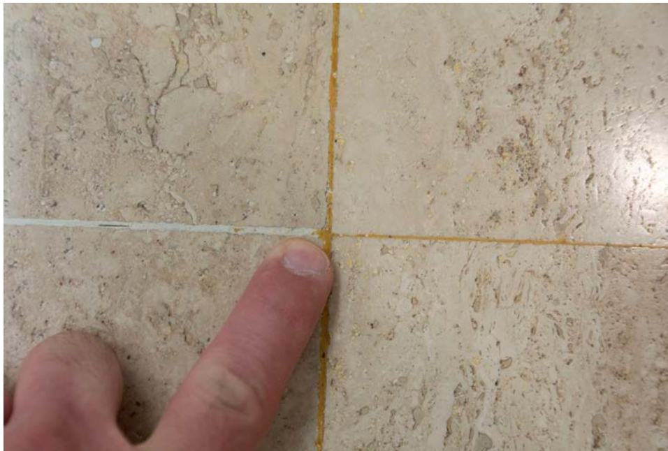
Figure 56 Yellowed later repair grout, typical.
