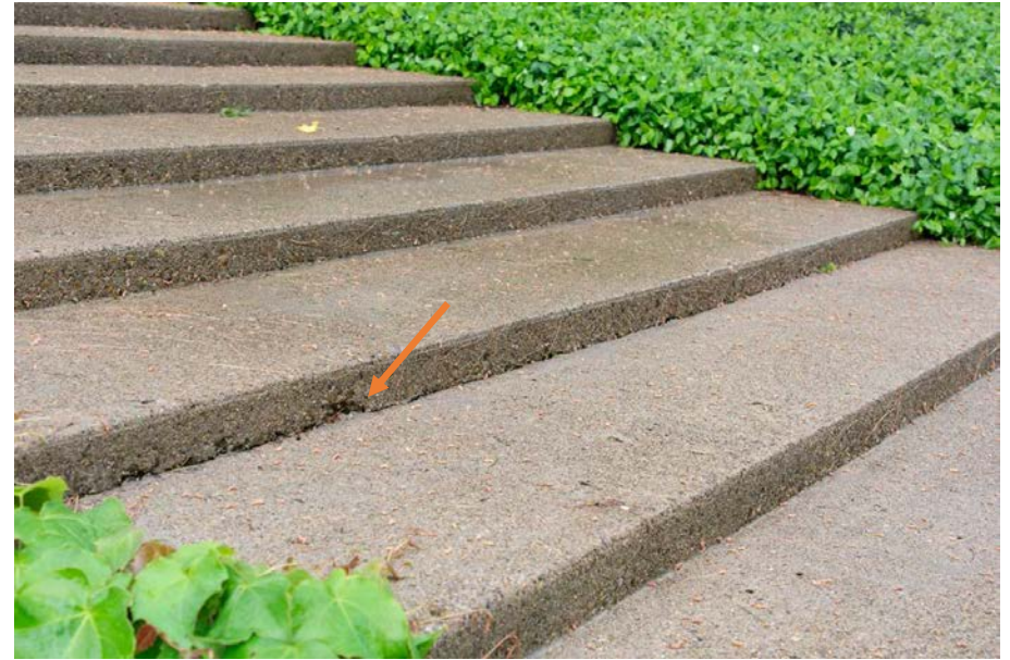
Figure 82 Small losses in monumental stair (arrow).
