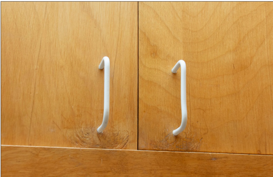
Fig. 6.8.10 Scratched veneer adjacent to wire pulls in Dressing Room. Date: June 2021. Photo credit: Building Conservation Associates
