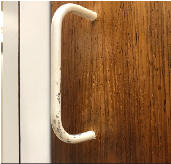
Fig. 6.8.9 Chipped paint on wire pulls and scratched adjacent wood veneer (likely as a result of cleaning) is a fairly typical condition, especially in the Kitchen. Date: June 2021. Photo credit: Scattergood Design
