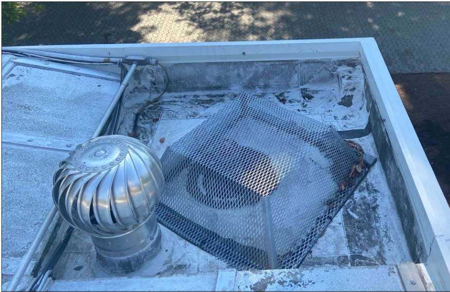
Fig. 6.4.9 Turbine ventilator and debris guard on roof drain on corner roof bay. Note electrical conduits and cables for security cameras and for heat-tracing at the roof drain. Date: June 8, 2020. Photo credit: Newfields.
