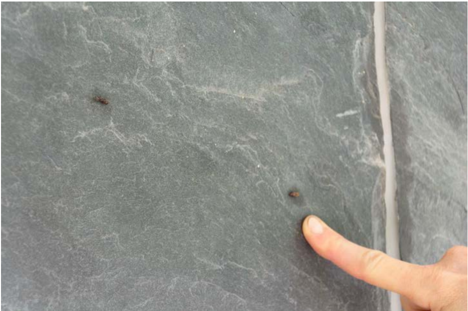
Figure 13 Detail of suspected guano showing apparent staining in the vicinity.
