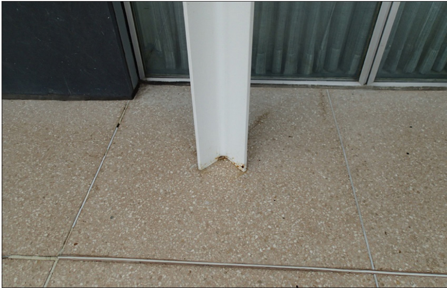
Fig. 6.3.3 Note paint flaking and corrosion at base of column. Date: 2019. Photo credit: Michael C. Henry
