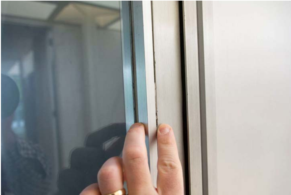
Figure 31 Sealant at all points in the glazing assemblies was typically failing.
