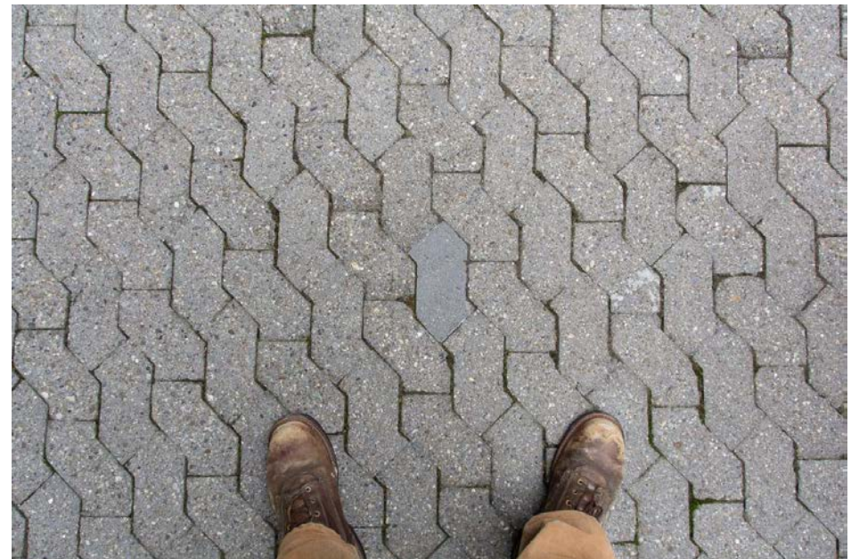
Figure 67 Recently installed paver. With binder intact, the unit appears mismatched.
