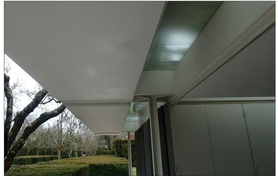
Fig. 6.4.19 Condensation on plaster soffits. Date February 2019. Photo credit: Michael C. Henry
