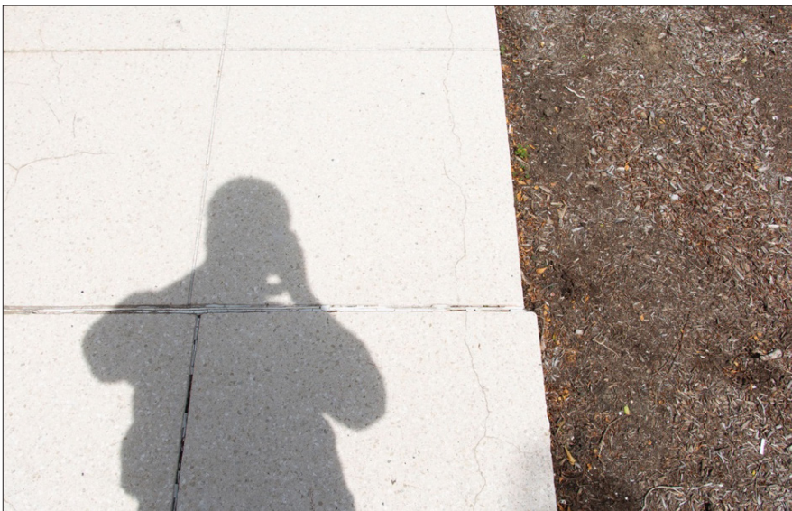
Fig. 6.2.3 Extent of displacement at the southwest corner of the house as evidenced by the protruding units in the bottom of the photograph. Note also that every unit is cracked. Date: June 2021. Photo credit: Building Conservation Associates
