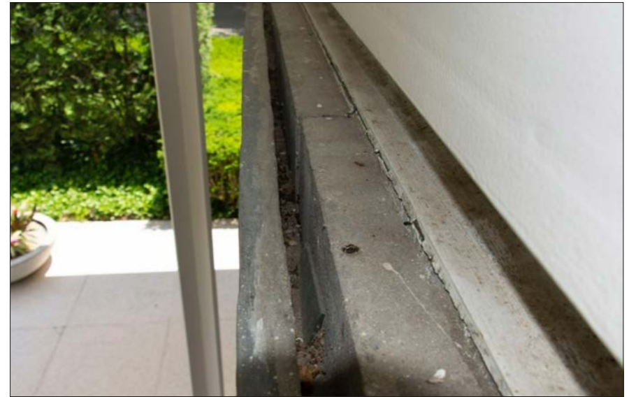
Fig. 6.6.12 Top of slate slab with joint entirely open. Note the large amount of debris in the cavity. Date: June 2021. Photo credit: Building Conservation Associates
