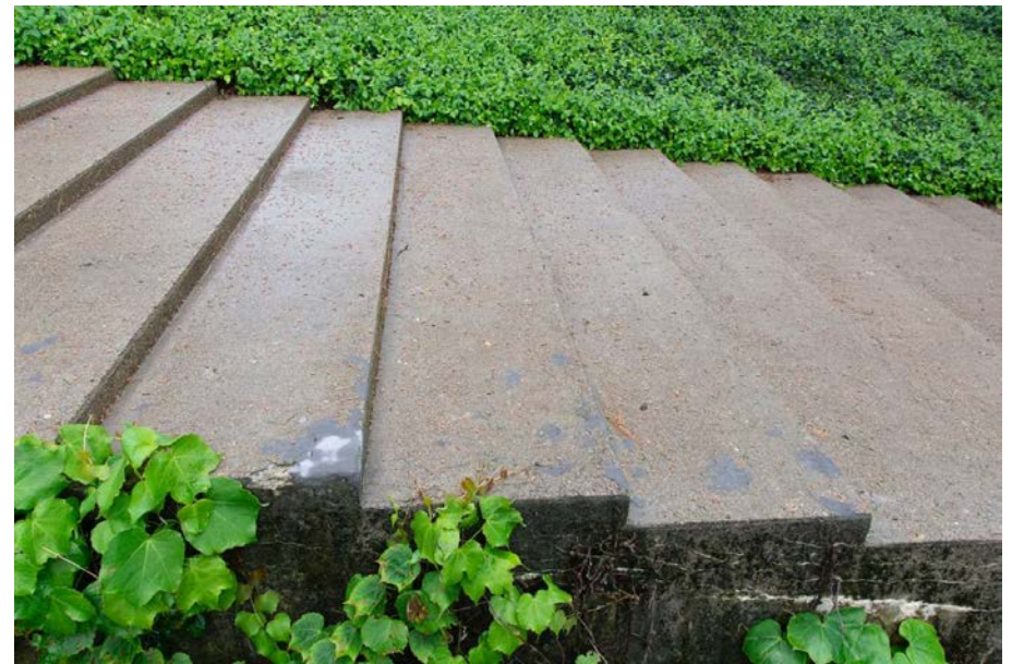
Figure 83 Incompatible patches on monumental stair.
