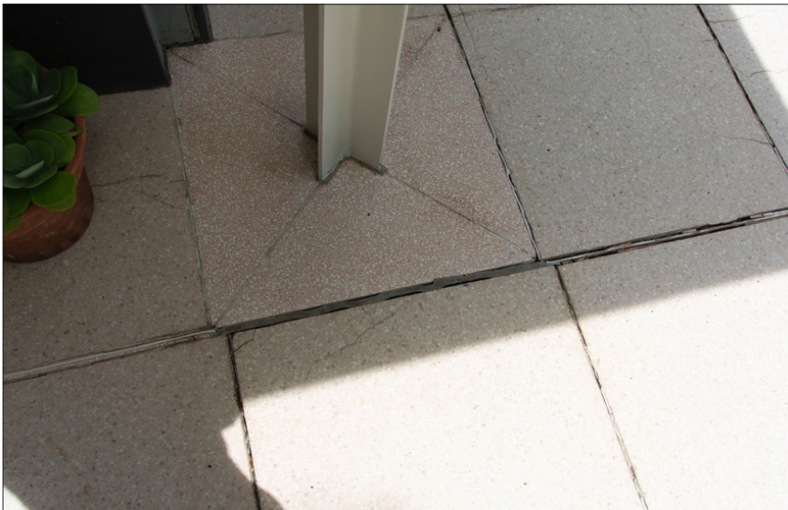
Fig. 6.2.2 Cracked and displaced terrazzo at the southwest corner of the house. Note how the joint lines have shifted. Date: June 2021. Photo credit: Building Conservation Associates
