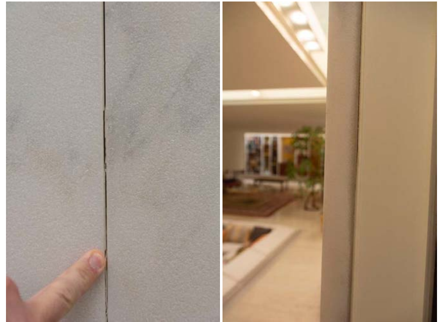
Figure 36 Failing grout and sealant joints at perimeter of marble slabs.
