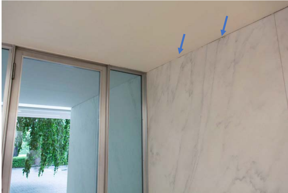
Figure 37 Small chips at top of slab (arrows) presumably from picture hangers such as those visible at right of photo.
