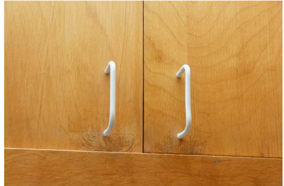
Figure 51 Heavily scratched veneer near cabinet handles, walk-in closet.
