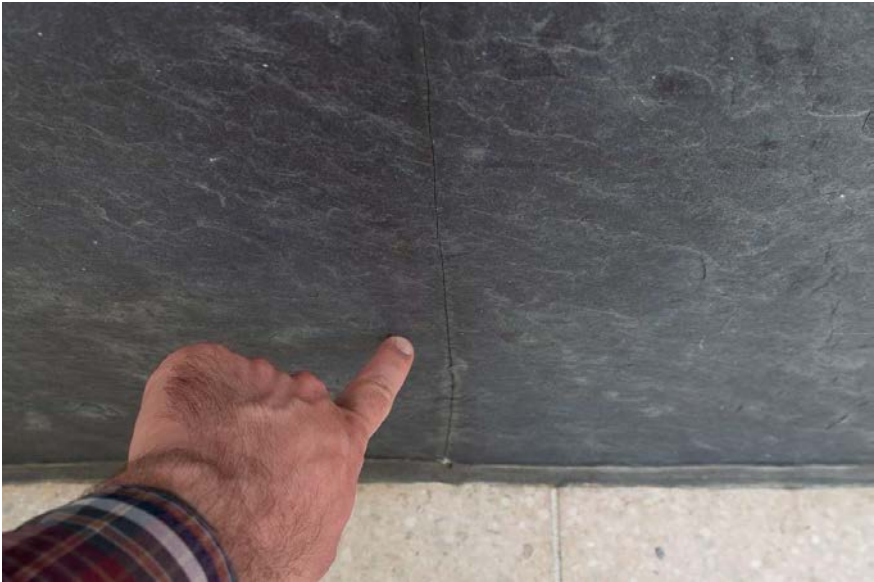
Figure 10 Gaps in sealant show what appears to be the edge of the terrazzo (arrows), which stops short of the slate. Note also that the divider strip cover clearly stops short of the slate.
