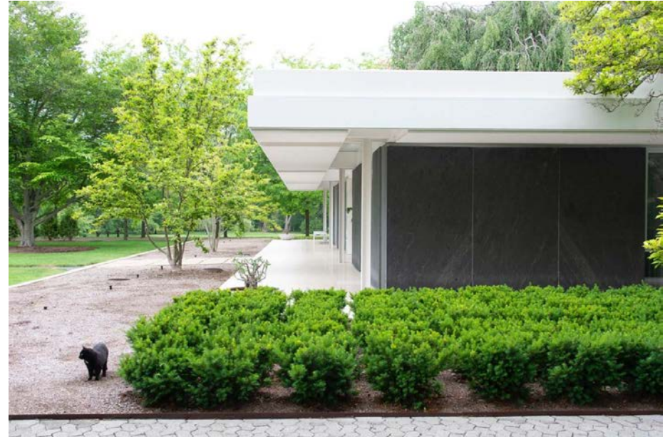
Figure 2 Southeast corner of the house, looking west. Note the row of white steel X-shaped columns. Both tiers of the soffit are C-shaped steel beams, oriented to open inwards.
