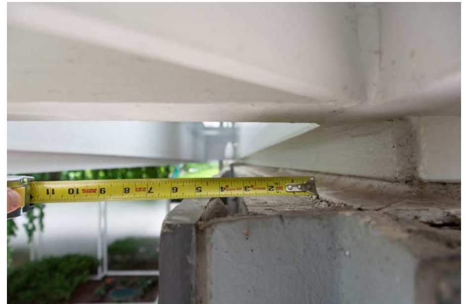
Figure 7 Gap between concrete backup and slate slab in excess of 1". However, note that the joint between the steel angle in the foreground and the slate slab is close to the 3/8" specified in the drawings.
