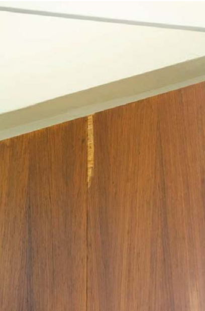
Figure 50 Largest loss of veneer, at storage wall door that may contact a steel column when opening.
