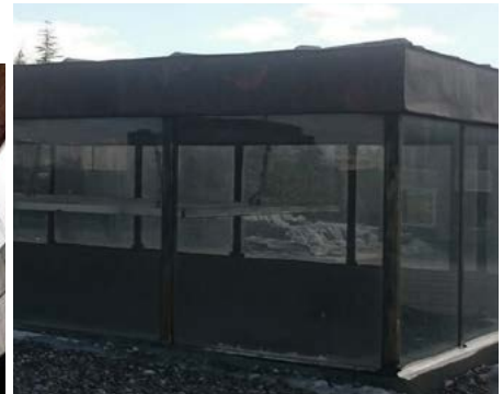
Figure 12: Details from the skylight.
