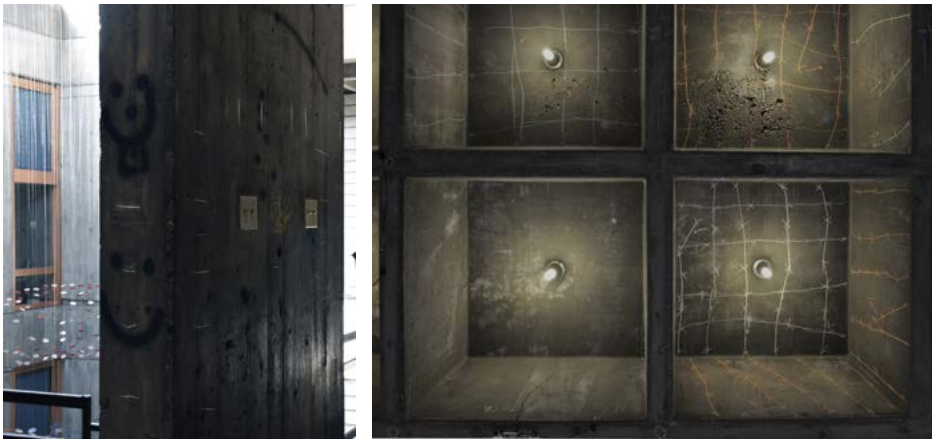
Figure 22: Rebar location of a column, waffle slab in F Block.
