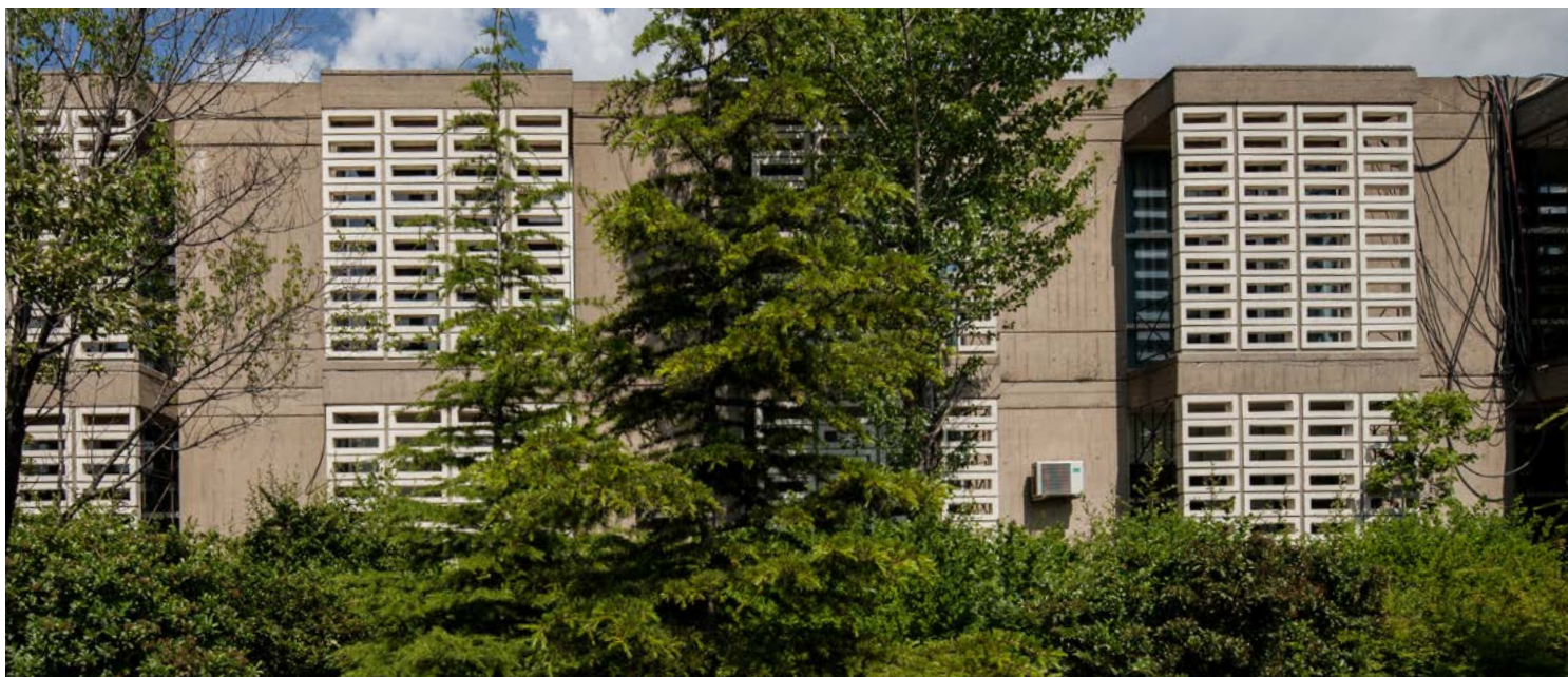
Figure 2: Passive shading elements on the west façade.
