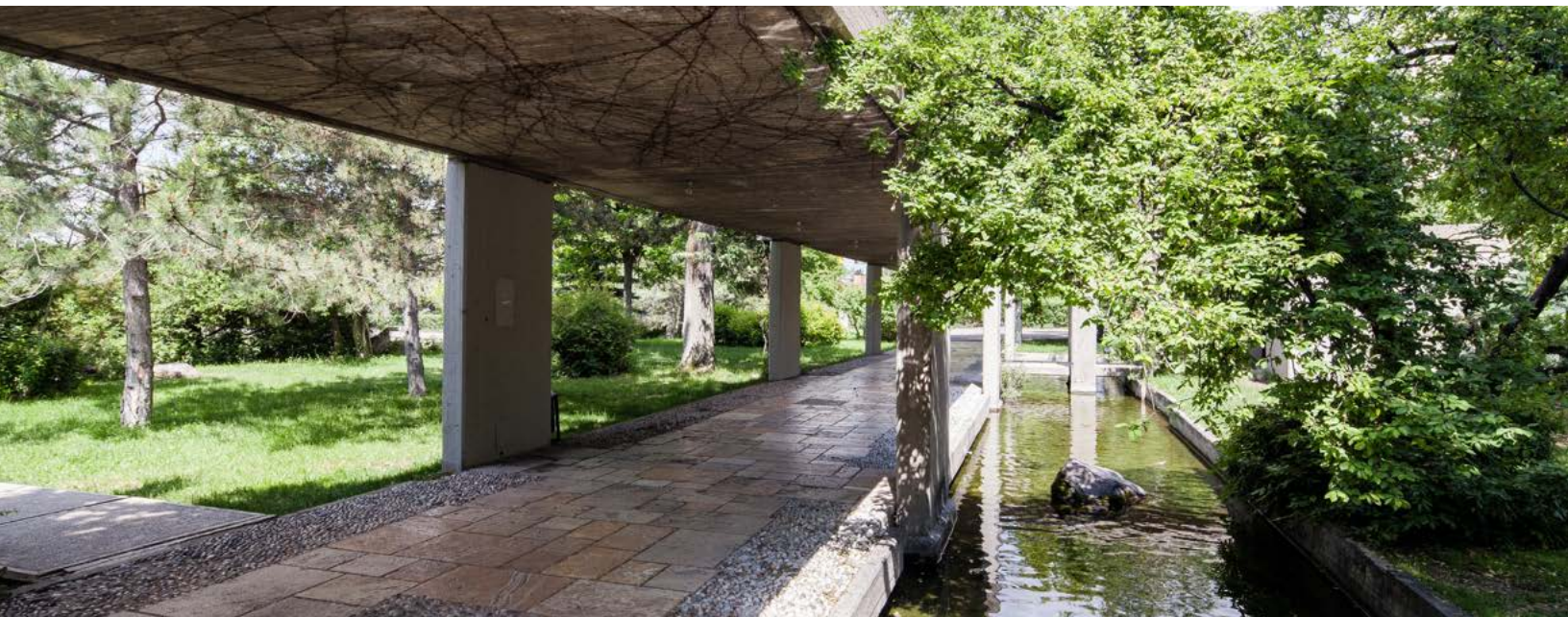
Figure 1: Main entrance during summer time.
