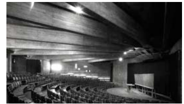
Figure 6: Interior view from the Amphitheatre, showing the structural system of concrete beams.
