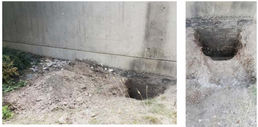
Figure 25: General view of the observation hole.
