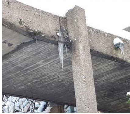
Figure 9: Detachment on exposed concrete surfaces in the form of multiple flakes and scales showing that detaching surfaces are the priority areas at risk of loss.
