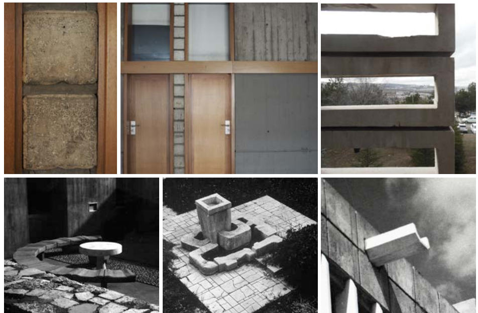
Figure 15: Different usages of cement: partition walls, brise soleils, water spouts, seating units, tables and sculptures.
