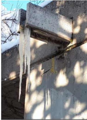
Figure 10: Exposed concrete surfaces suffering from material loss together with detachments are susceptible to frost damage, especially when they get wet.
