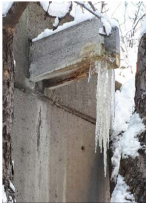
Figure 10: Exposed concrete surfaces suffering from material loss together with detachments are susceptible to frost damage, especially when they get wet.
