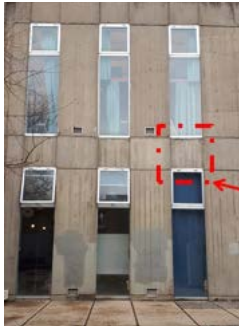
Figure 9: Detachment on exposed concrete surfaces in the form of multiple flakes and scales showing that detaching surfaces are the priority areas at risk of loss.
