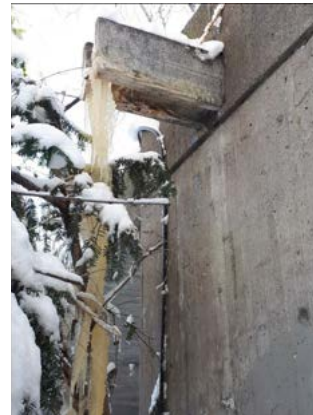
Figure 10: Exposed concrete surfaces suffering from material loss together with detachments are susceptible to frost damage, especially when they get wet.
