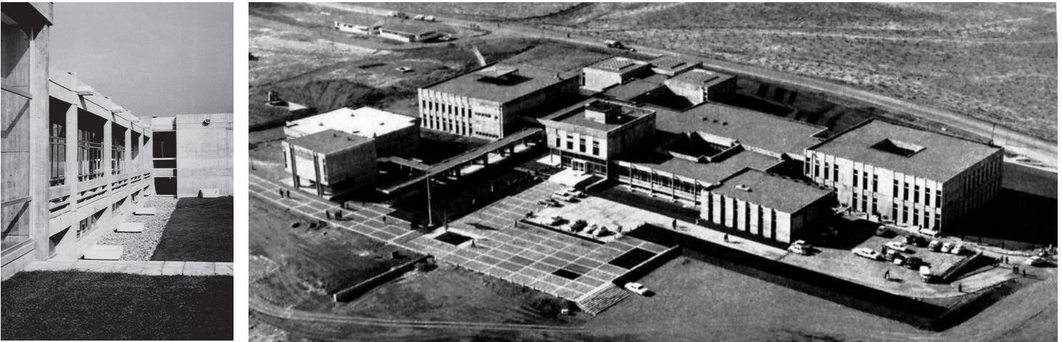
Figure 10: Black and white photographs of the faculty building, 1960s.
