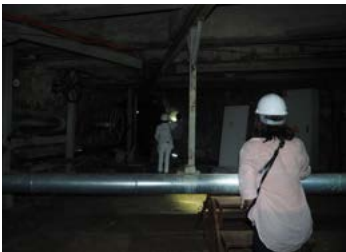
Figure 4: Photos from the original gallery, captured during the infrastructural inspection trip.
