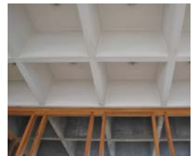
Figure 116: 1.20x1.20m waffle slab system
