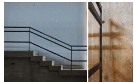
Figure 124: Black-painted thin iron balustrades- applied
