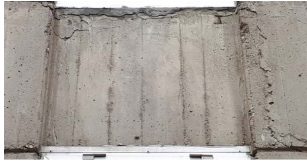
Figure 9: Detachment on exposed concrete surfaces in the form of multiple flakes and scales showing that detaching surfaces are the priority areas at risk of loss.
