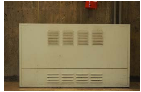
Figure 122: Fan coils of the METU Faculty of Architecture -A reproduction of the first fan coil fabricated in Turkey
