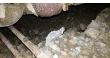
Figure 29: Gap underneath the slab.
