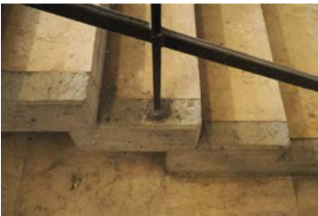
Figure 85: Exposed concrete sidesurfaces of the stairs.
