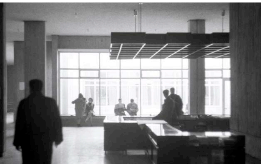
Figure 9: Black and white photographs of the faculty building, 1960s.
