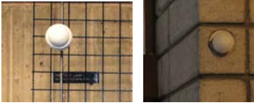
Figure 2: The original lamp over the door frames.
