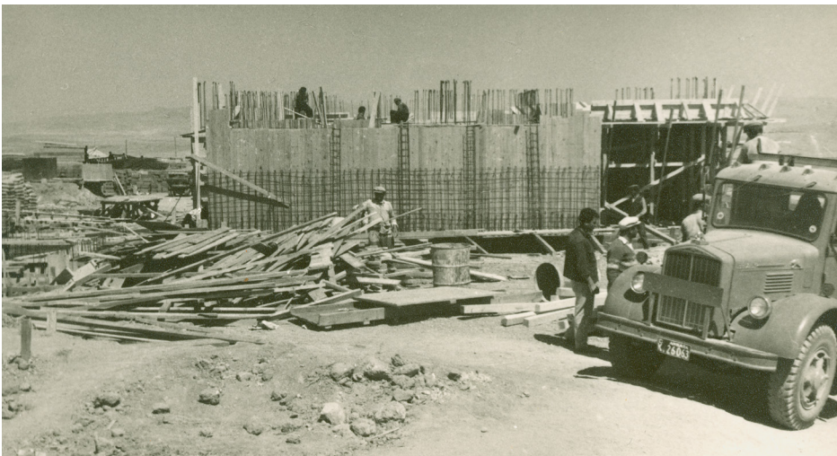
Figure 22: Construction process of METU Faculty of Architecture Main Building, METU Archive. “The horizontal bars have been placed as 8/20.” 12
