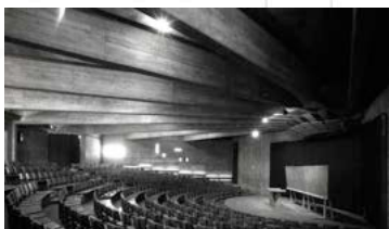
Figure 12: Interior view from the Amphitheatre, showing the structural system of concrete beams.
