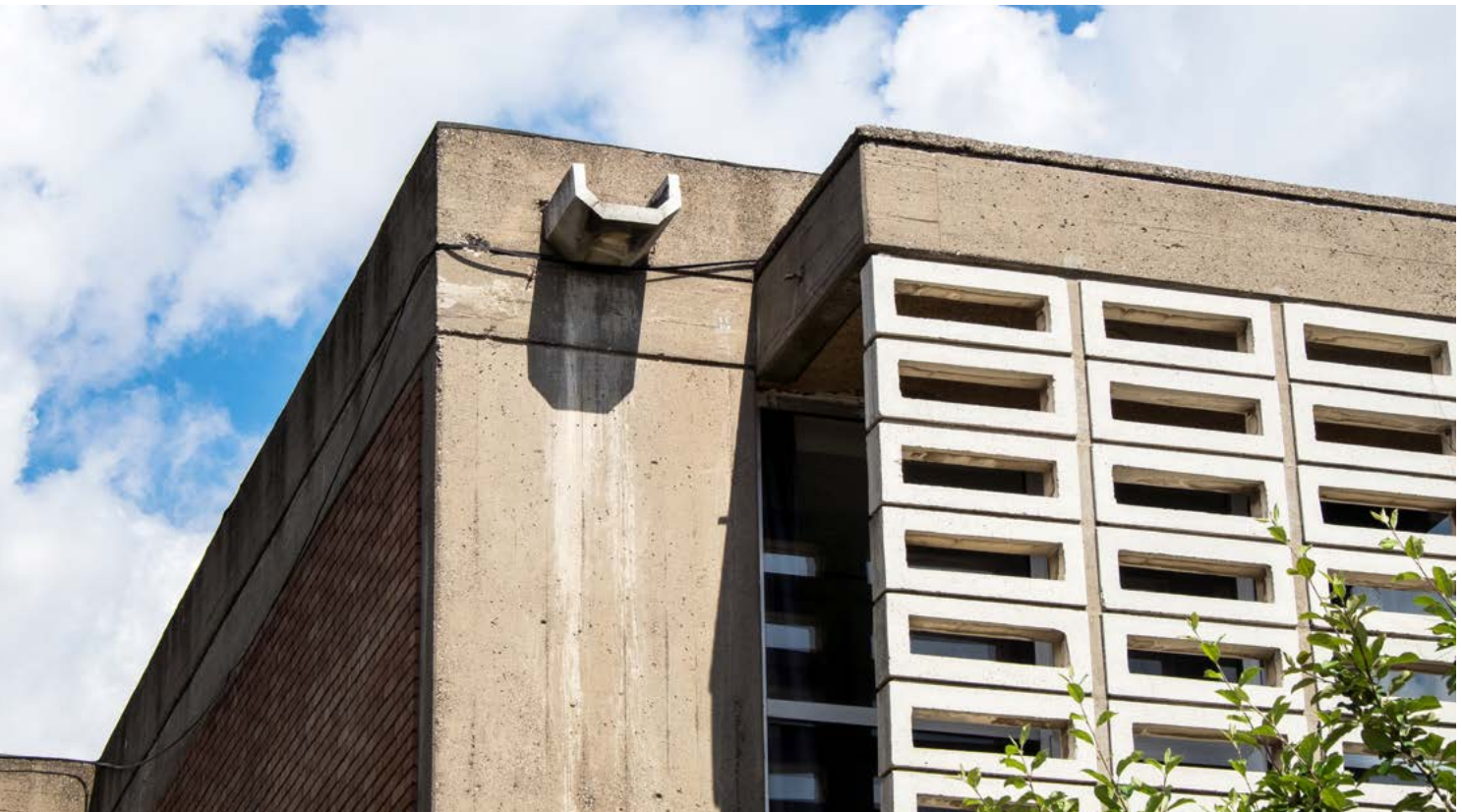
Figure 21: Brise-soleil shading elements on the west-facing classrooms
