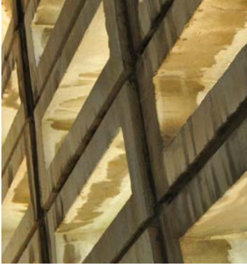
Figure 22: Brise-soleil shading elements on the west-facing classrooms
