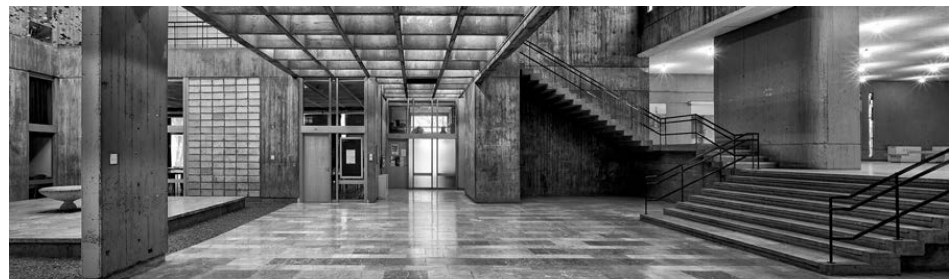
Figure 5: Waffle slab view on the selected part of the building, taken by Cemal Emden, retrieved from http://www.cemalemnden.com/ .
