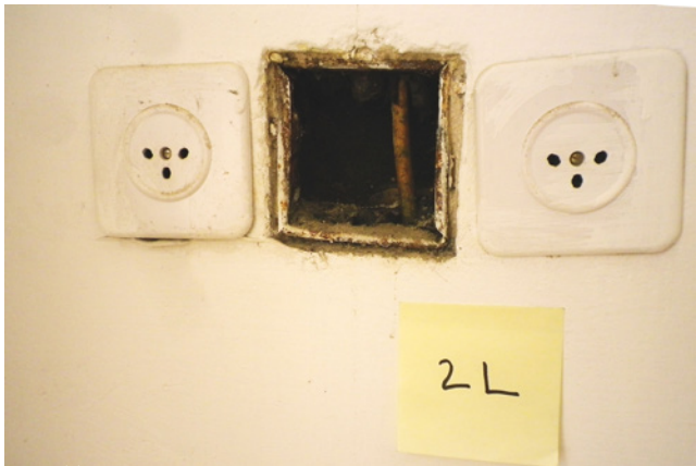
Fig. 144 Original sockets and electrical installations, 2015
