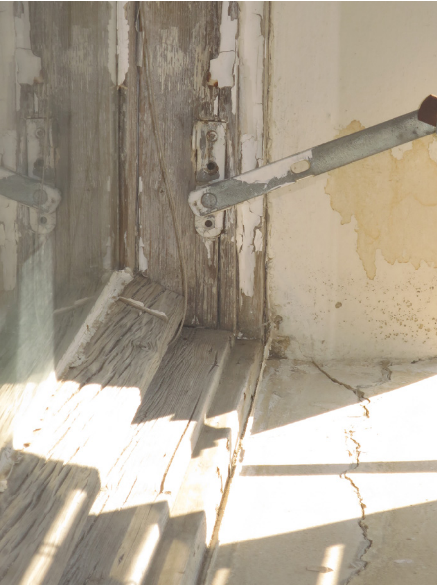
Fig. 176 Paint peeling off an original window frame, 2015
