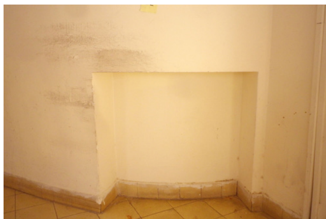
Fig. 123 Round corner, plastered wall with terrazzo base tiles in room 02.L, original radiator recess, 2015
