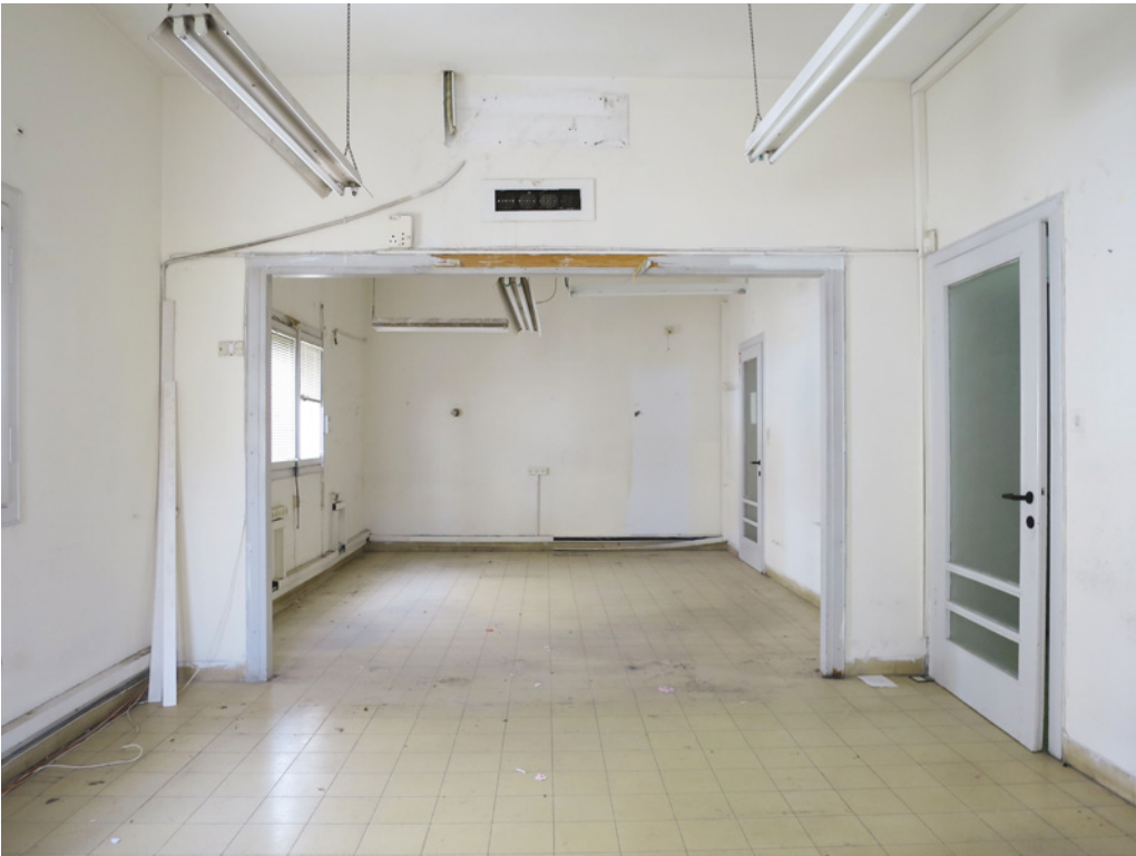
Fig. 116 Wall opening formerly closed by a folding door, third floor, 2015
