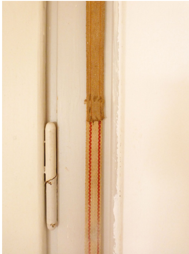
Fig. 106 Repaired roller shutter belt, upper part probably original, 2015
