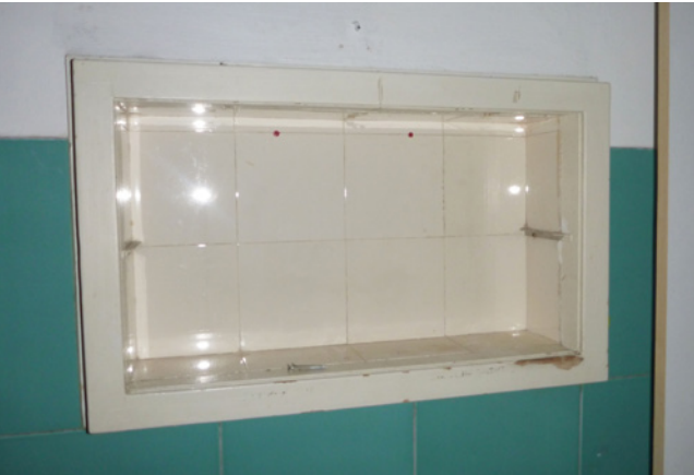
Fig. 127 Small bathroom cabinet, originally with sliding glass panels (type S.2), 2015
