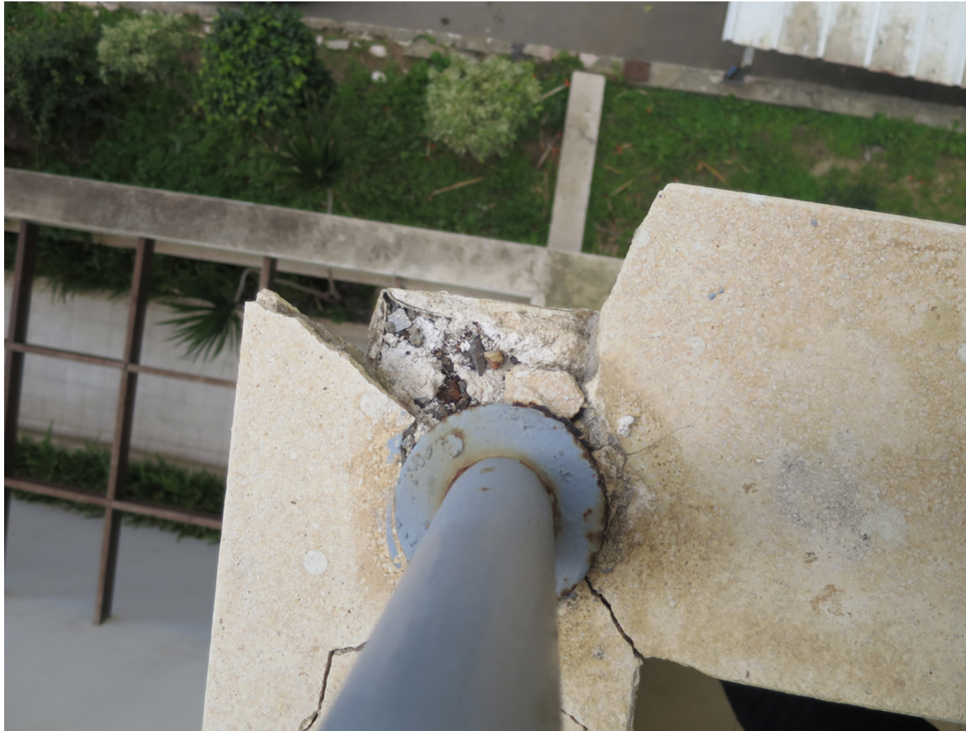
Fig. 174 Damaged terrazzo coping on the balcony, 2016
