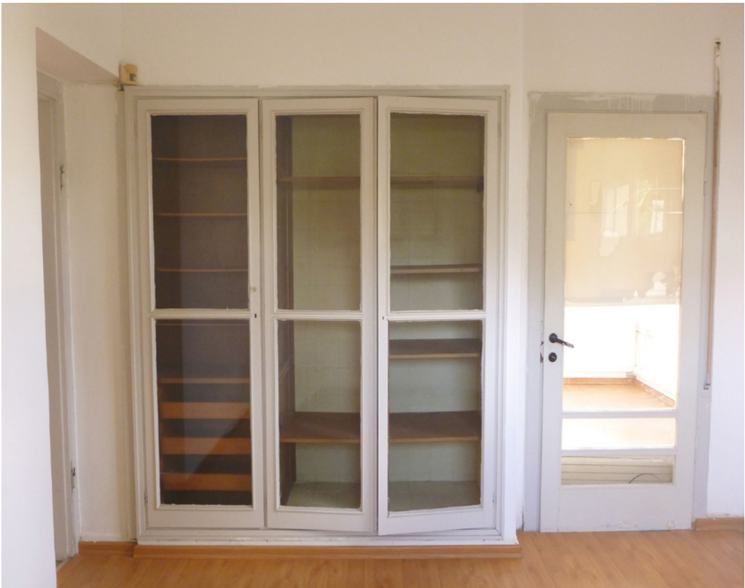
Fig. 137 Huge original built-in cupboard in room 02.O, cabinet on the left, wardrobe with tiles on the inner walls; on the right, glazed doors (type S.8), 2015
