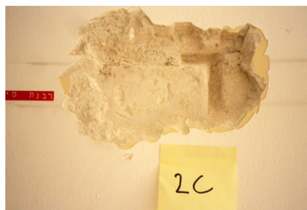
Fig. 125 Silicate bricks, sampling in room 02.C, 2015
