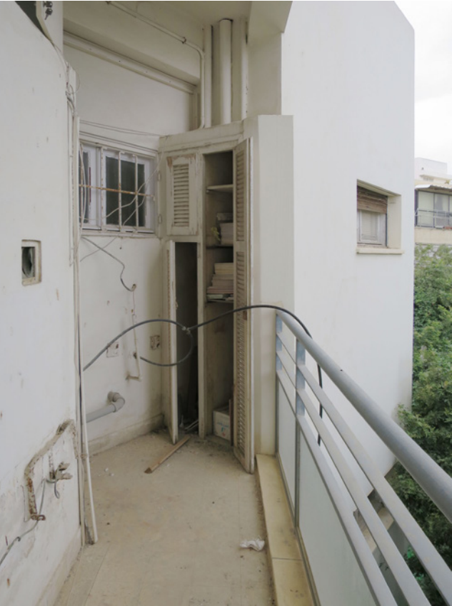
Fig. 126 Built-in cabinet on the balcony 01.K partly used for laundry reached from the bathroom 01.P through a hatch (type S.1), 2015
