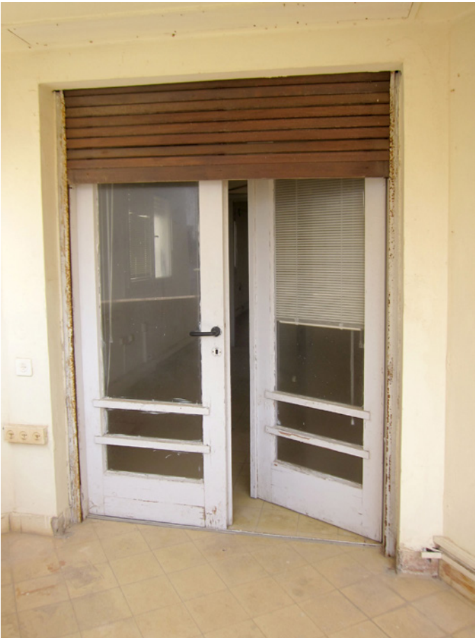
Fig. 110 Balcony door with roller shutters, 02.U, 2015
