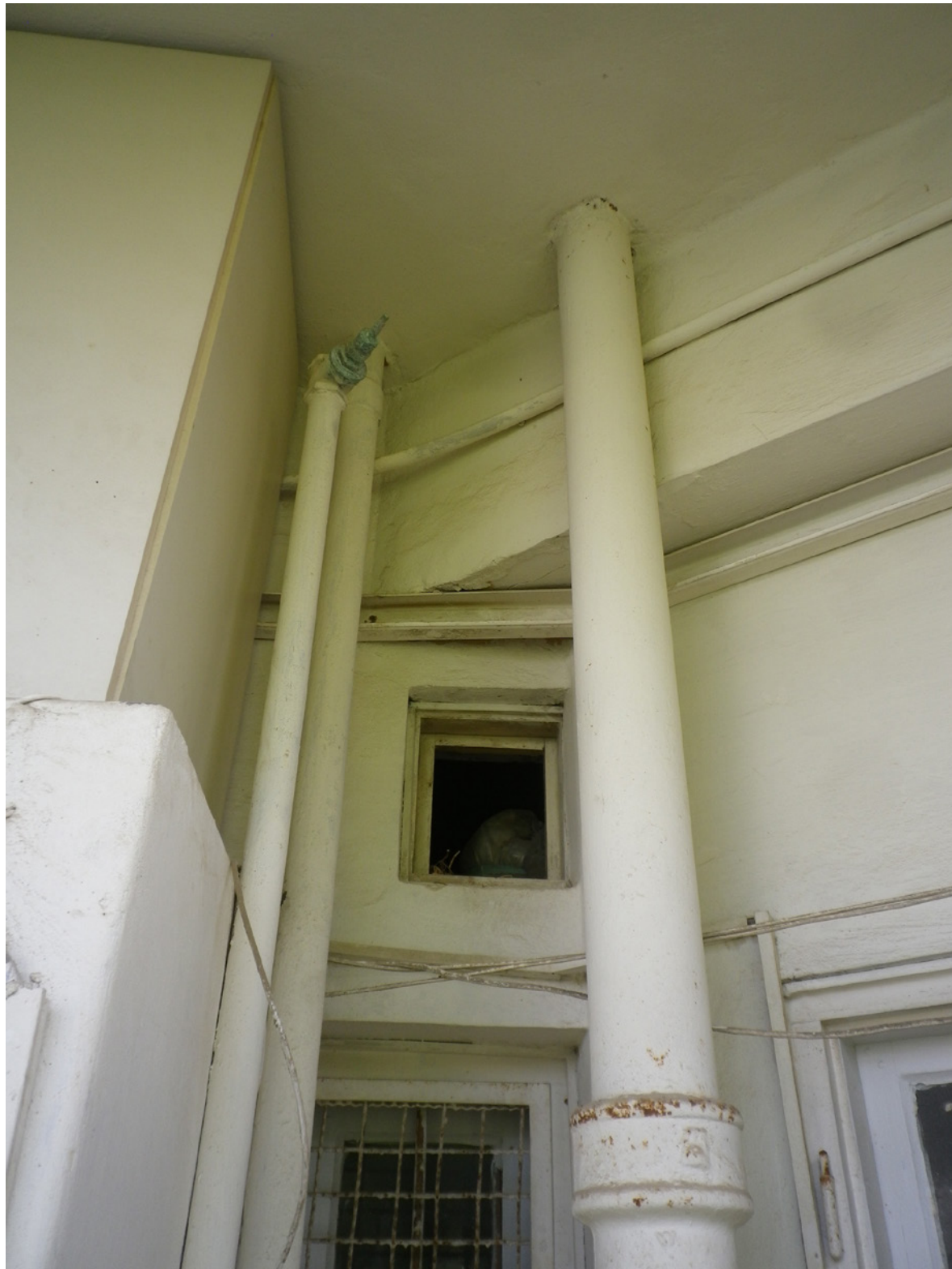
Fig. 38 Original water supply and wastewater lines on the utility balcony 02.K, 2015
