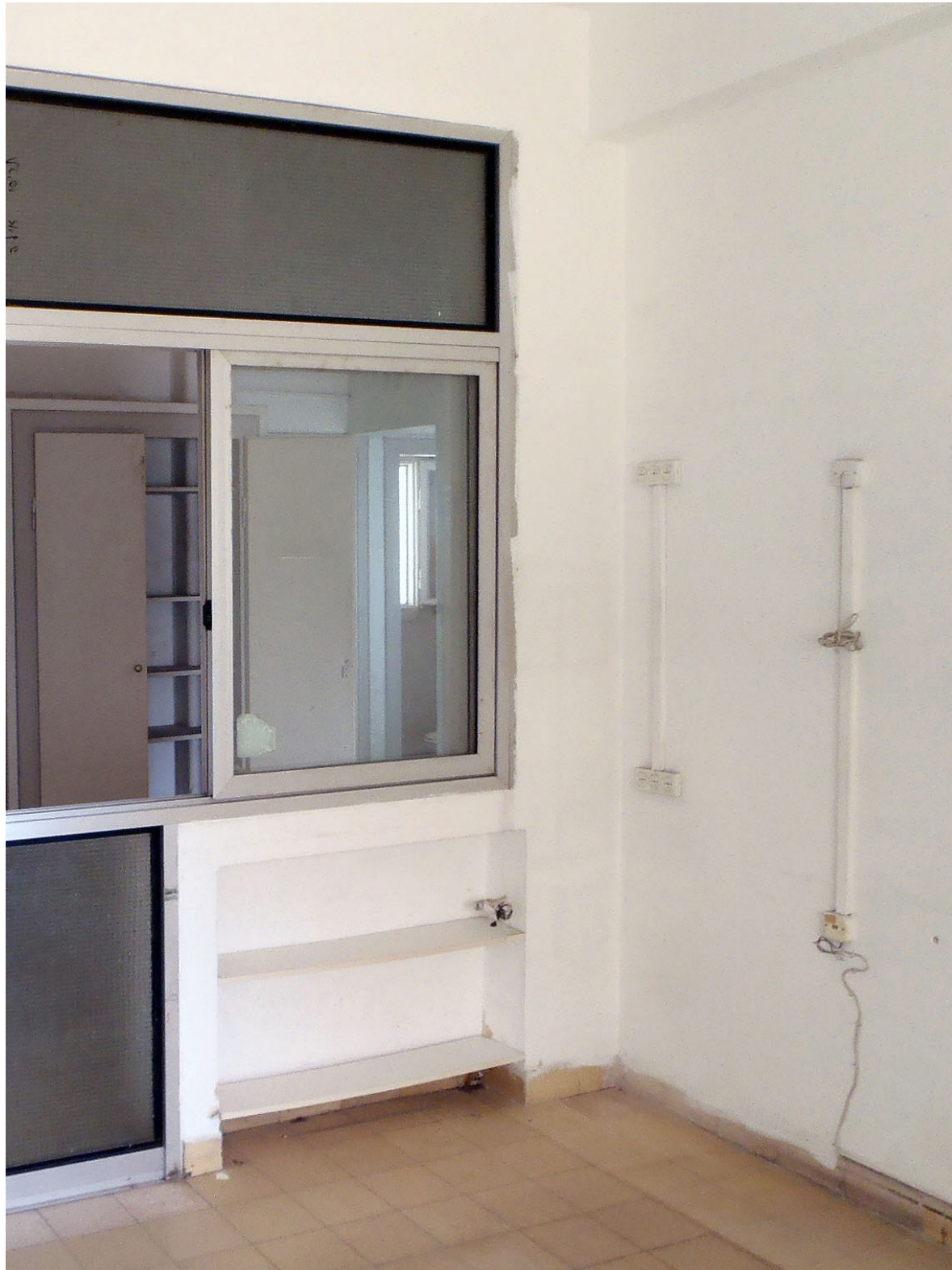
Fig. 34 Radiator recess in room 02.B with remains of a heating valve, 2015
