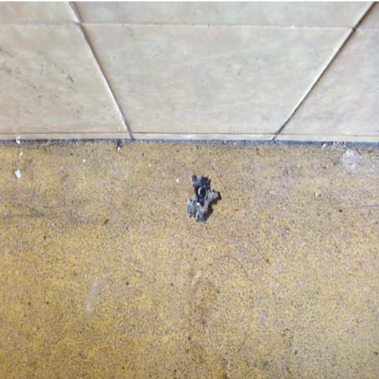
Fig. 121 Original terrazzo floor in the staircase, metal fixing for a carpet, 2015
