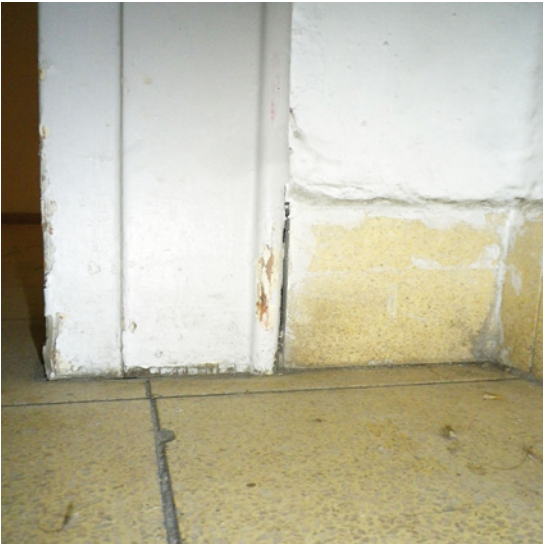
Fig. 120 Original tiles on the floor, connection between base tile and door frame, 2015
