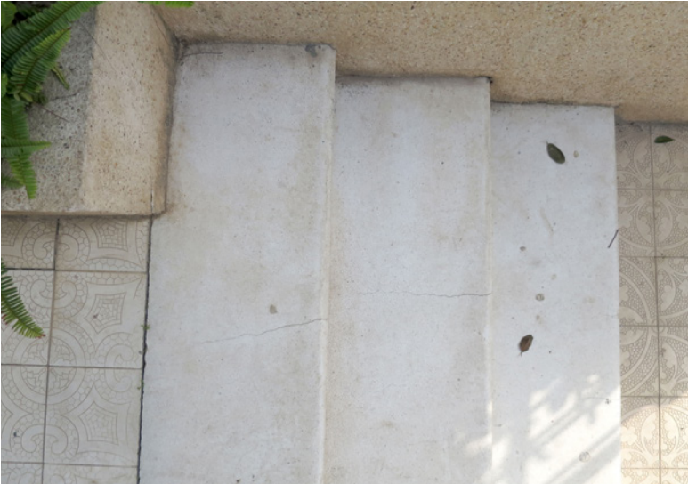
Fig. 119 White terrazzo steps on the entrance path. On the right side: cement replacement tiles; on the left side: original tiles, 2016
