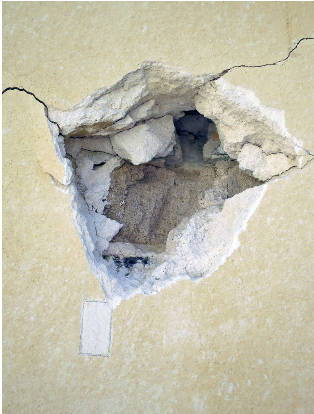
Fig. 35 Crack in the plaster where the wall material changes (bricks/concrete), roof zone of the staircase, 2016
