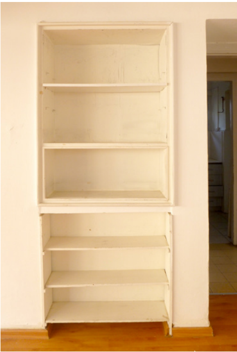
Fig. 138 Original built-in cabinet in room 02.N, new shelves added in the lower part (type S.9), 2015
