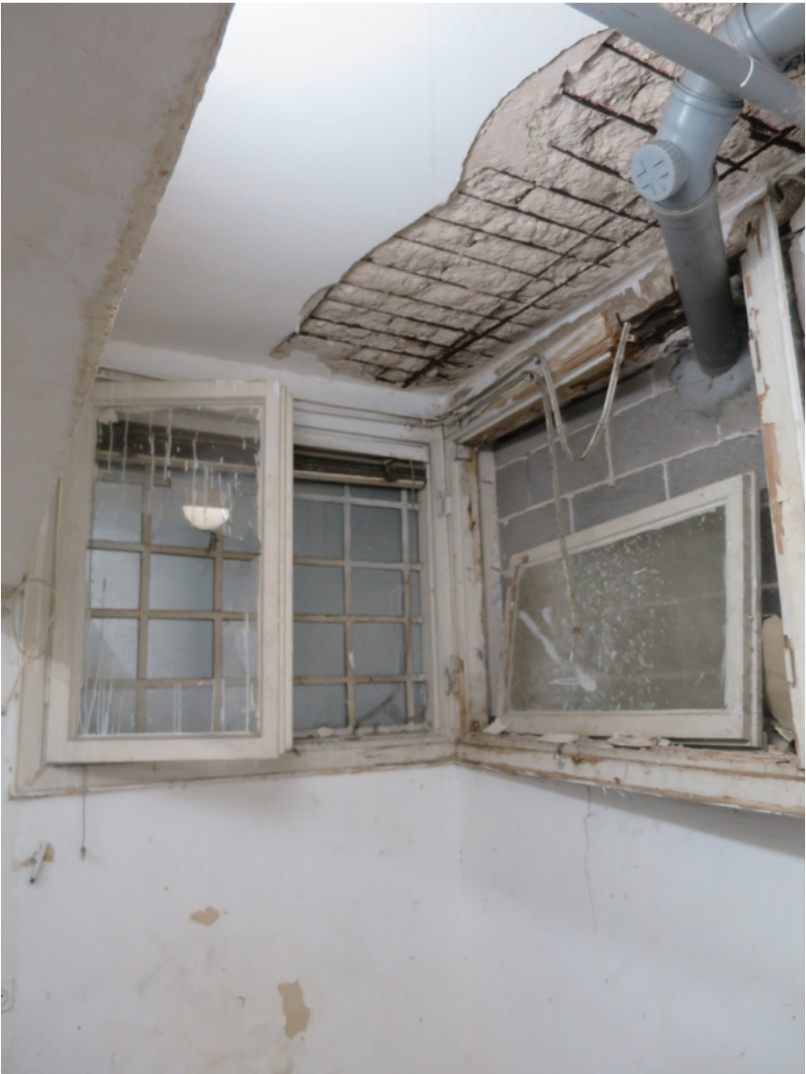
Fig. 175 Corroded reinforcement of a concrete ceiling in the basement, 2016
