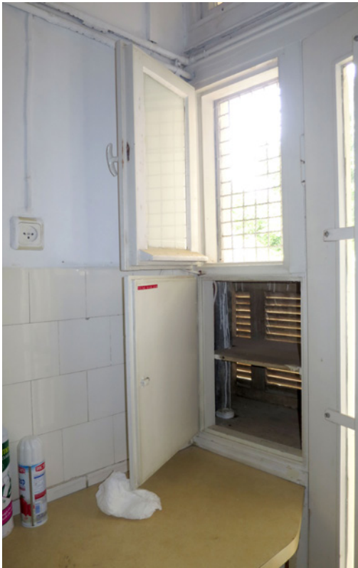
Fig. 129 Wall-mounted food storage cabinet with a hatch in kitchen 02.G (type S.3), 2015
