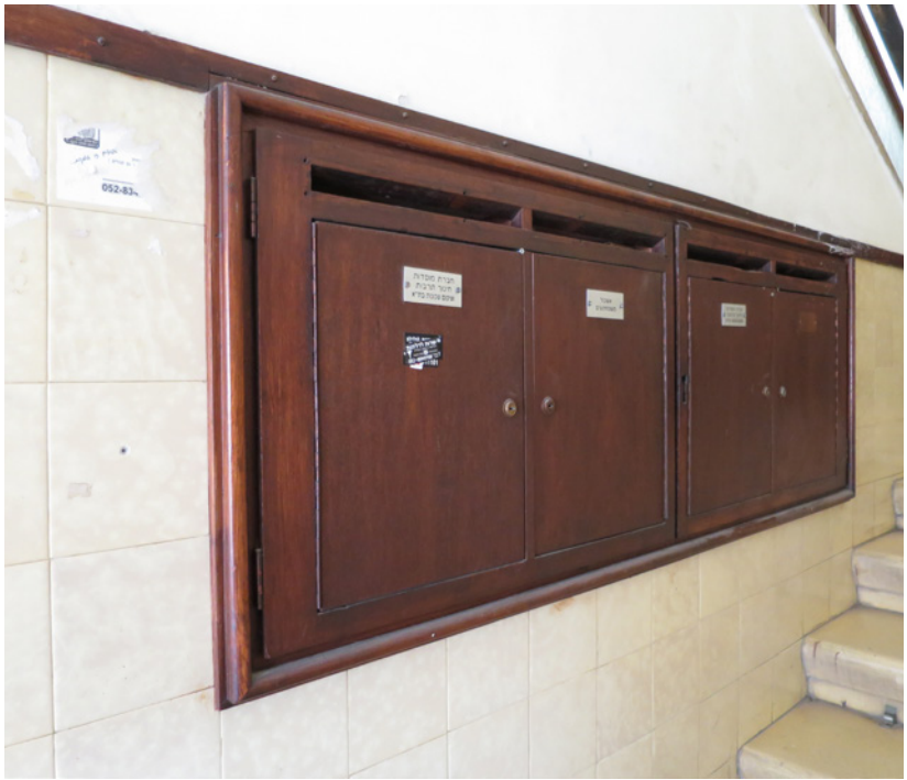
Fig. 139 Original built-in mailboxes with a storage space behind, entrance hall (type S.11), 2015
