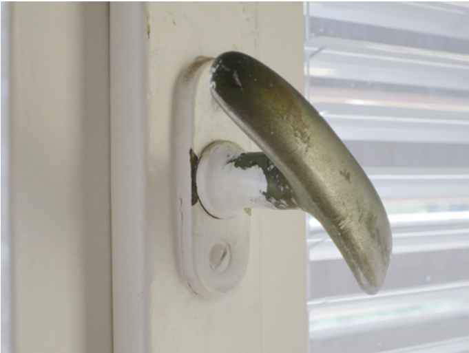
Fig. 111 Window handle, nickel silver, probably produced by the German producer „wehag“ (Wilhelm Engstfeld Heiligenhaus AG), 2015
