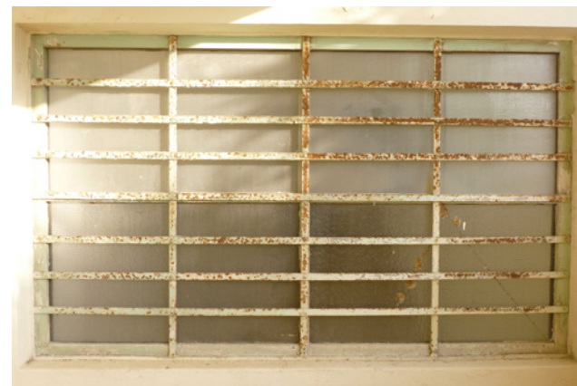
Fig. 109 Staircase window, upper part with two sliding sashes, 2015
