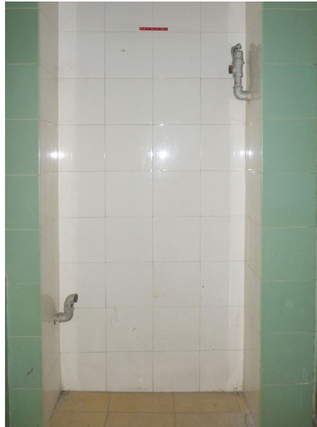
Fig. 124 White and green tiles in the bathroom 02.E, original radiator recess, 2015
