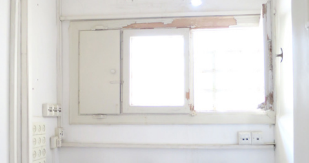
Fig. 128 Hatch in Bathroom 01.P connected with the built-in cupboard on balcony 01.K (type S.1), 2015
