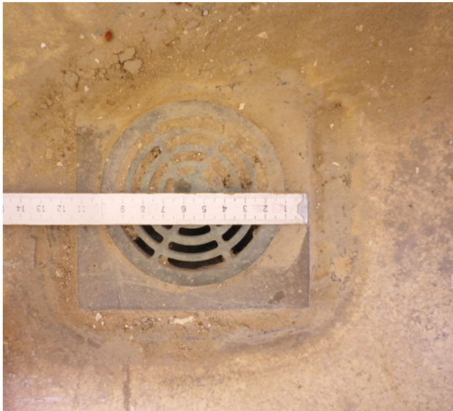
Fig. 143 Grating for a drainage inlet on the balcony 02.J, 2015
