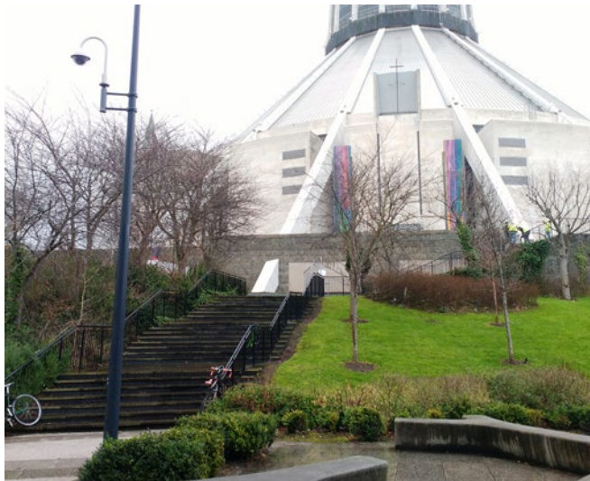
A view of the west stairs showing the variation in the handrails and the relationship of the staircase to the podium.
