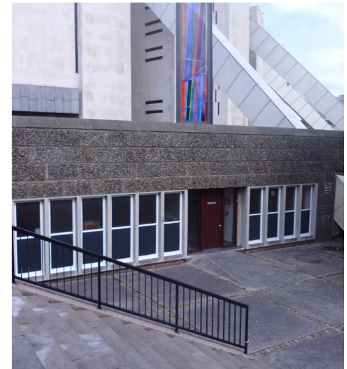
The east stairs shown in the context of the entrance to the administration rooms beneath the podium on the eastern side of the building.
