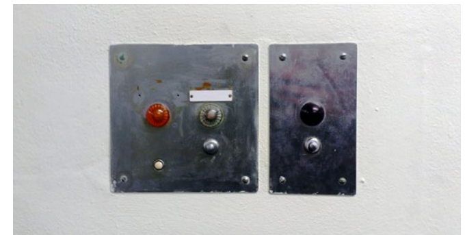
Original (and now defunct) building services chased into the fabric
