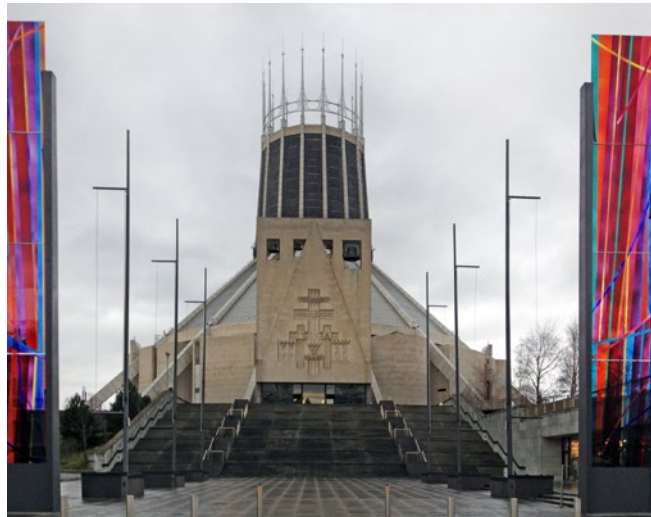
View looking up the steps towards the main entrance to the Cathedral. Approach steps were conceived as part of the original scheme but were only added in 2003
