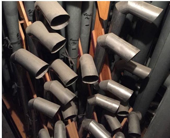
Organ pipes within the organ chamber
