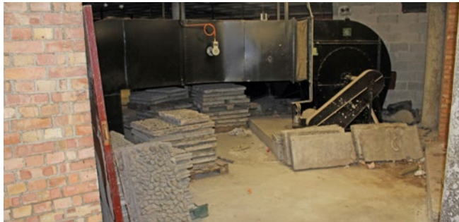
Area of the Gibberd podium used for the storage of the outer facing concrete panels of the building
