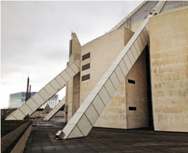
The concrete supports on the west side of the building
