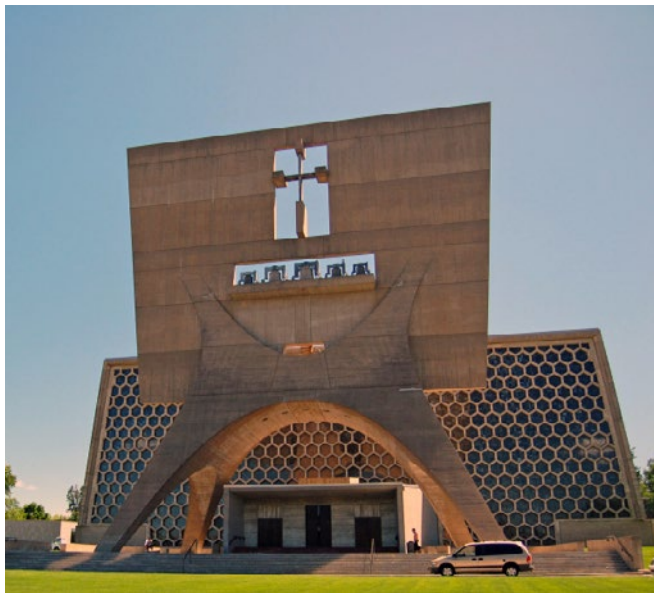
St John's by Marcel Breuer, completed in 1961. The free-standing 'banner' sits in front of the main church building.
