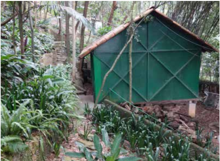
Wood panels external view
