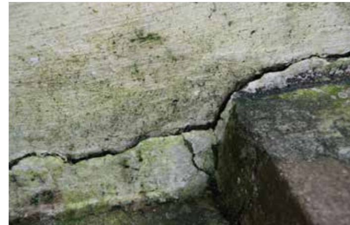
Concrete flooring on the staircases and external walkways
