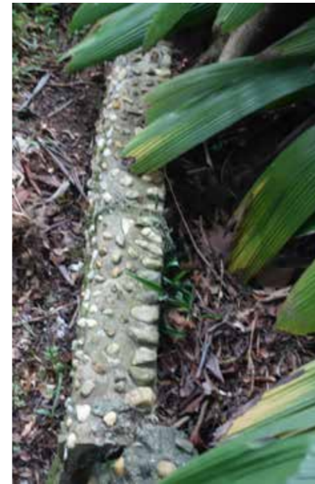
44 Light crack in the low garden wall
