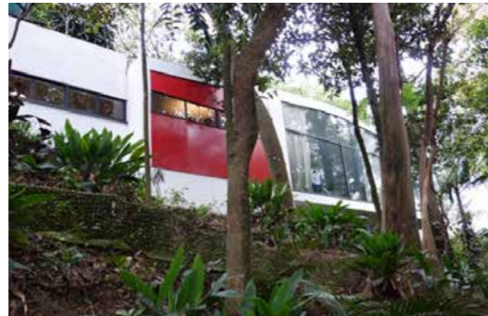
External view of the kitchen and main room windows
