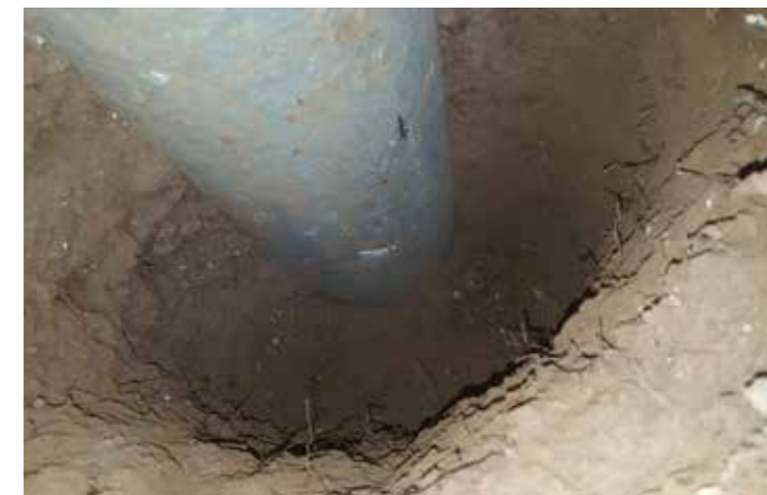
Image 5: Location of the top of the spread footing
