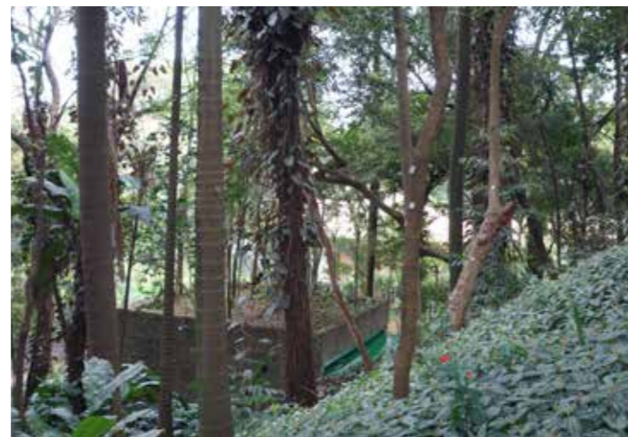
Large quantity of small and medium-sized vegetation on top of the waterproofed slab.
