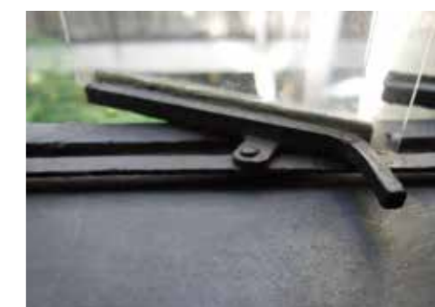
Detail of the opening mechanism and fixation of the glass
