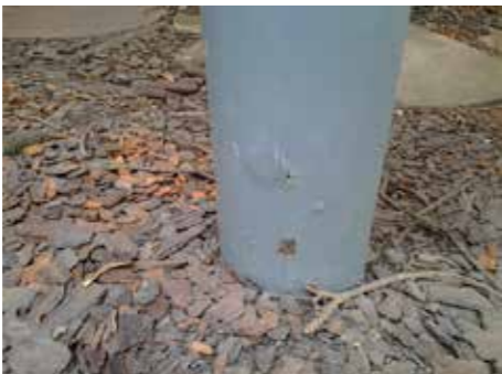
Pillars with oxidation pushing out the layer of paint
