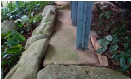
Load-bearing metal posts set into the concrete footing
