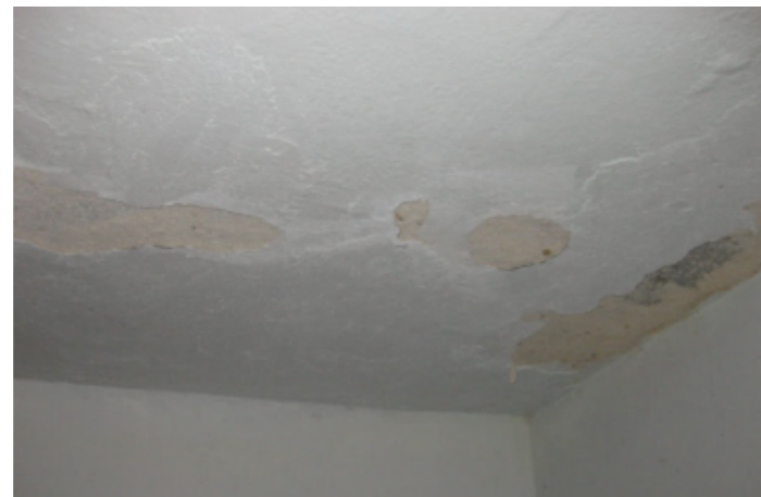
Situation before the renovation: Stains and detachment of the plaster finishing under the slab.
