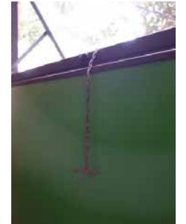
Combined panel casement, kitchen interior Combined panel, kitchen interior. Bascule pull.
