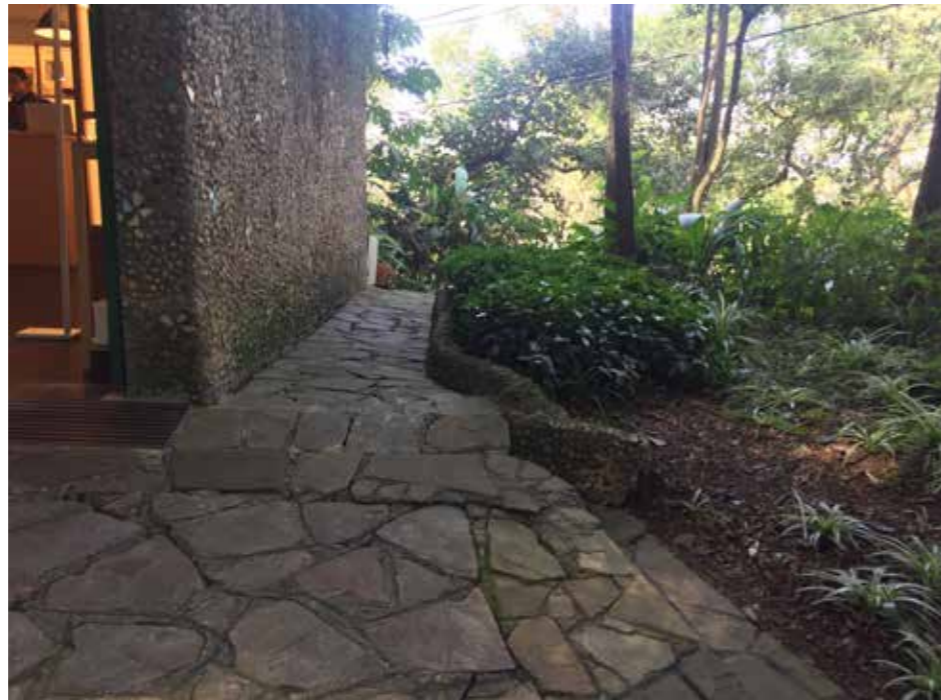
Lateral sidewalk in pink sandstone, with gutter in the foreground.
