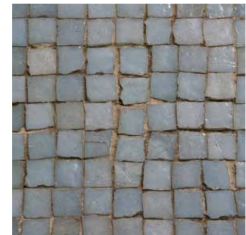
Floor of azure Vidrotil tiles in the living room
