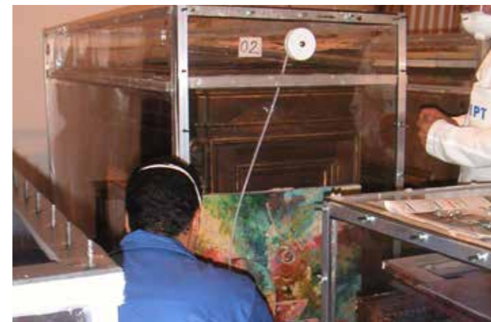
Figure 15. Restoration of the Vidrotile tile floor. 2007. Source: IB. Photography: MCB
