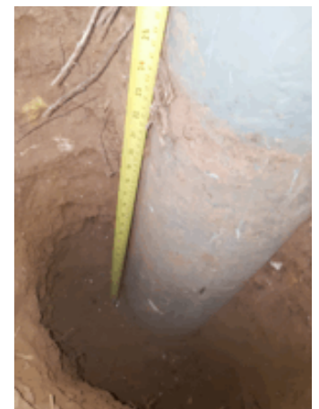
Image 6: Location of the top of the spread footing
