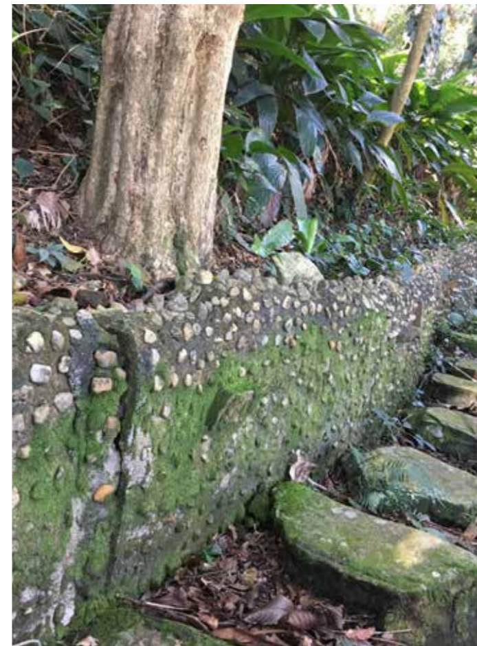
10 Light crack in low retaining wall due to tree growth
