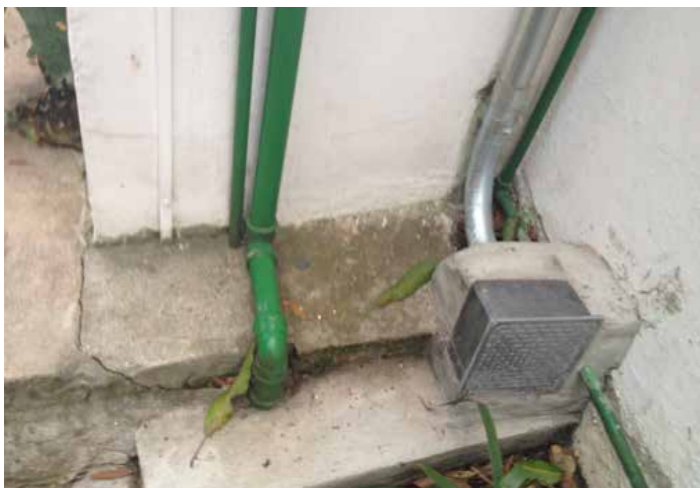
New installations with external tubes for electricity, telephone and data cables
