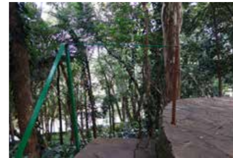
Staircase handrail along with vehicle ramp. Recomposition after damages due to automobile crash.
