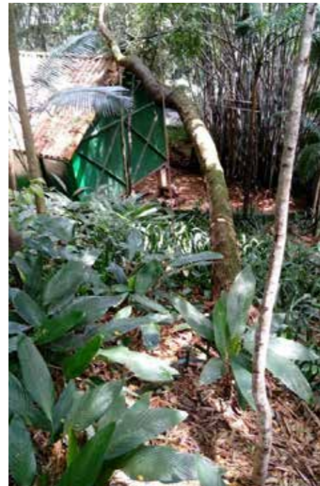
Tree (expected for complete pruning) fall over the studio.
