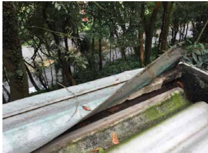
Casings covering the lateral platband beam along the entire perimeter
