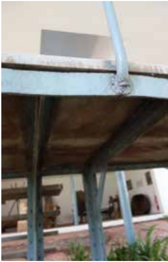
View from below of the landing fitting with the structure
