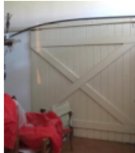
Solid wood doors in the passageways in the service area
