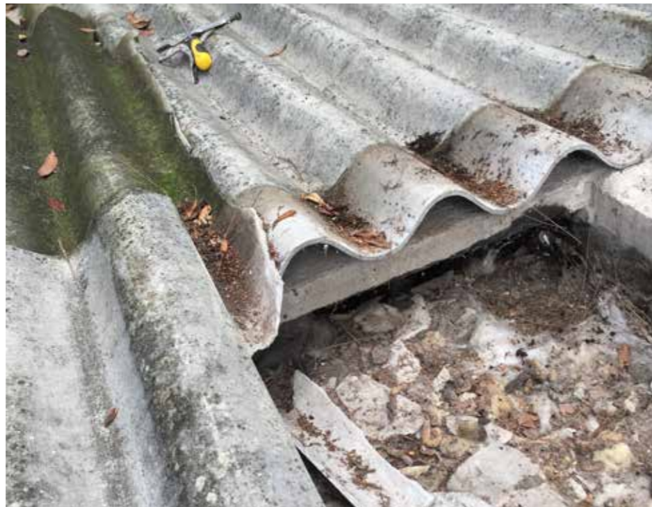
Asbestos cement roofing tile removed for inspection. Notice the load-bearing beams and glass wool for thermal insulation are worn and scattered about the slab, mixing with dried leaves.
