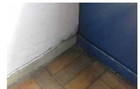
Meeting corner of wood block floor, metal panel and masonry wall. Oxidation onset.
