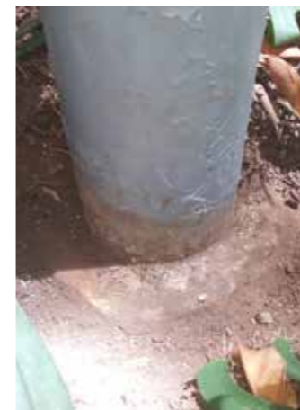
Image 4: Location of the top of the spread footing
