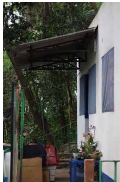
Exterior view of the bascule casements and metal door, mosquito screen and porch
