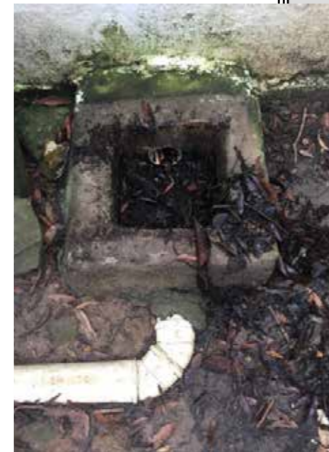
Inspection box of outflowing rainwater on the garden patio. Notice the presence of leaves that have flowed down through the duct.
