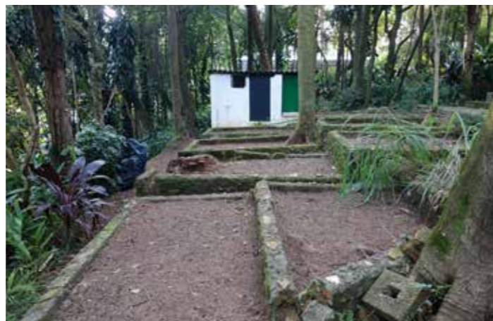
3,4,5 Damages in the vegetable garden walls
