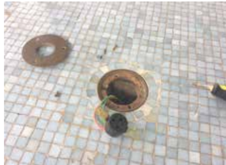
Image 8: Outlet on the floor slab
