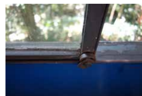
Window track and locking system
