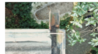
Image 18. Rain gutters and channel flashing on the edges of Casa de Vidro's
