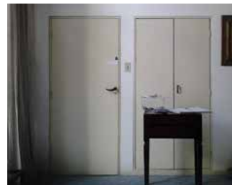
Internal doors of semi-hollow wood
