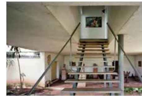
Situation of the piloti lining in 2006, with several spots of bulging and stains. Source: IB. Photo: Nelson Kon
