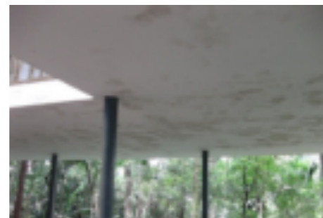
Stains on the slab's underside viewed from the pilotis
