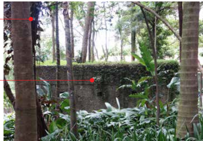
Side view of the garage. Vegetation on the rooftop slab and finishing camouflage the construction of the garden.
