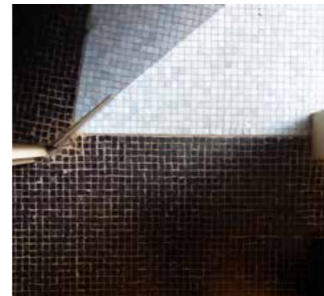
Section of floor where the azure Vidrotil tiles of the living room meet the black tiles of the pantry
