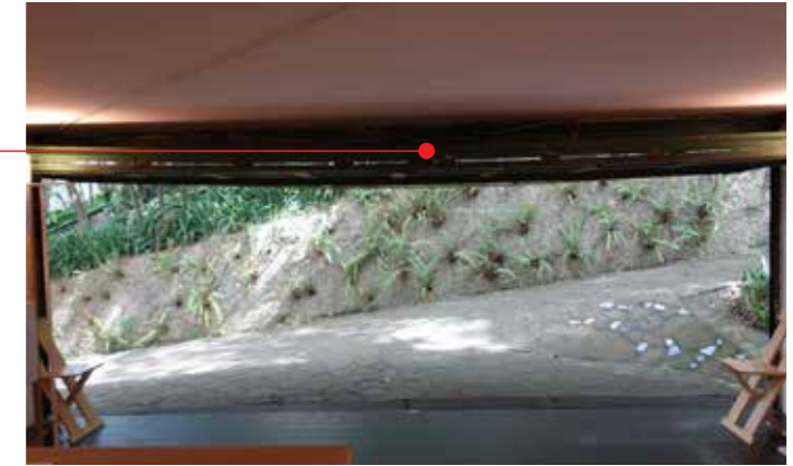
3-cm bend at the center of the gate, when opened, despite the supplementary "wagon"-style support structure.
