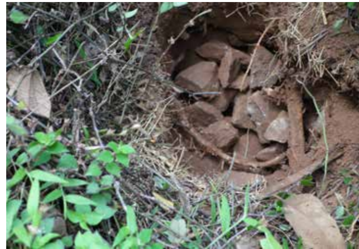
Survey of the layer of soil and gravel that precedes the layer of waterproof protection.
