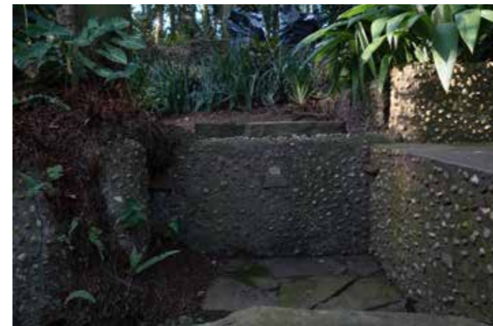
6 Light crack in the low retaining wall
