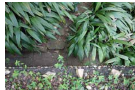
Finishing of external walls. Upper view from the platband.
