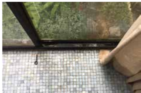
Pin as device serving to block the opening "Truck" for movement in the casements
