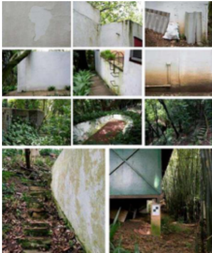
Fig. 15: main pathologies affecting the surfaces of part of the house
