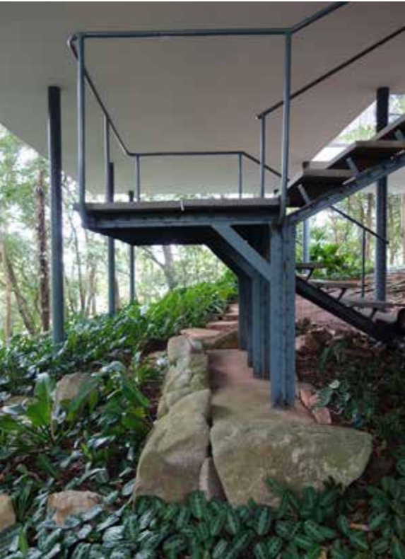
Granite landing supported on the structure by metal bracket
