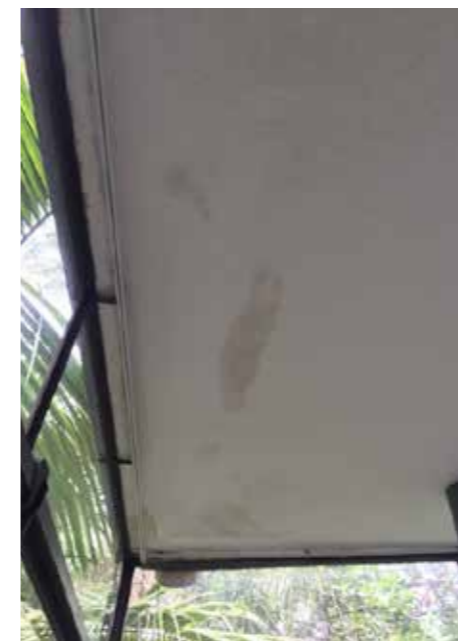
Infiltration in the living room ceiling resulting from the faulty connection between the gargoyles and the concrete gutter beam
