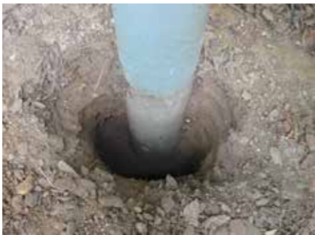
Excavations down to the foundation footing
