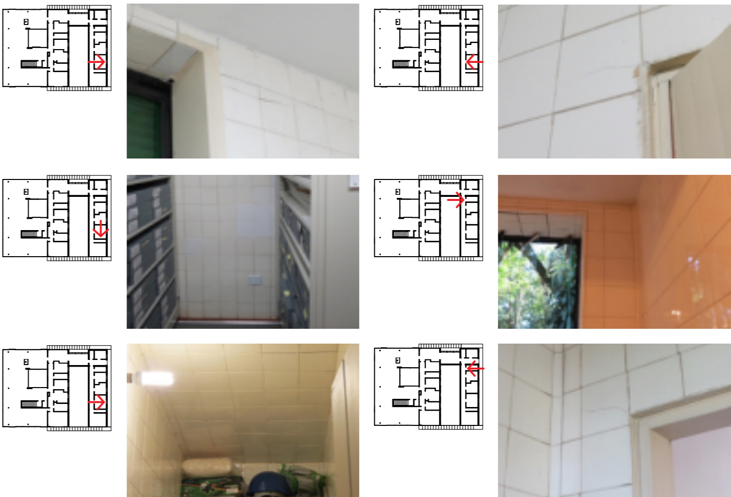
Tile finishing, also including the ceiling
