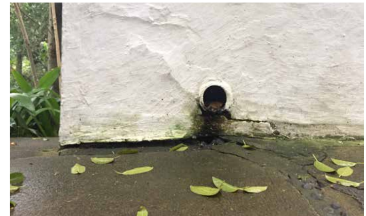
Drainpipe exit that empties directly onto the sidewalk from the vertical rainwater gutter in the laundry/service area
