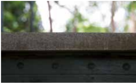
Detail of the rivets and sheet of granite on the landing
