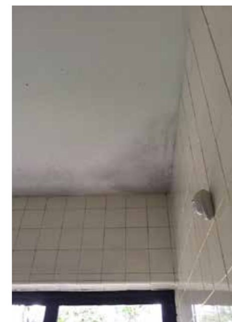
Infiltration in the living room ceiling resulting from the faulty connection between the gargoyles and the concrete gutter beam
