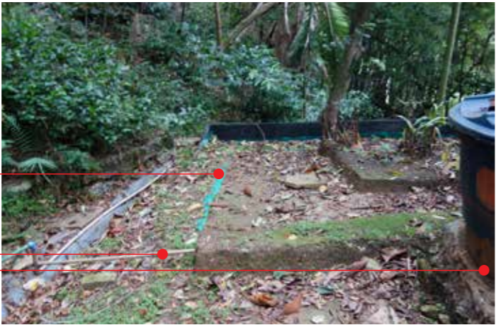
Rooftop garden. View of the slab with the soil cover partially removed to allow maintenance work on the waterproof sealing.
