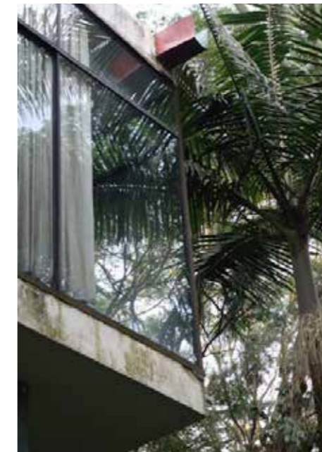
Typical detachment of the mortar layer at the edges of the slab
