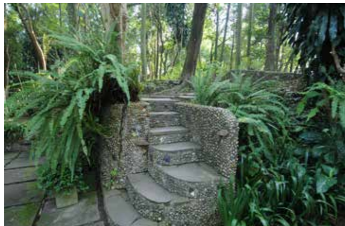
1 Light crack in the stair wall
