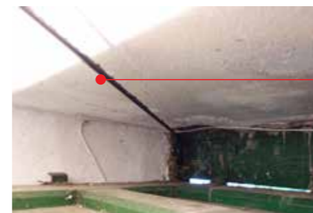
Cable with counterweight mechanism
