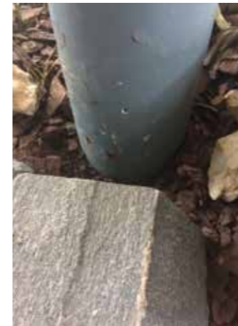
Image 1: Hole in the column
