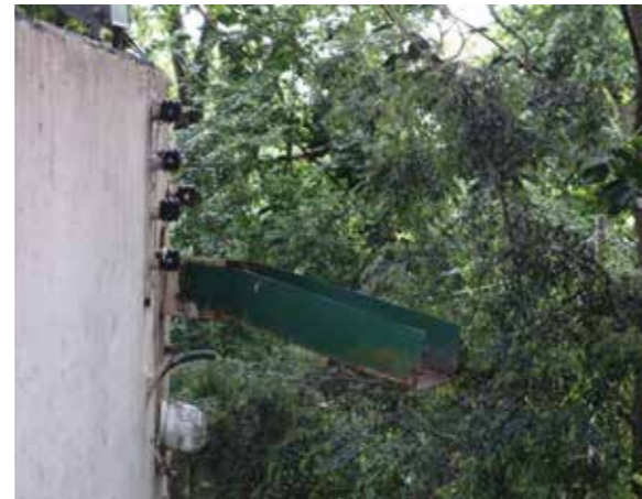
Gargoyle complement in galvanized sheet metal painted green.
