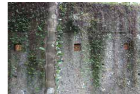
Finishing of external walls. General view of the wall
