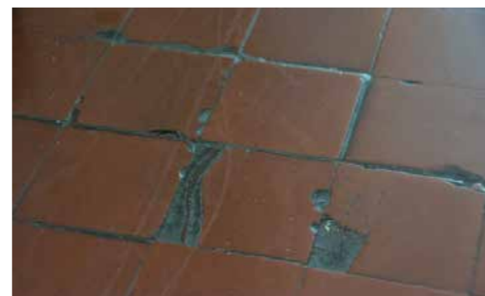
Red ceramic flooring with broken portions in the technical area
