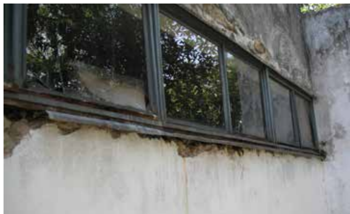
Figure 11. Lina Bo Bardi's room oxidation of the metal sheet casement, 2006. Source: IB. Photography: MCB
