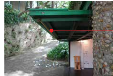
3-cm bend at the center of the gate, when opened, despite the supplementary "wagon"-style support structure.
