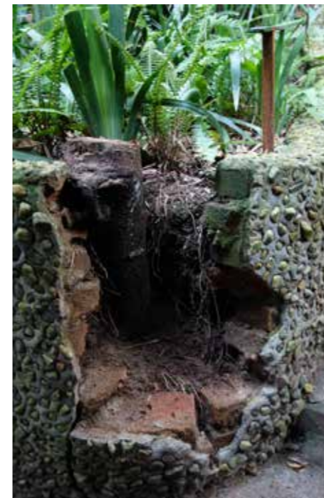
Wall damaged by the fall of tree 827, expected for complete pruning.
