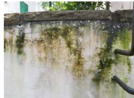
Fungi, stains, cracks and detachment of the finishing and peeling paint on the external walls
