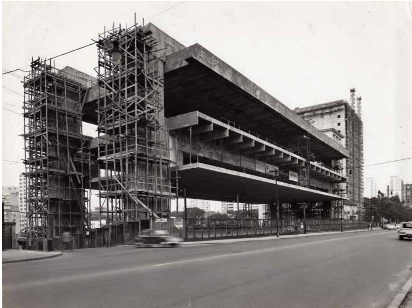
Figure 4 Construction of the São Paulo Art Museum, architect Lina Bo Bardi, 1957 - 1969, São Paulo. Source: IB. Photo: Hans Gunter Flieg, 1968.
