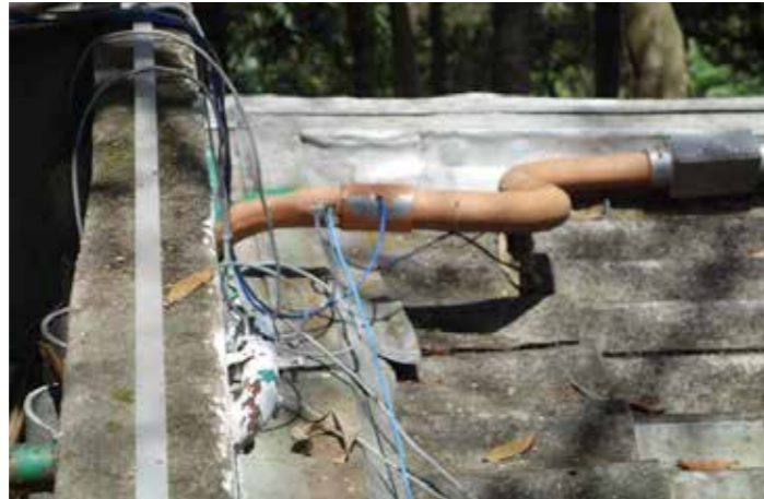
Telephone and logical system wire on the roof
