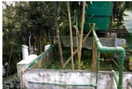
Rooftop garden over the kitchen. PVC water tank, boiler and external piping (CV.04.02) installed in 1989 to replace the original system. Though they function well, the installations had made a strong aesthetic impact on the architecture
