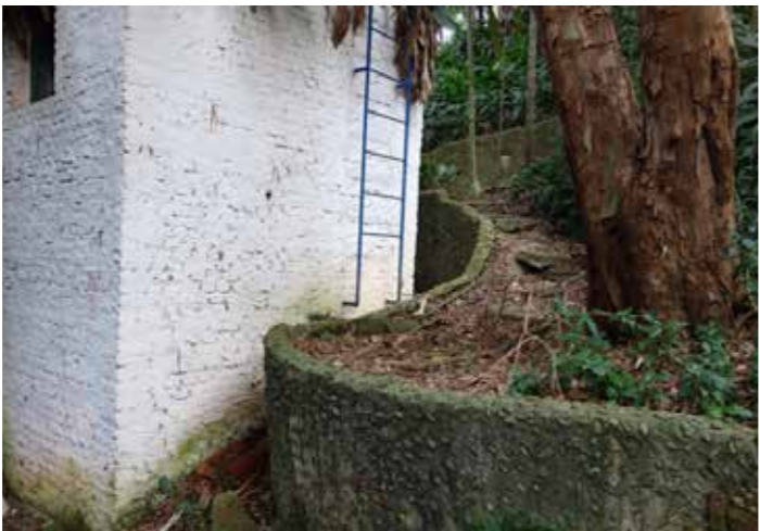
Boat boarding ladder embedded in the stonework
