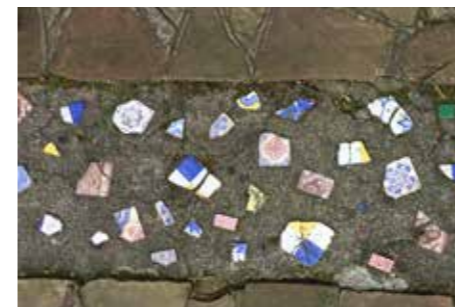
Incrusted ceramic shards in colorful enamel between the two tracks for automobile tires on the ramp's first section.
