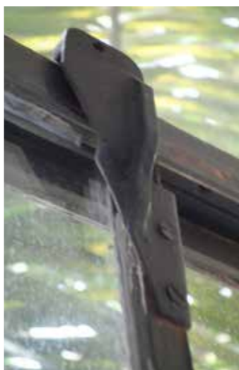
Pin as device serving to block the opening "Truck" for movement in the casements
