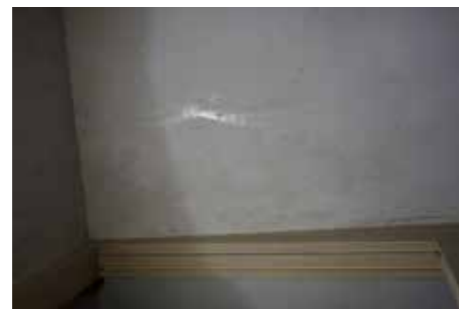
Infiltration in the vestibule ceiling resulting from clogs in the tube for falling rainwater
