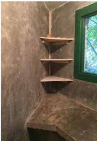
Masonry walls finished in burnt cement on the inside facade and whitewashed on the exterior facade.
