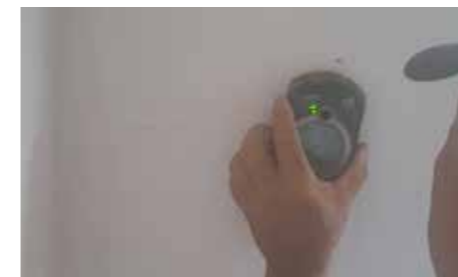
Image 11: Smaller specimens extraction: detection of concrete cover with cover meter
