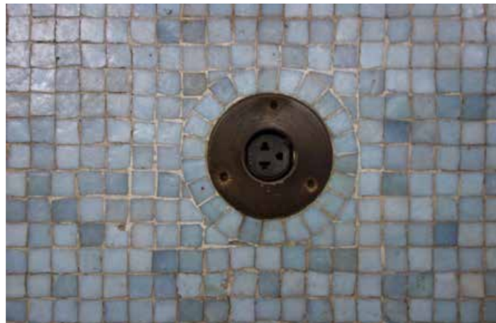
Electrical outlets in the living room floor.
