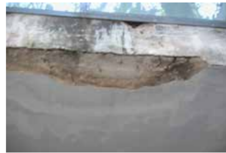
Situation reached in 2006 with displacement of layers of mortar at the slab's edges . Source: IB. Photo: MVB
