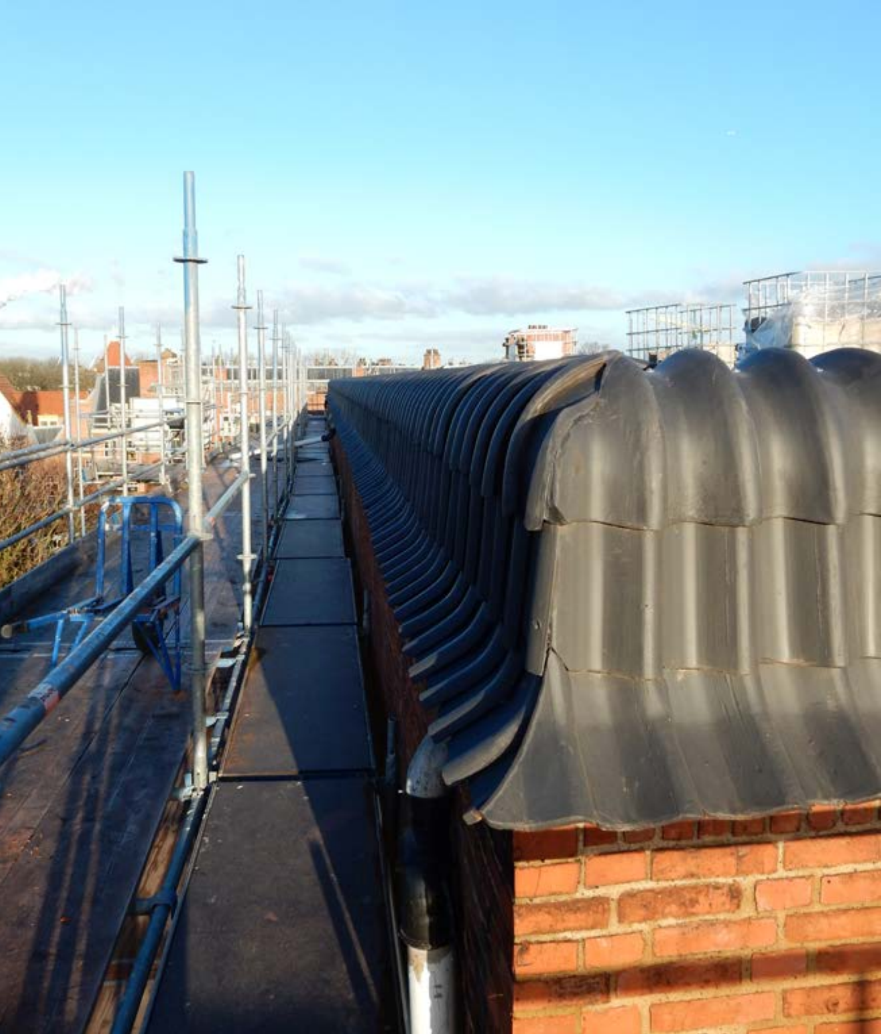
12.09 Corner detail of the roof edge with cut and glued corner tiles.
