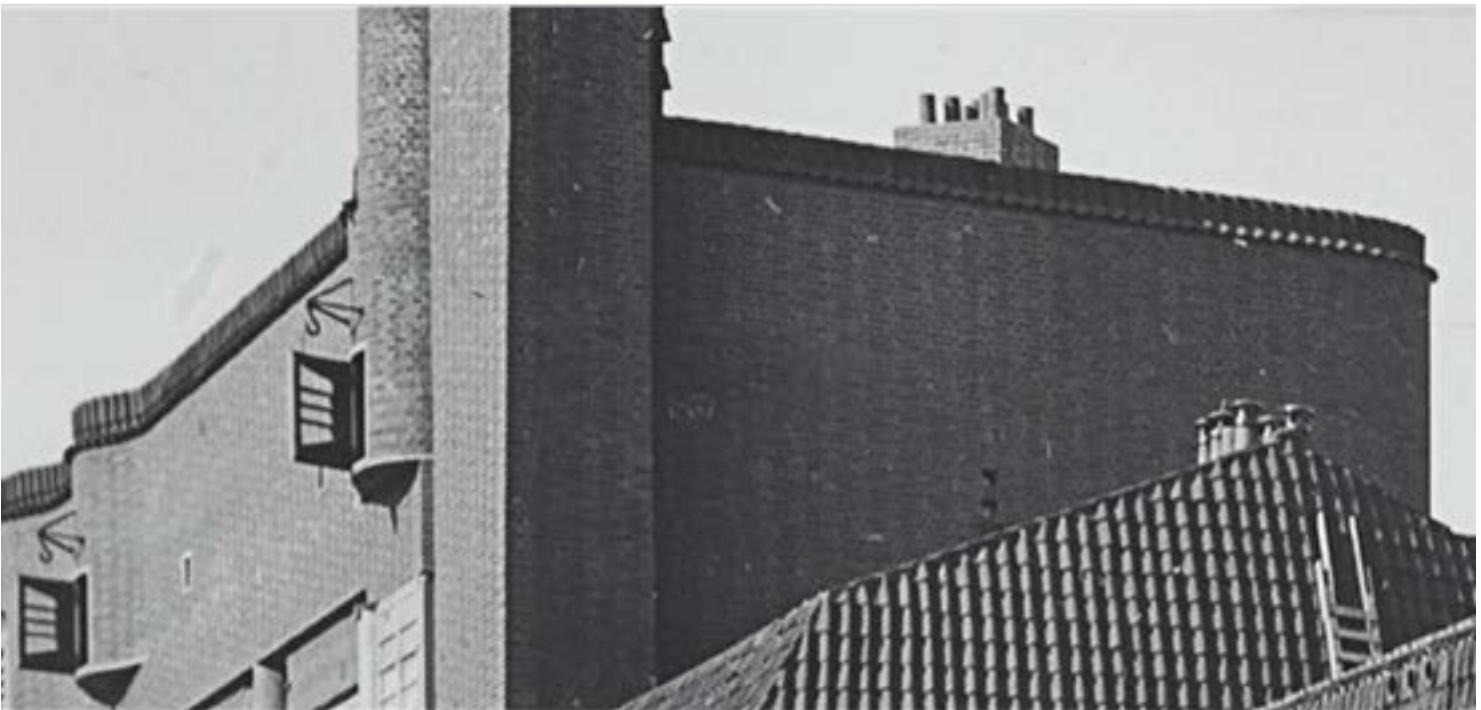
12.16 Rainwater discharge at top of rear façade at the connection of the school building to the apartments, 2015.
