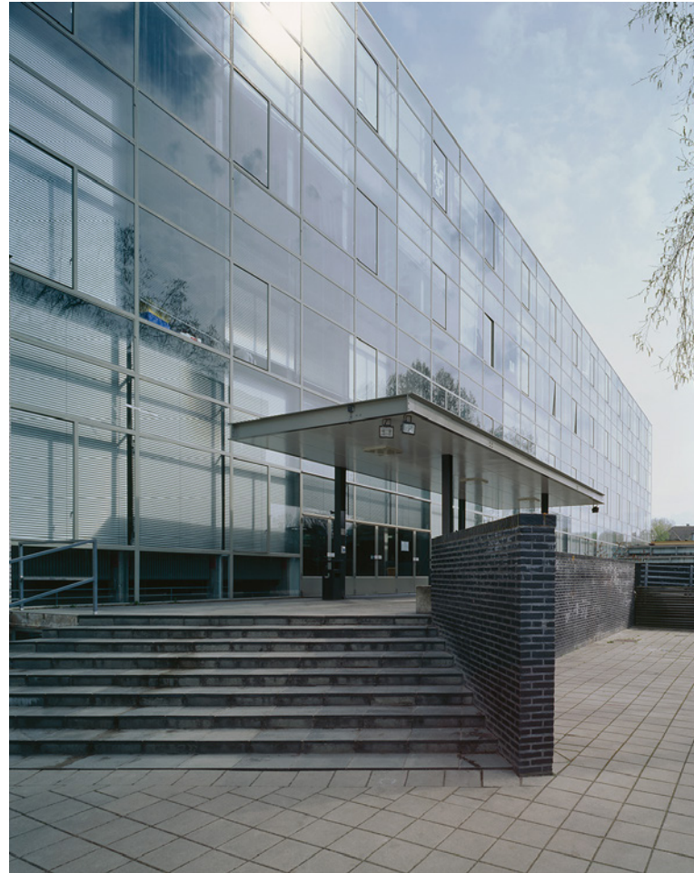
1. Flat full-glazed curtain wall, photo Ton Roelofsma (1967)
