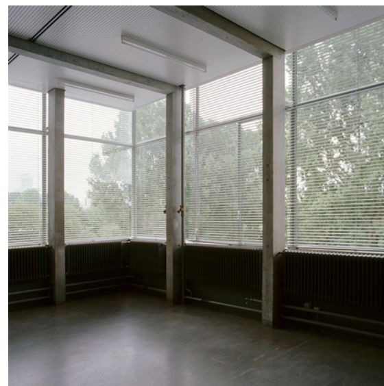
27. Radiators between the columns photo Kim Zwarts (2008)
