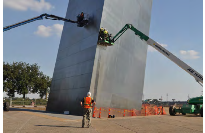
Figure 2-33—Inspection of the lower reaches of the north leg with personnel lifts. Source: S. Kelley
