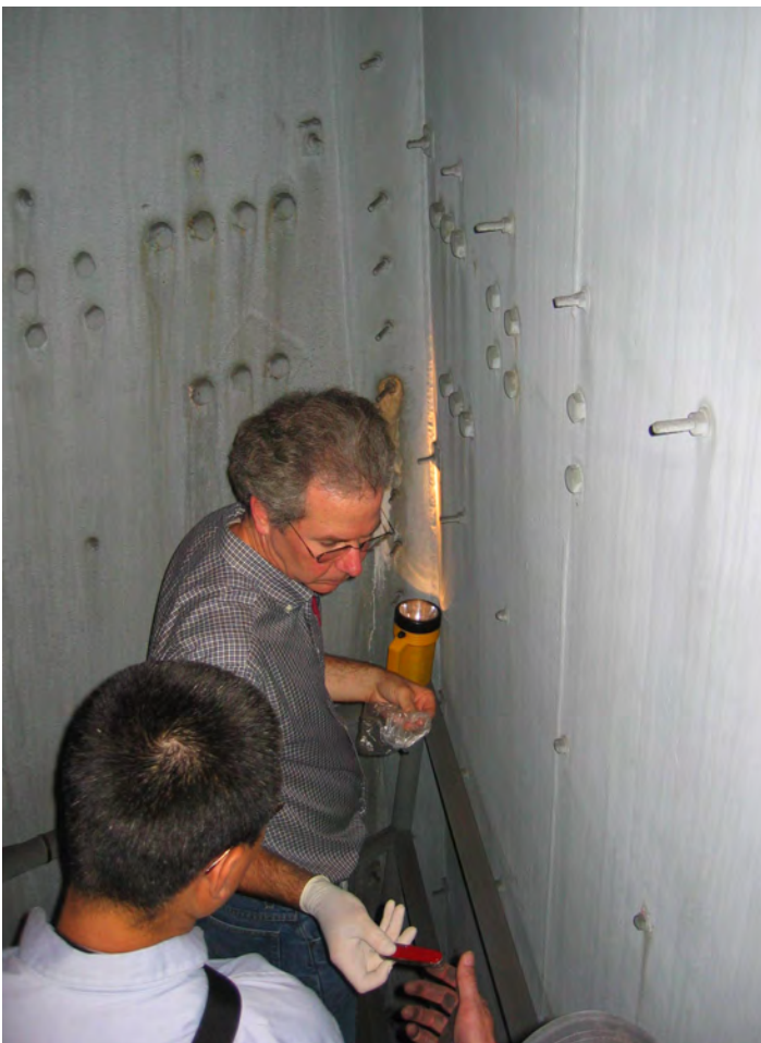
Figure 2-23—Close up inspection of the interior carbon steel skin from the interior stairs. Source: S. Kelley
