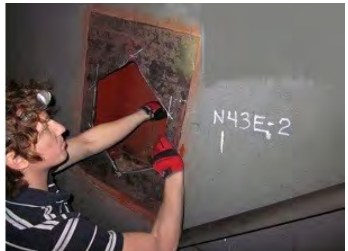
Figure 2-30—Large hexagonal inspection opening at North Station 43 east face. Source: S. Kelley
