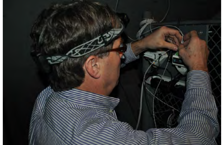
Figure 2-31—Installation of a long-term temperature and relative humidity monitoring system at various heights of both legs of the arch. Source: S. Kelley
