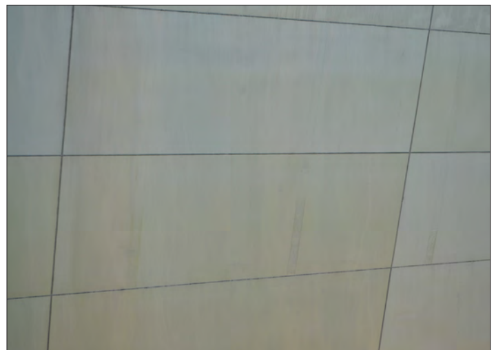
Figure 5-7—Blemishes in the form of darkened vertical lines caused by straps that were used to handle the segment of the monument during shipping. Source: S. Kelley
