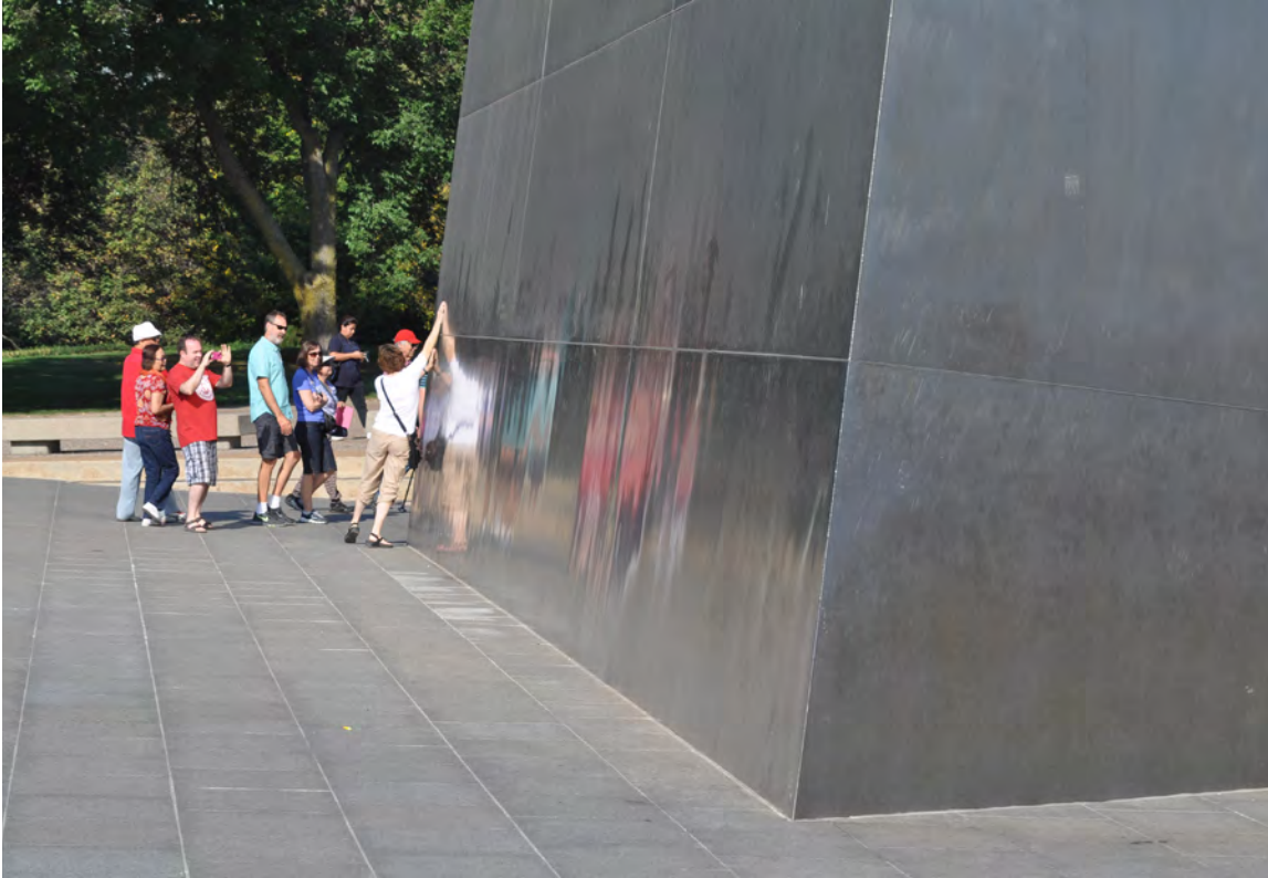
Figure 5-5— Oil deposits at the base of the monument from visitors touching the stainless steel surface.
