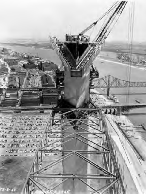
Figure 3-15— View of the trussed strut installed during construction to resist overturning and deflection of the cantilevered Arch legs.
