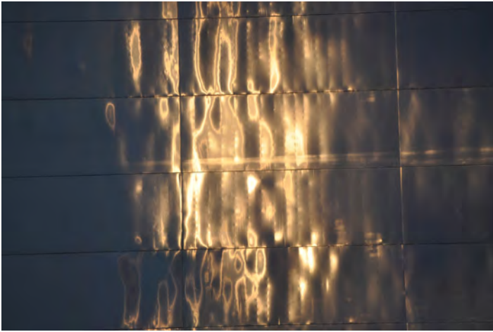
Figure 5-9—Oil canning of the stainless steel surface at the upper reaches of the Monument can easily be seen during some lighting conditions. Source: S. Kelley
