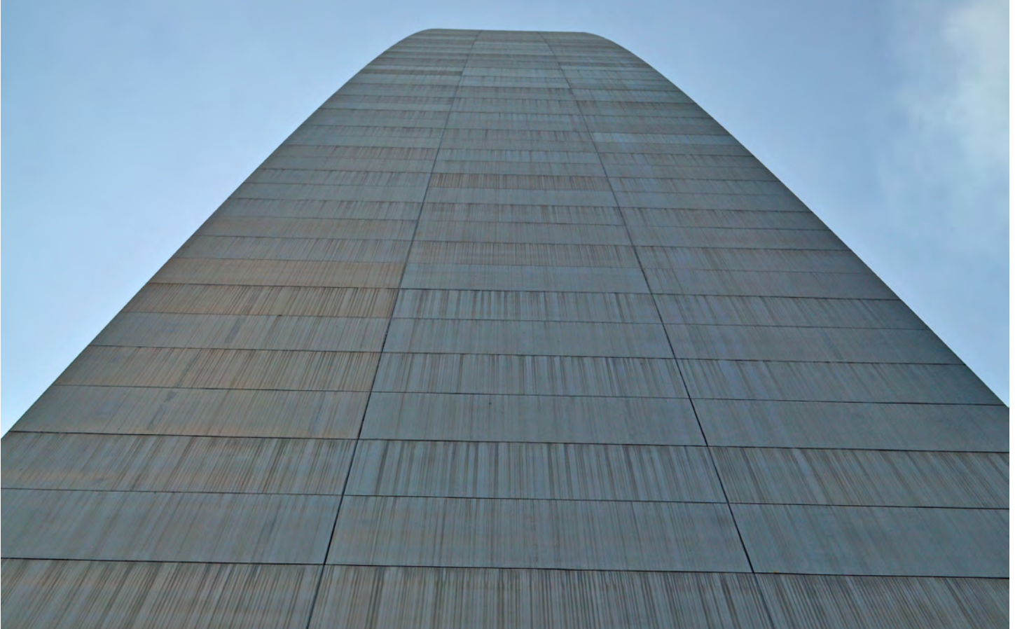
Figure 5-3—Deposits composed of atmospheric pollutants that cause vertical streaking emanating from field welds and shop welds. Source: S. Kelley
