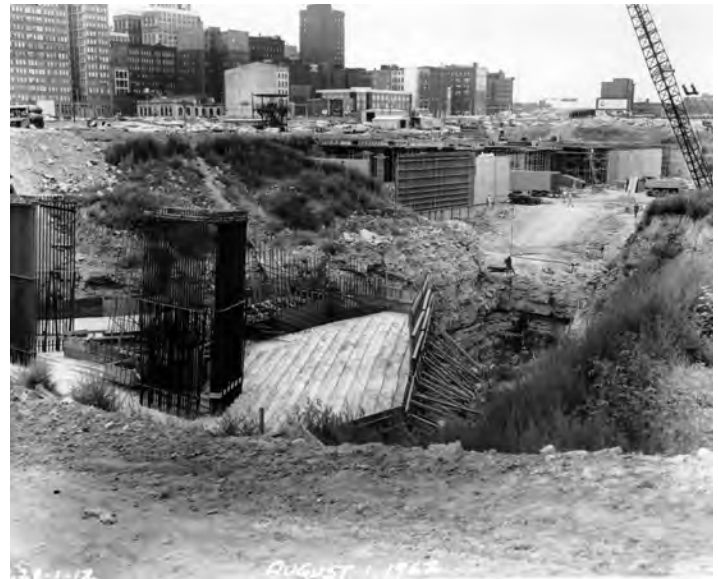
Figure 3-9—Overall view in archival photograph, showing concrete footing and post-tensioning bars in extrados corners. Source: JNEM archive, image V106-3877
