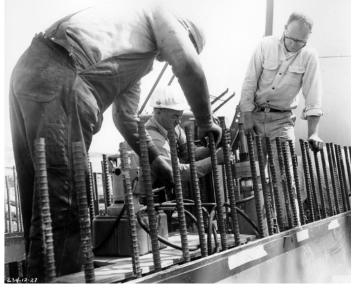
Figure 2-14—Applying tensile stress to the post-tensioning bars, 1963. Source: JNEM archives, image V106-3974
