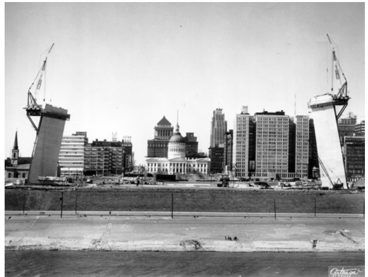
Figure 2-15—The Arch legs under construction with the creeper cranes in place, late summer 1963. Source: JNEM archives, image V106-4034
