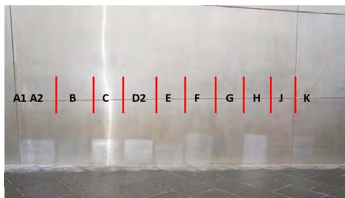
Figure 5-49—The labeled areas of the testing on the east face of the north leg of the monument in 2014. The successful tests were found to be A, C, F and H. Source: 2015 Gateway Arch Corrosion Investigation Part III, WJE
