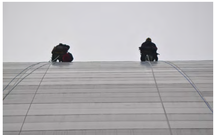
Figure 2-36—Inspection of the welds on the extrados of the north leg using DAT. Source: S. Kelley
