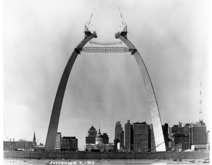
Figure 2-17—The Arch nears completion with the stabilizing strut in place, September 9, 1965. Source: JNEM archives, image V106-4124
