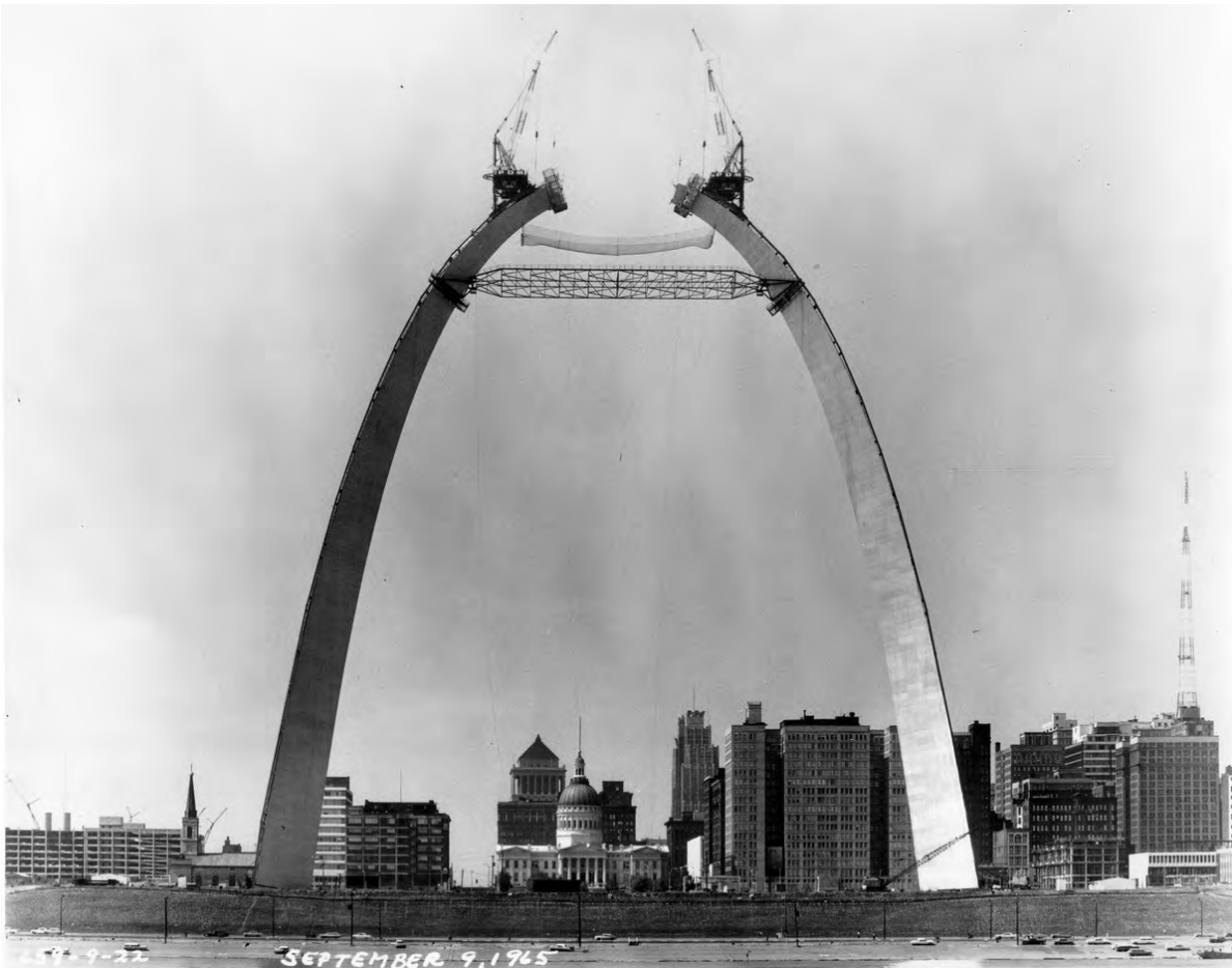
Figure 3-16— Overall view of the strut installed during construction.
