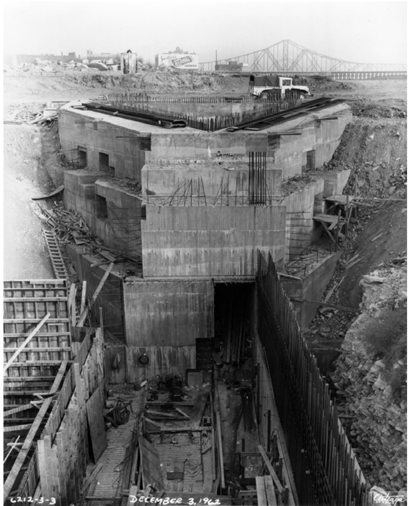
Figure 2-11—Construction of the Arch foundation, December 3, 1962. Source: JNEM archives, image V106-3938
