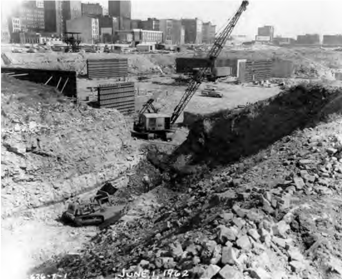
Figure 3-5—View showing excavation for concrete footings of Arch. Source: JNEM archive, image V106-3865
