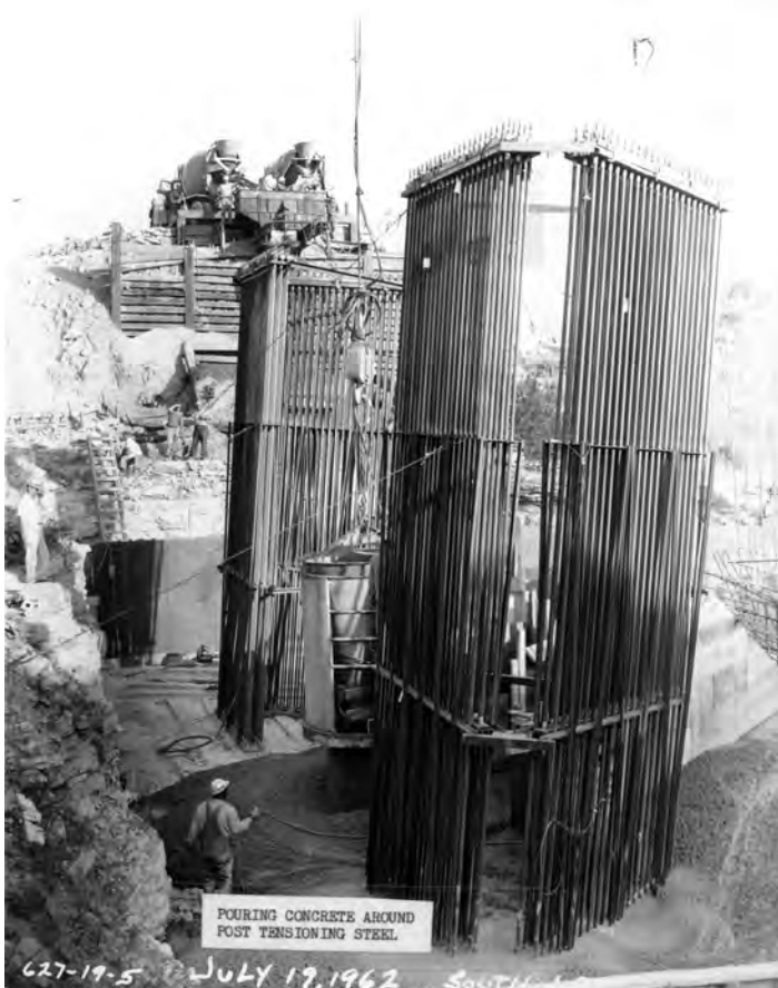
Figure 3-9—Overall view in archival photograph, showing concrete footing and post-tensioning bars in extrados corners. Source: JNEM archive, image V106-3877
