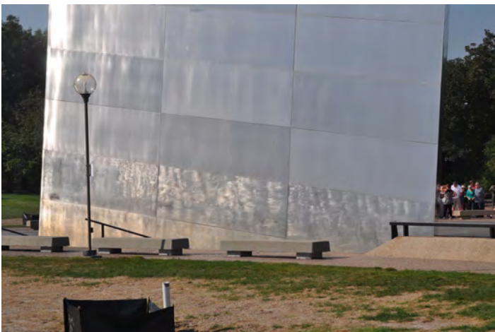
Figure 5-13—Unsuccessful refinishing of the east face of the south leg, date of refinishing unknown.
