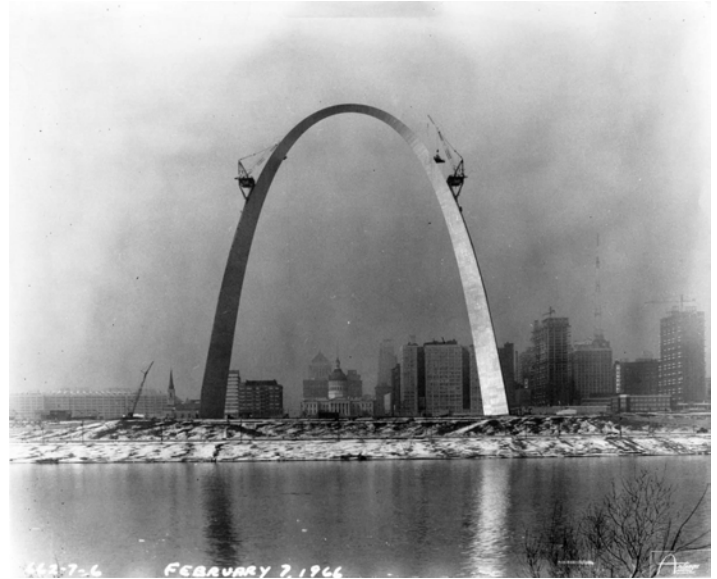
Figure 2-19—Cleaning the Arch and removing the creeper cranes, February 7, 1966. Source: JNEM archives, image V106-4147
