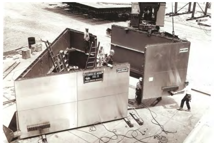
Figure 3-4—Typical segment above concrete fill (Station 0 to Station 44) constructed as three L-sections. Source: Arteaga Photos, Ltd. (from Gateway Arch: An Architectural Dream, pg. 104)
