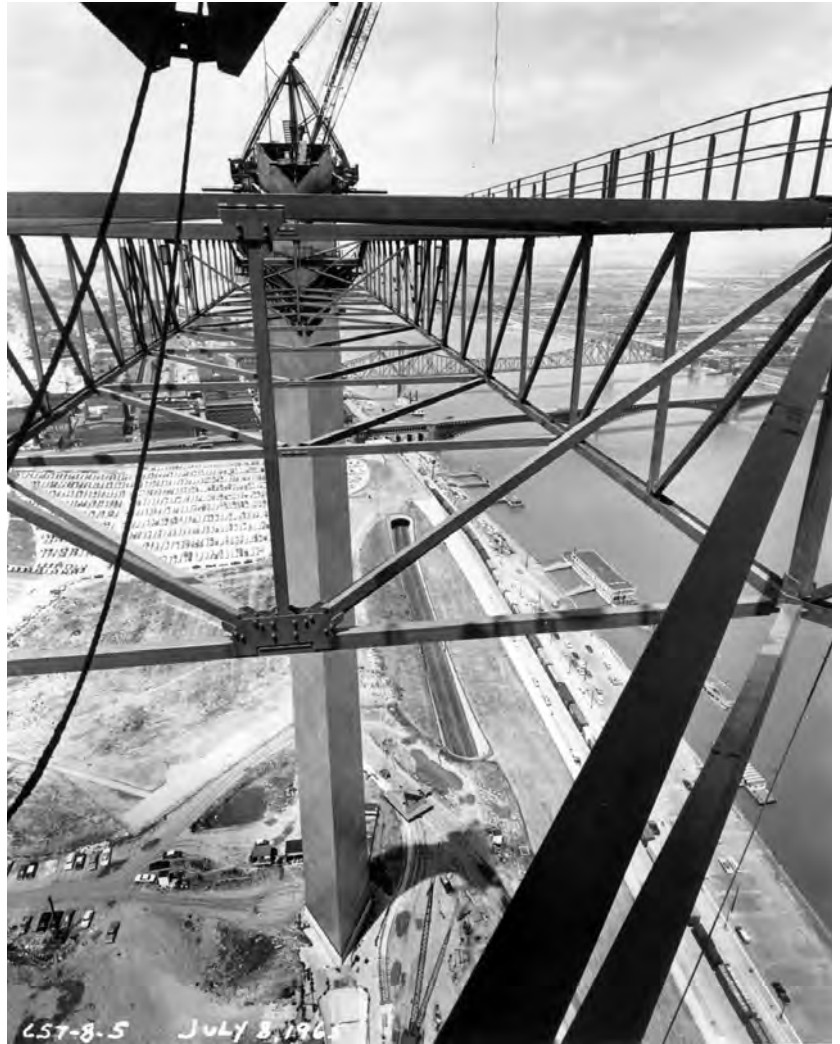
Figure 3-14—Close up view of the trussed strut installed during construction to resist overturning and deflection of the cantilevered Arch legs. Source: JNEM archive, image V106-4111
