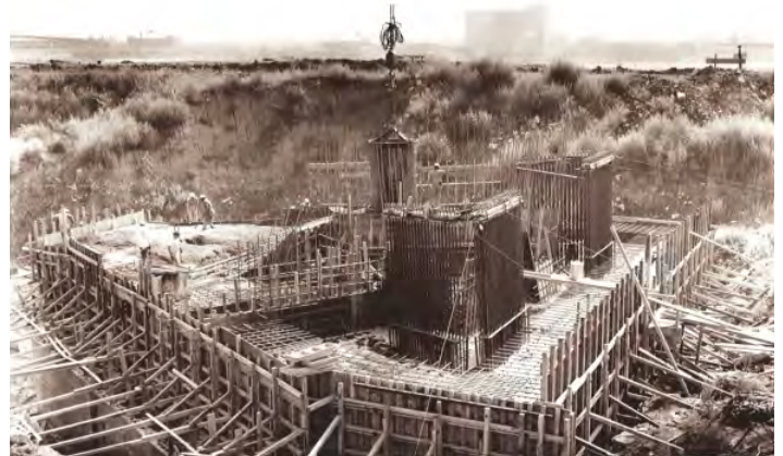
Figure 3-6—View showing completed reinforced concrete footing, including reinforcing and post-tensioning bars. Source: Arteaga Photos, Ltd. (from Gateway Arch: An Architectural Dream, pg. 59)
