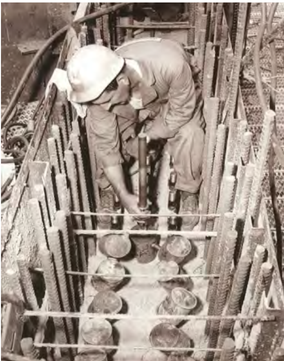
Figure 3-13—View of tensioning the reinforcing bars below the 300 foot level. Source: Arteaga Photos, Ltd. (Gateway Arch: An Architectural Dream, pg. 60)
