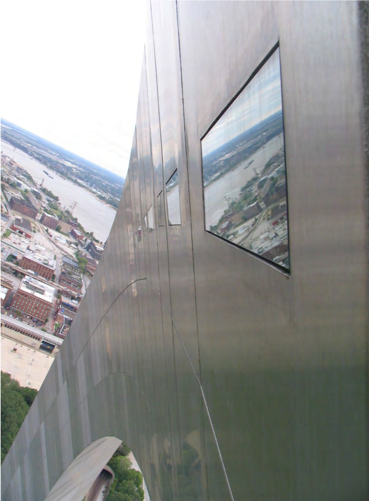
Figure 2-25— Inspection of the skin from a window of the visitors' viewing area.
