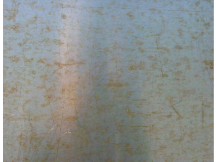
Figure 5-1—Discoloration in the form of superficial corrosion staining to the stainless steel surface. This is a typical condition at the base and lower reaches of the monument. Source: S. Kelley
