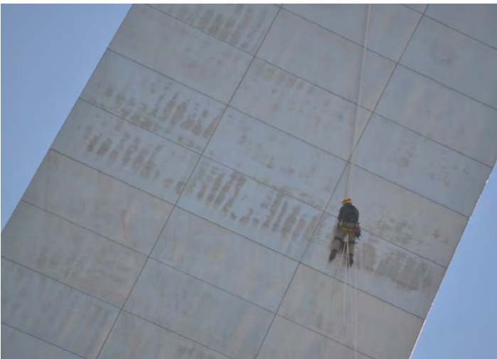
Figure 5-4—Deposits on the upper reaches of the monument that collect on the indented “oil canning” of the panels that occurs between interior stiffeners.
