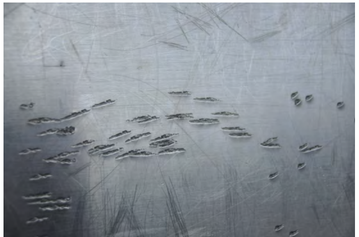
Figure 5-12—Damage to the surface of the Monument caused by striking with the claw of a hammer. Source: S. Kelley
