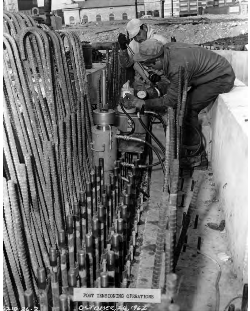
Figure 3-12—View of tensioning the reinforcing bars below the 300-foot level. Source: JNEM archive, image V106-3933
