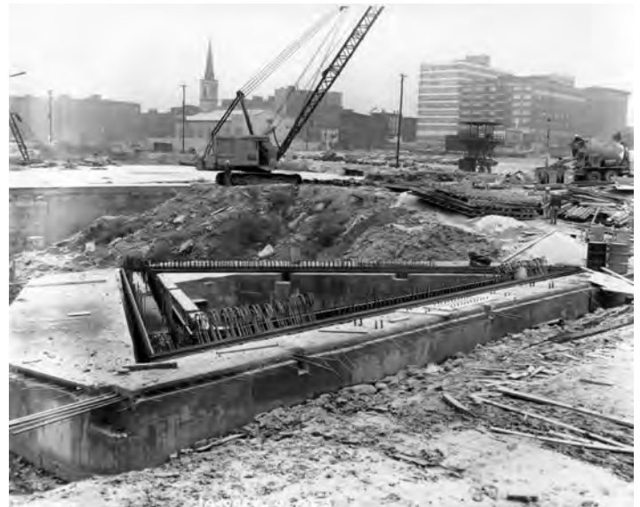
Figure 3-11—Overall view showing integration of the reinforcing bars at the concrete footing and concrete filled portion of the steel skins. Source: JNEM archive, image V106-3940
