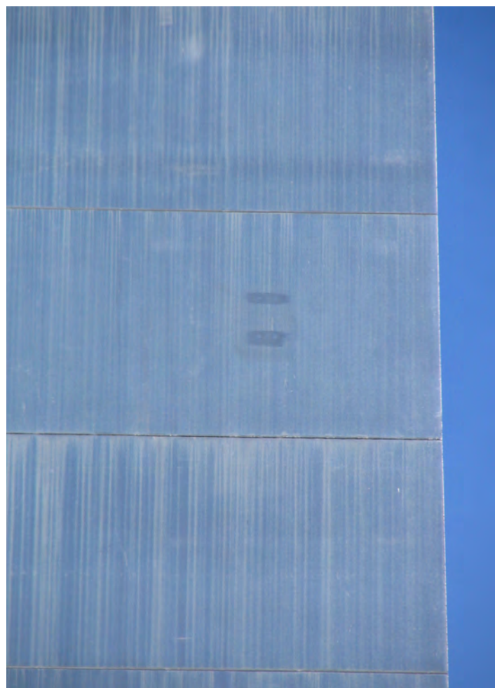
Figure 5-8—Blemishes on the extrados where the creeper crane was attached to the leg during erection. Source: S. Kelley
