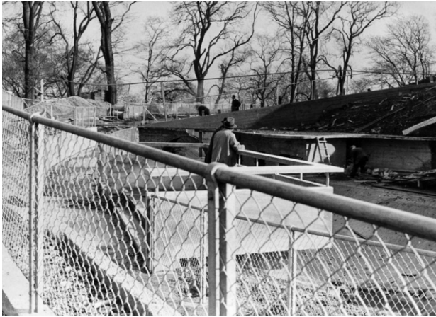
Fig 101. Sea Lion Pool under construction with Lubetkin overlooking from the terrace, 1937
