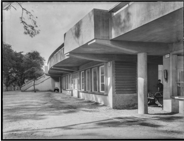
Fig 72. Image of the former Elephant House, Exterior view of the Elephant House showing cantilevered terrace with corrugated finish on facing concrete and saddles for elephant rides, 1937
