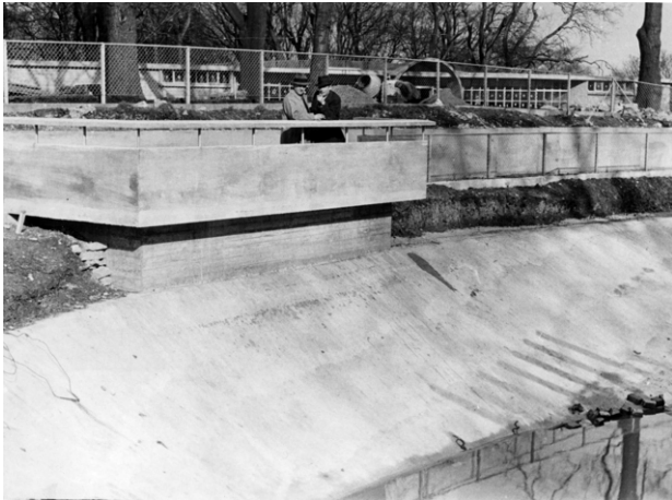
Fig 103. Sea Lion Pool under construction with Lubetkin overlooking from the terrace, 1937
