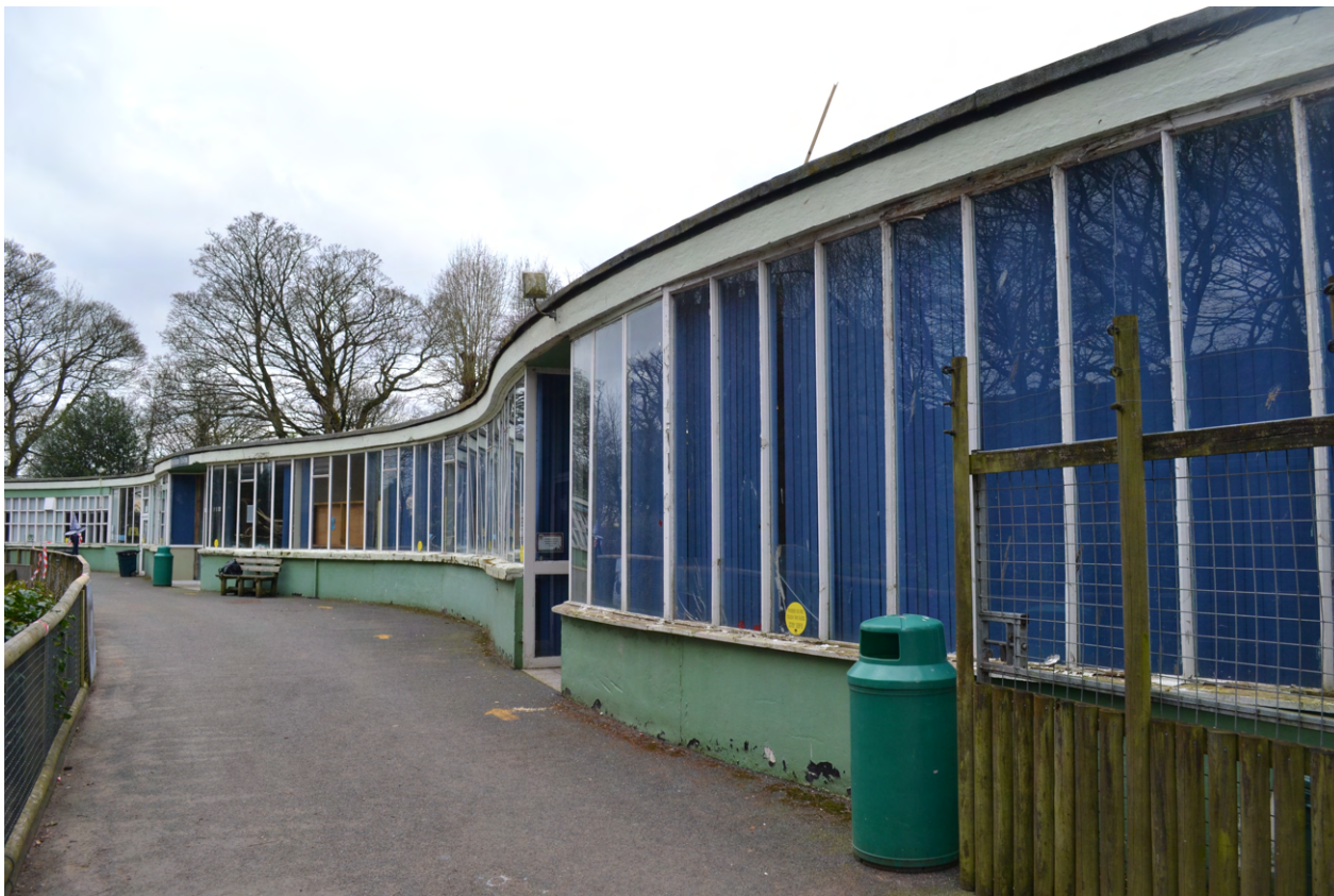
Fig 28. Image of the Discovery Centre, former Moat Cafe
