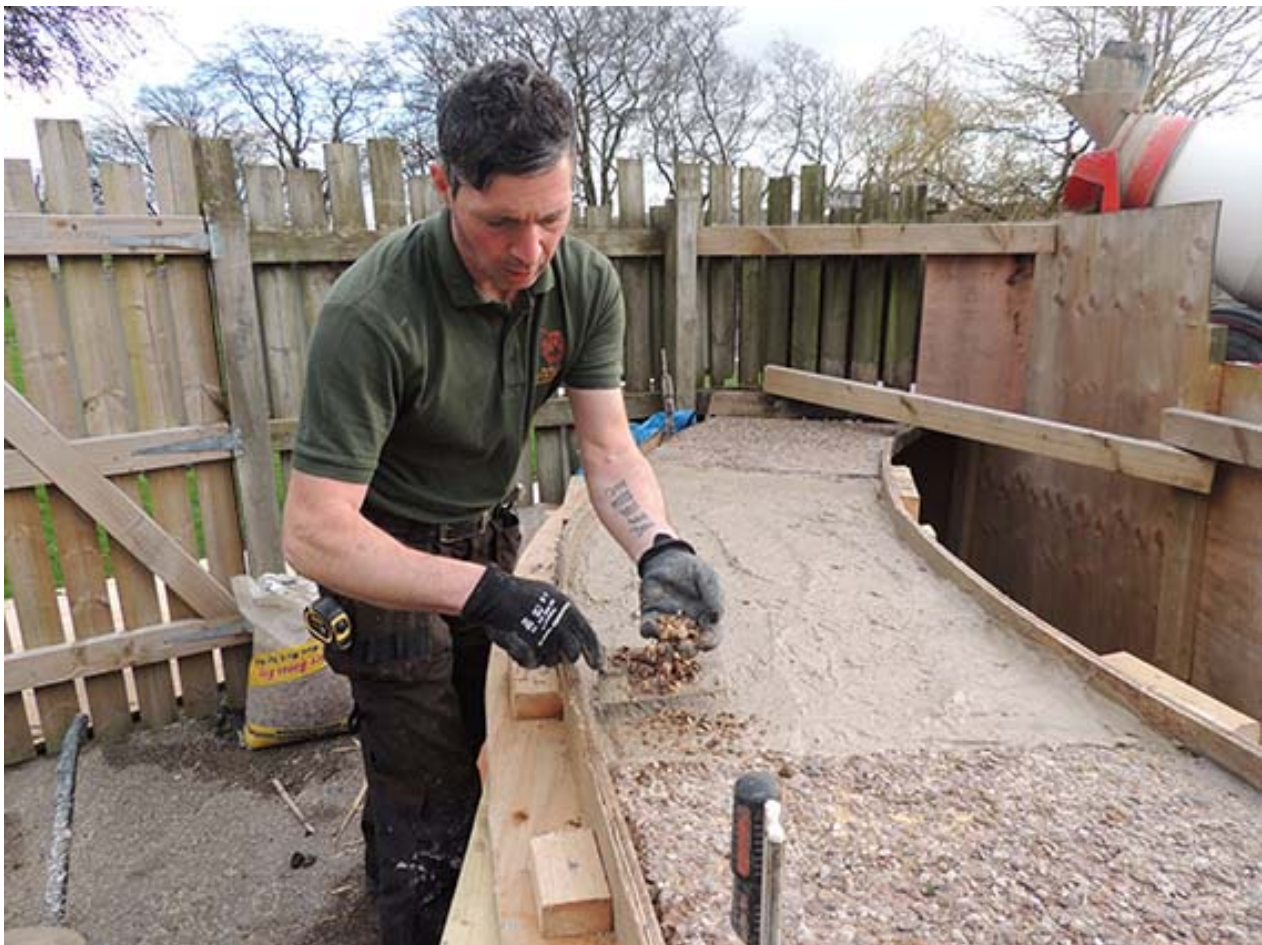
Fig 41. Image of the repair works to the Meerkat Enclosure.
