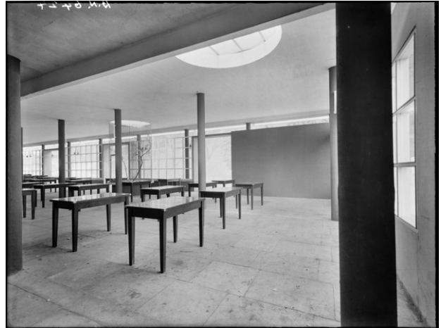
Fig 85. Image of the former Station Café, Interior view of the station café showing pilotis, cylindrical birdcage and circular skylights, 1937
