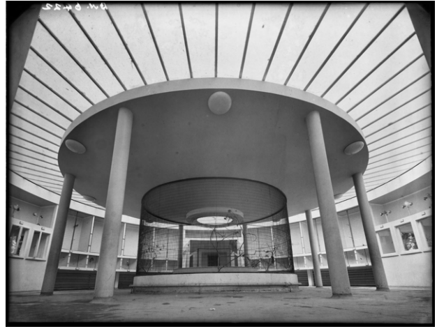
Fig 50. Image of the former Bird House, Interior view of the Bird House showing circular plan form, arrangement of the cages and inverted roof light, 1937
