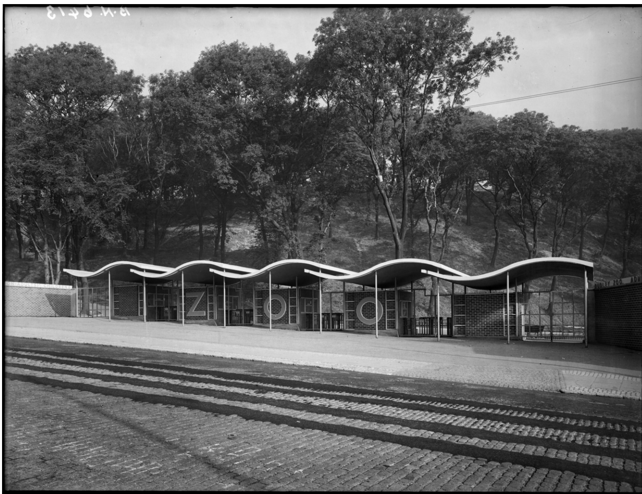
Fig 75. Image of the former Entrance Gateway, View of the canopied entrance kiosks and wooded hill behind, 1937
