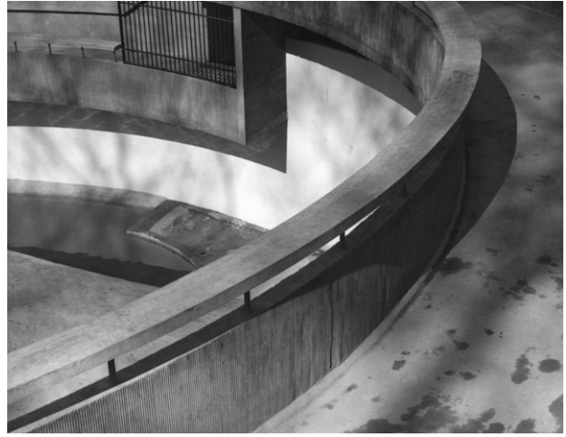
Fig 110. Image of the former Polar Bear Pit and Lion and Tiger Ravines, Detail view of upper spectator terrace looking into the central arena, showing corrugated finish on facing concrete, the tip of the concrete iceberg and water in the pool below, 1937
