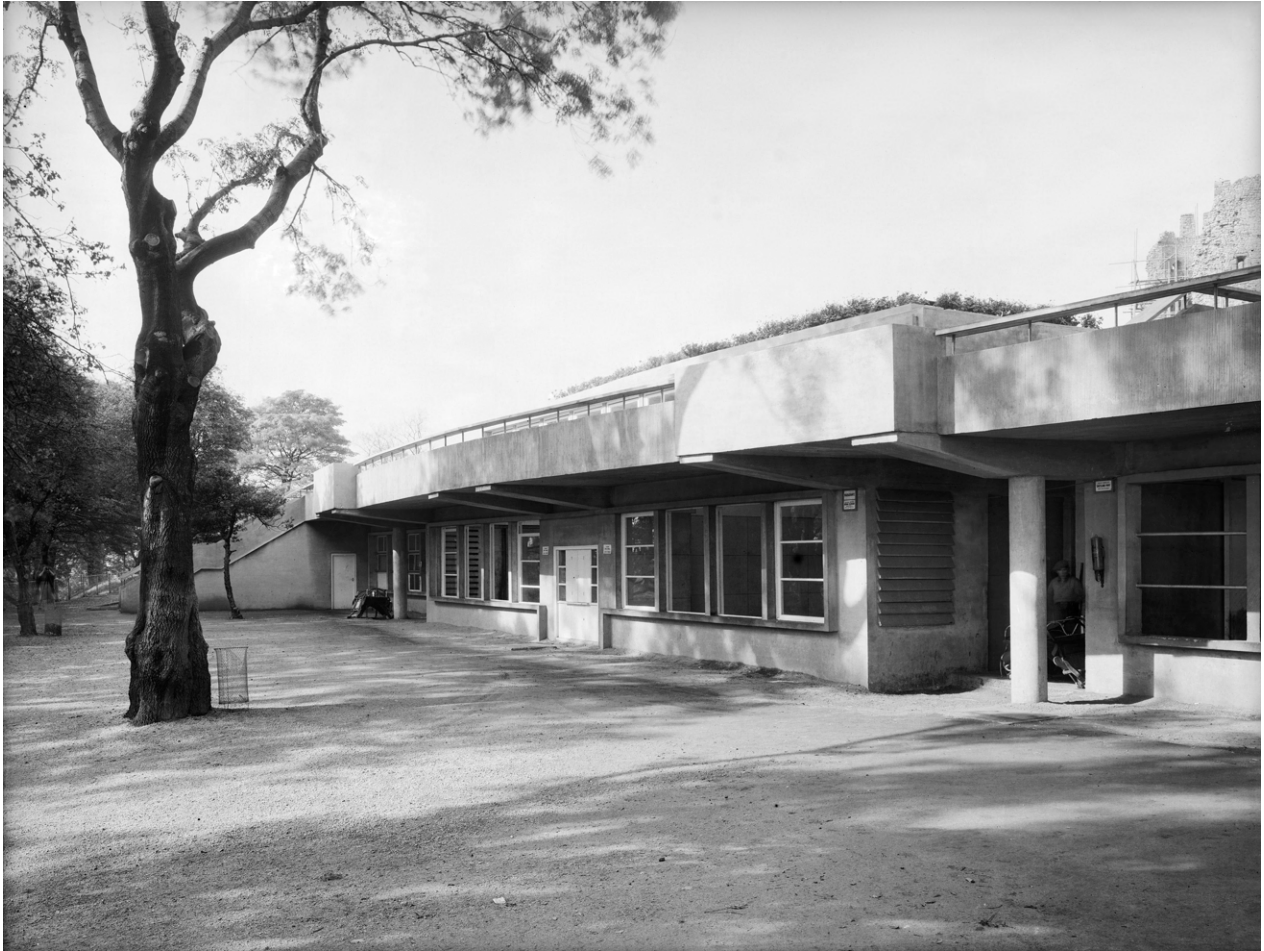
Fig 70. Image of the former Elephant House, Exterior view of the Elephant House showing cantilevered terrace and saddles for rides, 1937
