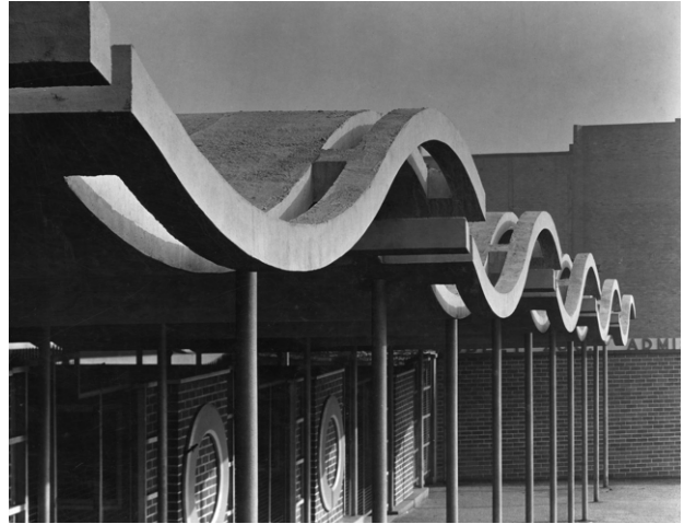
Fig 78. Image of the Entrance Gateway, Detail view of the roofline showing the overlapping concrete canopies, 1937
