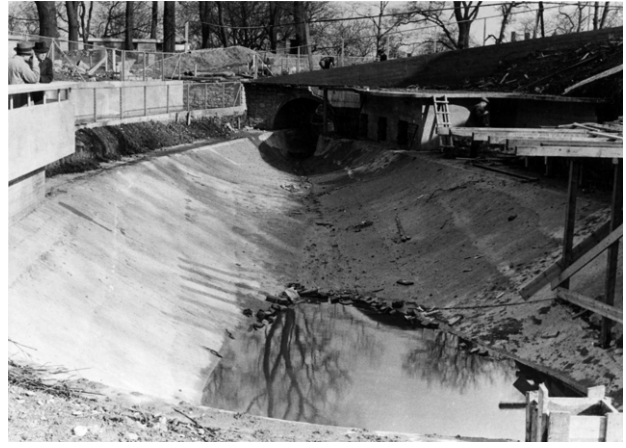
Fig 102. Sea Lion Pool under construction with Lubetkin overlooking from the terrace, 1937
