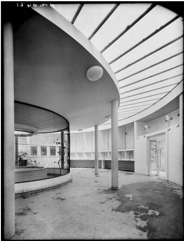
Fig 51. Image of the former Bird House, Interior view of the Bird House showing the arrangement of cages and inverted roof light, 1937
