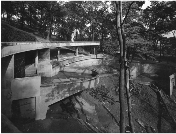
Fig 93. Image of the former Bear Ravine, View of the Bear Ravine showing cantilevered balcony and upper terrace supported by mushroom-headed colonnade, 1937
