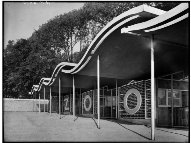
Fig 80. Image of the Entrance Gateway, View of the entrance kiosks shielded by overlapping concrete canopies, 1937
