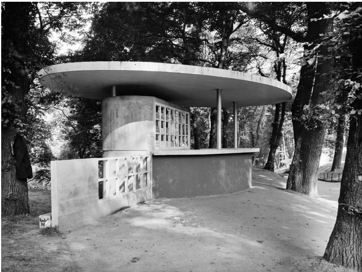
Fig 43. Image of the Kiosk, View of the kiosk looking in the direction of the Polar Bear Pit and Lion and Tiger Ravine, 1937
