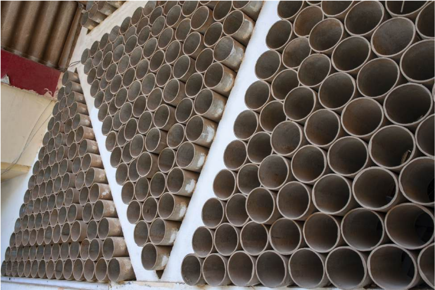
Fig.127: close-up of ventilated PVC pipe facade (photo: Elyse Fitte-Duval, 2021).
