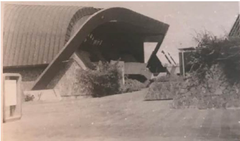
Fig.18: (A-C) (above): photographs of the CICES auditorium under construction c. 1972-3 (personal archives of Marin).
