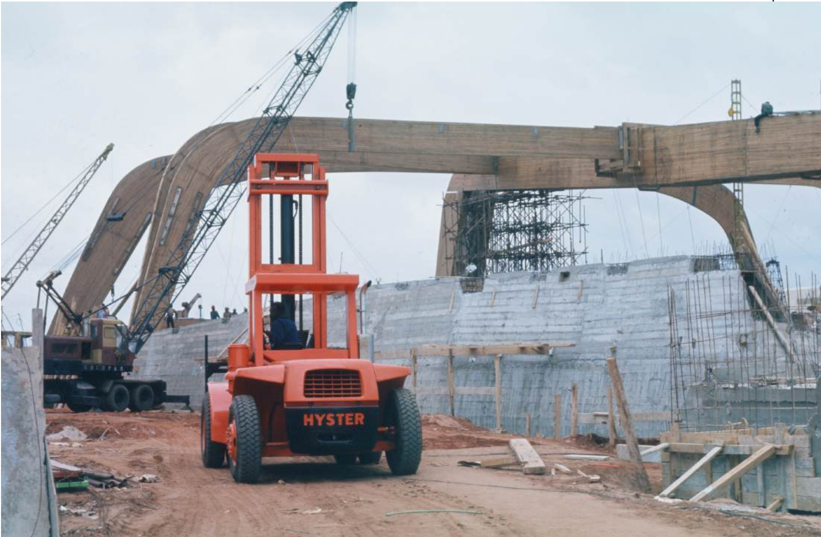
Fig.6: (A+B) The CICES auditorium under construction (personal archives of Marin, c. 1971-5).
