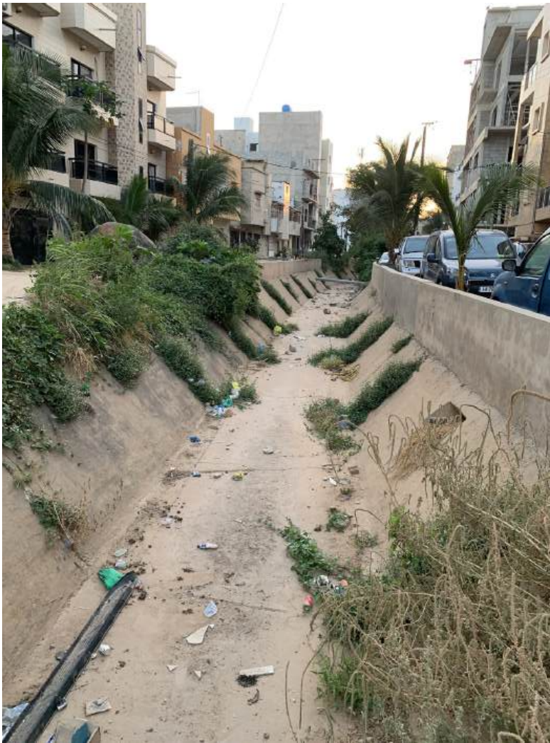
Fig.48: The original CICES drainage canal integrated into the CICES Foire neighbourhood (photo: Dana Salama, 2021).
