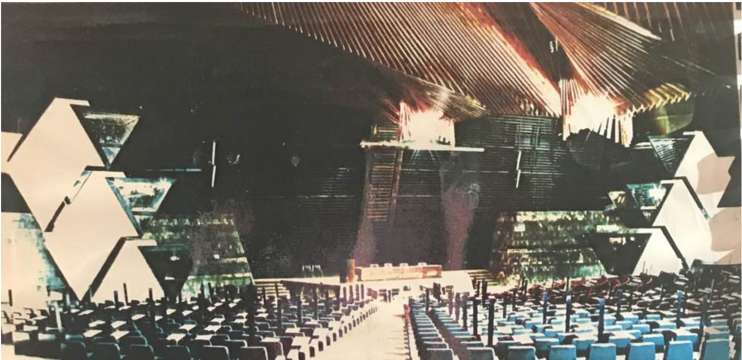
Fig.19: Photograph of the auditorium shell under construction c. 1971-5 (scan from an unknown magazine page).
