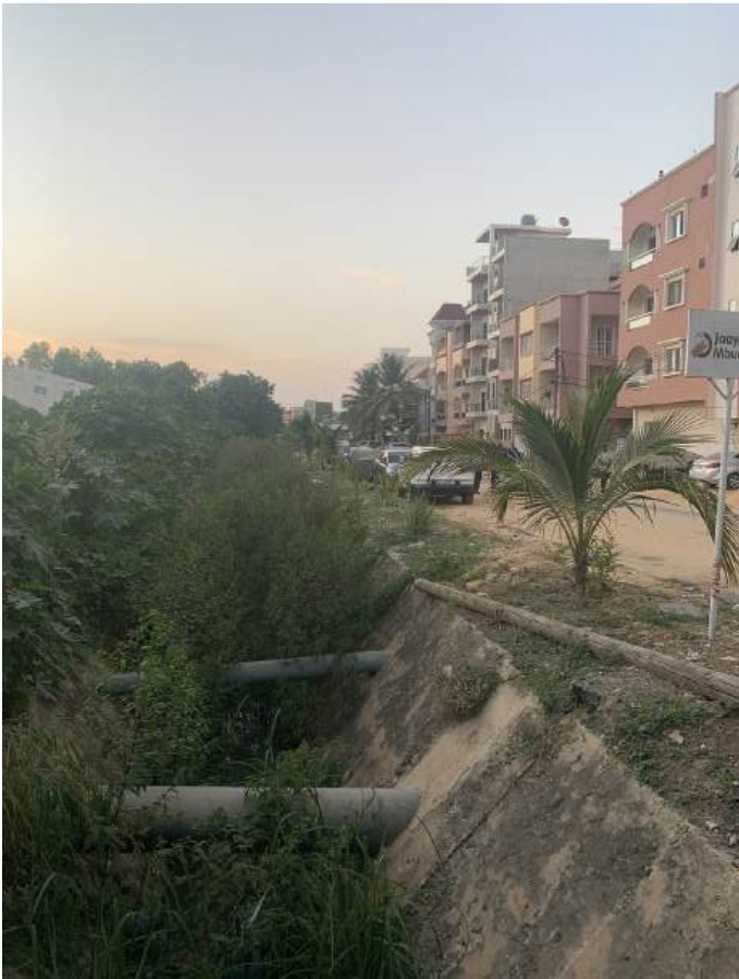
Fig.49: The drainage canal functions as a linear green park of sorts, with walkways alongside it and pedestrian bridges across (photo: Dana Salama, 2021).
