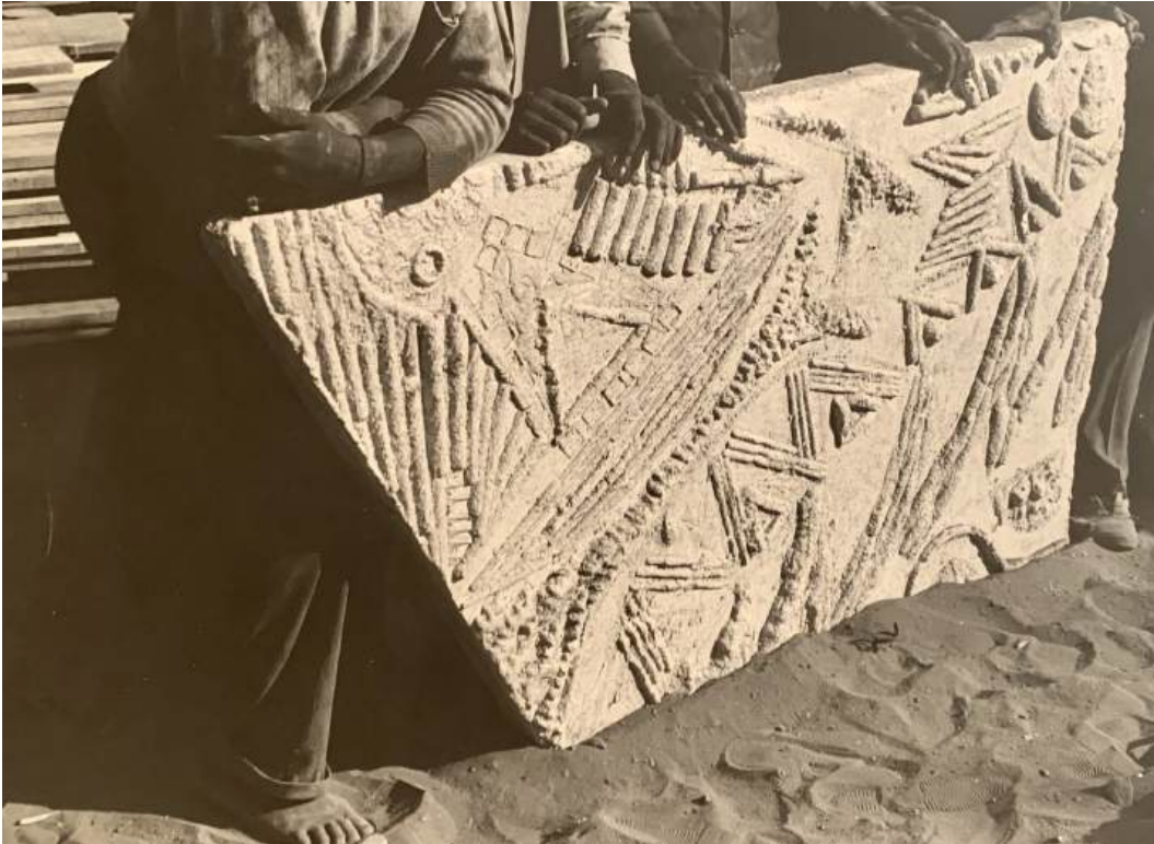
Fig.14: Workers holding a panel from the regional pavilions, created from a 1:1 styrofoam prototype (personal archives of Lamoureux, c. 1972-5).
