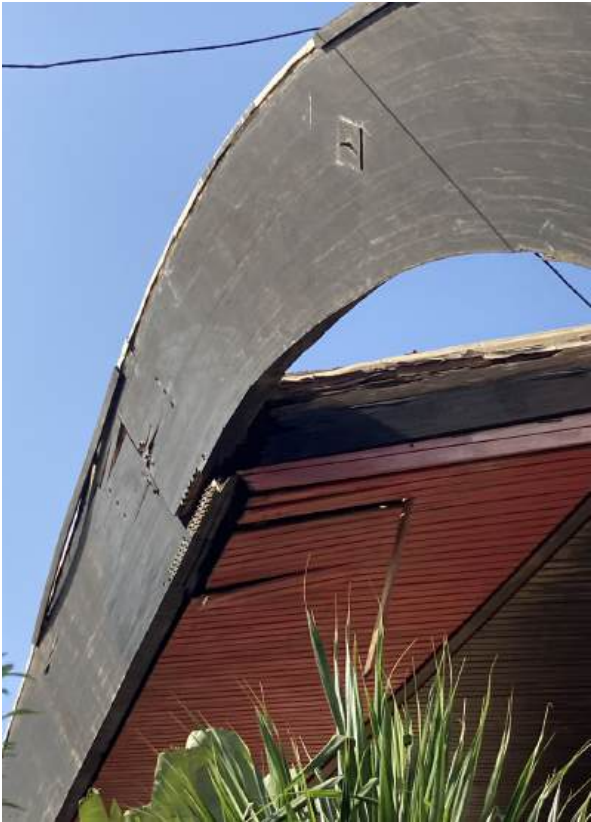
Fig.64: (top-right) the exterior glulam structural frame and wood cladding in the soffit splitting from the main structure due to corroding bolts causing deflection (photo: Dana Salama, 2021).
