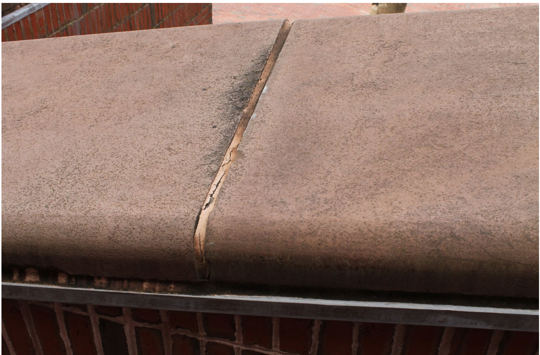
Brownstone with sealant mortar joint (May 23, 2018).
