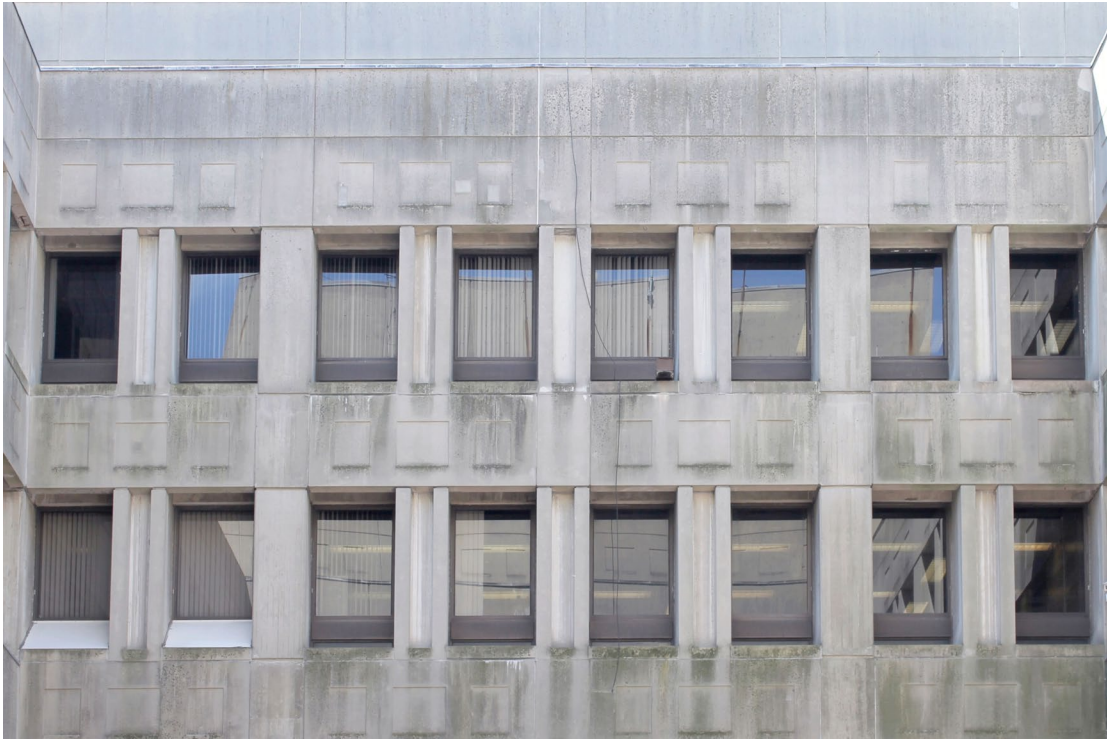
Courtyard at sixth and seventh floors, north-facing facade—representative soiling conditions on precast concrete sections (May 23, 2018).
