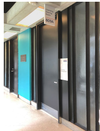
Entrance to the licensing hearing room showing newer hollow metal door and frame inserted into the mullioned interior storefront.
