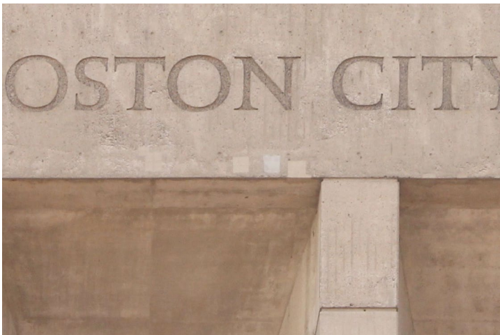
Example of poorly matched patches.
