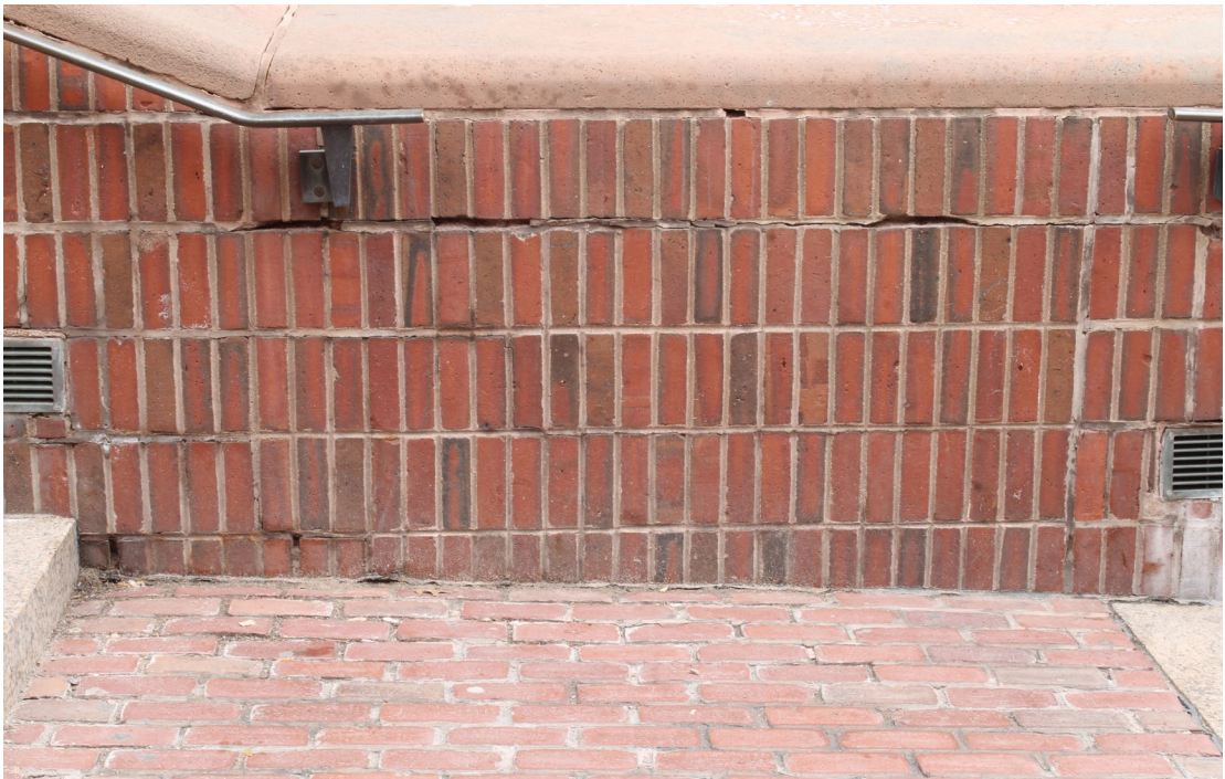
Failed mortar joints (January 11, 2021).
