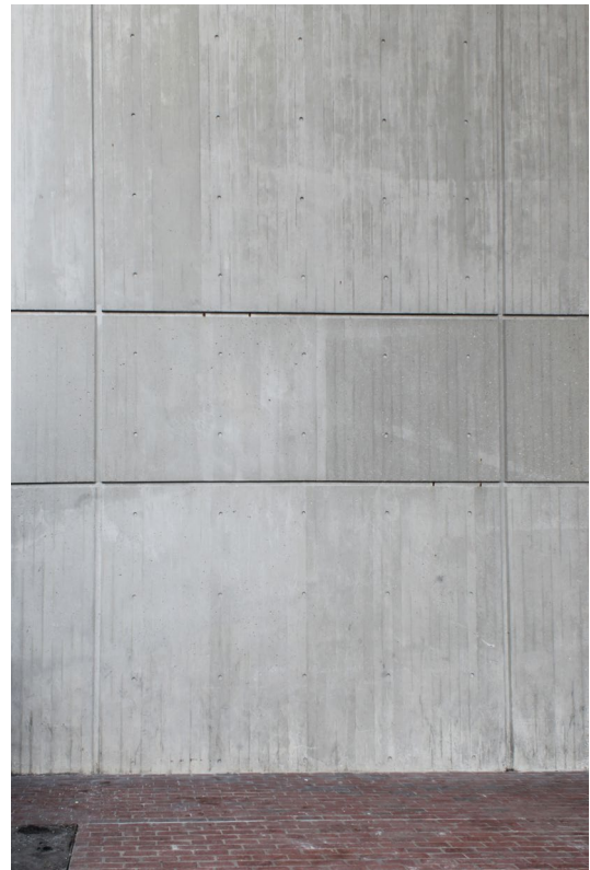
Sample of wall with filled form tie holes at the columns and partially filled tie holes in the field (January 11, 2021).
