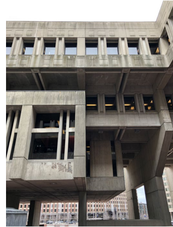
Spalling and organic staining.
