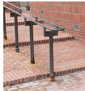
Rusting of railing attachment into the brick paving surface (May 23, 2018).
