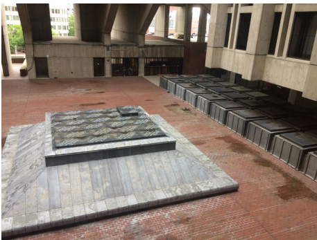
View of central skylight showing metal cladding and Grace I&W covering the top opening.
