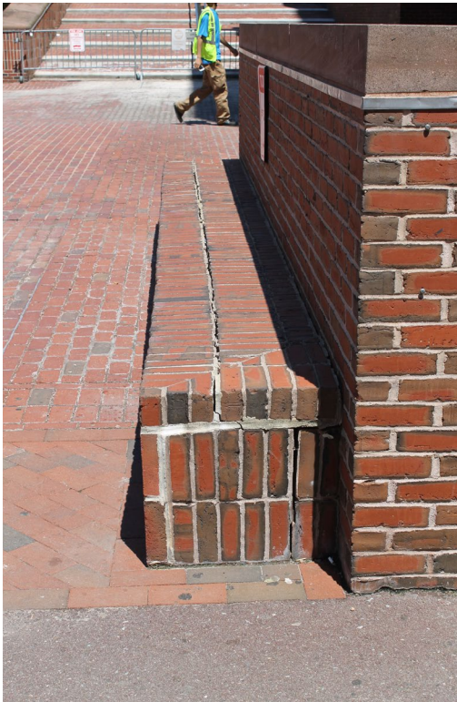
Top: General masonry failure adjacent to accessible ramp to the west entry (May 23, 2018).
