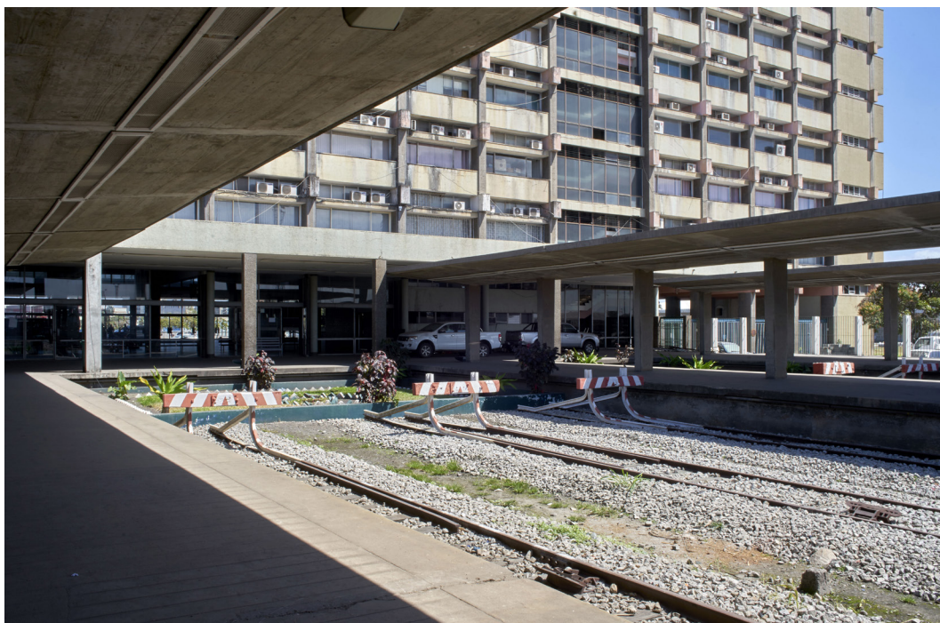
Figure 5.11 Air conditioners on the back elevation of the Beira Central Station (EM, 2019)
