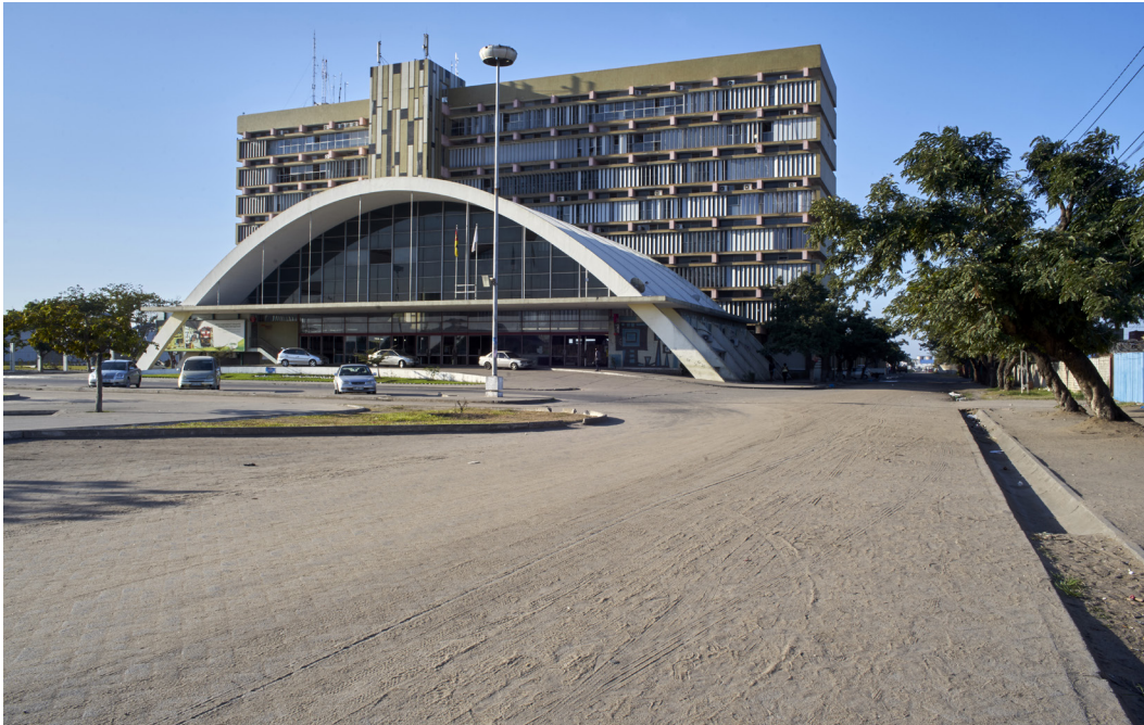
Figure 3.10 Beira Central Station, public atrium and administration blocks (EM, 2019)
