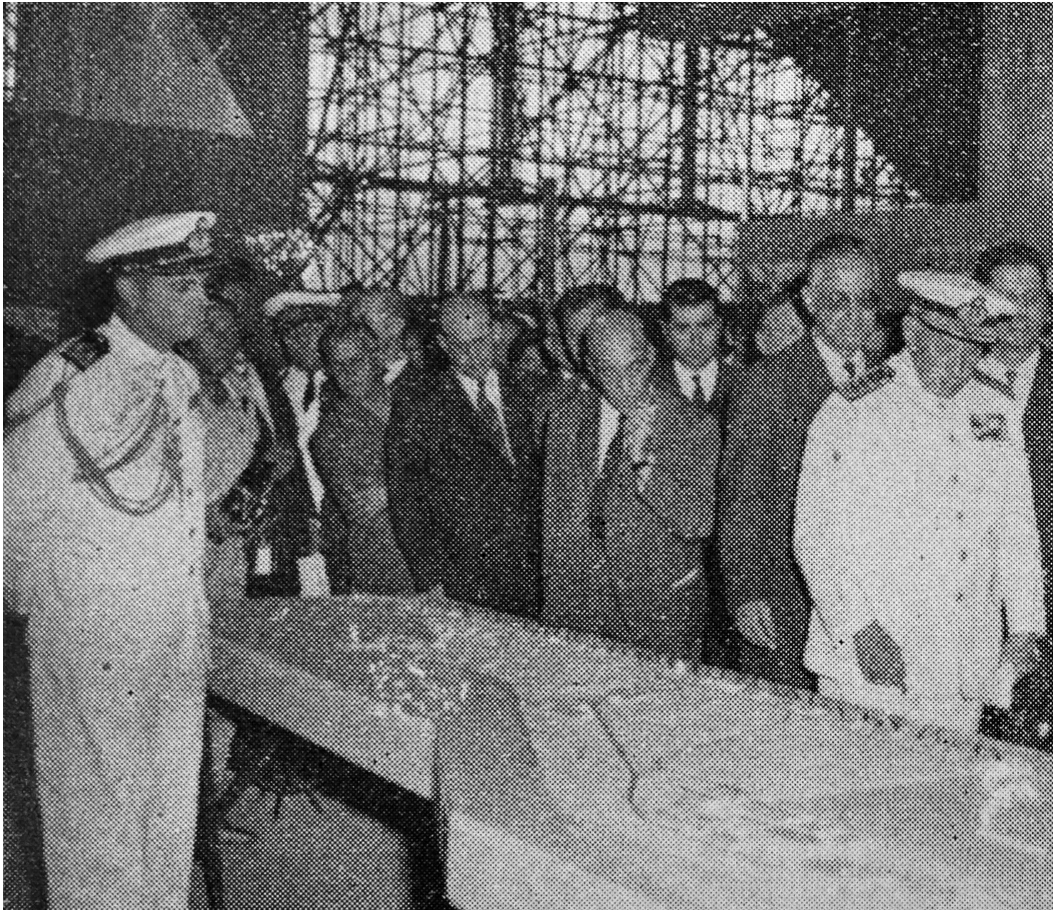
Figure 2.89 Exhibition of scale models in the passage atrium of the Beira Central Station under construction, July 1964 ( Boletim dos Portos, Caminhos de Ferro e Transportes de Moçambique , July 1964: 21 | MC-FM | EM, 2019).
