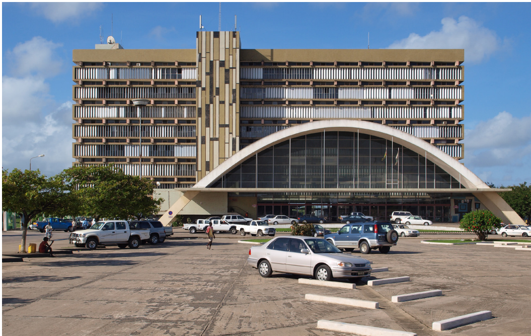
Figure 3.29 Beira Central Station, public atrium and administration blocks (EM, 2009)
