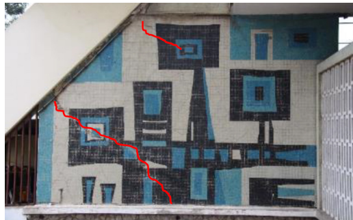
Figure 4.55 Vertical crack on a beam of the first floor of the administration block.
