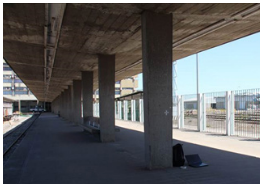
Figure 4.41 Locations selected for coring: column at the command building (location G).
