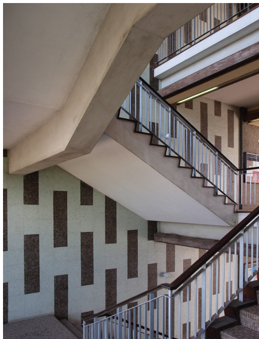
Figure 3.34 Beira Central Station, administration block, main staircase (EM, 2009)
