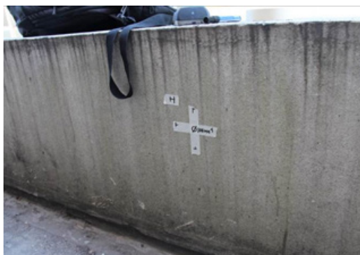
Figure 4.43 Locations selected for coring: beam protruding from the slab over the transition space (location I).
