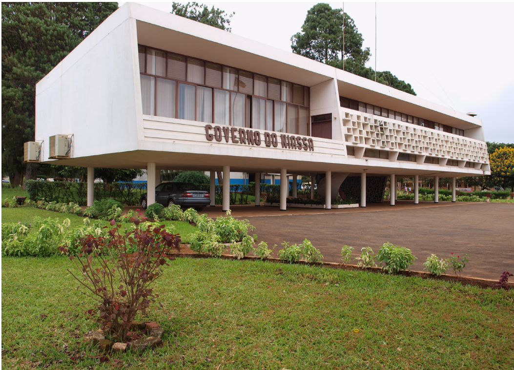
Figure 2.31 Administrative Offices, Vila Cabral (1959-1962) (EM, 2009).
