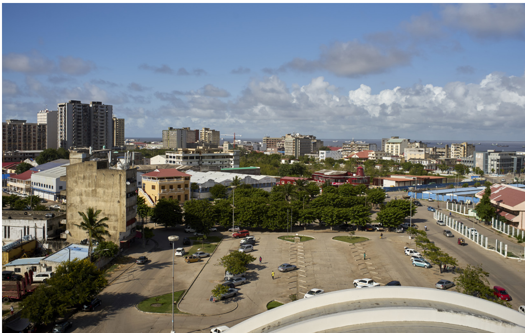
Figure 4.7 Frontal square from the Beira Central Station (EM, 2020)
