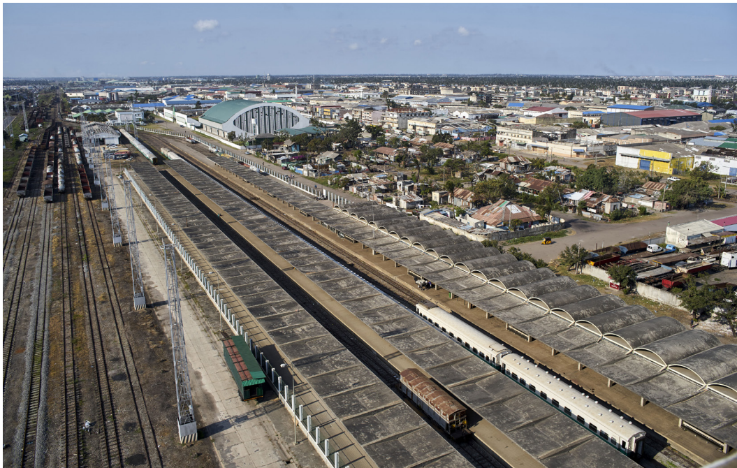
Figure 3.24 Beira Central Station, platforms area and command building (EM, 2019)
