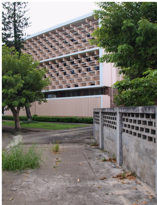
Figure 2.51 Megaza Building, Beira (1955-1959) (EM, 2009).
