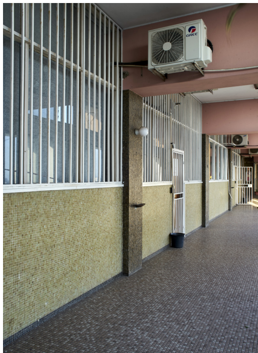
Figure 4.67 Closing of the glass fronts to the galleries of the administration block (EM, 2019).
