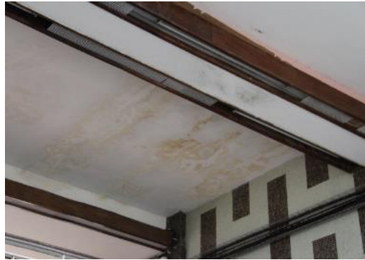
Figure 4.44 Bottom of concrete slab at the transition space between the administration building and platforms' area.
