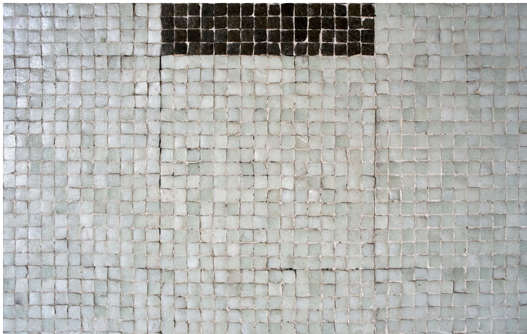
Figure 3.44 Beira Central Station, vitreous mosaic coating detail (EM, 2019)
