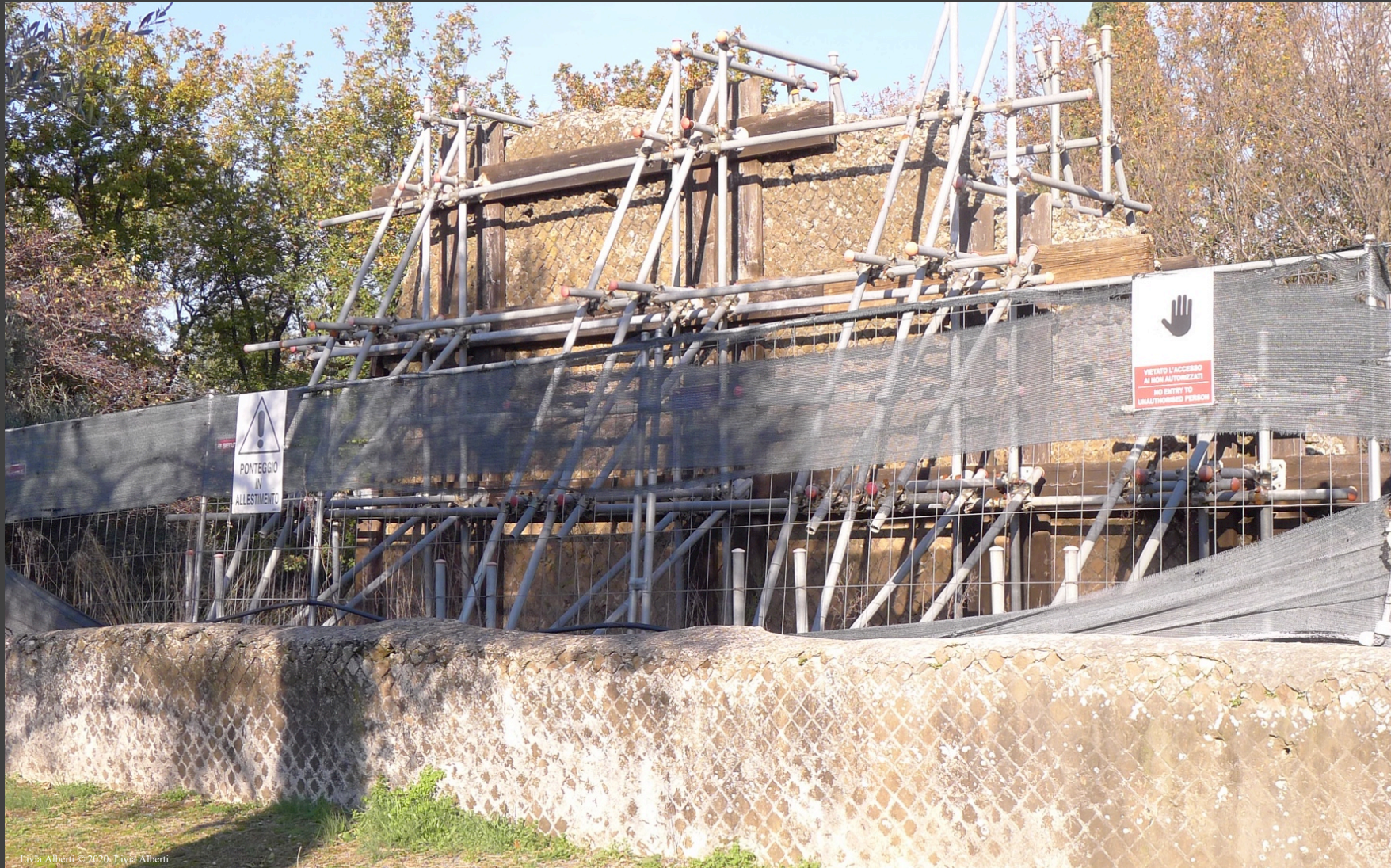
Temporary metal structure buttress
