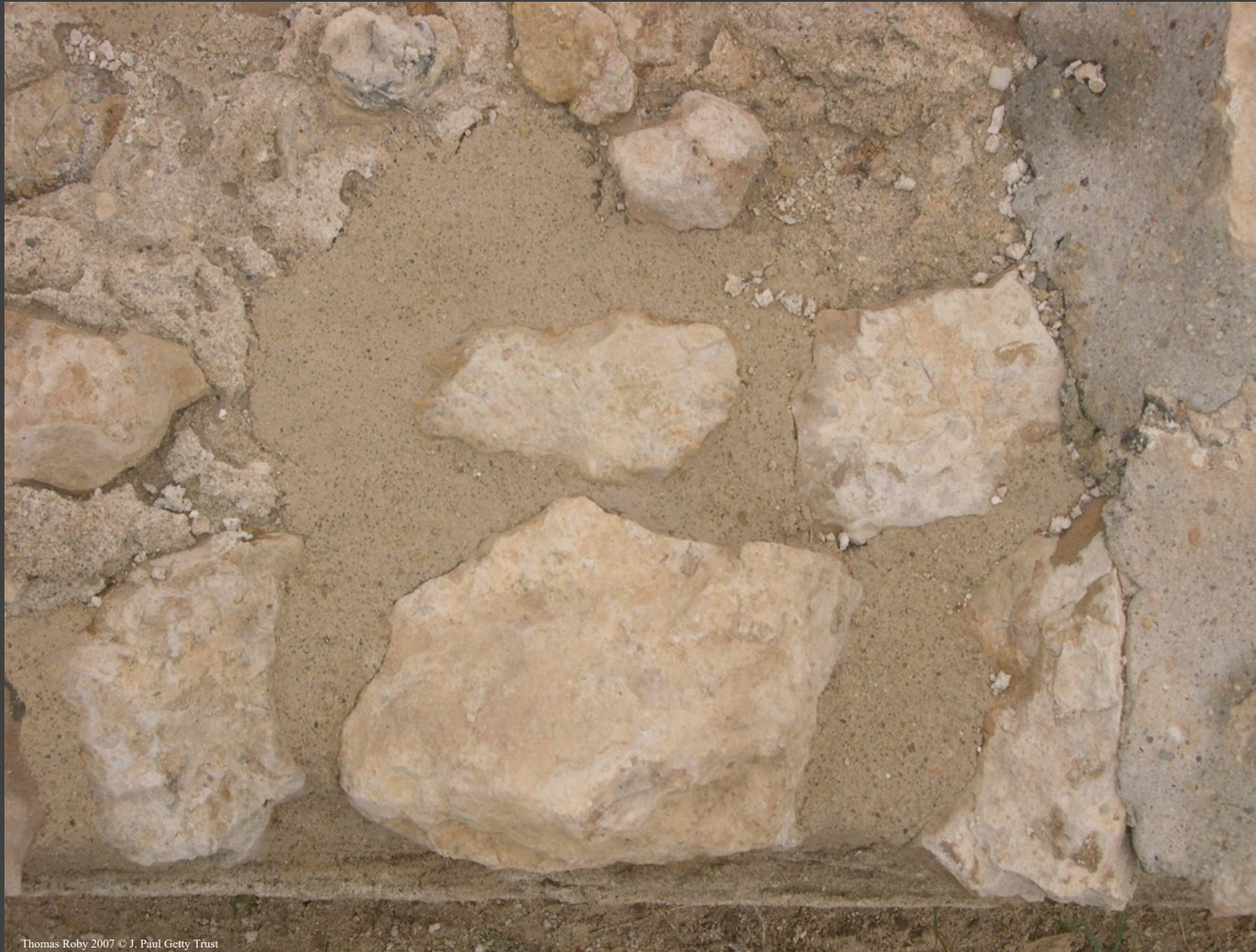
Infilling of lacunae with stones and mortar
