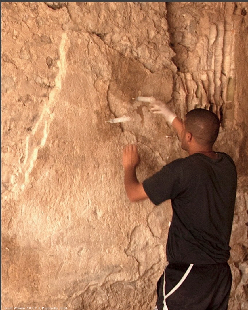
Grouting voids between preparatory layers
