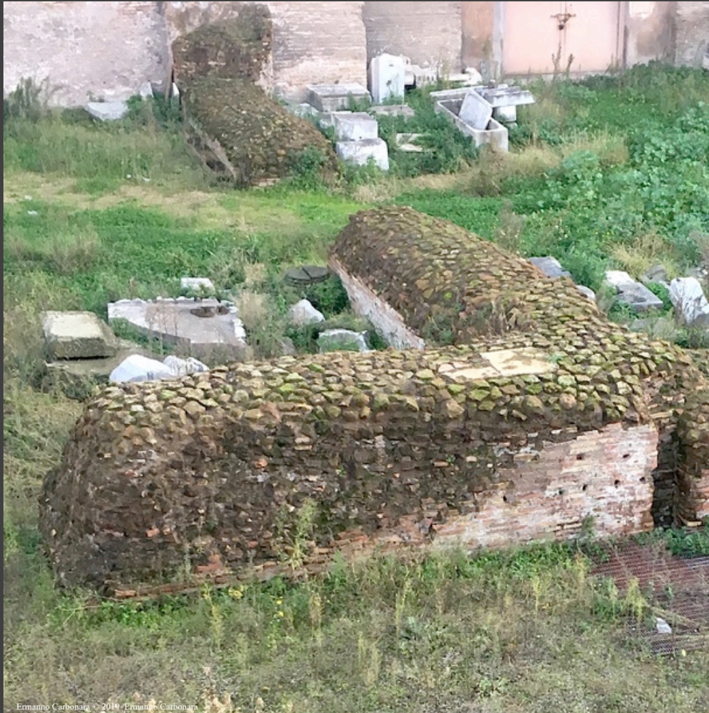
Wall capping using a layer of mortar and small stones
