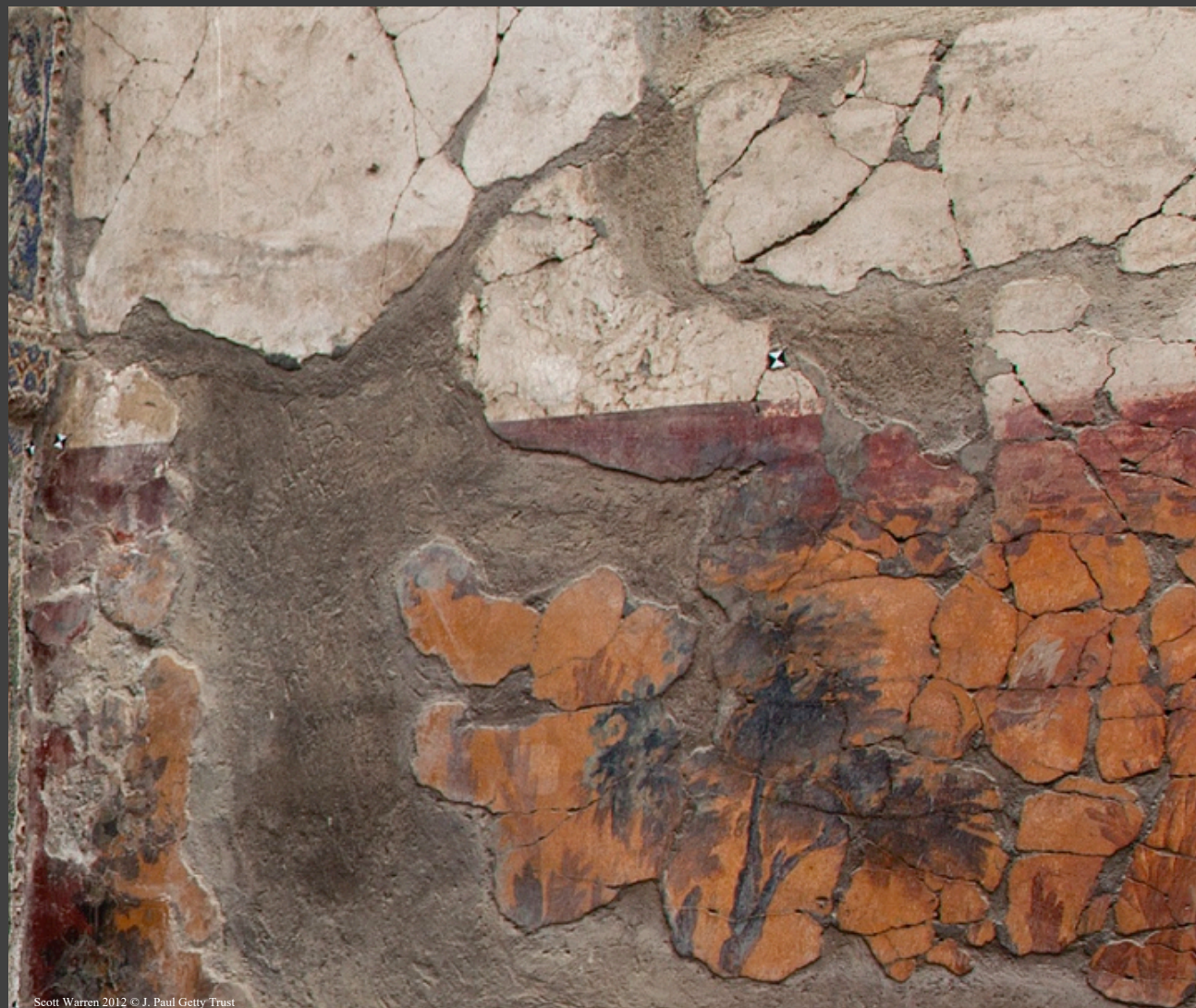
Recognizable integration below the original surface level
