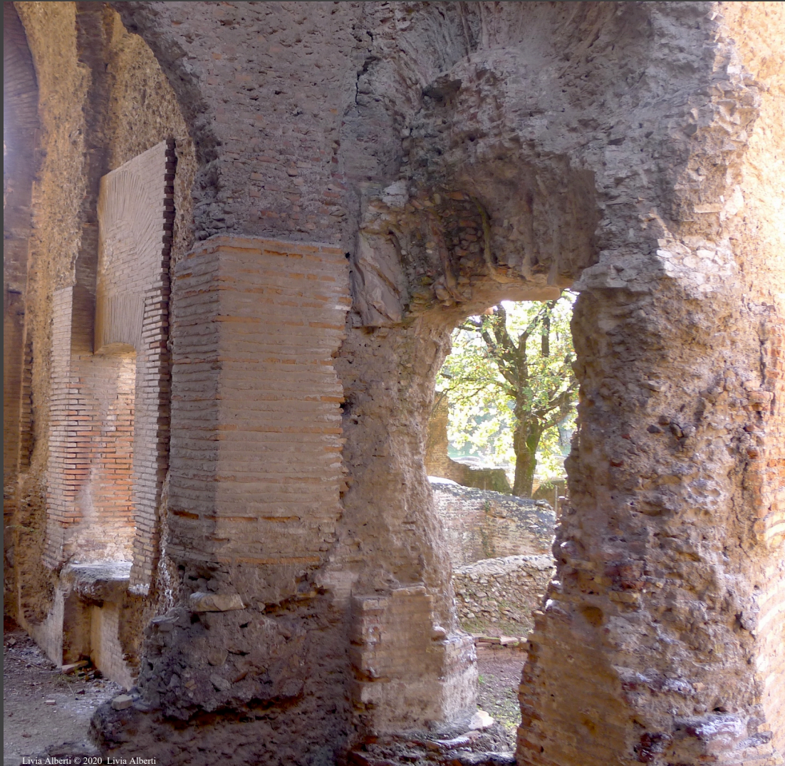
Reinforcement with masonry
