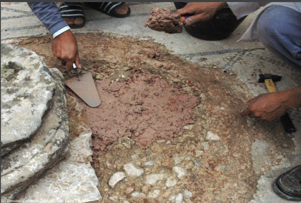
Applying the first layer of mortar
