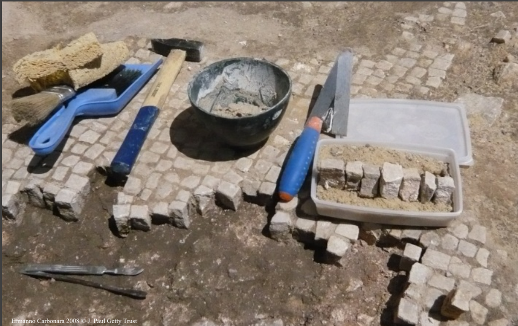
Temporarily removing detached tesserae to a bedding of sand
