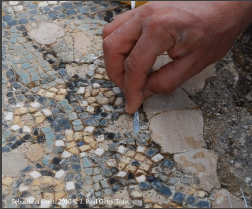
Filling of interstices with mortar
