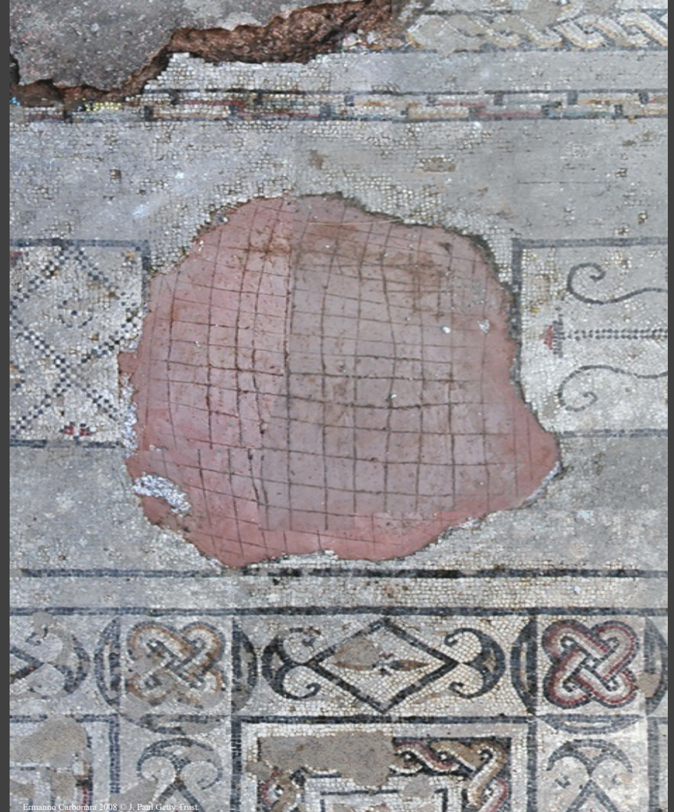
Treatment of the surface for good attachment to the second layer
