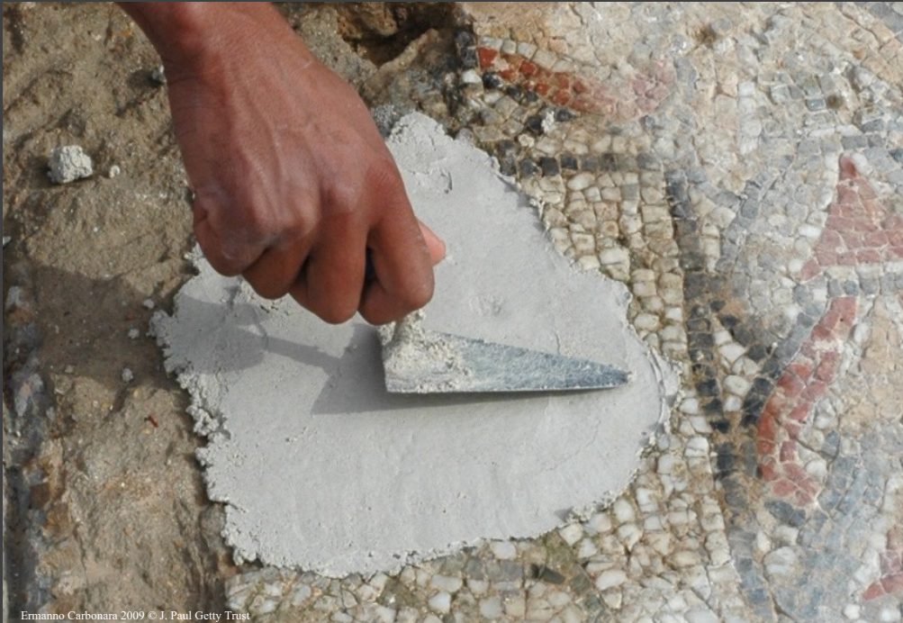
Application of surface layer of mortar
