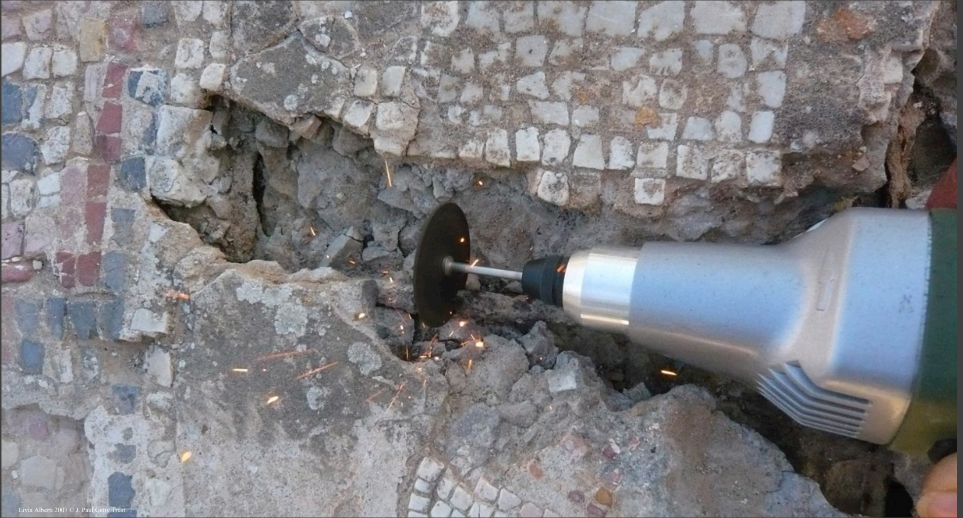
Cutting the steel bar
