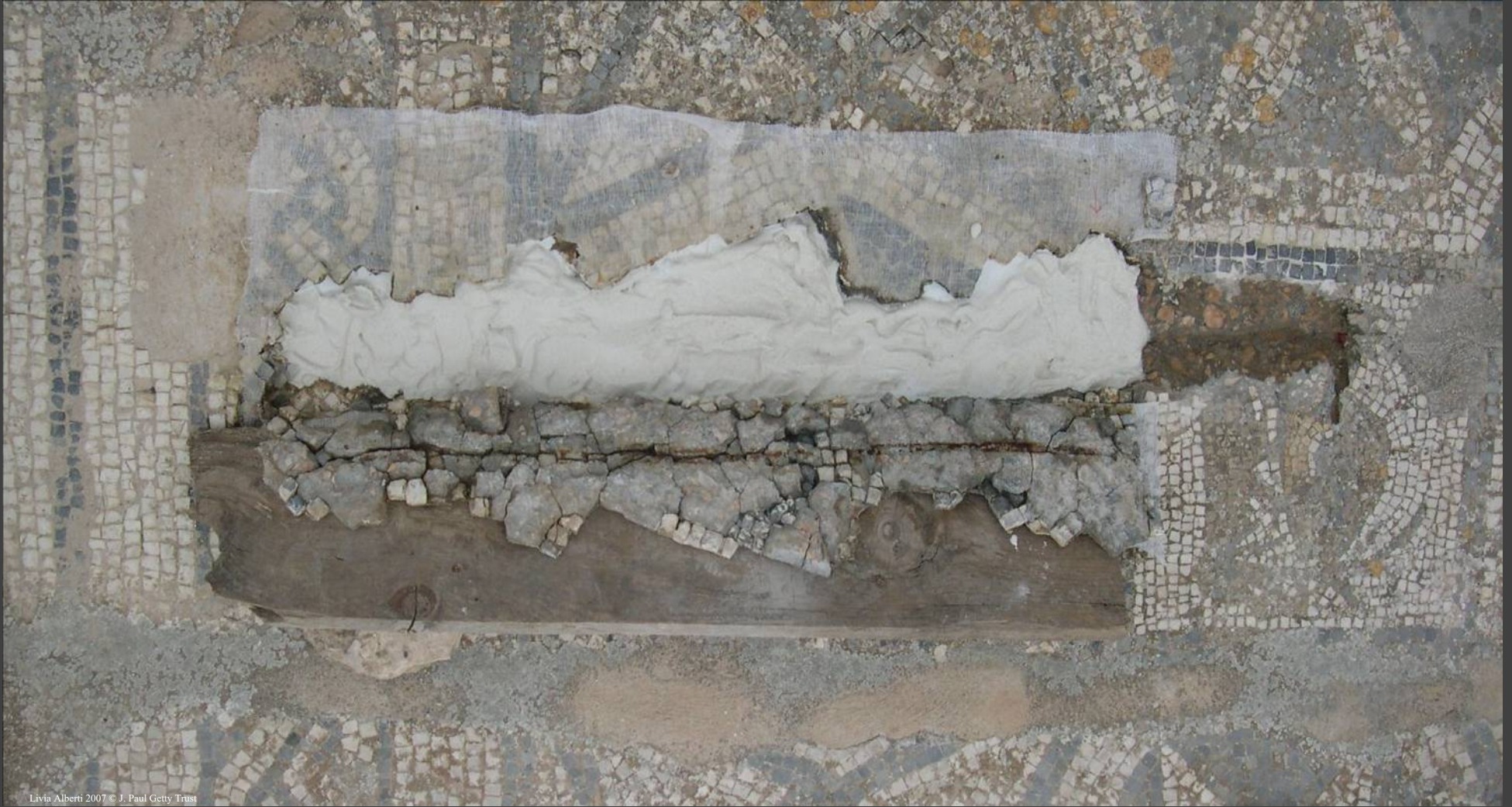
Filling with mortar the space left by the removed bar and concrete debris
