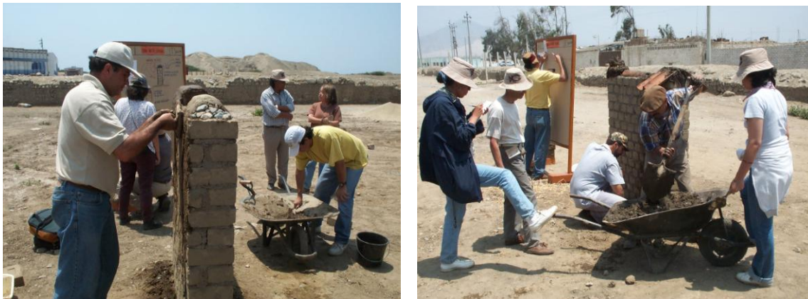
Figure 5.2.3 (left) and 5.2.4 (right) PAT students capping test walls with different methods PAT course, 1999 © J. Paul Getty Trust
