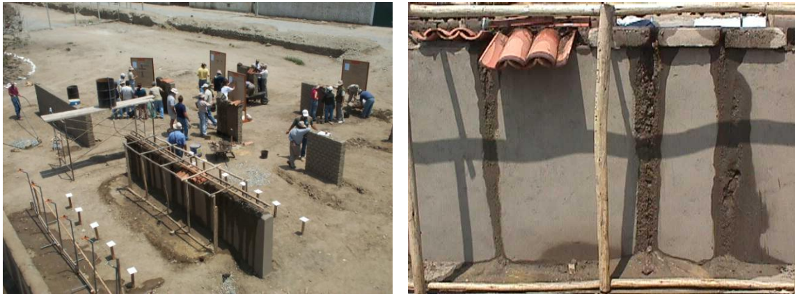
Figure 5.2.1 (left) and 5.2.2 (right) Left: View of demonstration walls for capping and rendering Right: Capping demonstration wall after accelerated weathering PAT course, 1999 © J. Paul Getty Trust
