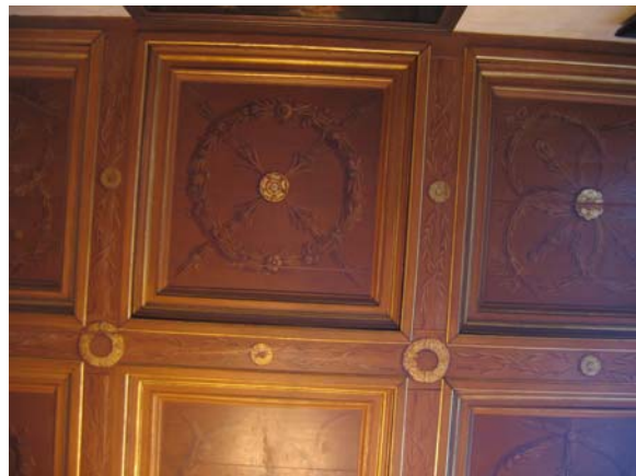
The Sael and the wooden ceiling (showing a crack in the lower panel) (photo: ICN)
