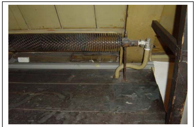
Heating at the base of the fixed church benches (photo: TU/E)
