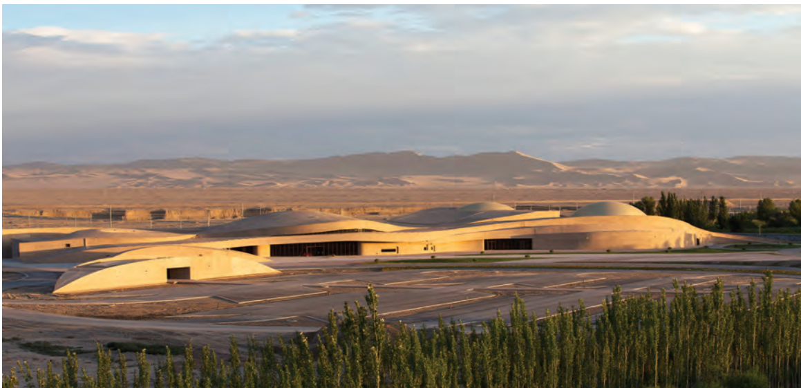
Fig. 2. View of the Mogao Grottoes visitor center during final construction.
