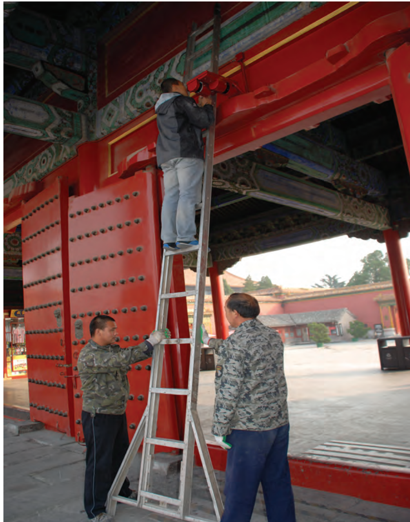
Figure 5. Installing visitor monitoring system in 2013.
