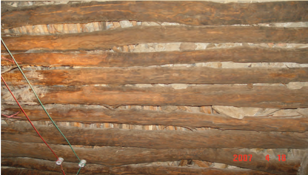
Fig. 5. The traditional wooden structure of the Potala Palace must bear enormous loads as a result of the increase in visitors.
