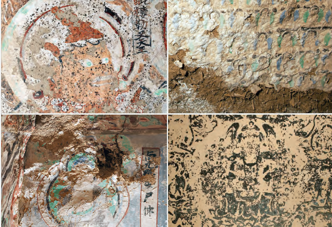
Fig. 3. Deterioration conditions of wall paintings include mold, flaking, detachment, disruption, and color loss.
