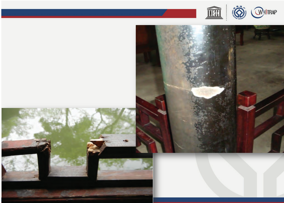
Fig. 7. Architectural elements in the gardens damaged due to excessive visitation.
