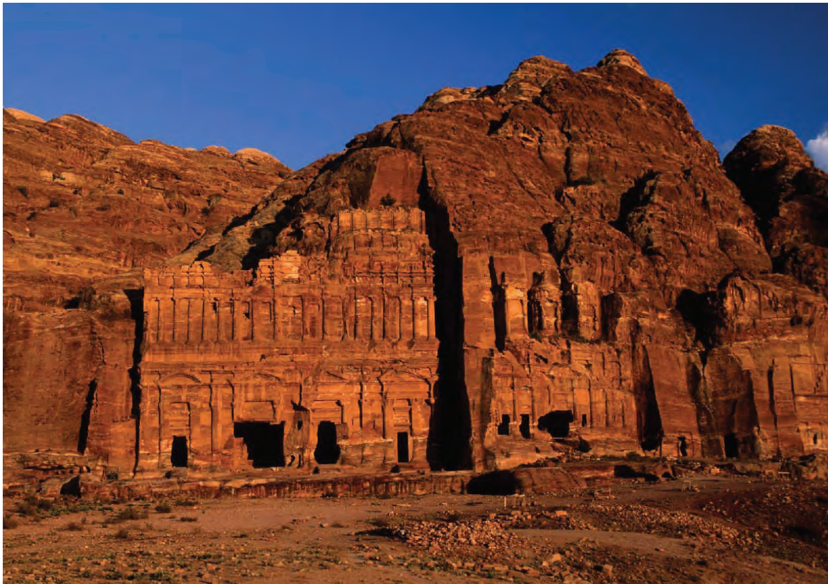
Fig. 4. The Royal Tombs, seen here are among the best preserved at Petra, but display the characteristic 'key-hole' deterioration at ground-level entrances. This is produced by salt-laden flood waters that are absorbed by the sandstone from which the tombs are caved.
