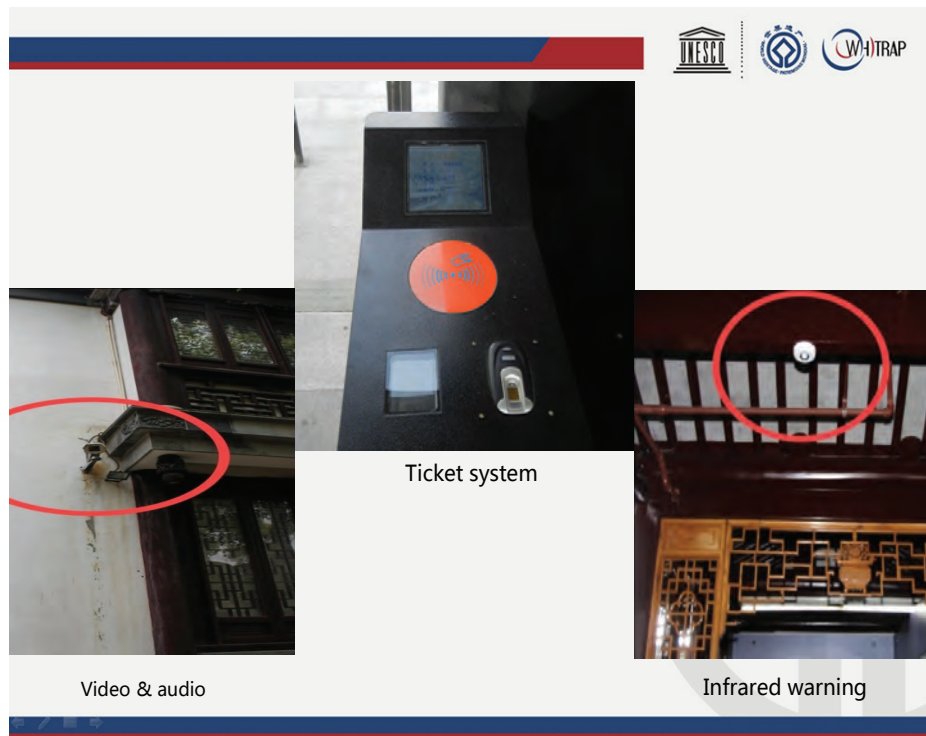
Fig. 9. Equipment installed in the gardens to improve visitor management includes video and audio monitoring system, automated ticket checking system, and infrared warning system.
