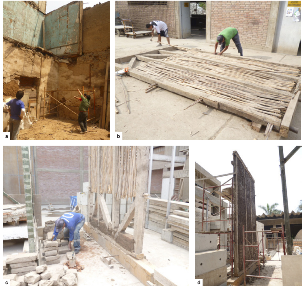
FIGURE 4.8. Construction of original quincha test sample panel: (a) original quincha panel in existing location (second floor of Hotel El Comercio); (b) reassembly of panel; (c) insertion of masonry infill at citara base; (d) panel prior to mud plaster finish, with mud mortar over canes and complete infill at base.
