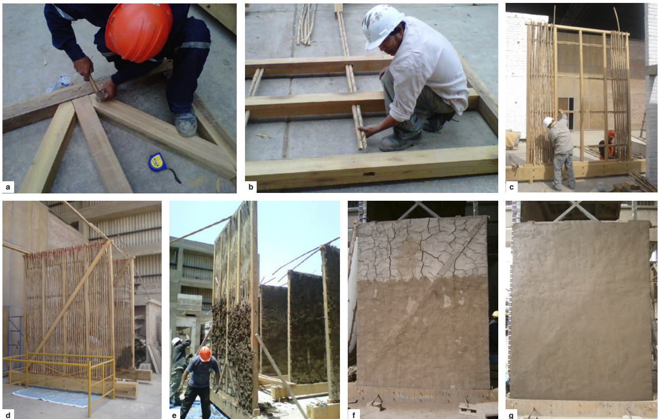
FIGURE 4.7. Construction of new quincha test sample panel: (a) fastening of the citara (diagonal element at base), representative of the second-floor structure (MA); (b) insertion of transversal canes into posts; (c, d) construction of third-floor panel (MB) with diagonal timber element; (e) infilling of the panel (MA) with mud mortar; (f) quincha panel showing shrinkage cracks in the first layer of mud plaster; (g) quincha panel after application of a second layer of mud plaster.
