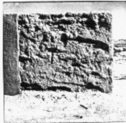
Example of Serious Erosion (2W1)
