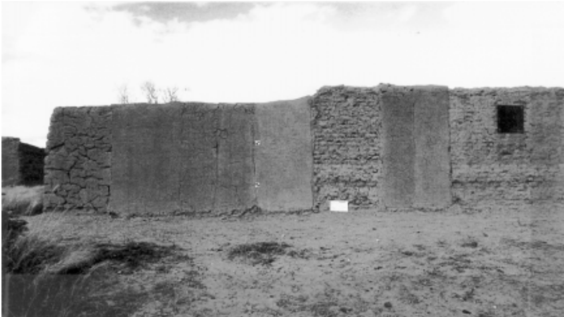
Figure 6. The 1997 appearance of protective coating test panels 1-6, which were applied to historic walls in 1992. Panel 1, the control, is at the left end and panel 6 is at the right end. This photograph is of the south face of the south wall of Features 16 and 17.
