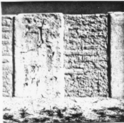
Example of Moderate Erosion (2E7)
