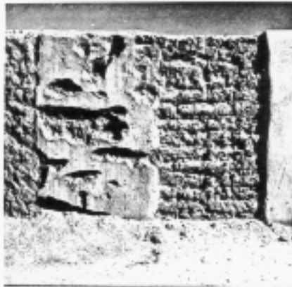
Example of Very Serious Erosion (2W12)
