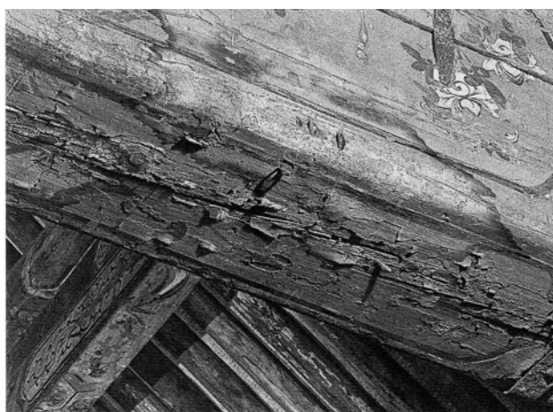
Figure 7 Ground-facing surface of a main beam from the palace hall illustrating the flaking and loss of paint.
