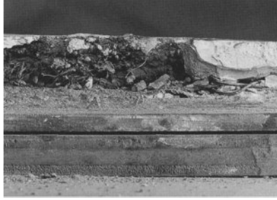
Figure 3 Bearer of Good Wishes (shown in Fig. 2), cross-sectional detail of original rendering layers and added modern support layers prior to conservation.
